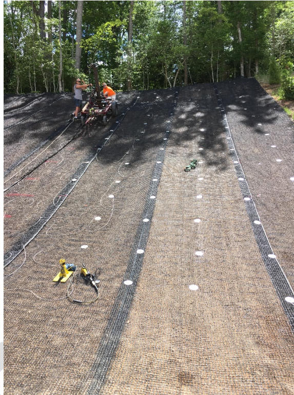
Figure 5 – ARGS Installation
