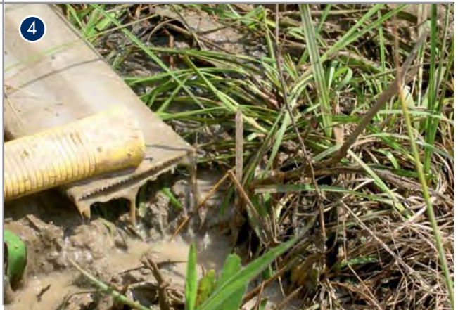
Drive Plati-Drain® into optimum position
