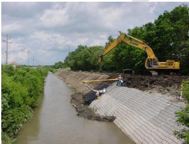
Figure 6 – Articulated Concrete Block (ACB) Revetment System
