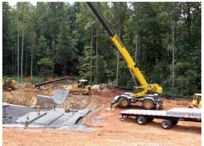
The use of a crane is optimal for fast and safe unloading and installation of the mats.
