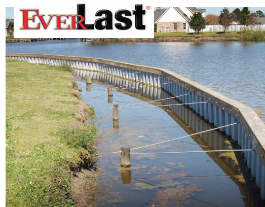
A water jet is often used to drive the vinyl piling into granular soil. In the above photo, you see a drive guide is used which provides a firm surface to drive the sheets plumb and straight.
