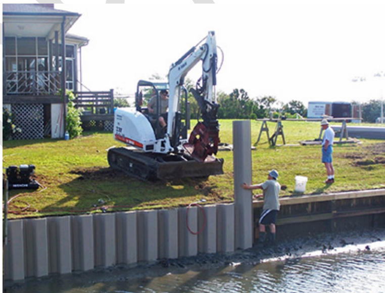
Figure 7 - Synthetic Sheet Piling Wall Installation
