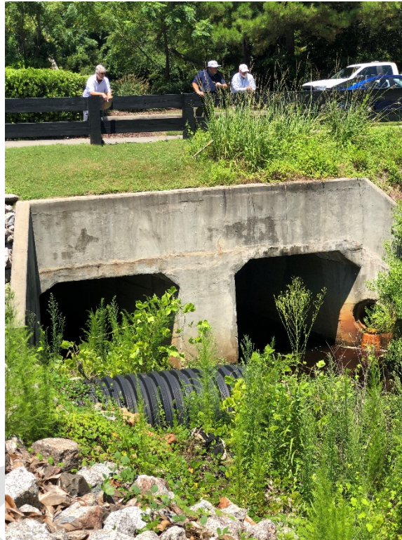
Figure 10 - Existing Culverts under Barefoot Resort Bridge Road
