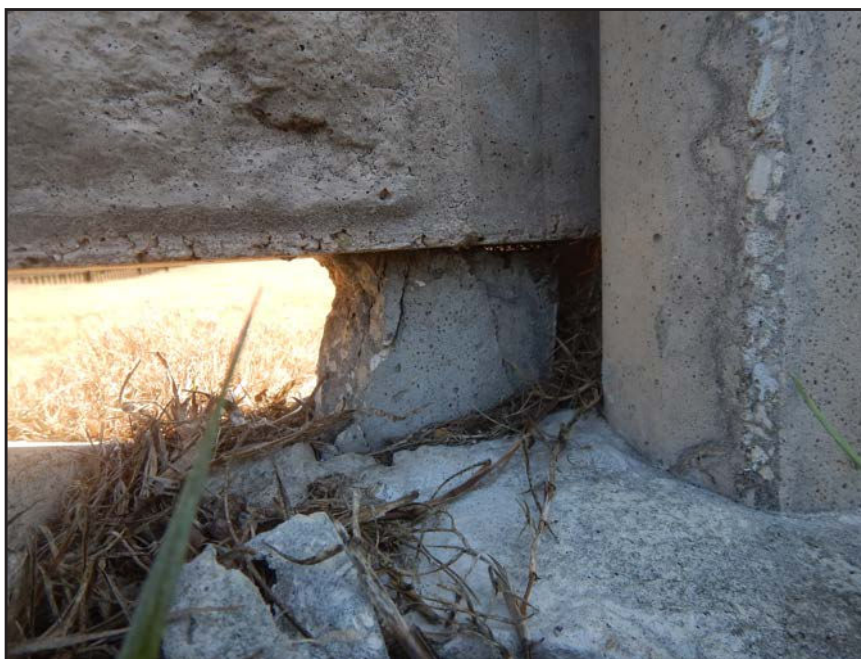
NO. 135 - COLUMN 58S - INADEQUATE BEARING OF A PRECAST WALL PANEL ON A FAILED GROUT PEDESTAL OR A FAILED PRECAST TONGUE
