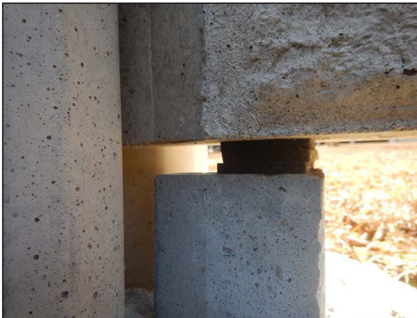
NO. 81 - COLUMN 3SM - INADEQUATE BEARING OF A PRECAST WALL PANEL ON A 2" x 2" NEOPRENE BEARING PAD
