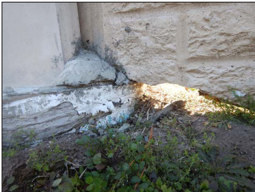
NO. 118 - COLUMN 11NM - INADEQUATE BEARING OF A PRECAST WALL PANEL ON A FAILED GROUT PEDESTAL OR A FAILED PRECAST TONGUE
