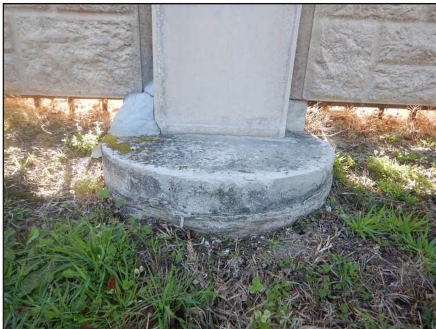
NO. 112 - COLUMN 45N - INADEQUATE BEARING OF A PRECAST WALL PANEL ON A FAILED GROUT PEDESTAL OR A FAILED PRECAST TONGUE
