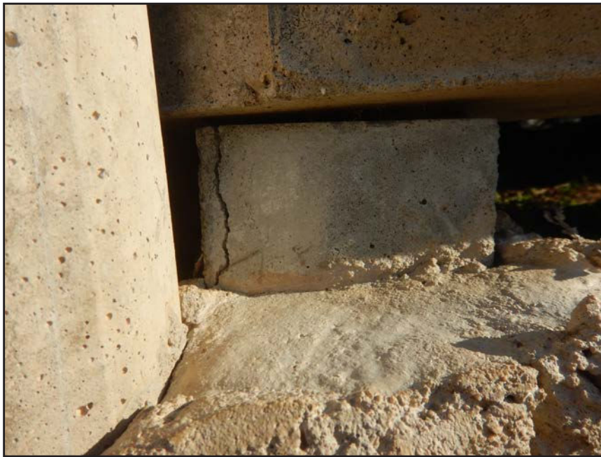
NO. 160 - COLUMN 13SS - INADEQUATE BEARING OF A PRECAST WALL PANEL ON A FAILED GROUT PEDESTAL OR A FAILED PRECAST TONGUE
