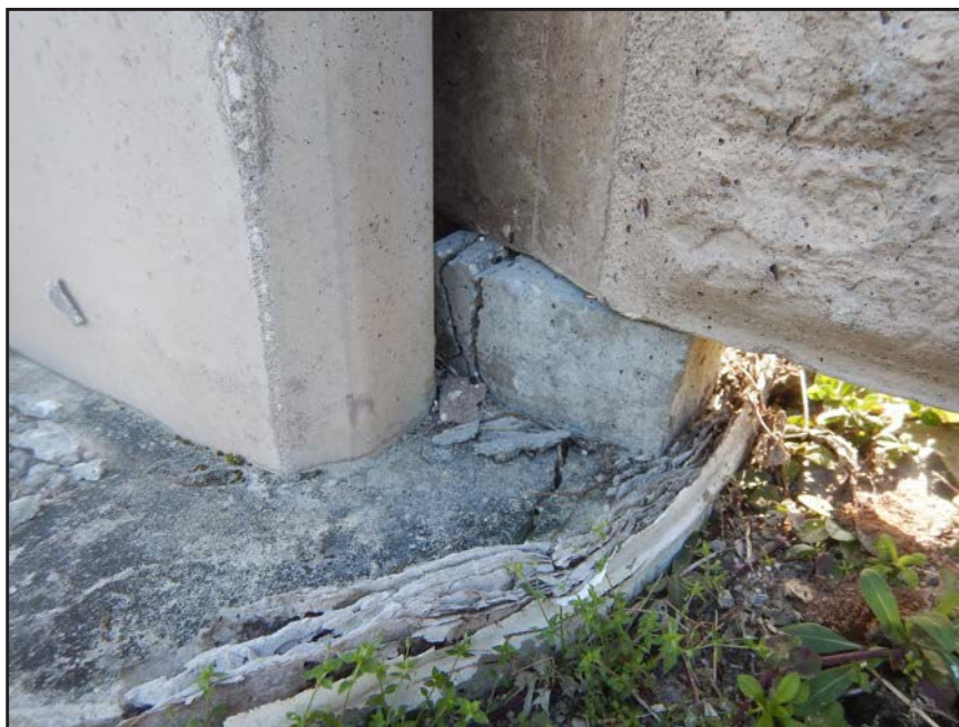
NO. 119 - COLUMN 12NM - INADEQUATE BEARING OF A PRECAST WALL PANEL ON A FAILED GROUT PEDESTAL OR A FAILED PRECAST TONGUE
