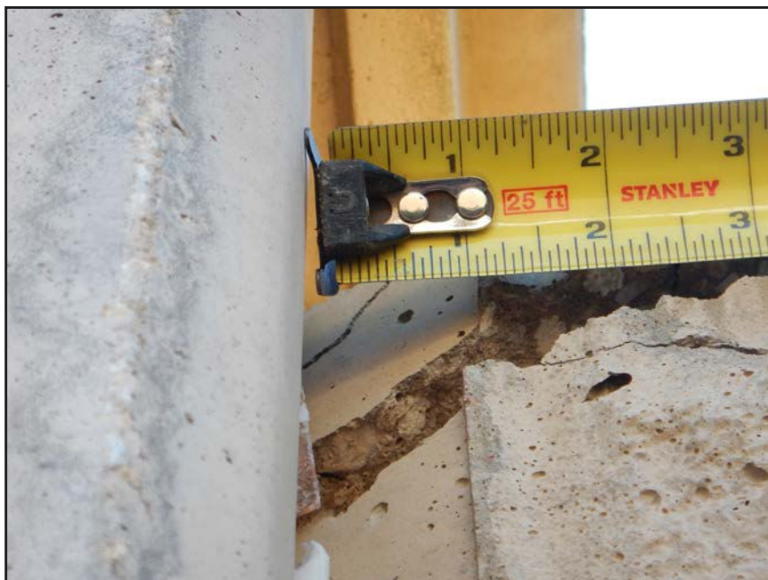
NO. 6 - COLUMN 13NM - DROPPED PRECAST PANEL WITH A 1" GAP AT THE TOP AND A 2 7/8" GAP AT THE BOTTOM
