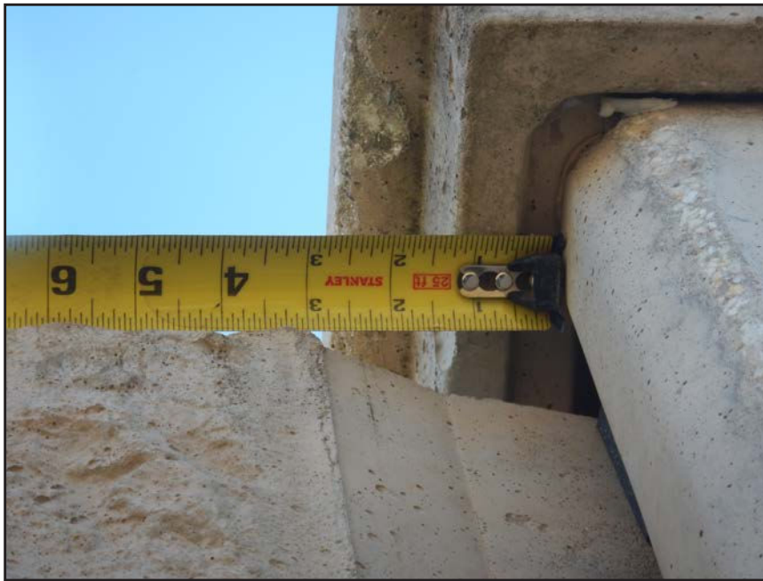
NO. 232 - COLUMN 58S - INSUFFICIENT SEATING OF A PRECAST WALL PANEL IN A PRECAST COLUMN
