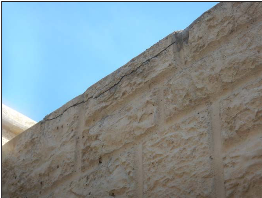
NO. 466 - COLUMN 17S - CRACKED AND SPALLED PRECAST CONCRETE
