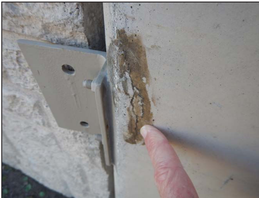
NO. 424 - COLUMN 14N - INADEQUATE ADDED CLIP ANGLE CONNECTION AT A DEFICIENT WALL PANEL TO COLUMN CONNECTION
