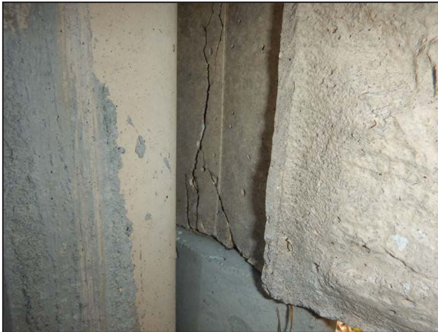
NO. 322 - COLUMN 19S - CRACKED AND FAILED TONGUE OF A PRECAST WALL PANEL IN A PRECAST COLUMN
