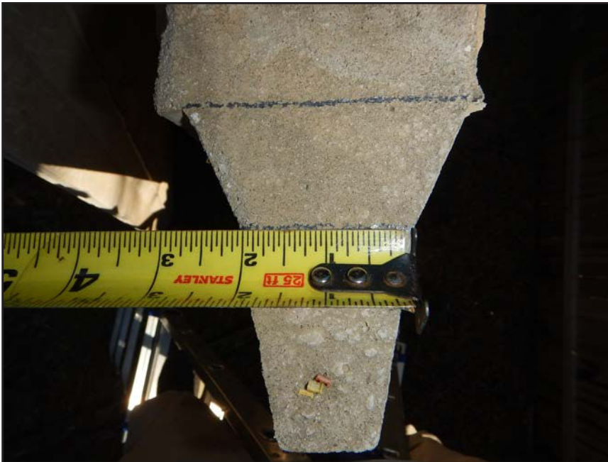
NO. 27 - STORED EXCESS WALL PANELS - TYPICAL TONGUE DIMENSIONS
