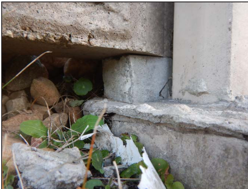
NO. 178 - COLUMN 65SS - INADEQUATE BEARING OF A PRECAST WALL PANEL ON A FAILED GROUT PEDESTAL OR A FAILED PRECAST TONGUE
