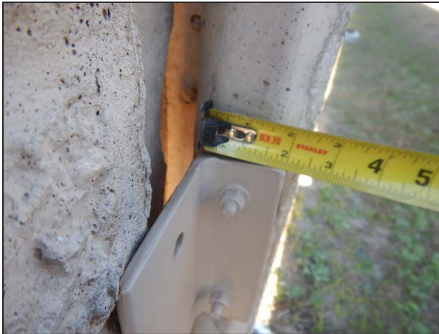
NO. 441 - COLUMN 50N - INADEQUATE ADDED CLIP ANGLE CONNECTION AT A DEFICIENT WALL PANEL TO COLUMN CONNECTION
