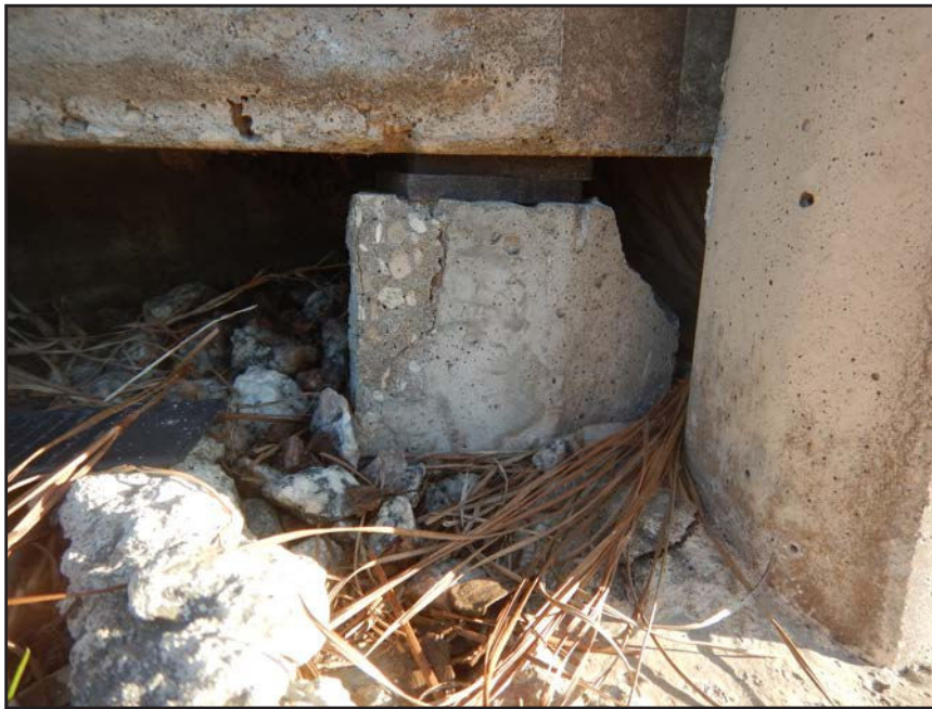
NO. 168 - COLUMN 32SS - INADEQUATE BEARING OF A PRECAST WALL PANEL ON A FAILED GROUT PEDESTAL OR A FAILED PRECAST TONGUE
