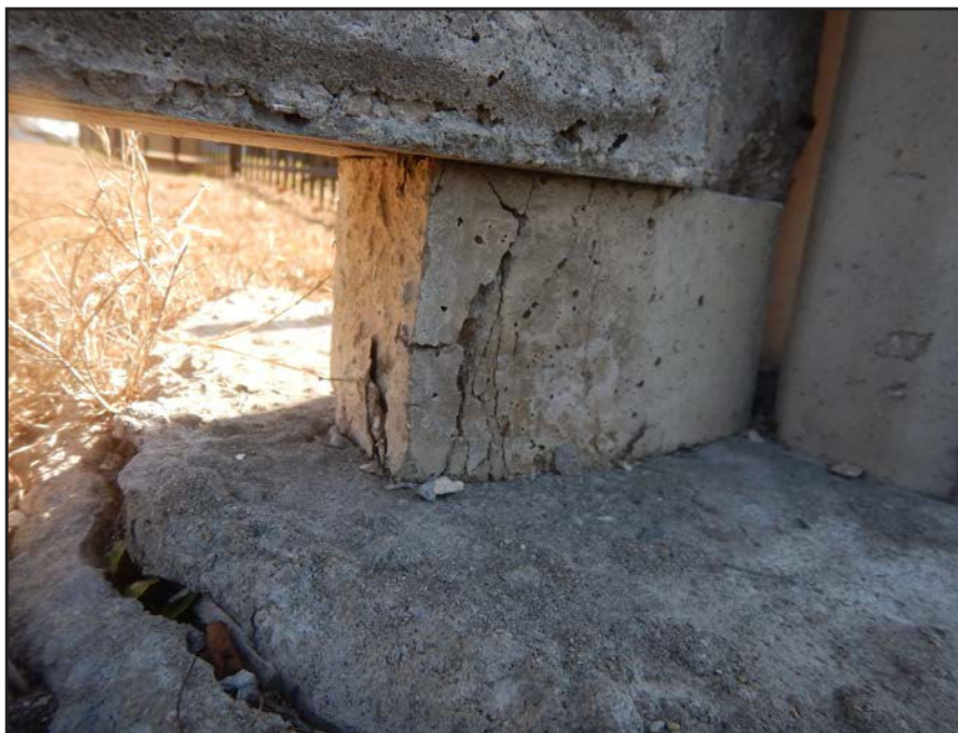
NO. 134 - COLUMN 55S - INADEQUATE BEARING OF A PRECAST WALL PANEL ON A FAILED GROUT PEDESTAL OR A FAILED PRECAST TONGUE
