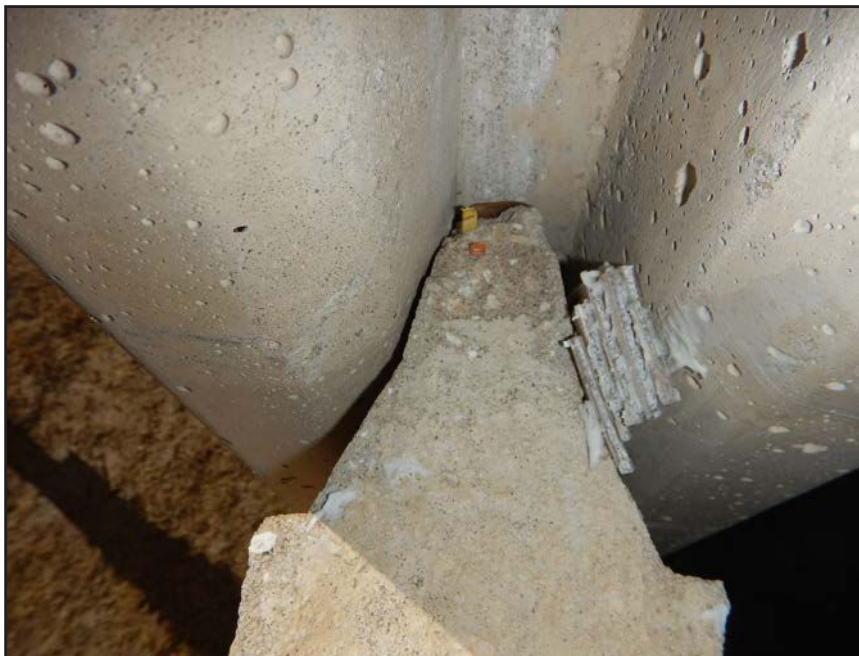
NO. 22 - COLUMN 22N - FIELD MEASURED COLUMN AND WALL PANEL TONGUE
