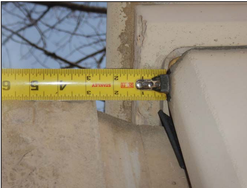
NO. 261 - COLUMN 80SS - INSUFFICIENT SEATING OF A PRECAST WALL PANEL IN A PRECAST COLUMN
