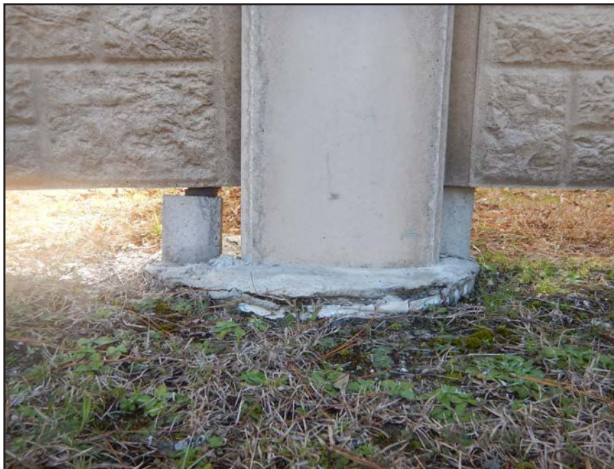
NO. 74 - COLUMN 14NM - INADEQUATE BEARING OF A PRECAST WALL PANEL ON A 2" x 2" NEOPRENE BEARING PAD
