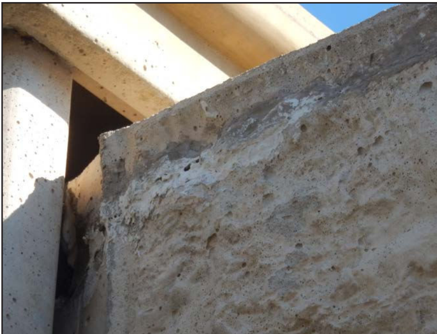
NO. 469 - COLUMN 52S - CRACKED AND SPALLED PRECAST CONCRETE
