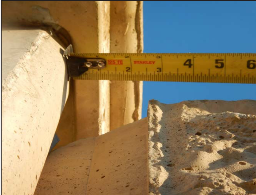
NO. 254 - COLUMN 46SS - INSUFFICIENT SEATING OF A PRECAST WALL PANEL IN A PRECAST COLUMN
