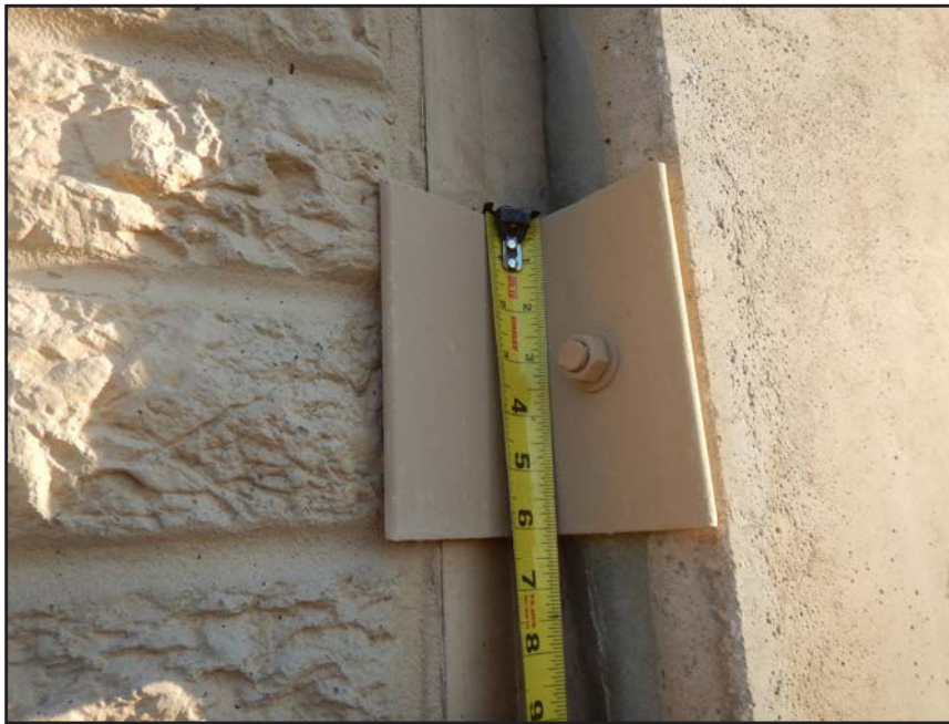
NO. 454 - COLUMN 41SS - INADEQUATE ADDED CLIP ANGLE CONNECTION AT A DEFICIENT WALL PANEL TO COLUMN CONNECTION
