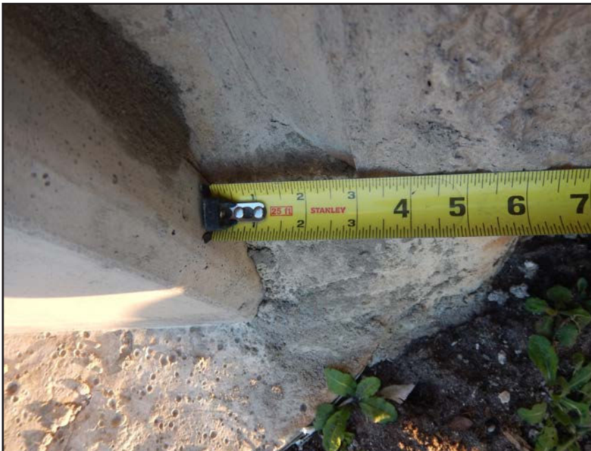
NO. 259 - COLUMN 55SS - INSUFFICIENT SEATING OF A PRECAST WALL PANEL IN A PRECAST COLUMN
