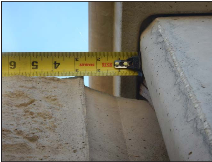
NO. 222 - COLUMN 34S - INSUFFICIENT SEATING OF A PRECAST WALL PANEL IN A PRECAST COLUMN
