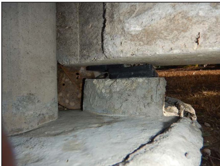
NO. 16 - COLUMN 3N - TYPICAL WALL PANEL BEARING CONDITION AT A GROUT PEDESTAL WITH 2" x 2" NEOPRENE BEARING PADS
