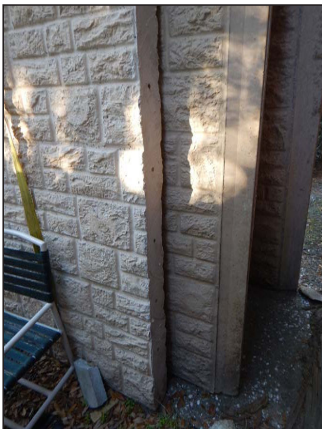
NO. 42 - SAW CUT STORED EXCESS WALL PANEL - TYPICAL HORIZONTAL REINFORCING BARS
