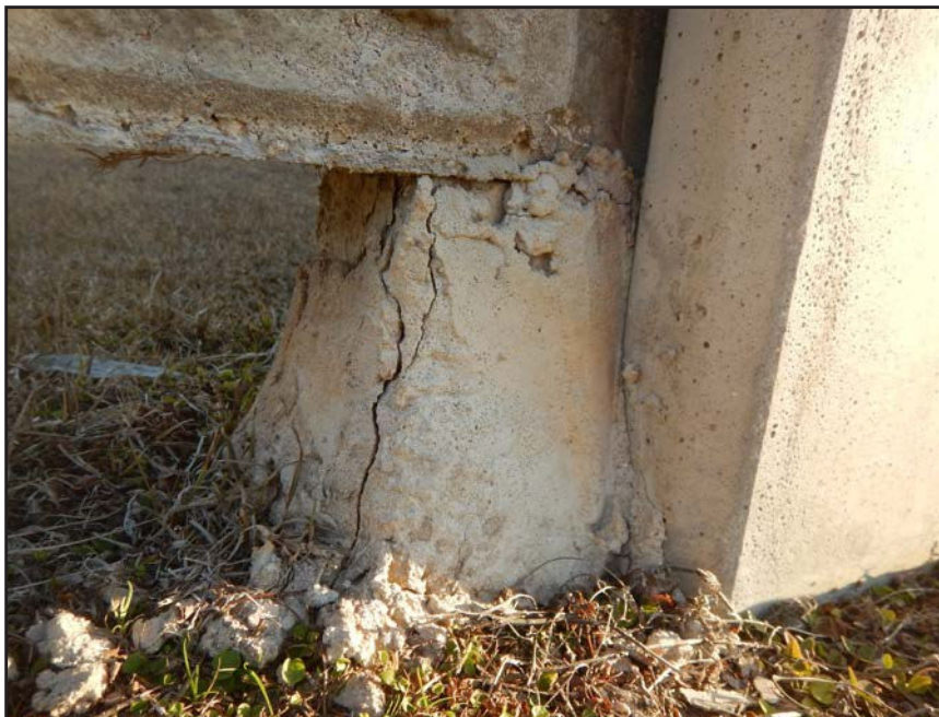
NO. 173 - COLUMN 45SS - INADEQUATE BEARING OF A PRECAST WALL PANEL ON A FAILED GROUT PEDESTAL OR A FAILED PRECAST TONGUE
