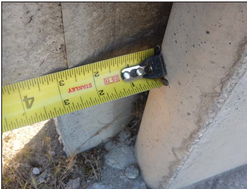
NO. 221 - COLUMN 29S - INSUFFICIENT SEATING OF A PRECAST WALL PANEL IN A PRECAST COLUMN
