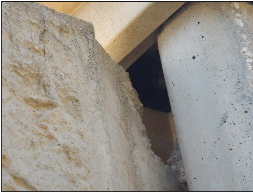
NO. 311 - COLUMN 8NM - CRACKED AND FAILED TONGUE OF A PRECAST WALL PANEL IN A PRECAST COLUMN
