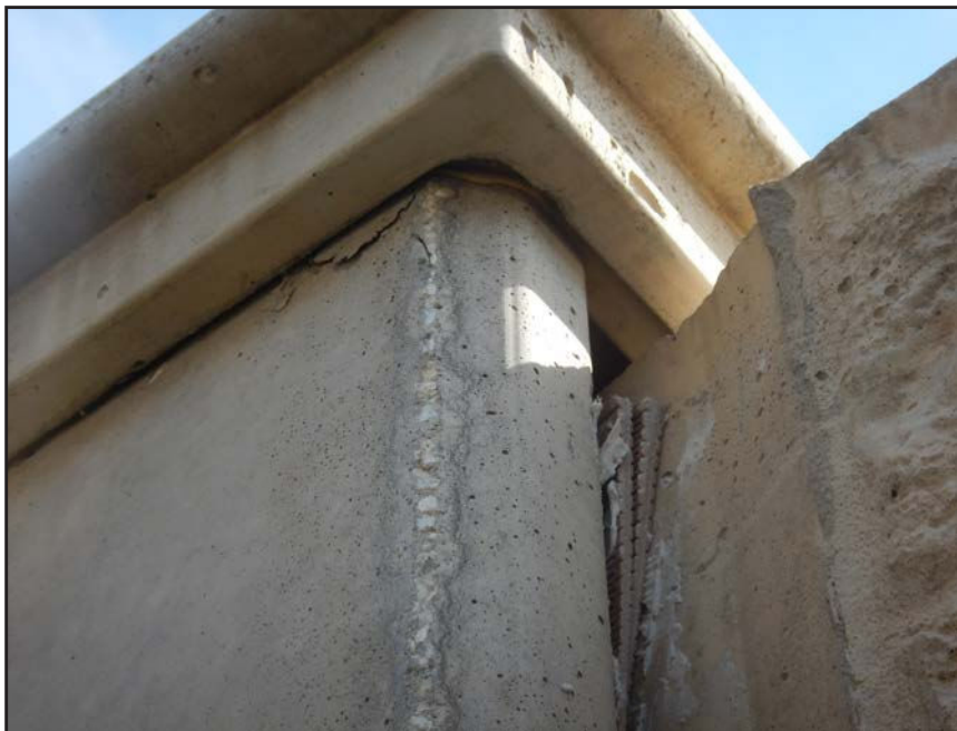
NO. 464 - COLUMN 13S - CRACKED AND SPALLED PRECAST CONCRETE
