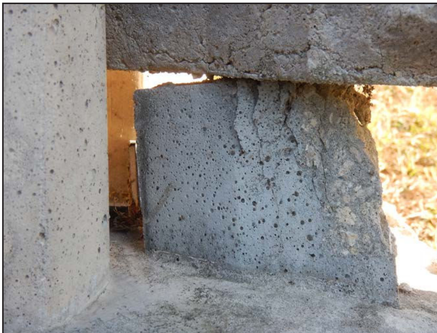
NO. 147 - COLUMN 75S - INADEQUATE BEARING OF A PRECAST WALL PANEL ON A FAILED GROUT PEDESTAL OR A FAILED PRECAST TONGUE
