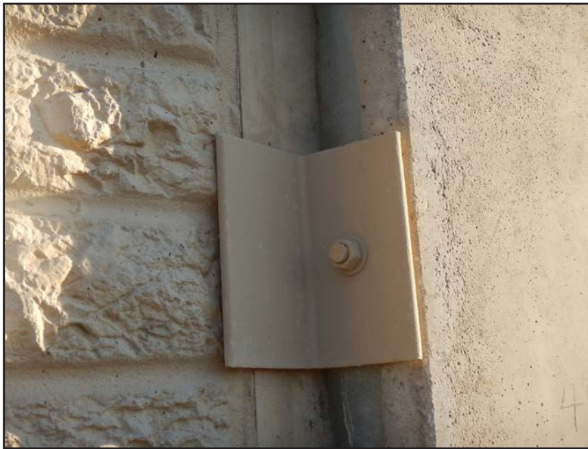
NO. 451 - COLUMN 41SS - INADEQUATE ADDED CLIP ANGLE CONNECTION AT A DEFICIENT WALL PANEL TO COLUMN CONNECTION
