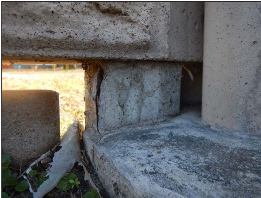
NO. 146 - COLUMN 75S - INADEQUATE BEARING OF A PRECAST WALL PANEL ON A FAILED GROUT PEDESTAL OR A FAILED PRECAST TONGUE
