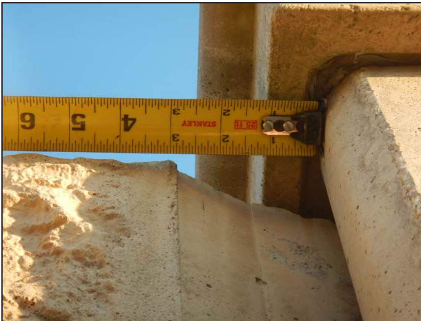
NO. 255 - COLUMN 47SS - INSUFFICIENT SEATING OF A PRECAST WALL PANEL IN A PRECAST COLUMN
