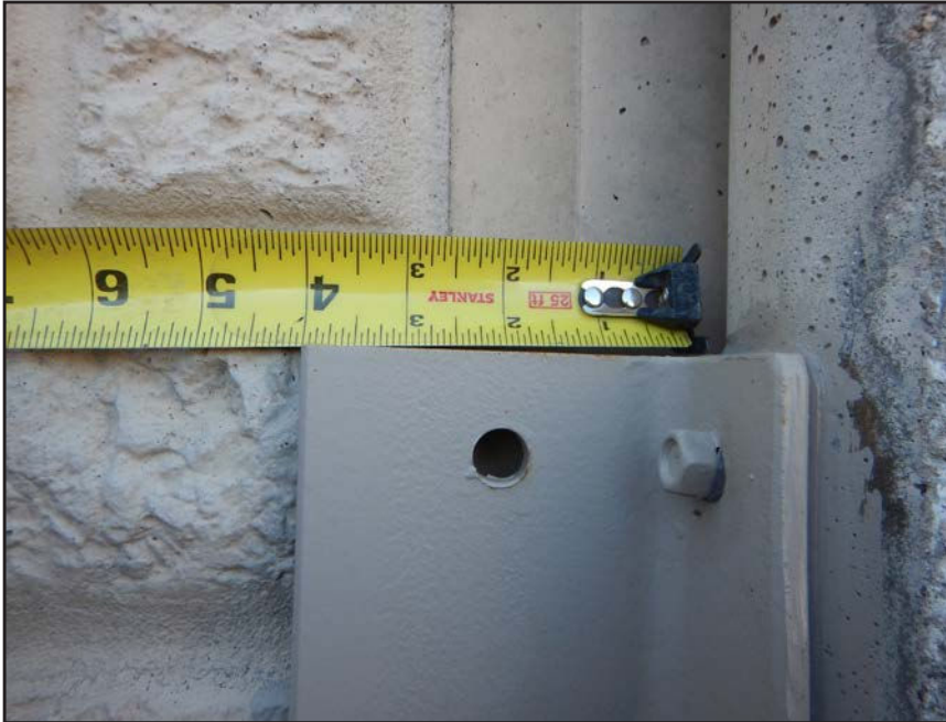
NO. 404 - COLUMN 1NE - INADEQUATE ADDED CLIP ANGLE CONNECTION AT A DEFICIENT WALL PANEL TO COLUMN CONNECTION
