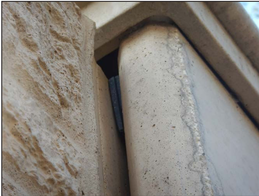
NO. 271 - COLUMN 26SM - INADEQUATE SHIMS STABILIZING A WALL PANEL TO COLUMN CONNECTION AT EXCESSIVE PLAY BETWEEN ADJACENT MEMBERS
