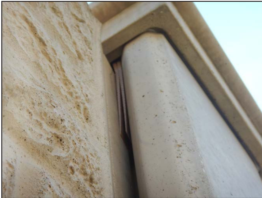
NO. 277 - COLUMN 31S - INADEQUATE SHIMS STABILIZING A WALL PANEL TO COLUMN CONNECTION AT EXCESSIVE PLAY BETWEEN ADJACENT MEMBERS
