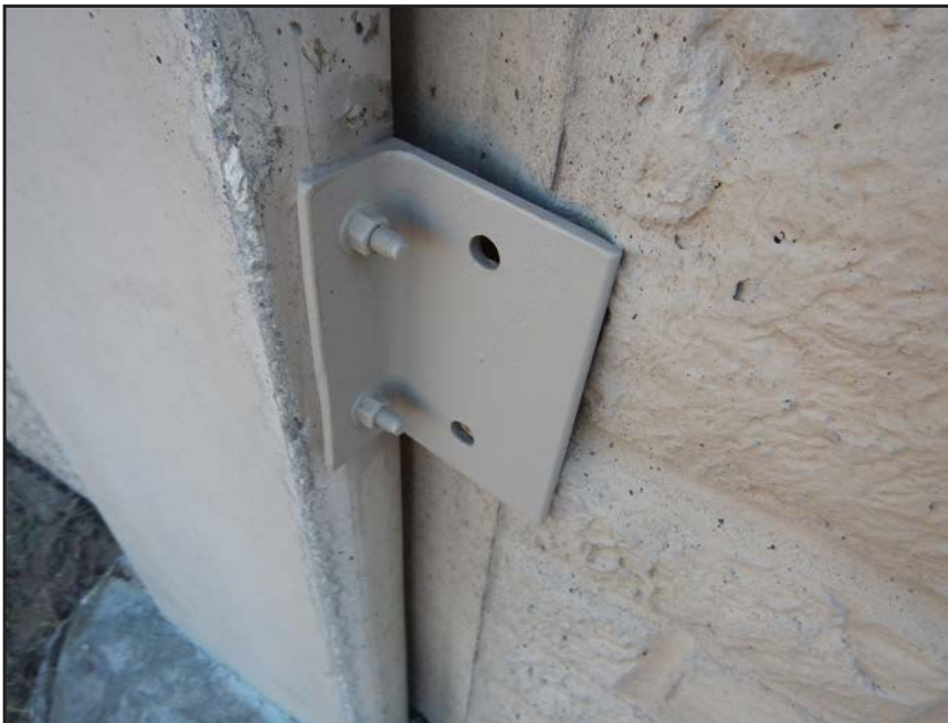
NO. 411 - COLUMN 6N - INADEQUATE ADDED CLIP ANGLE CONNECTION AT A DEFICIENT WALL PANEL TO COLUMN CONNECTION
