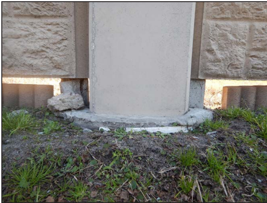
NO. 148 - COLUMN 76S - INADEQUATE BEARING OF A PRECAST WALL PANEL ON A FAILED GROUT PEDESTAL OR A FAILED PRECAST TONGUE
