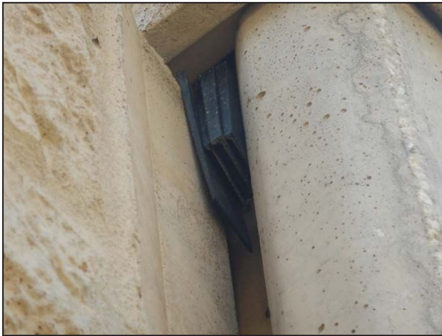
NO. 273 - COLUMN 10S - INADEQUATE SHIMS STABILIZING A WALL PANEL TO COLUMN CONNECTION AT EXCESSIVE PLAY BETWEEN ADJACENT MEMBERS
