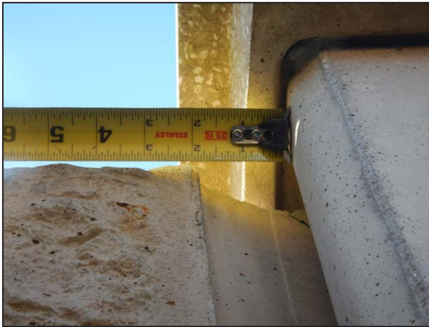
NO. 293 - COLUMN 44N - CRACKED AND FAILED TONGUE OF A PRECAST WALL PANEL IN A PRECAST COLUMN
