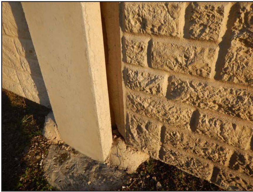
NO. 370 - COLUMN 46SS - CRACKED AND FAILED TONGUE OF A PRECAST WALL PANEL IN A PRECAST COLUMN
