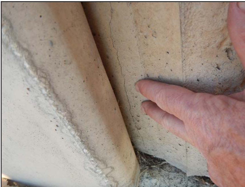
NO. 377 - COLUMN 47SS - CRACKED AND FAILED TONGUE OF A PRECAST WALL PANEL IN A PRECAST COLUMN
