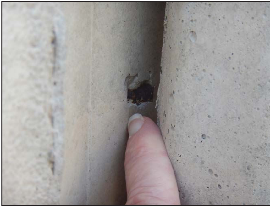
NO. 500 - COLUMN 12S - EXPOSED REINFORCING STEEL WITH INADEQUATE CONCRETE COVER
