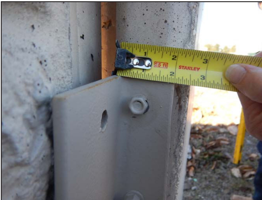
NO. 405 - COLUMN 1NE - INADEQUATE ADDED CLIP ANGLE CONNECTION AT A DEFICIENT WALL PANEL TO COLUMN CONNECTION
