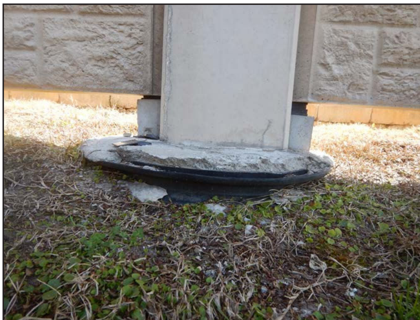
NO. 90 - COLUMN 33S - INADEQUATE BEARING OF A PRECAST WALL PANEL ON A 2" x 2" NEOPRENE BEARING PAD
