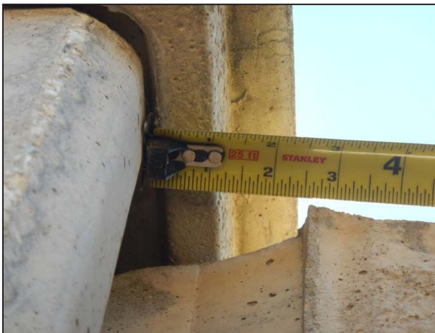
NO. 198 - COLUMN 57N - INSUFFICIENT SEATING OF A PRECAST WALL PANEL IN A PRECAST COLUMN
