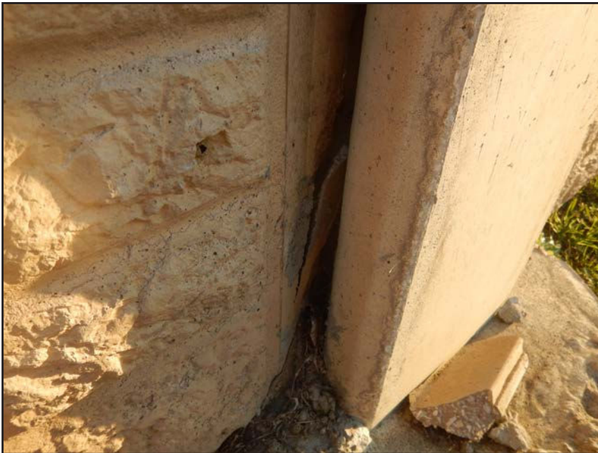
NO. 374 - COLUMN 47SS - CRACKED AND FAILED TONGUE OF A PRECAST WALL PANEL IN A PRECAST COLUMN
