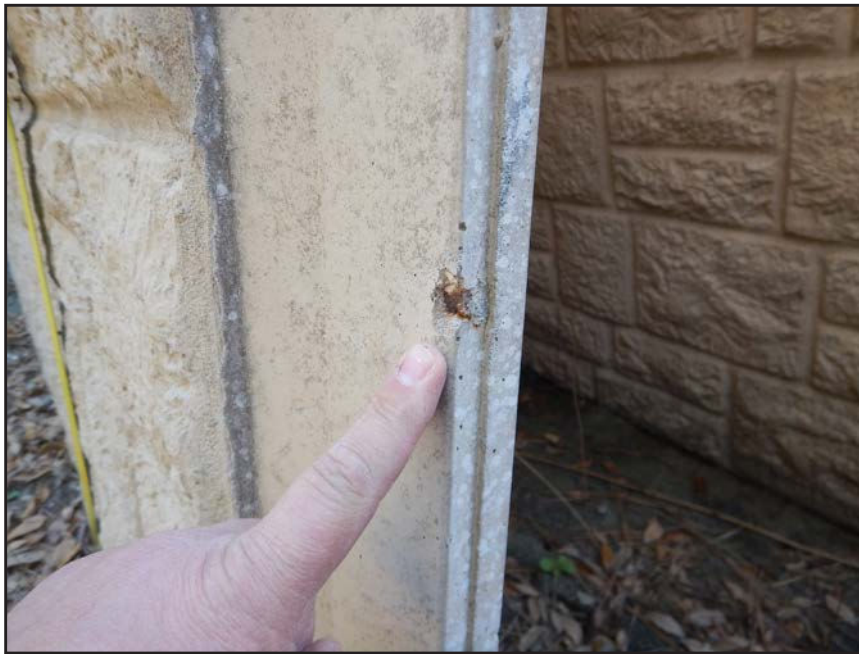
NO. 36 - STORED EXCESS WALL PANEL - TONGUE REINFORCING STEEL WITH INADEQUATE CONCRETE COVER
