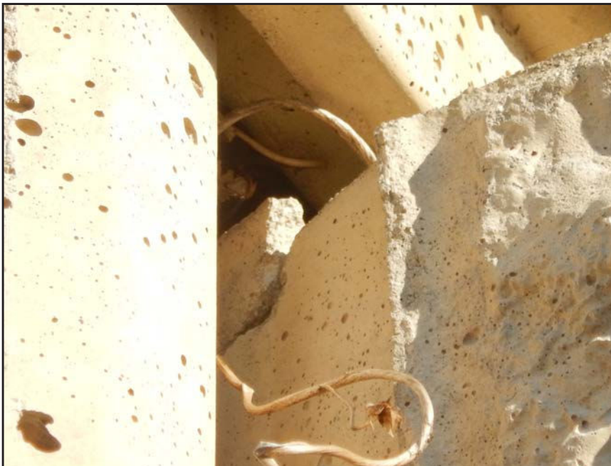
NO. 360 - COLUMN 25SS - CRACKED AND FAILED TONGUE OF A PRECAST WALL PANEL IN A PRECAST COLUMN
