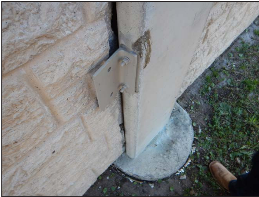
NO. 422 - COLUMN 14N - INADEQUATE ADDED CLIP ANGLE CONNECTION AT A DEFICIENT WALL PANEL TO COLUMN CONNECTION
