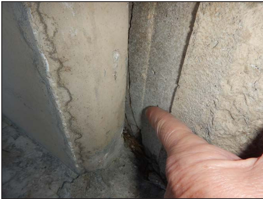
NO. 337 - COLUMN 70S - CRACKED AND FAILED TONGUE OF A PRECAST WALL PANEL IN A PRECAST COLUMN
