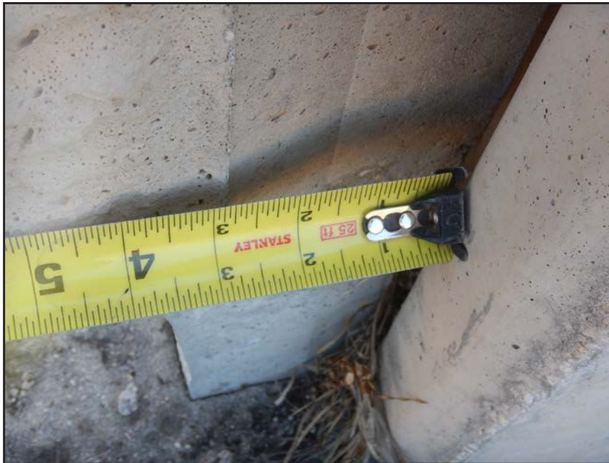
NO. 230 - COLUMN 47S - INSUFFICIENT SEATING OF A PRECAST WALL PANEL IN A PRECAST COLUMN
