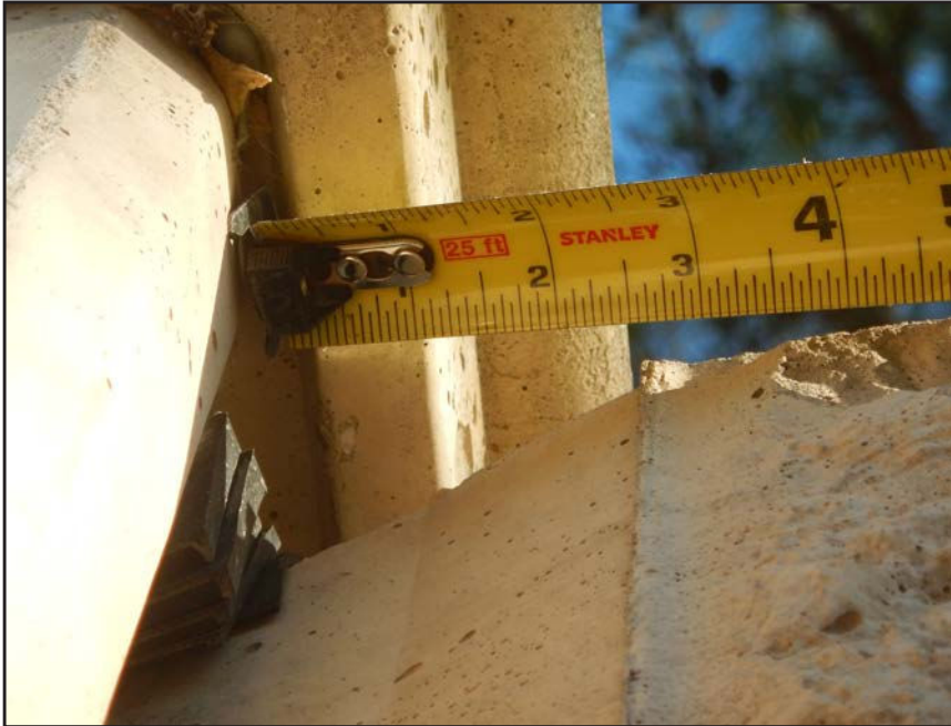
NO. 249 - COLUMN 24SS - INSUFFICIENT SEATING OF A PRECAST WALL PANEL IN A PRECAST COLUMN
