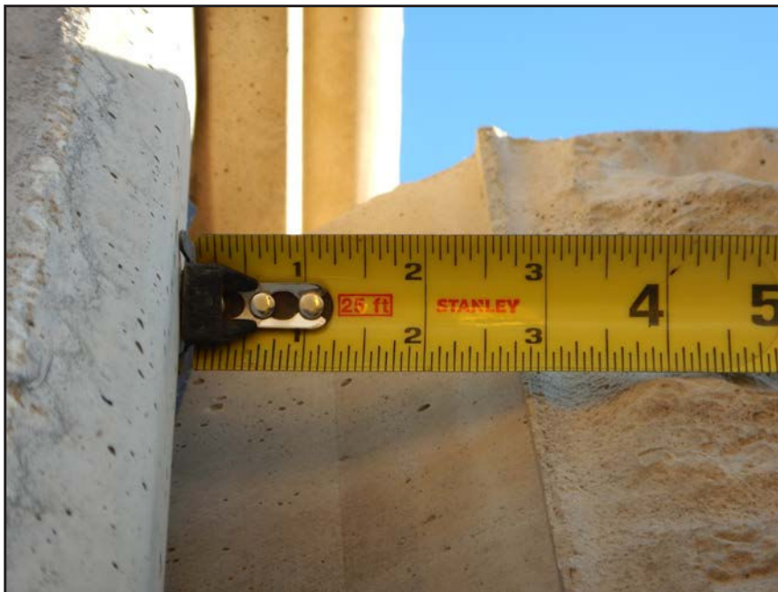
NO. 190 - COLUMN 28N - INSUFFICIENT SEATING OF A PRECAST WALL PANEL IN A PRECAST COLUMN
