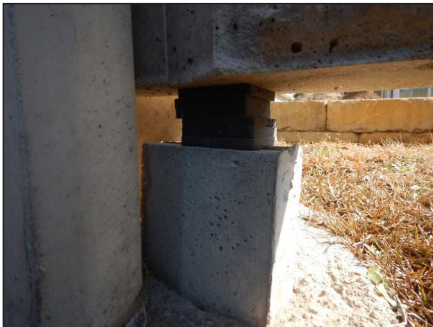
NO. 91 - COLUMN 33S - INADEQUATE BEARING OF A PRECAST WALL PANEL ON A 2" x 2" NEOPRENE BEARING PAD
