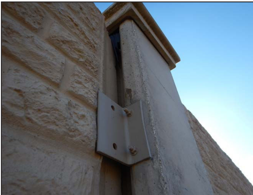
NO. 430 - COLUMN 20N - INADEQUATE ADDED CLIP ANGLE CONNECTION AT A DEFICIENT WALL PANEL TO COLUMN CONNECTION
