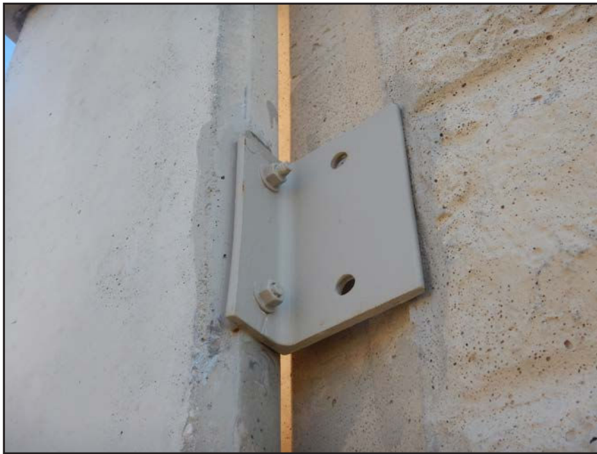
NO. 444 - COLUMN 55S - INADEQUATE ADDED CLIP ANGLE CONNECTION AT A DEFICIENT WALL PANEL TO COLUMN CONNECTION
