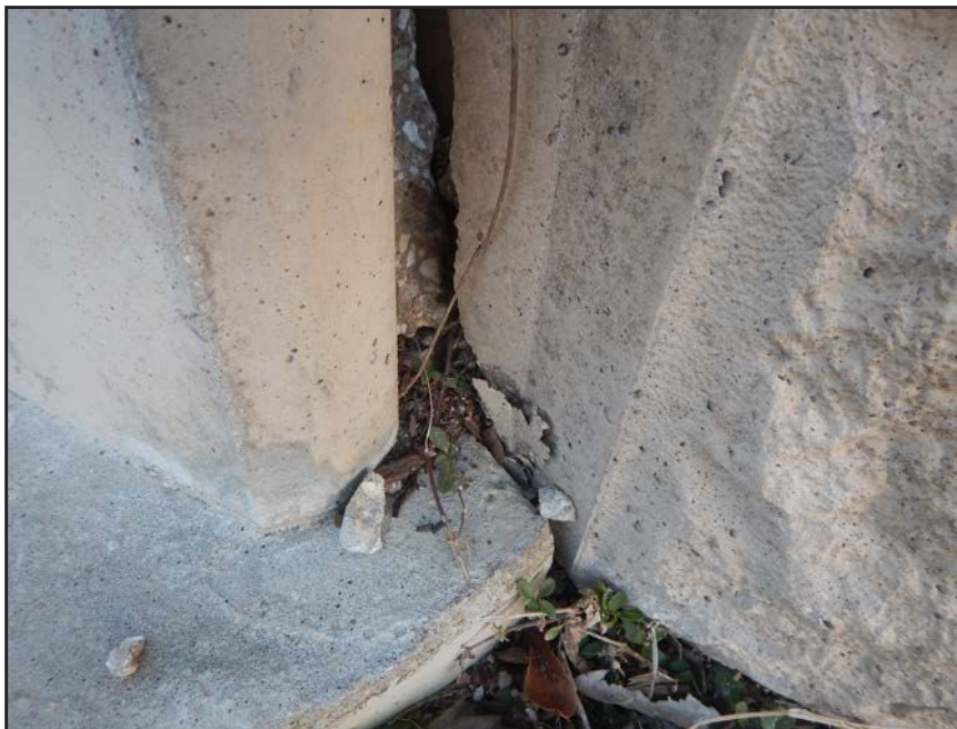
NO. 395 - COLUMN 70SS - CRACKED AND FAILED TONGUE OF A PRECAST WALL PANEL IN A PRECAST COLUMN
