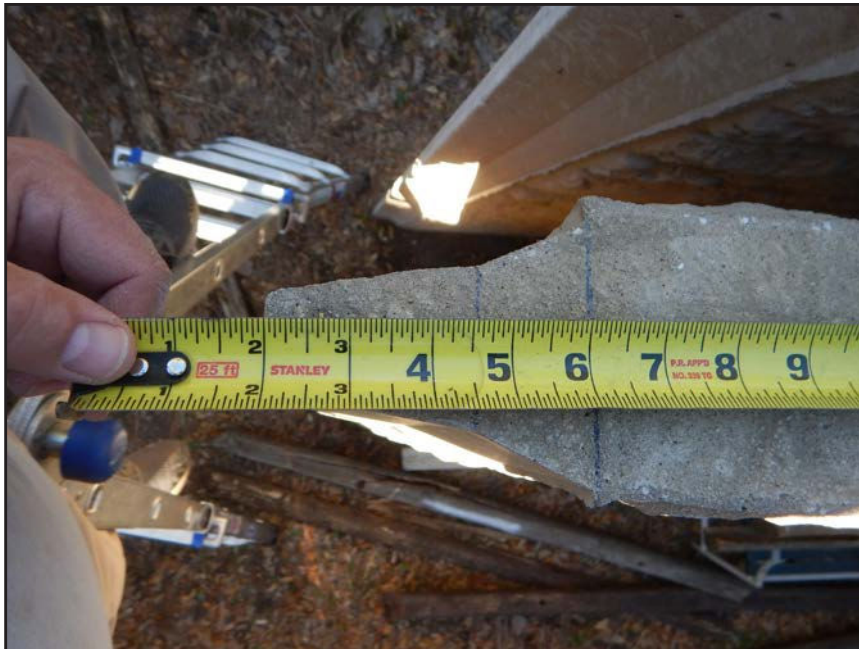
NO. 30 - STORED EXCESS WALL PANELS - TYPICAL TONGUE DIMENSIONS
