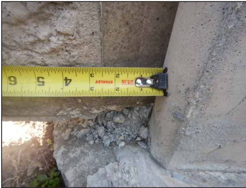
NO. 216 - COLUMN 12S - INSUFFICIENT SEATING OF A PRECAST WALL PANEL IN A PRECAST COLUMN
