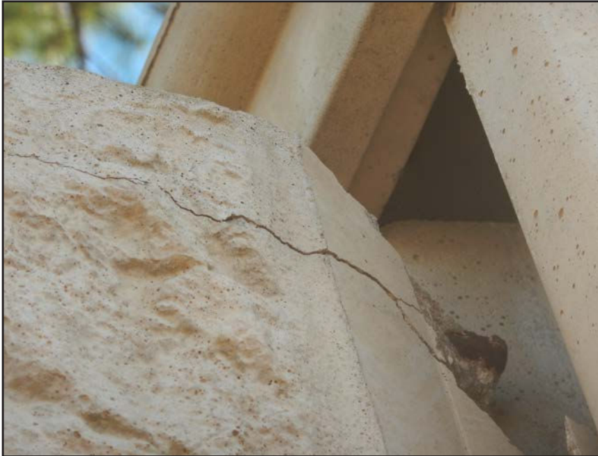
NO. 503 - COLUMN 25SS - EXPOSED REINFORCING STEEL WITH INADEQUATE CONCRETE COVER
