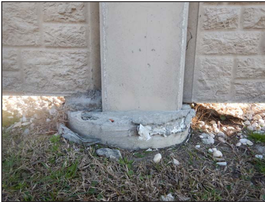
NO. 139 - COLUMN 67S - INADEQUATE BEARING OF A PRECAST WALL PANEL ON A FAILED GROUT PEDESTAL OR A FAILED PRECAST TONGUE
