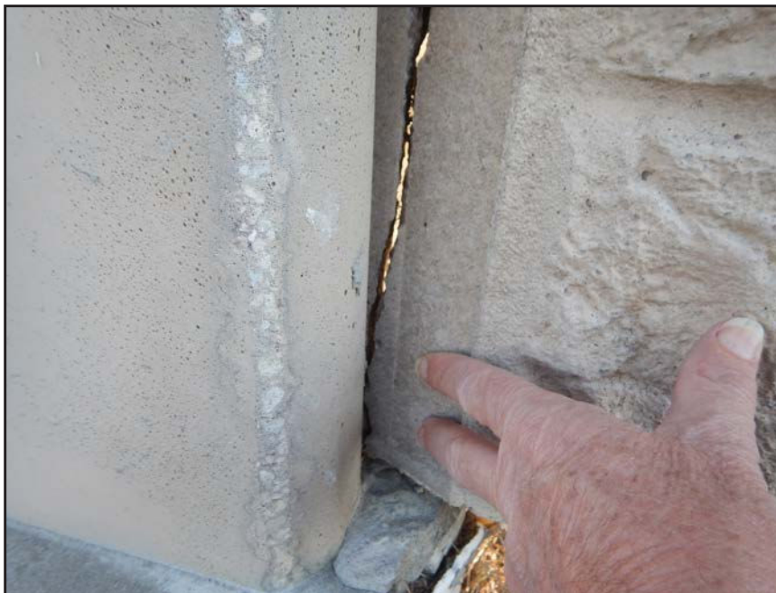
NO. 336 - COLUMN 67S - CRACKED AND FAILED TONGUE OF A PRECAST WALL PANEL IN A PRECAST COLUMN
