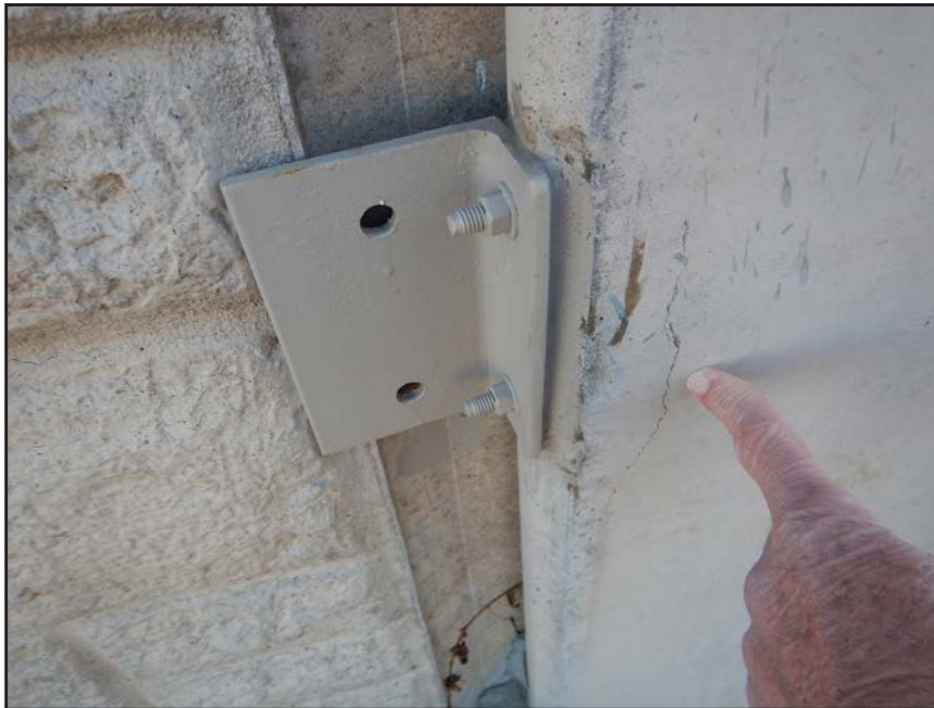
NO. 415 - COLUMN 9N - INADEQUATE ADDED CLIP ANGLE CONNECTION AT A DEFICIENT WALL PANEL TO COLUMN CONNECTION
