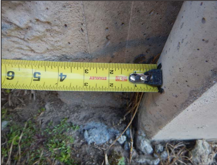
NO. 191 - COLUMN 30N - INSUFFICIENT SEATING OF A PRECAST WALL PANEL IN A PRECAST COLUMN
