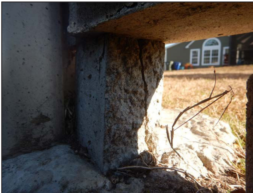
NO. 150 - COLUMN 76S - INADEQUATE BEARING OF A PRECAST WALL PANEL ON A FAILED GROUT PEDESTAL OR A FAILED PRECAST TONGUE
