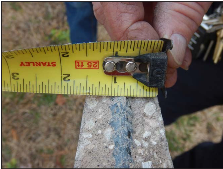
NO. 57 - SPALLED WALL PANEL ON THE SOUTH SIDE OF COLUMN 13NM - TONGUE REINFORCING DOWEL WITH INADEQUATE CONCRETE COVER
