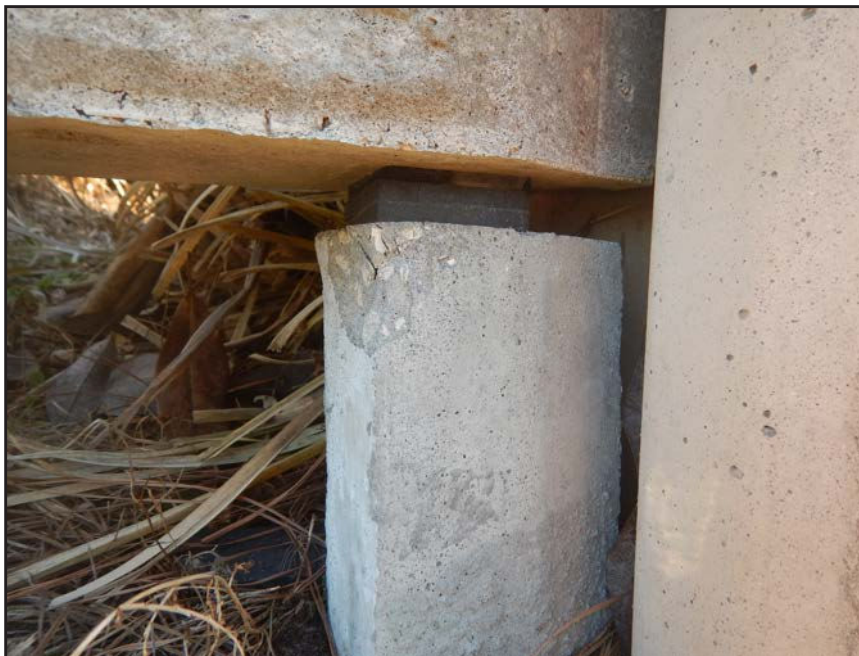
NO. 170 - COLUMN 33SS - INADEQUATE BEARING OF A PRECAST WALL PANEL ON A FAILED GROUT PEDESTAL OR A FAILED PRECAST TONGUE
