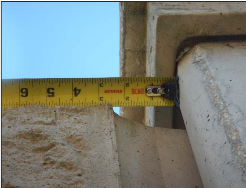
NO. 239 - COLUMN 76S - INSUFFICIENT SEATING OF A PRECAST WALL PANEL IN A PRECAST COLUMN
