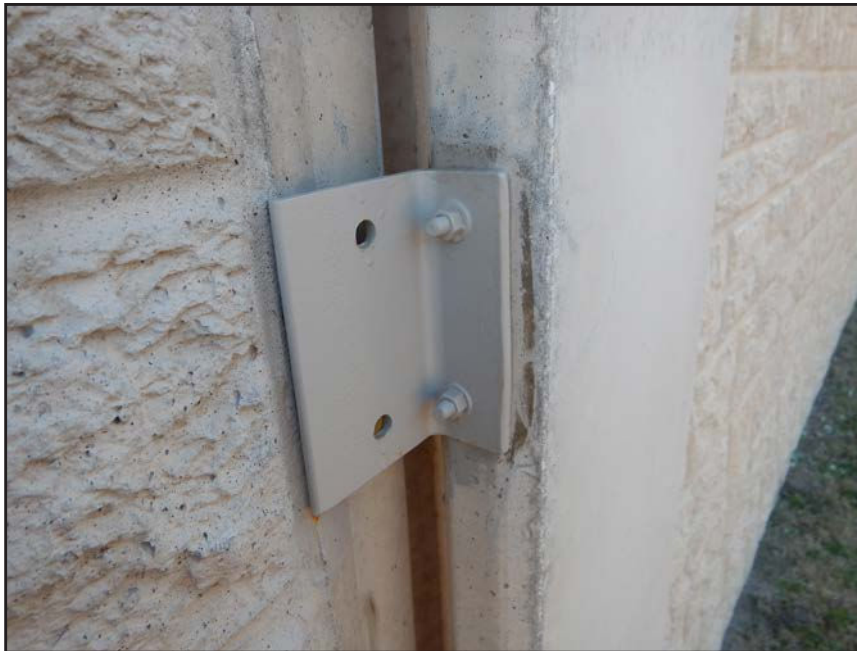
NO. 427 - COLUMN 19N - INADEQUATE ADDED CLIP ANGLE CONNECTION AT A DEFICIENT WALL PANEL TO COLUMN CONNECTION
