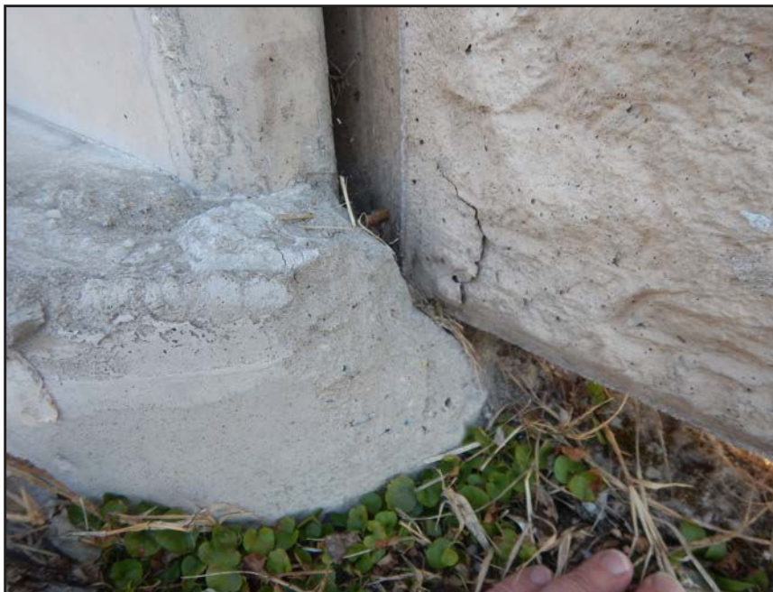
NO. 133 - COLUMN 53S - INADEQUATE BEARING OF A PRECAST WALL PANEL ON A FAILED GROUT PEDESTAL OR A FAILED PRECAST TONGUE
