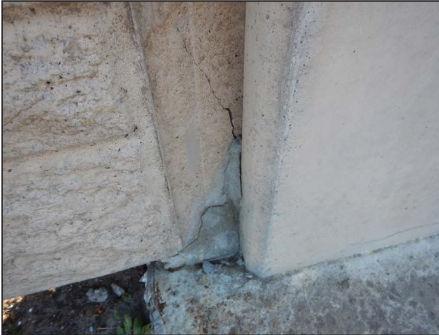
NO. 287 - COLUMN 9N - CRACKED AND FAILED TONGUE OF A PRECAST WALL PANEL IN A PRECAST COLUMN
