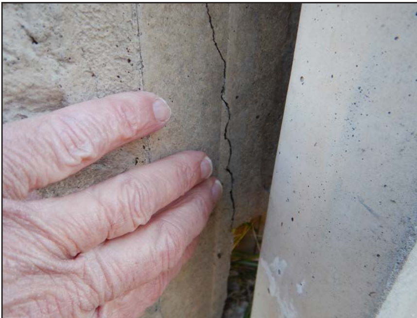
NO. 290 - COLUMN 28N - CRACKED AND FAILED TONGUE OF A PRECAST WALL PANEL IN A PRECAST COLUMN
