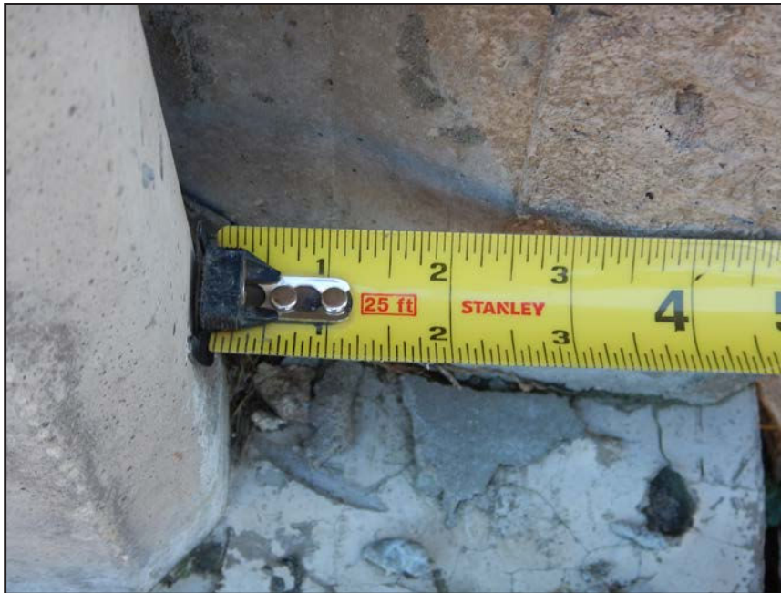
NO. 194 - COLUMN 36N - INSUFFICIENT SEATING OF A PRECAST WALL PANEL IN A PRECAST COLUMN
