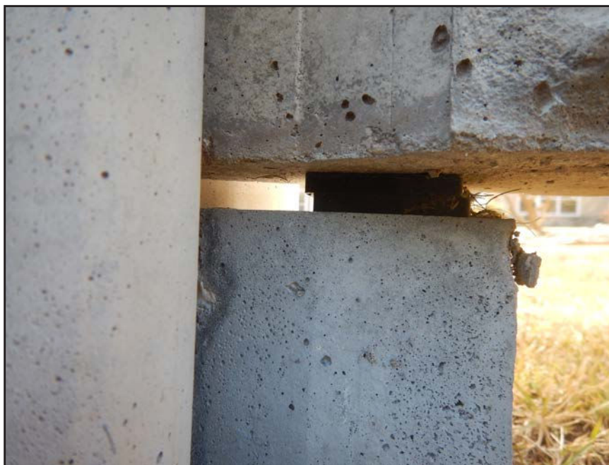
NO. 84 - COLUMN 15SM - INADEQUATE BEARING OF A PRECAST WALL PANEL ON A 2" x 2" NEOPRENE BEARING PAD
