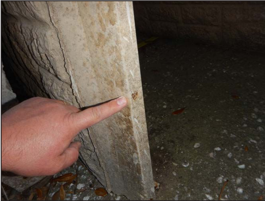
NO. 40 - STORED EXCESS WALL PANEL - TONGUE REINFORCING STEEL WITH INADEQUATE CONCRETE COVER
