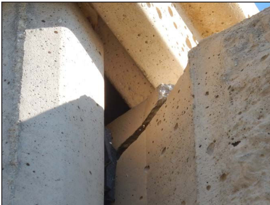
NO. 326- COLUMN 50S - CRACKED AND FAILED TONGUE OF A PRECAST WALL PANEL IN A PRECAST COLUMN
