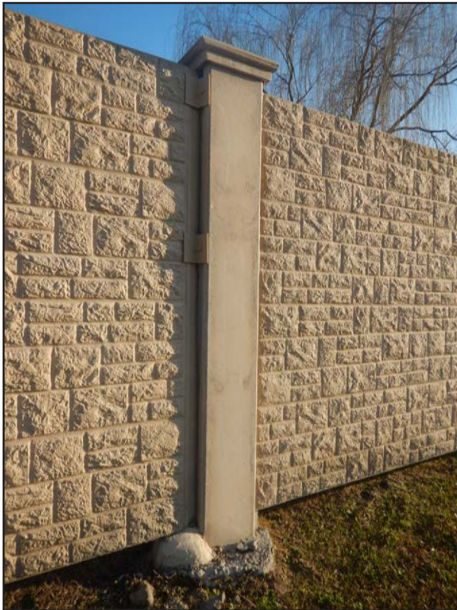
NO. 449 - COLUMN 41SS - INADEQUATE ADDED CLIP ANGLE CONNECTION AT A DEFICIENT WALL PANEL TO COLUMN CONNECTION
