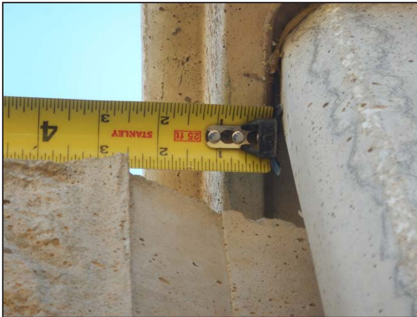
NO. 240 - COLUMN 79S - INSUFFICIENT SEATING OF A PRECAST WALL PANEL IN A PRECAST COLUMN
