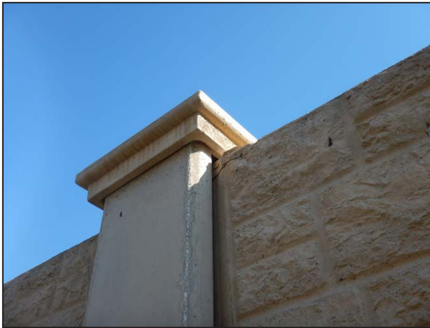
NO. 475 - COLUMN 78S - CRACKED AND SPALLED PRECAST CONCRETE
