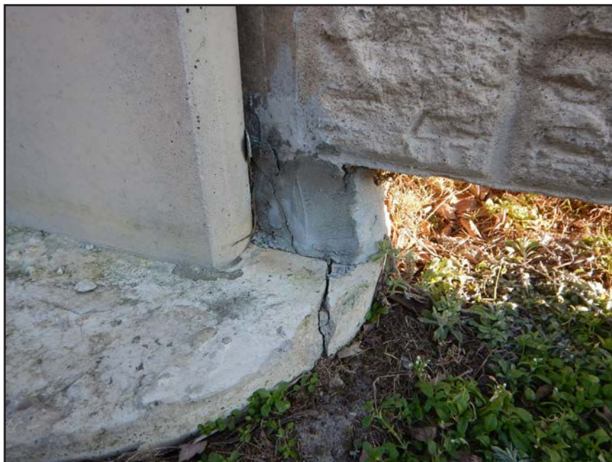
NO. 109 - COLUMN 41N - INADEQUATE BEARING OF A PRECAST WALL PANEL ON A FAILED GROUT PEDESTAL OR A FAILED PRECAST TONGUE
