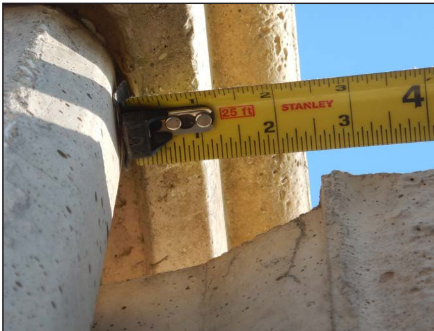
NO. 234 - COLUMN 68S - INSUFFICIENT SEATING OF A PRECAST WALL PANEL IN A PRECAST COLUMN
