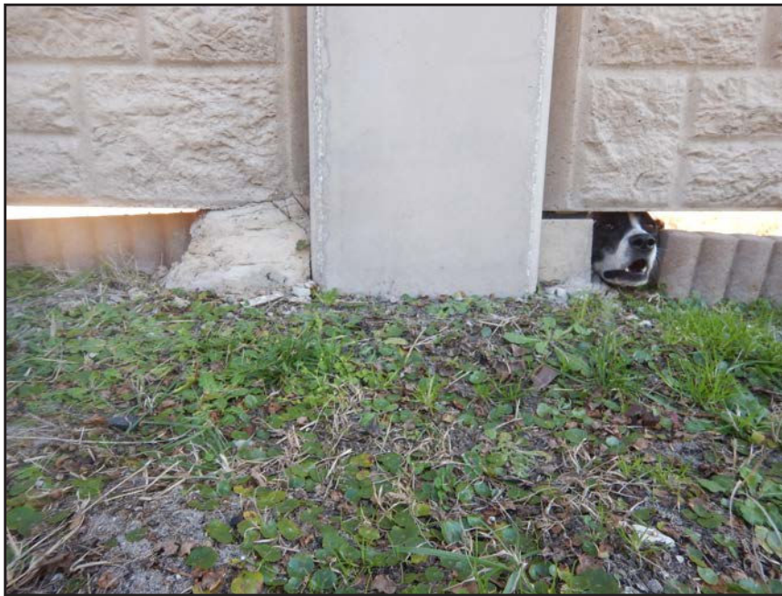
NO. 151 - COLUMN 78S - INADEQUATE BEARING OF A PRECAST WALL PANEL ON A FAILED GROUT PEDESTAL OR A FAILED PRECAST TONGUE
