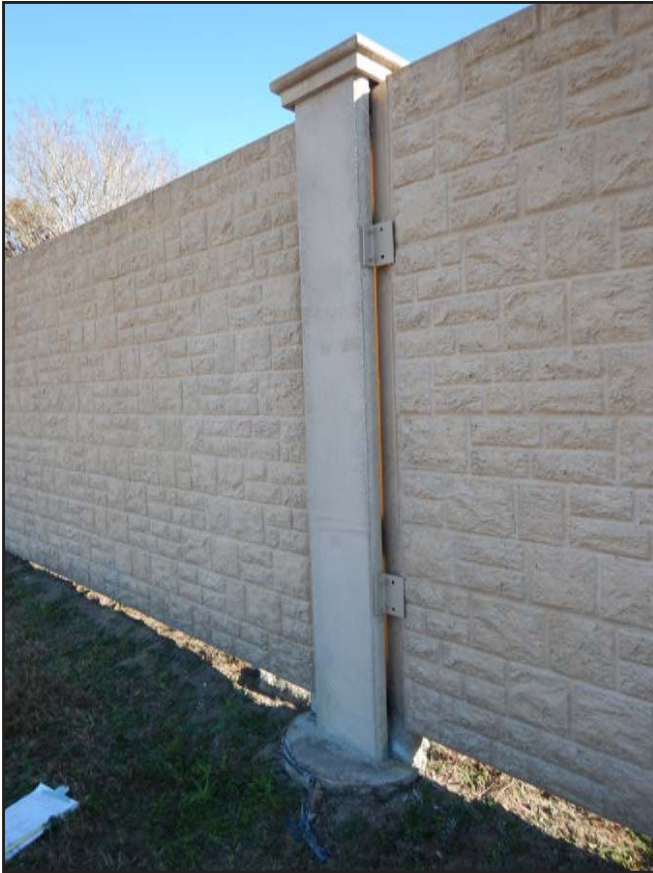
NO. 417 - COLUMN 10N - INADEQUATE ADDED CLIP ANGLE CONNECTION AT A DEFICIENT WALL PANEL TO COLUMN CONNECTION
