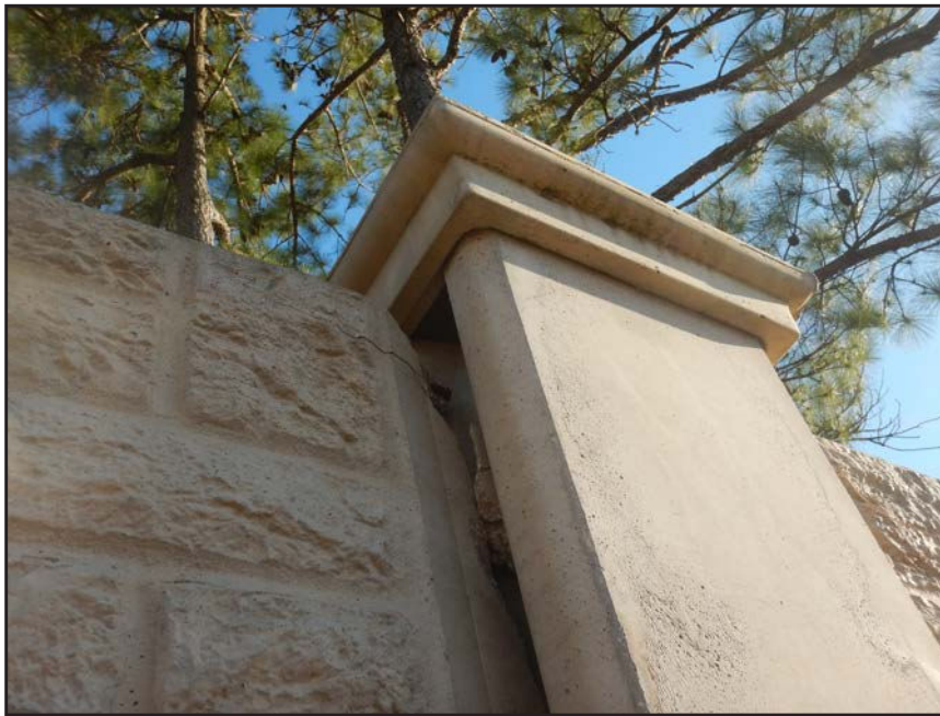
NO. 356 - COLUMN 25SS - CRACKED AND FAILED TONGUE OF A PRECAST WALL PANEL IN A PRECAST COLUMN
