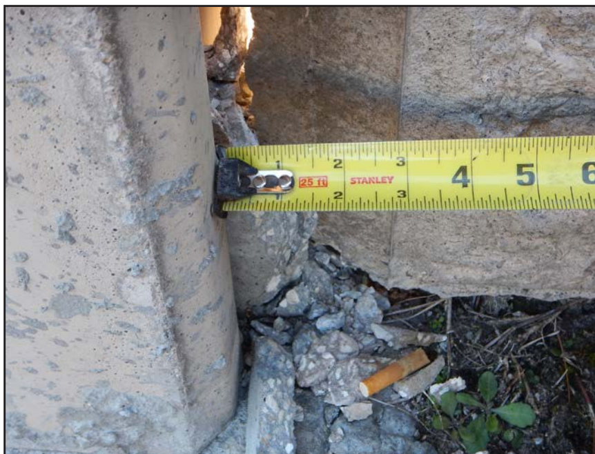
NO. 7 - COLUMN 13NM - DROPPED PRECAST PANEL WITH A 1" GAP AT THE TOP AND A 2 7/8" GAP AT THE BOTTOM
