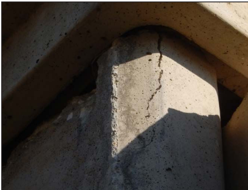
NO. 472 - COLUMN 75S - CRACKED AND SPALLED PRECAST CONCRETE
