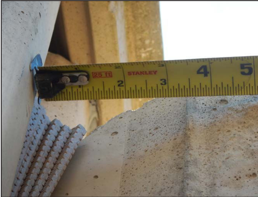
NO. 205 - COLUMN 11NM - INSUFFICIENT SEATING OF A PRECAST WALL PANEL IN A PRECAST COLUMN
