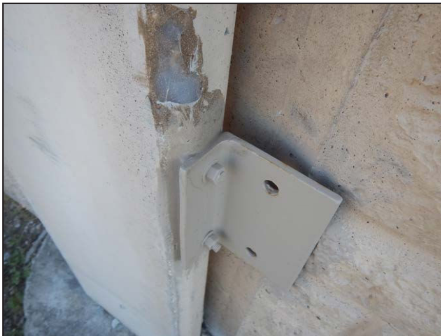
NO. 446 - COLUMN 55S - INADEQUATE ADDED CLIP ANGLE CONNECTION AT A DEFICIENT WALL PANEL TO COLUMN CONNECTION
