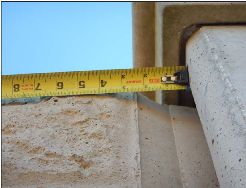
NO. 187 - COLUMN 18N - INSUFFICIENT SEATING OF A PRECAST WALL PANEL IN A PRECAST COLUMN
