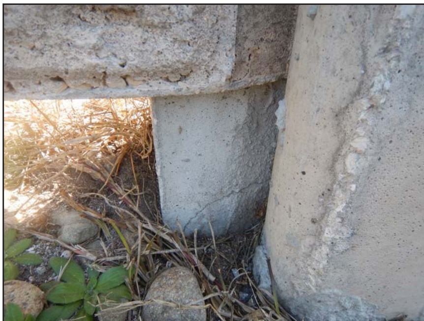
NO. 129 - COLUMN 37S - INADEQUATE BEARING OF A PRECAST WALL PANEL ON A FAILED GROUT PEDESTAL OR A FAILED PRECAST TONGUE
