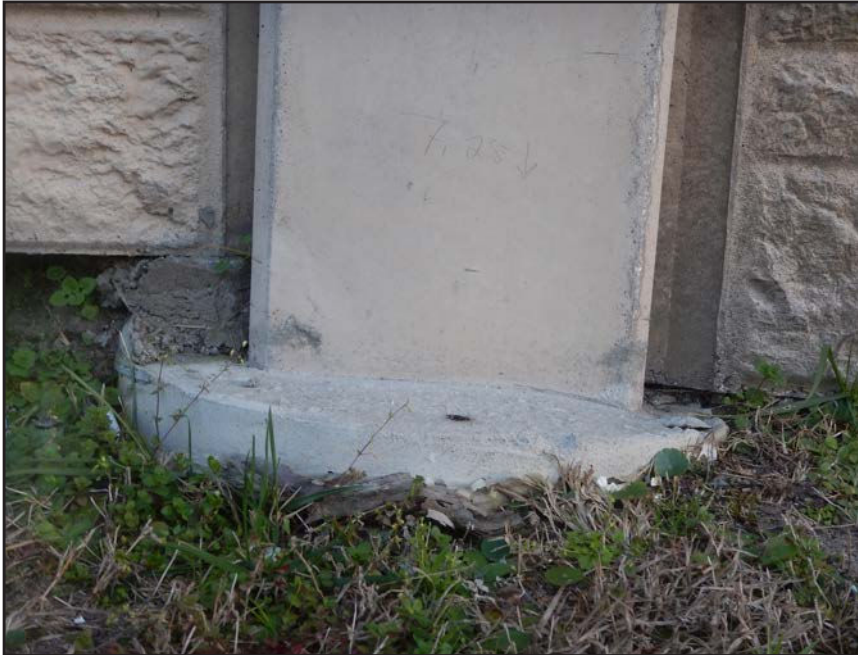
NO. 181 - COLUMN 71SS - INADEQUATE BEARING OF A PRECAST WALL PANEL ON A FAILED GROUT PEDESTAL OR A FAILED PRECAST TONGUE
