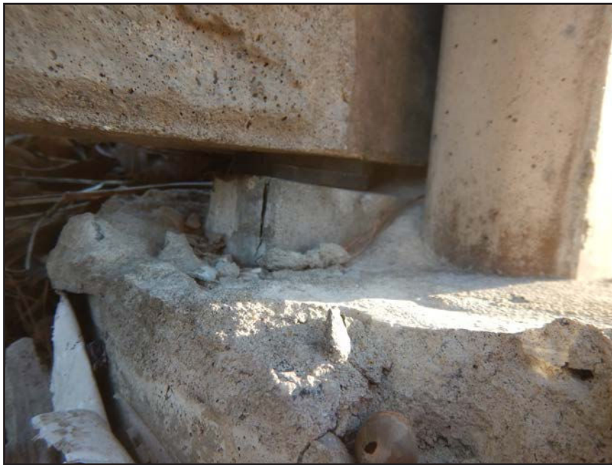
NO. 171 - COLUMN 35SS - INADEQUATE BEARING OF A PRECAST WALL PANEL ON A FAILED GROUT PEDESTAL OR A FAILED PRECAST TONGUE
