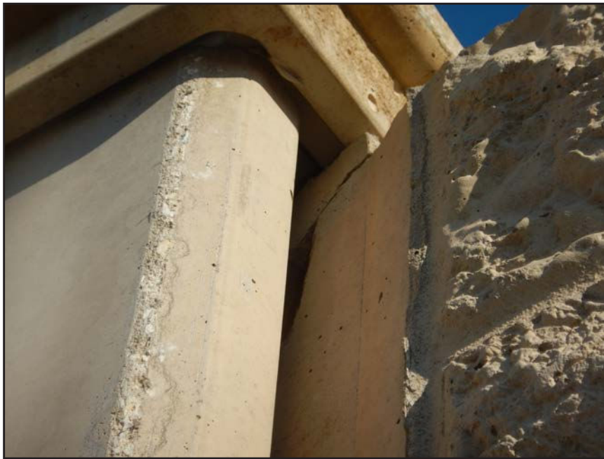
NO. 344 - COLUMN 8SS - CRACKED AND FAILED TONGUE OF A PRECAST WALL PANEL IN A PRECAST COLUMN
