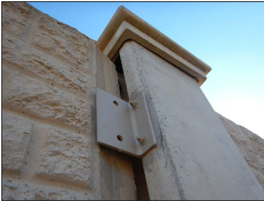
NO. 426 - COLUMN 19N - INADEQUATE ADDED CLIP ANGLE CONNECTION AT A DEFICIENT WALL PANEL TO COLUMN CONNECTION
