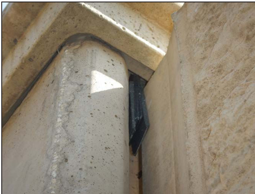
NO. 272 - COLUMN 4S - INADEQUATE SHIMS STABILIZING A WALL PANEL TO COLUMN CONNECTION AT EXCESSIVE PLAY BETWEEN ADJACENT MEMBERS
