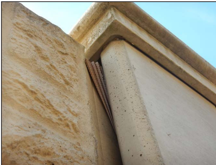
NO. 269 - COLUMN 24SM - INADEQUATE SHIMS STABILIZING A WALL PANEL TO COLUMN CONNECTION AT EXCESSIVE PLAY BETWEEN ADJACENT MEMBERS
