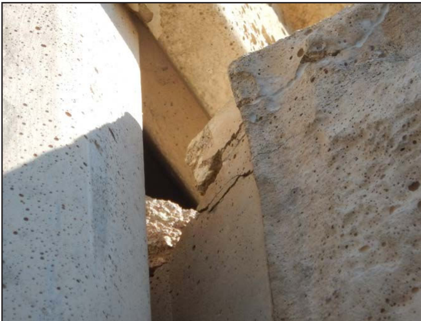
NO. 333 - COLUMN 62S - CRACKED AND FAILED TONGUE OF A PRECAST WALL PANEL IN A PRECAST COLUMN
