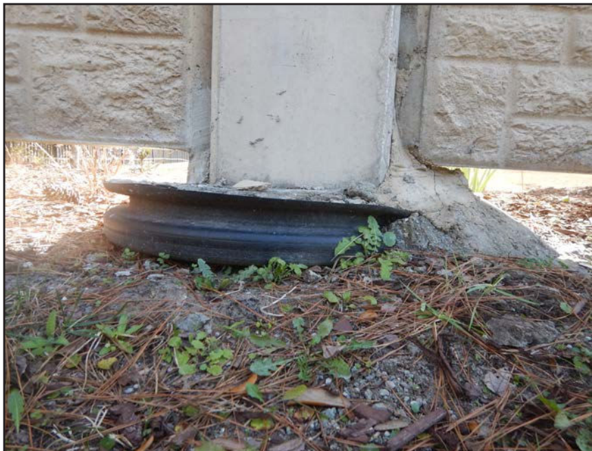
NO. 121 - COLUMN 2S - INADEQUATE BEARING OF A PRECAST WALL PANEL ON A FAILED GROUT PEDESTAL OR A FAILED PRECAST TONGUE
