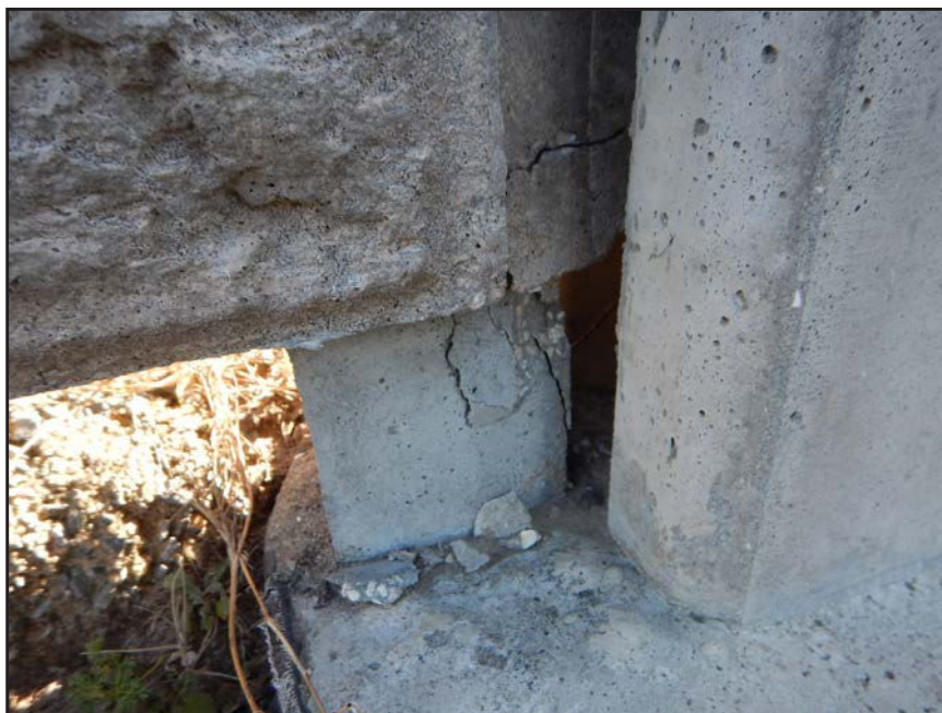
NO. 107 - COLUMN 10N - INADEQUATE BEARING OF A PRECAST WALL PANEL ON A FAILED GROUT PEDESTAL OR A FAILED PRECAST TONGUE
