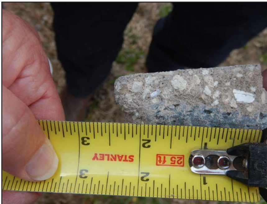
NO. 59 - SPALLED WALL PANEL ON THE SOUTH SIDE OF COLUMN 13NM - TONGUE REINFORCING DOWEL WITH INADEQUATE CONCRETE COVER
