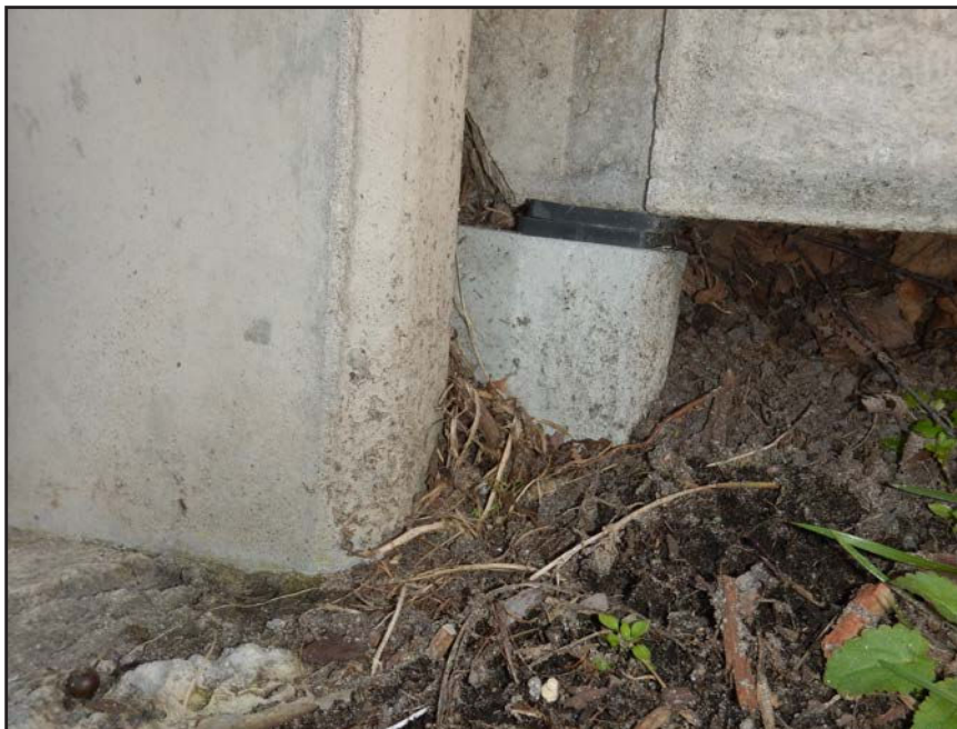
NO. 398 - COLUMN 76SS - CRACKED AND FAILED TONGUE OF A PRECAST WALL PANEL IN A PRECAST COLUMN
