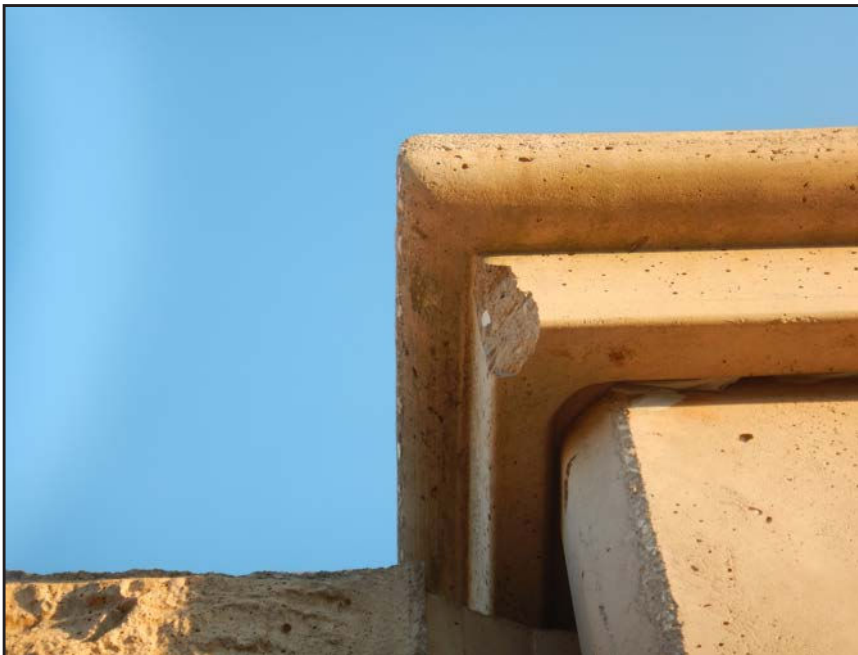
NO. 483 - COLUMN 55SS - CRACKED AND SPALLED PRECAST CONCRETE
