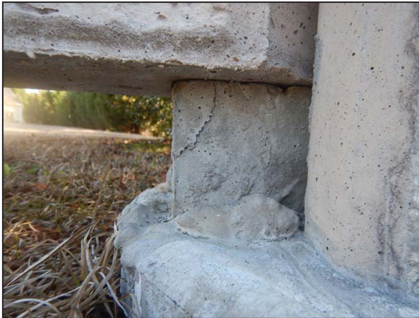
NO. 155 - COLUMN 82S - INADEQUATE BEARING OF A PRECAST WALL PANEL ON A FAILED GROUT PEDESTAL OR A FAILED PRECAST TONGUE
