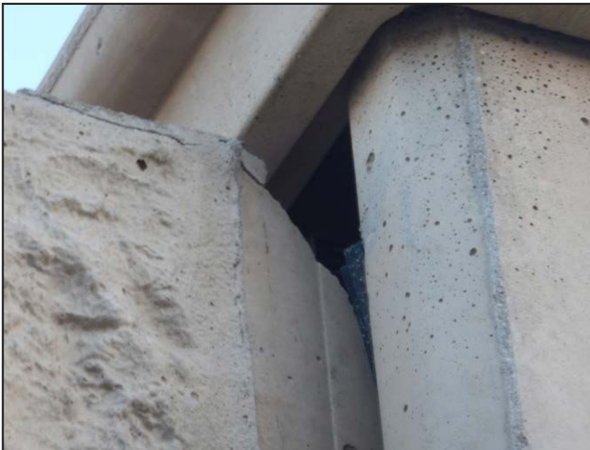
NO. 390 - COLUMN 65SS - CRACKED AND FAILED TONGUE OF A PRECAST WALL PANEL IN A PRECAST COLUMN
