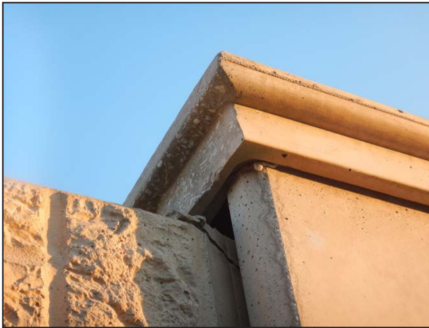
NO. 386 - COLUMN 62SS - CRACKED AND FAILED TONGUE OF A PRECAST WALL PANEL IN A PRECAST COLUMN
