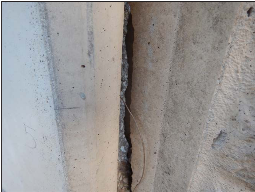
NO. 394 - COLUMN 70SS - CRACKED AND FAILED TONGUE OF A PRECAST WALL PANEL IN A PRECAST COLUMN
