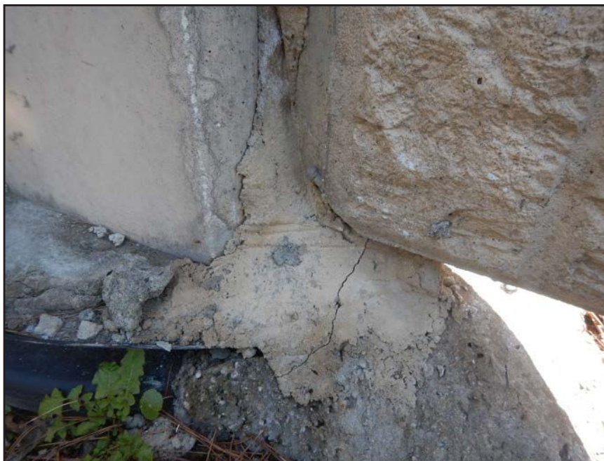
NO. 122 - COLUMN 2S - INADEQUATE BEARING OF A PRECAST WALL PANEL ON A FAILED GROUT PEDESTAL OR A FAILED PRECAST TONGUE
