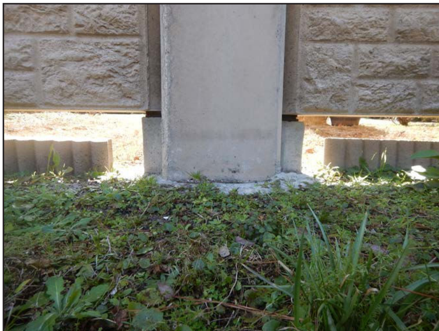
NO. 85 - COLUMN 22SM - INADEQUATE BEARING OF A PRECAST WALL PANEL ON A 2" x 2" NEOPRENE BEARING PAD
