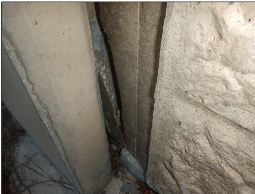
NO. 355 - COLUMN 22SS - CRACKED AND FAILED TONGUE OF A PRECAST WALL PANEL IN A PRECAST COLUMN
