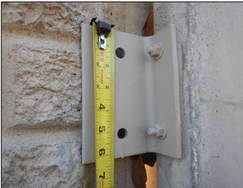
NO. 439 - COLUMN 50N - INADEQUATE ADDED CLIP ANGLE CONNECTION AT A DEFICIENT WALL PANEL TO COLUMN CONNECTION
