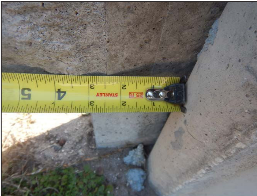
NO. 228 - COLUMN 42S - INSUFFICIENT SEATING OF A PRECAST WALL PANEL IN A PRECAST COLUMN
