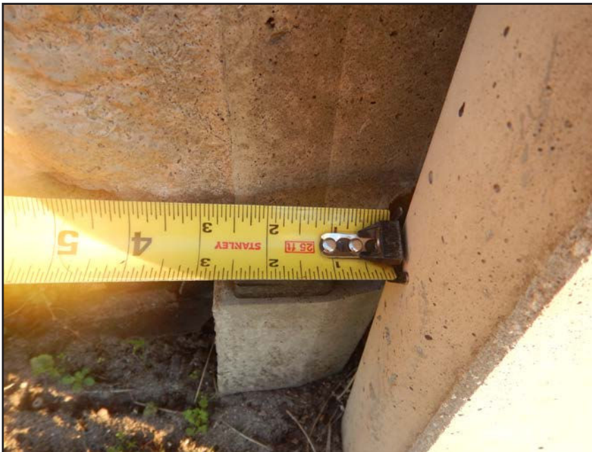
NO. 257 - COLUMN 51SS - INSUFFICIENT SEATING OF A PRECAST WALL PANEL IN A PRECAST COLUMN
