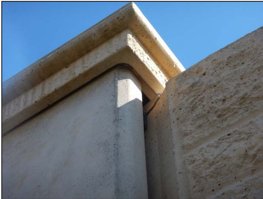
NO. 325 - COLUMN 50S - CRACKED AND FAILED TONGUE OF A PRECAST WALL PANEL IN A PRECAST COLUMN
