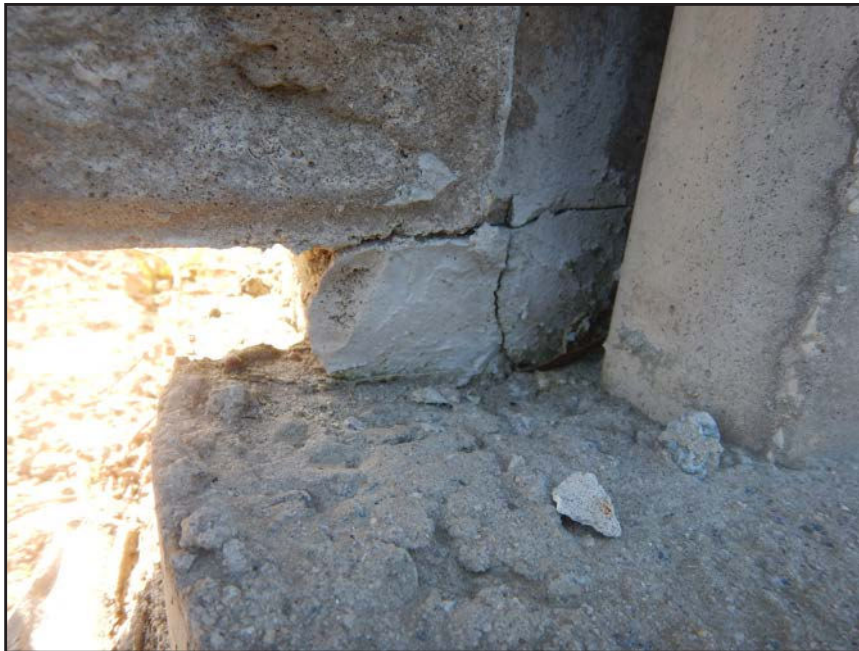
NO. 116 - COLUMN 55N - INADEQUATE BEARING OF A PRECAST WALL PANEL ON A FAILED GROUT PEDESTAL OR A FAILED PRECAST TONGUE
