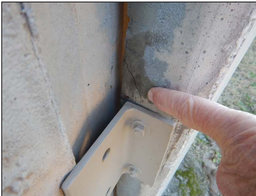
NO. 433 - COLUMN 20N - INADEQUATE ADDED CLIP ANGLE CONNECTION AT A DEFICIENT WALL PANEL TO COLUMN CONNECTION
