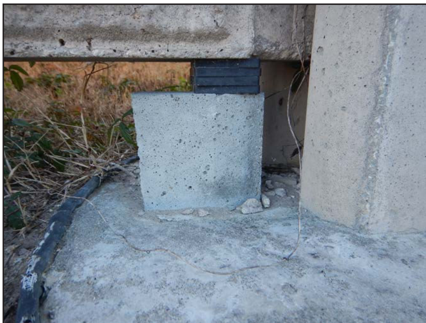
NO. 67 - COLUMN 11N - INADEQUATE BEARING OF A PRECAST WALL PANEL ON A 2" x 2" NEOPRENE BEARING PAD
