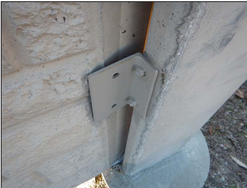
NO. 403 - COLUMN 1NE - INADEQUATE ADDED CLIP ANGLE CONNECTION AT A DEFICIENT WALL PANEL TO COLUMN CONNECTION
