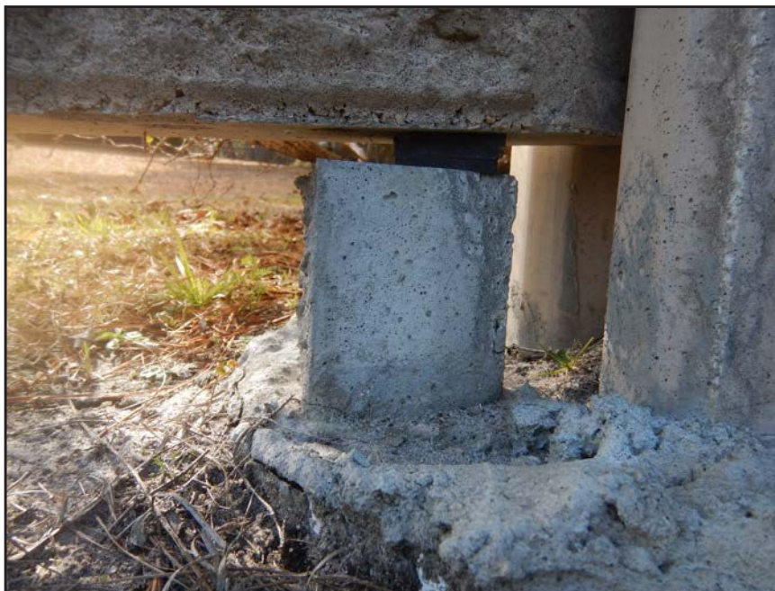
NO. 75 - COLUMN 14NM - INADEQUATE BEARING OF A PRECAST WALL PANEL ON A 2" x 2" NEOPRENE BEARING PAD
