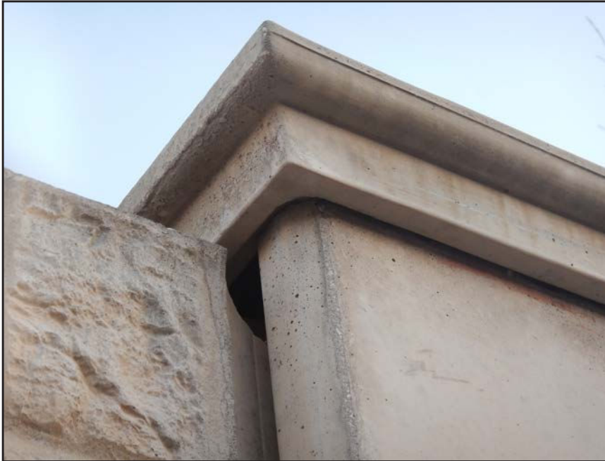
NO. 399 - COLUMN 78SS - CRACKED AND FAILED TONGUE OF A PRECAST WALL PANEL IN A PRECAST COLUMN
