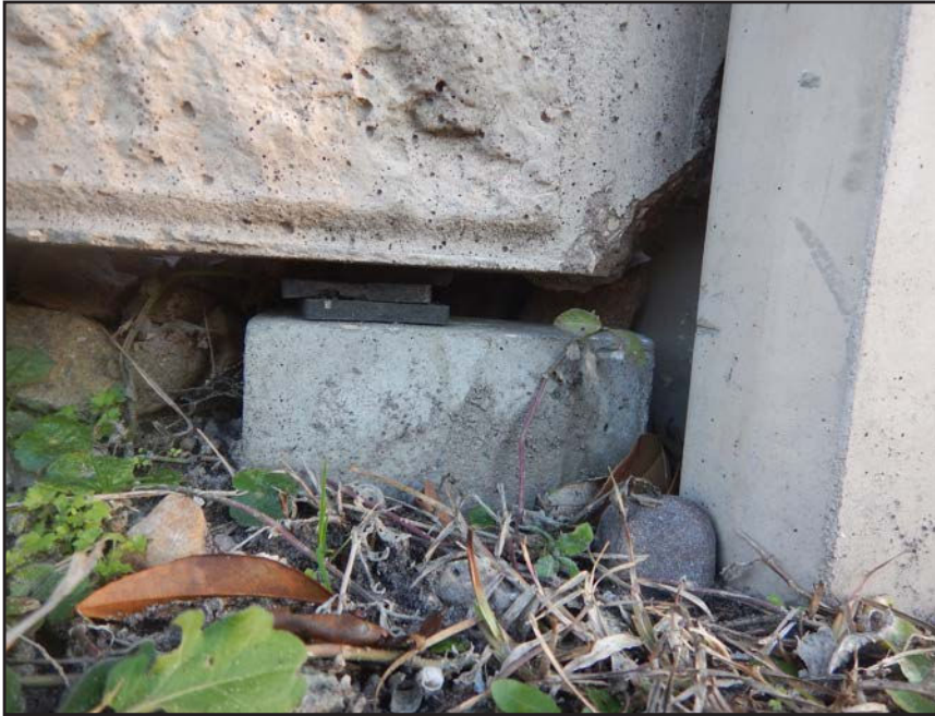
NO. 384 - COLUMN 60SS - CRACKED AND FAILED TONGUE OF A PRECAST WALL PANEL IN A PRECAST COLUMN
