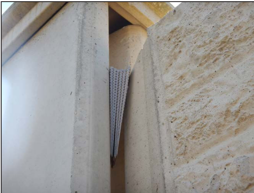
NO. 266 - COLUMN 11NM - INADEQUATE SHIMS STABILIZING A WALL PANEL TO COLUMN CONNECTION AT EXCESSIVE PLAY BETWEEN ADJACENT MEMBERS
