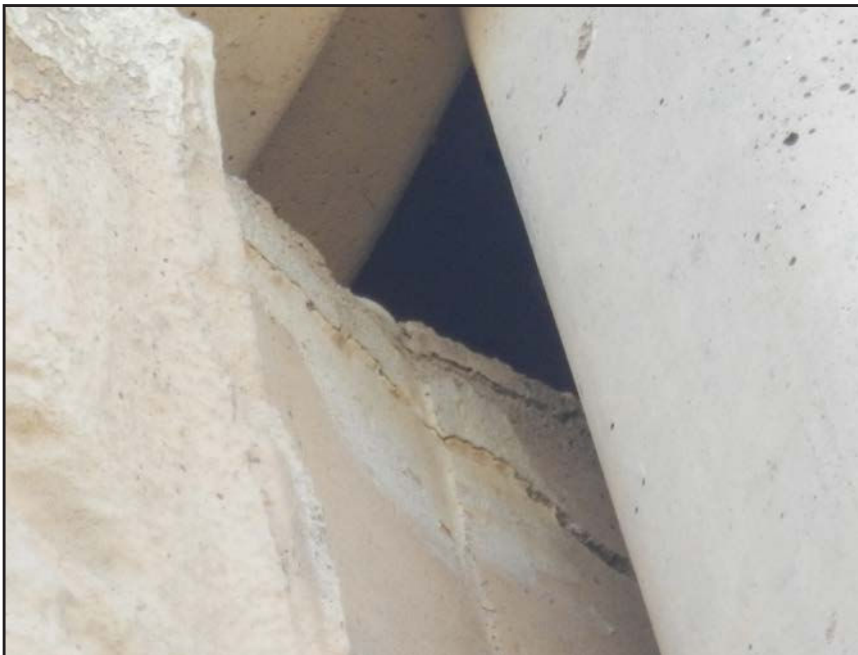
NO. 328 - COLUMN 54S - CRACKED AND FAILED TONGUE OF A PRECAST WALL PANEL IN A PRECAST COLUMN
