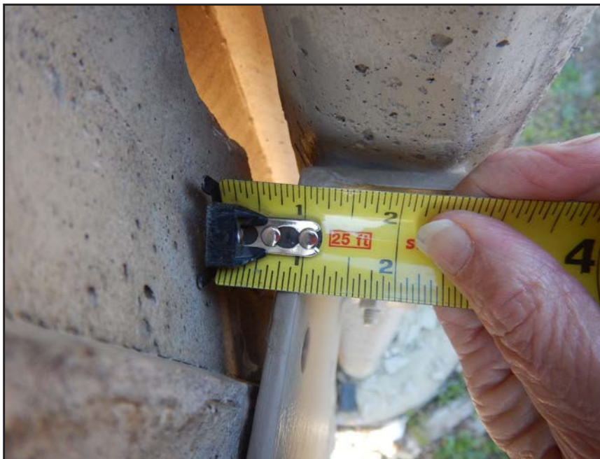
NO. 442 - COLUMN 50N - INADEQUATE ADDED CLIP ANGLE CONNECTION AT A DEFICIENT WALL PANEL TO COLUMN CONNECTION
