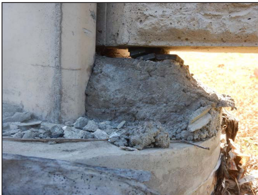
NO. 72 - COLUMN 10NM - INADEQUATE BEARING OF A PRECAST WALL PANEL ON A 2" x 2" NEOPRENE BEARING PAD
