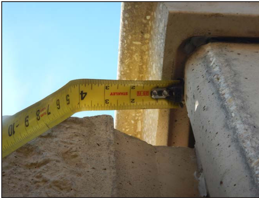
NO. 202 - COLUMN 7NM - INSUFFICIENT SEATING OF A PRECAST WALL PANEL IN A PRECAST COLUMN
