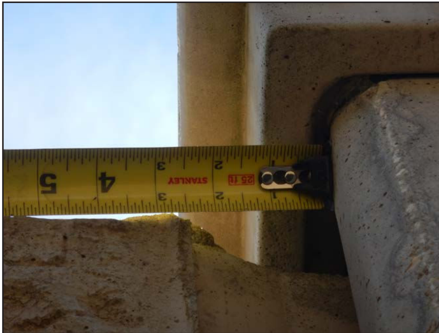
NO. 211 - COLUMN 19SM - INSUFFICIENT SEATING OF A PRECAST WALL PANEL IN A PRECAST COLUMN
