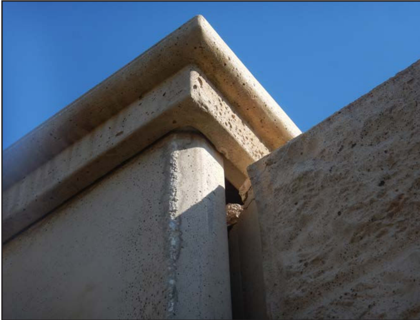
NO. 332 - COLUMN 62S - CRACKED AND FAILED TONGUE OF A PRECAST WALL PANEL IN A PRECAST COLUMN
