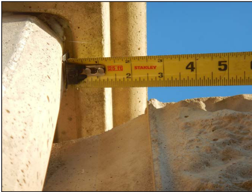
NO. 251 - COLUMN 28SS - INSUFFICIENT SEATING OF A PRECAST WALL PANEL IN A PRECAST COLUMN
