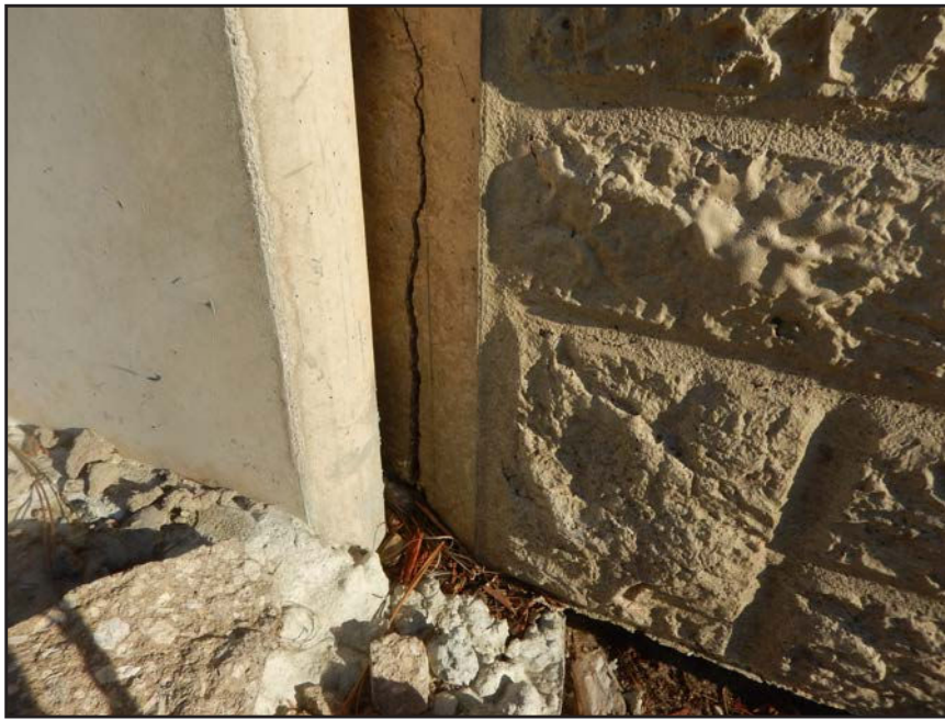
NO. 353 - COLUMN 21SS - CRACKED AND FAILED TONGUE OF A PRECAST WALL PANEL IN A PRECAST COLUMN
