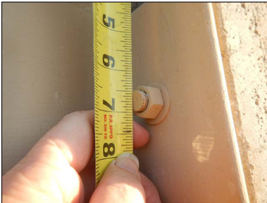
NO. 456 - COLUMN 41SS - INADEQUATE ADDED CLIP ANGLE CONNECTION AT A DEFICIENT WALL PANEL TO COLUMN CONNECTION
