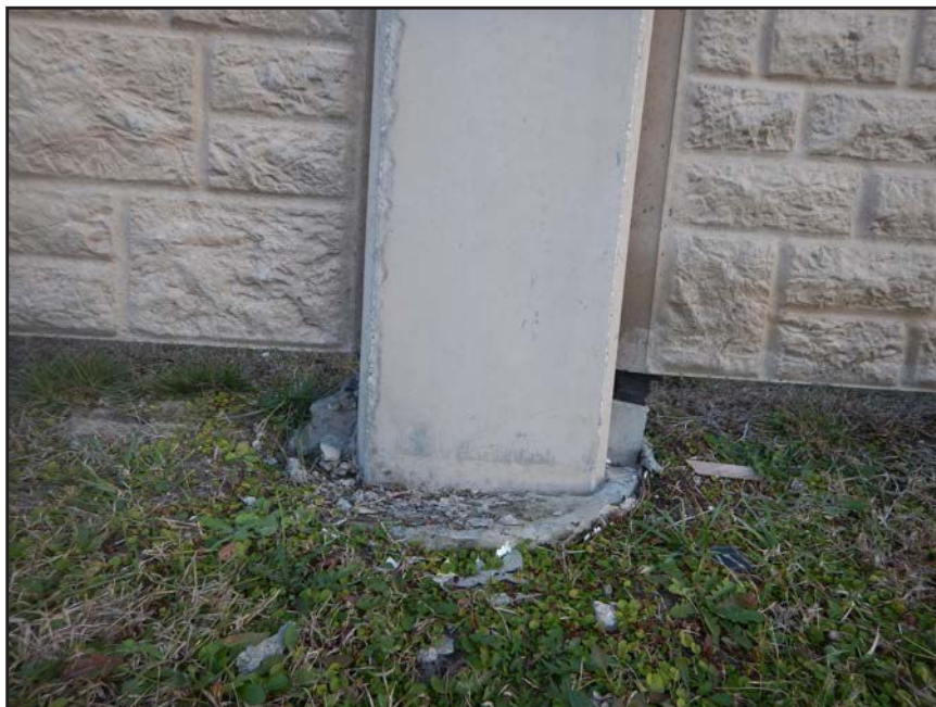
NO. 100 - COLUMN 67SS - INADEQUATE BEARING OF A PRECAST WALL PANEL ON A 2" x 2" NEOPRENE BEARING PAD
