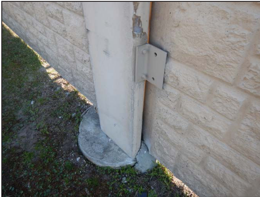
NO. 445 - COLUMN 55S - INADEQUATE ADDED CLIP ANGLE CONNECTION AT A DEFICIENT WALL PANEL TO COLUMN CONNECTION
