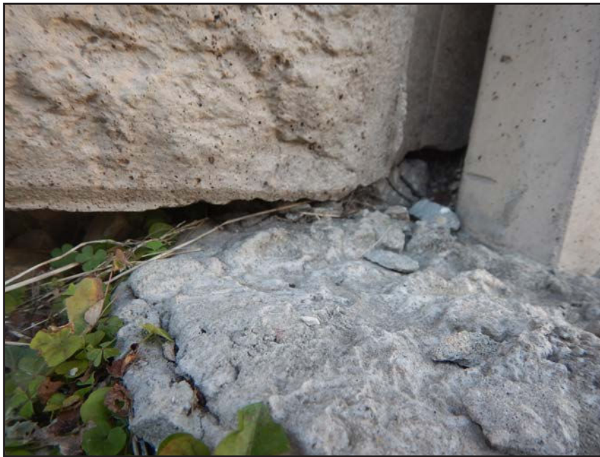
NO. 176 - COLUMN 64SS - INADEQUATE BEARING OF A PRECAST WALL PANEL ON A FAILED GROUT PEDESTAL OR A FAILED PRECAST TONGUE
