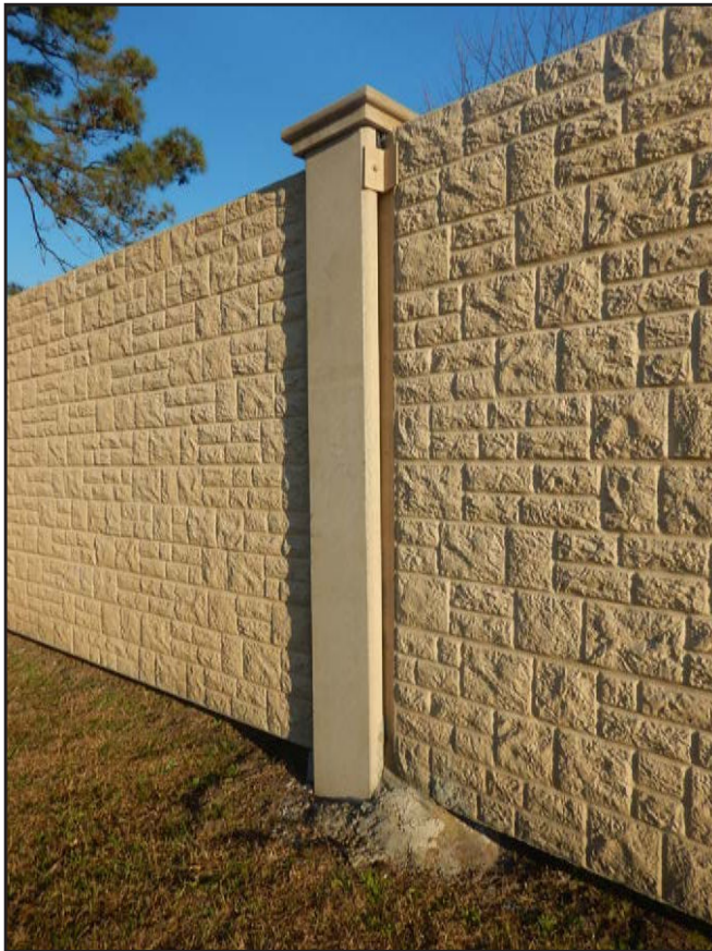
NO. 447 - COLUMN 40SS - INADEQUATE ADDED CLIP ANGLE CONNECTION AT A DEFICIENT WALL PANEL TO COLUMN CONNECTION
