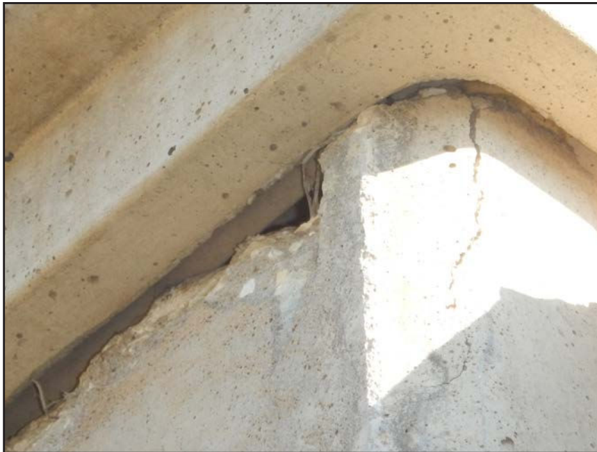
NO. 471 - COLUMN 75S - CRACKED AND SPALLED PRECAST CONCRETE
