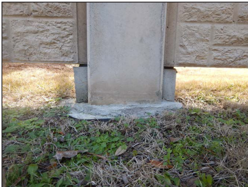
NO. 82 - COLUMN 15SM - INADEQUATE BEARING OF A PRECAST WALL PANEL ON A 2" x 2" NEOPRENE BEARING PAD
