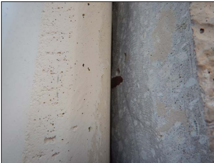
NO. 507 - COLUMN 79SS - EXPOSED REINFORCING STEEL WITH INADEQUATE CONCRETE COVER
