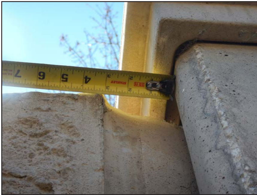
NO. 199 - COLUMN 2NM - INSUFFICIENT SEATING OF A PRECAST WALL PANEL IN A PRECAST COLUMN
