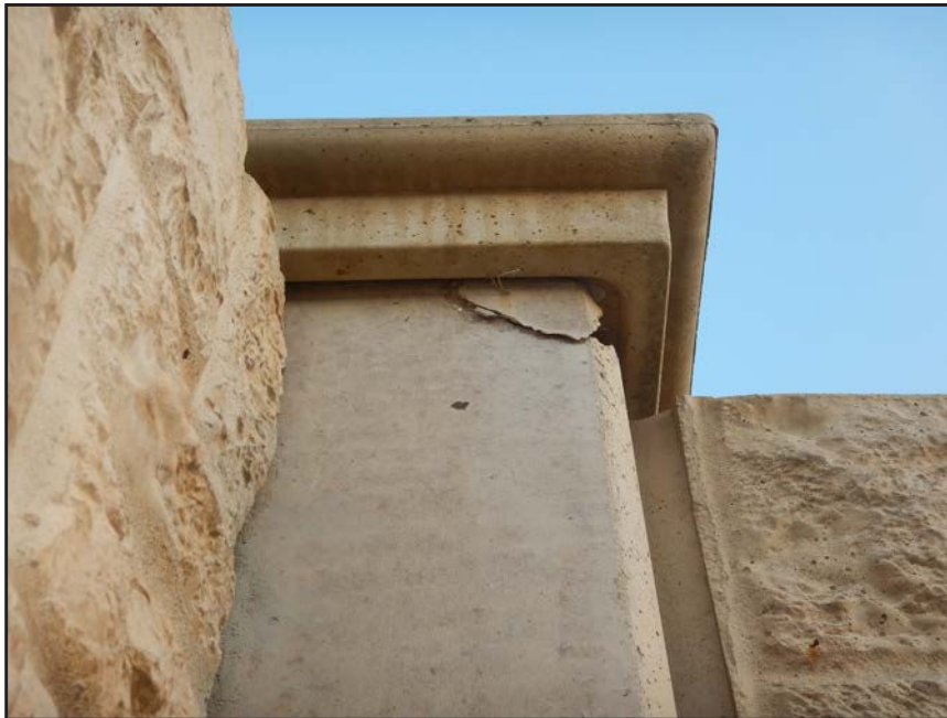
NO. 489 - COLUMN 68SS (BACK) - CRACKED AND SPALLED PRECAST CONCRETE
