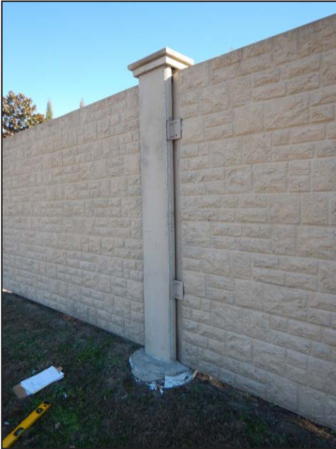
NO. 409 - COLUMN 6N - INADEQUATE ADDED CLIP ANGLE CONNECTION AT A DEFICIENT WALL PANEL TO COLUMN CONNECTION
