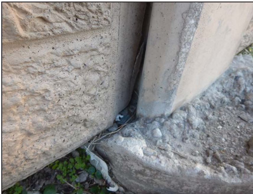
NO. 380 - COLUMN 59SS - CRACKED AND FAILED TONGUE OF A PRECAST WALL PANEL IN A PRECAST COLUMN
