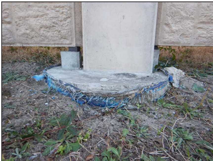
NO. 66 - COLUMN 11N - INADEQUATE BEARING OF A PRECAST WALL PANEL ON A 2" x 2" NEOPRENE BEARING PAD
