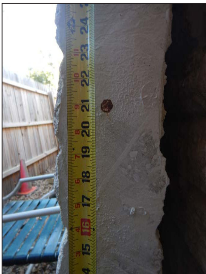
NO. 47 - SAW CUT STORED EXCESS WALL PANEL - TYPICAL HORIZONTAL REINFORCING BARS
