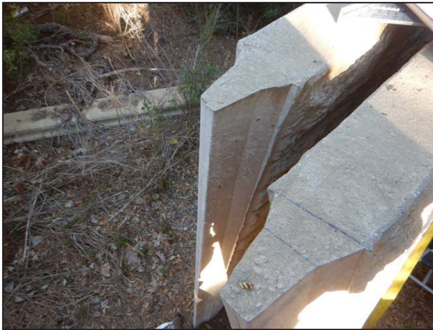
NO. 29 - STORED EXCESS WALL PANELS - TYPICAL TONGUE DIMENSIONS
