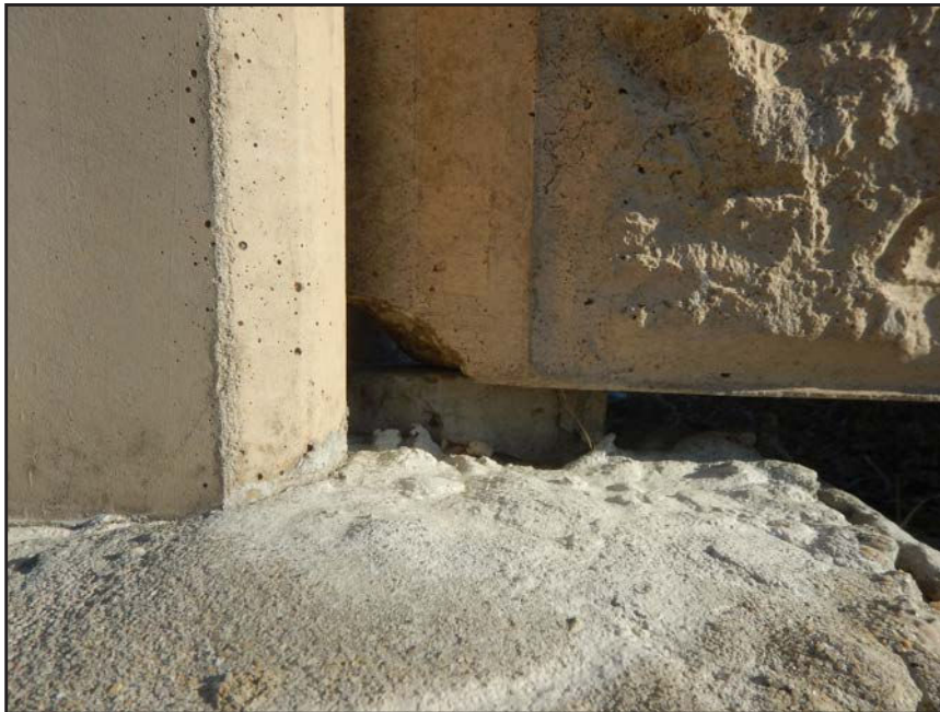
NO. 161 - COLUMN 16SS - INADEQUATE BEARING OF A PRECAST WALL PANEL ON A FAILED GROUT PEDESTAL OR A FAILED PRECAST TONGUE
