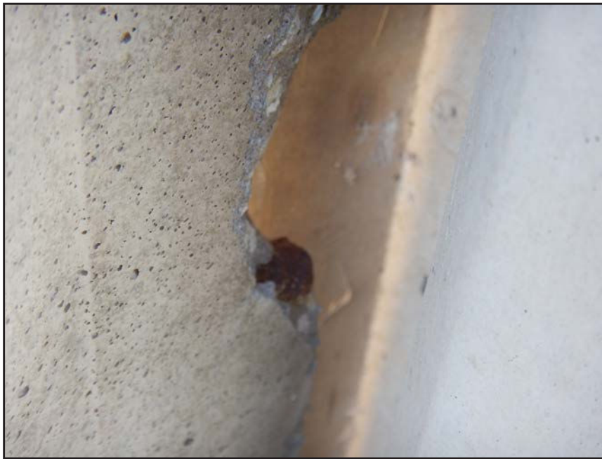
NO. 497 - COLUMN 11NM - EXPOSED REINFORCING STEEL WITH INADEQUATE CONCRETE COVER
