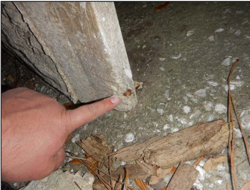
NO. 41 - STORED EXCESS WALL PANEL - TONGUE REINFORCING STEEL WITH INADEQUATE CONCRETE COVER
