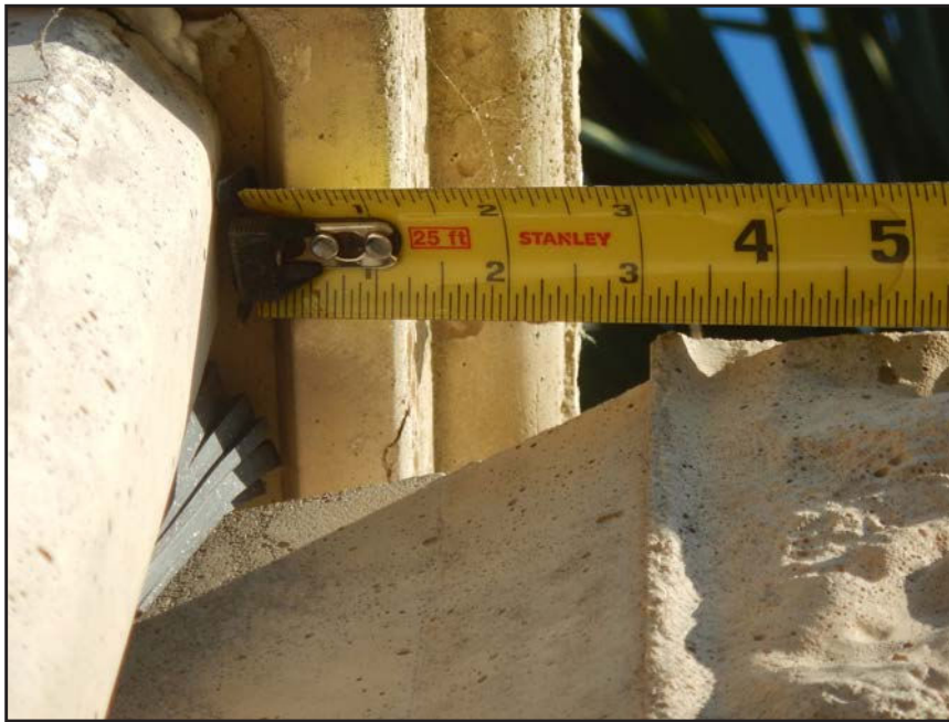
NO. 246 - COLUMN 6SS - INSUFFICIENT SEATING OF A PRECAST WALL PANEL IN A PRECAST COLUMN
