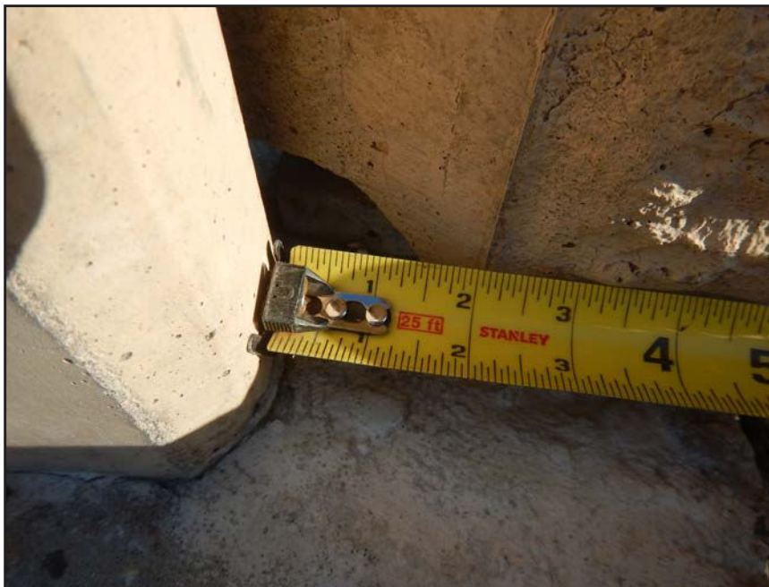
NO. 162 - COLUMN 16SS - INADEQUATE BEARING OF A PRECAST WALL PANEL ON A FAILED GROUT PEDESTAL OR A FAILED PRECAST TONGUE
