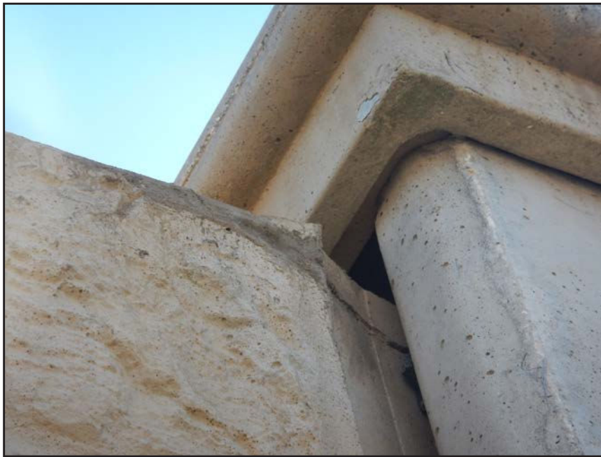
NO. 329 - COLUMN 56S - CRACKED AND FAILED TONGUE OF A PRECAST WALL PANEL IN A PRECAST COLUMN
