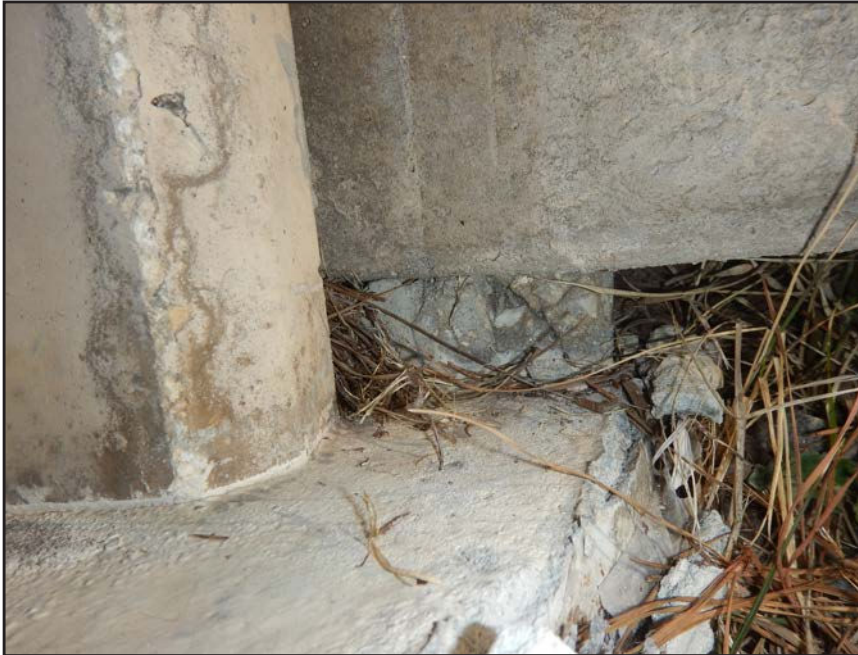
NO. 166 - COLUMN 27SS - INADEQUATE BEARING OF A PRECAST WALL PANEL ON A FAILED GROUT PEDESTAL OR A FAILED PRECAST TONGUE
