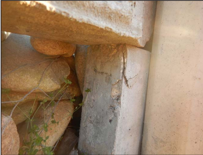
NO. 174 - COLUMN 50SS - INADEQUATE BEARING OF A PRECAST WALL PANEL ON A FAILED GROUT PEDESTAL OR A FAILED PRECAST TONGUE
