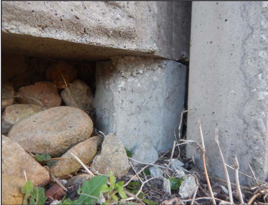
NO. 179 - COLUMN 66SS - INADEQUATE BEARING OF A PRECAST WALL PANEL ON A FAILED GROUT PEDESTAL OR A FAILED PRECAST TONGUE
