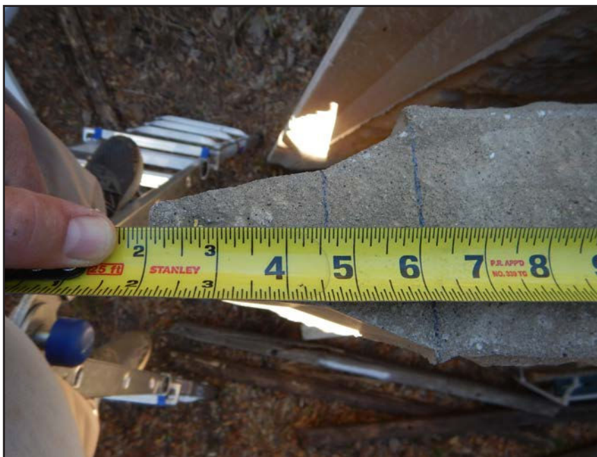
NO. 31 - STORED EXCESS WALL PANELS - TYPICAL TONGUE DIMENSIONS
