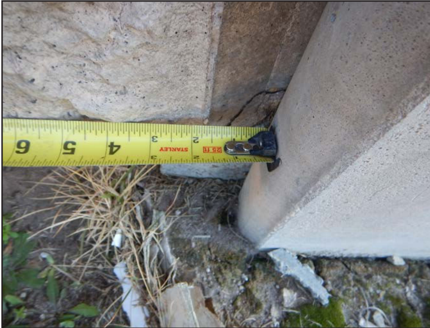
NO. 291 - COLUMN 33N - CRACKED AND FAILED TONGUE OF A PRECAST WALL PANEL IN A PRECAST COLUMN
