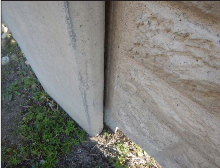
NO. 319 - COLUMN 15S - CRACKED AND FAILED TONGUE OF A PRECAST WALL PANEL IN A PRECAST COLUMN
