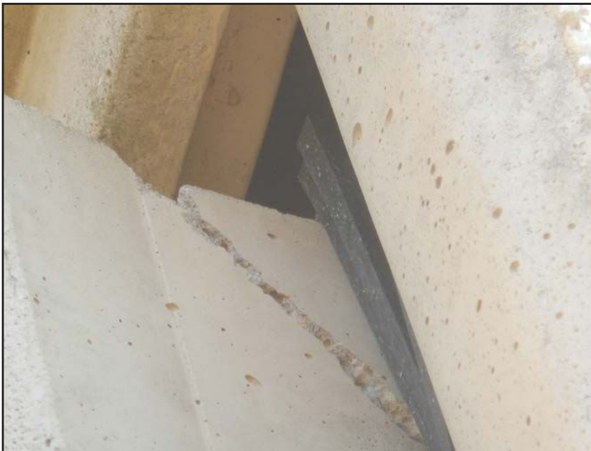
NO. 343 - COLUMN 6SS - CRACKED AND FAILED TONGUE OF A PRECAST WALL PANEL IN A PRECAST COLUMN
