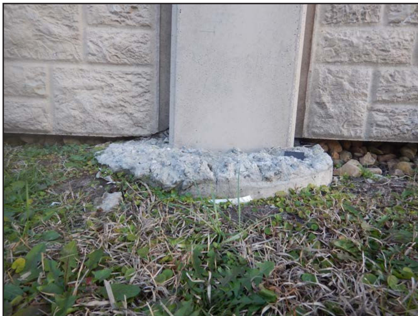
NO. 97 - COLUMN 64SS - INADEQUATE BEARING OF A PRECAST WALL PANEL ON A 2" x 2" NEOPRENE BEARING PAD
