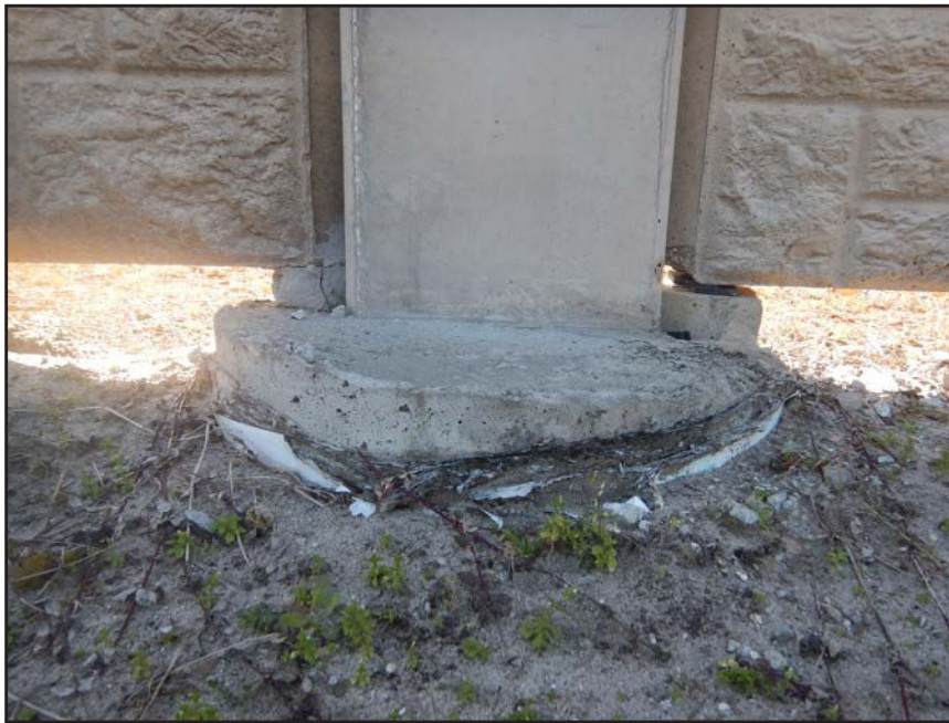
NO. 115 - COLUMN 55N - INADEQUATE BEARING OF A PRECAST WALL PANEL ON A FAILED GROUT PEDESTAL OR A FAILED PRECAST TONGUE
