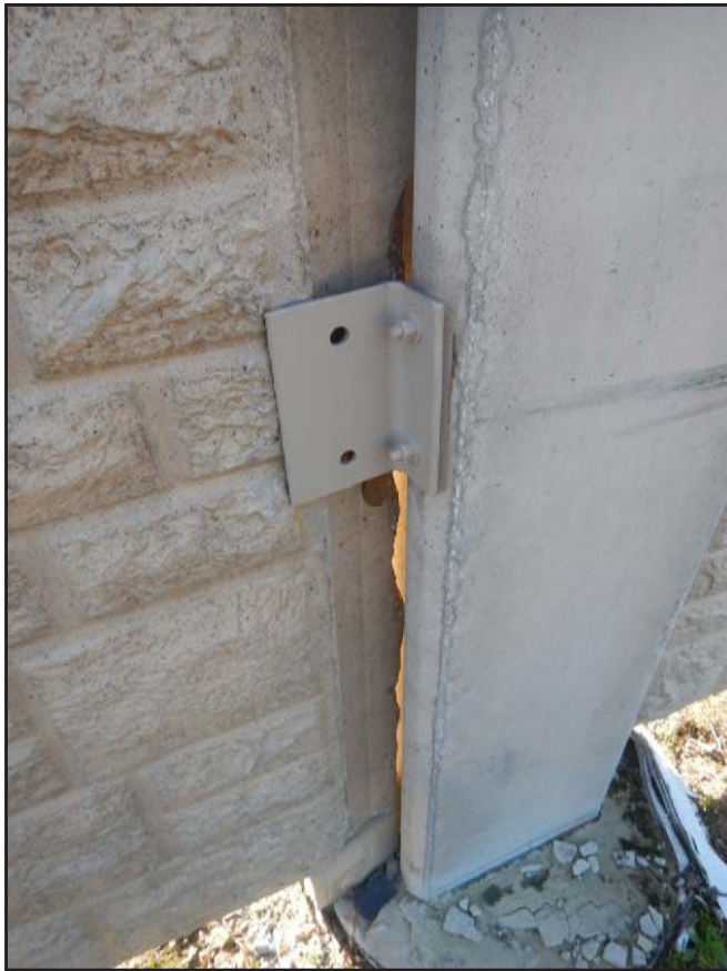
NO. 299 - COLUMN 50N - CRACKED AND FAILED TONGUE OF A PRECAST WALL PANEL IN A PRECAST COLUMN
