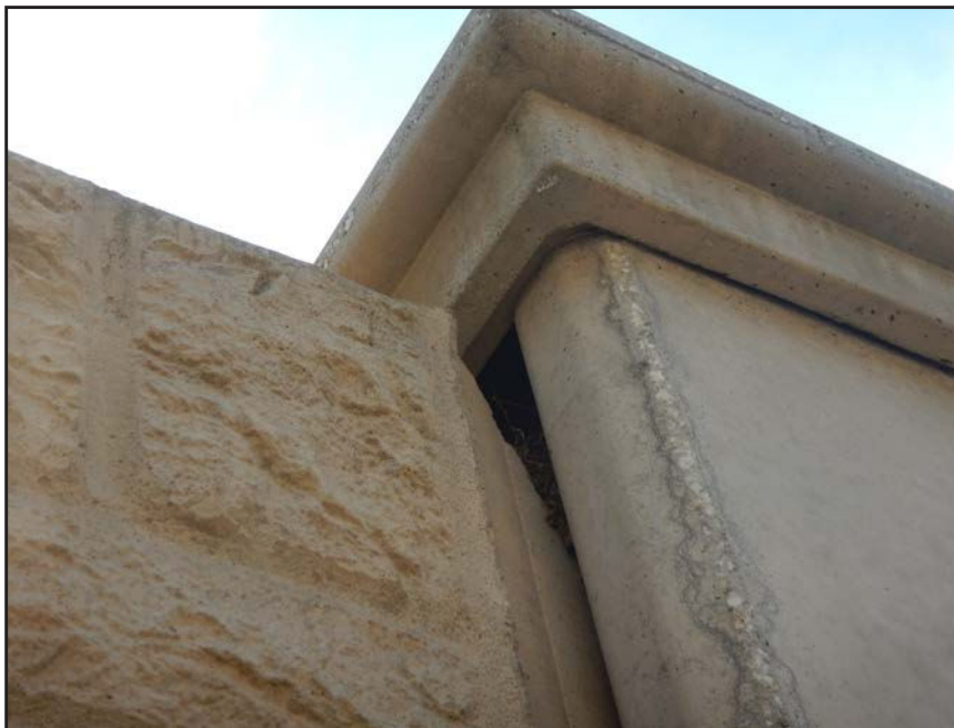
NO. 316 - COLUMN 3S - CRACKED AND FAILED TONGUE OF A PRECAST WALL PANEL IN A PRECAST COLUMN
