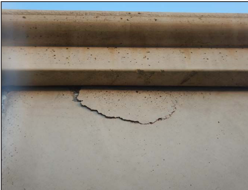
NO. 487 - COLUMN 64SS - CRACKED AND SPALLED PRECAST CONCRETE
