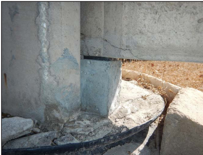
NO. 123 - COLUMN 4S - INADEQUATE BEARING OF A PRECAST WALL PANEL ON A FAILED GROUT PEDESTAL OR A FAILED PRECAST TONGUE
