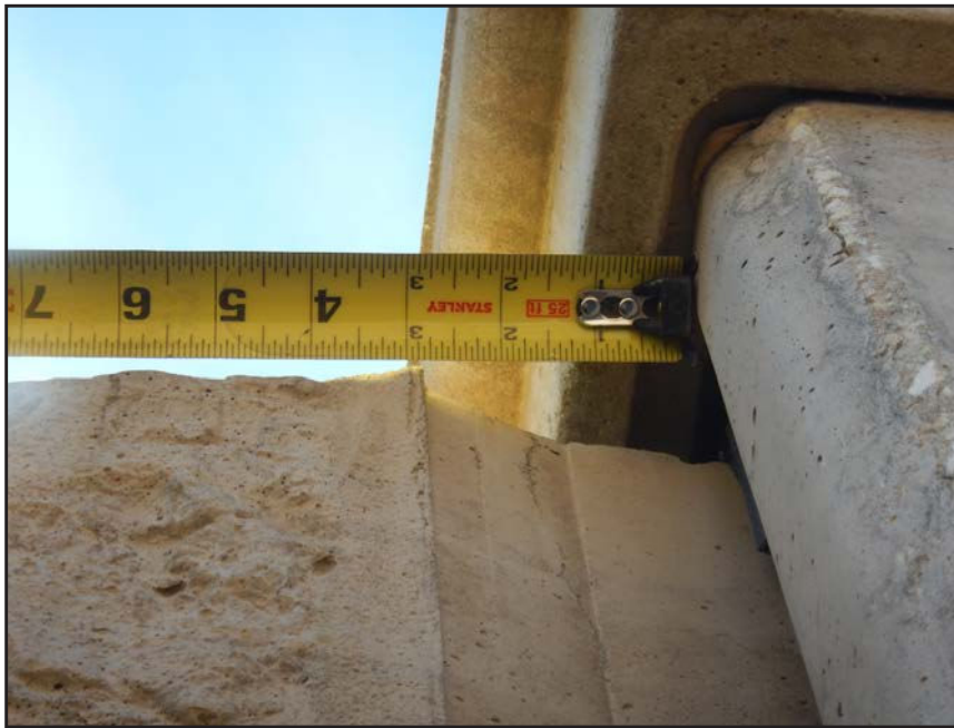
NO. 196 - COLUMN 57N - INSUFFICIENT SEATING OF A PRECAST WALL PANEL IN A PRECAST COLUMN
