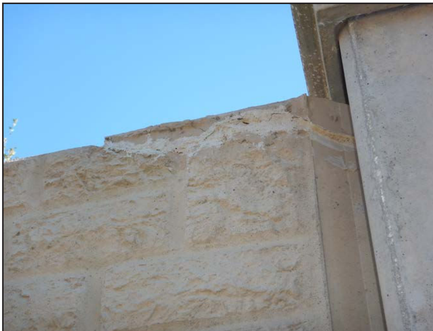
NO. 461 - COLUMN 30N - CRACKED AND SPALLED PRECAST CONCRETE
