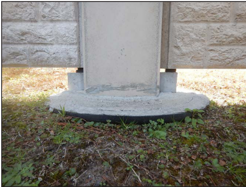
NO. 79 - COLUMN 3SM - INADEQUATE BEARING OF A PRECAST WALL PANEL ON A 2" x 2" NEOPRENE BEARING PAD
