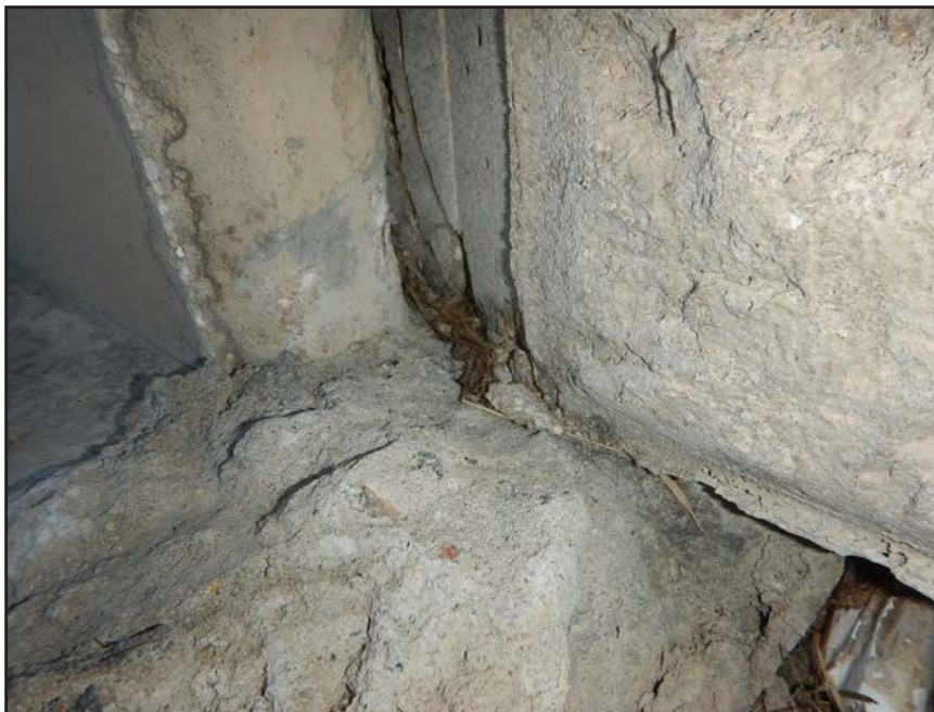
NO. 339 - COLUMN 70S - CRACKED AND FAILED TONGUE OF A PRECAST WALL PANEL IN A PRECAST COLUMN
