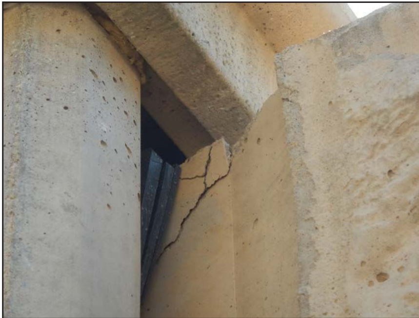
NO. 315 - COLUMN 16SM - CRACKED AND FAILED TONGUE OF A PRECAST WALL PANEL IN A PRECAST COLUMN
