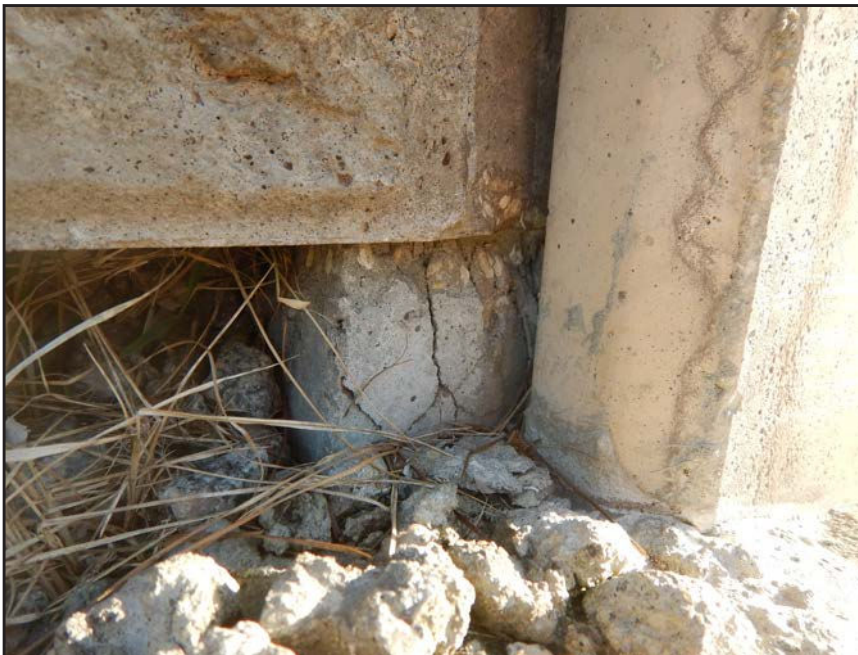
NO. 167 - COLUMN 29SS - INADEQUATE BEARING OF A PRECAST WALL PANEL ON A FAILED GROUT PEDESTAL OR A FAILED PRECAST TONGUE
