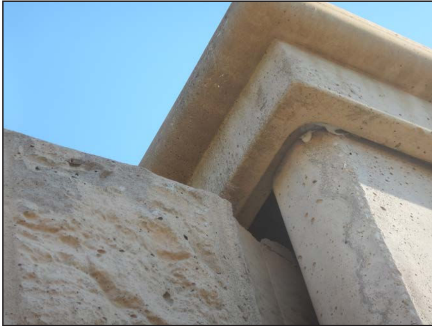
NO. 348 - COLUMN 16SS - CRACKED AND FAILED TONGUE OF A PRECAST WALL PANEL IN A PRECAST COLUMN
