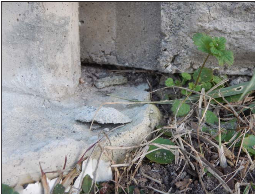
NO. 182 - COLUMN 71SS - INADEQUATE BEARING OF A PRECAST WALL PANEL ON A FAILED GROUT PEDESTAL OR A FAILED PRECAST TONGUE
