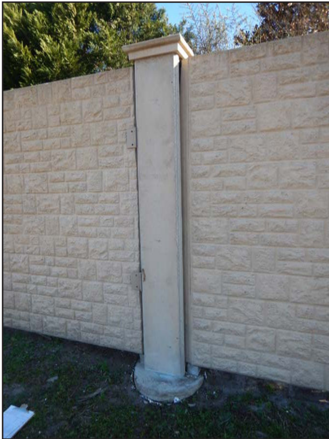
NO. 420 - COLUMN 14N - INADEQUATE ADDED CLIP ANGLE CONNECTION AT A DEFICIENT WALL PANEL TO COLUMN CONNECTION
