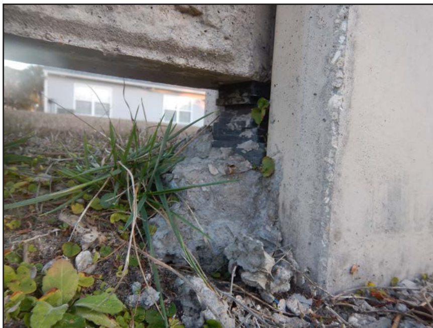
NO. 101 - COLUMN 67SS - INADEQUATE BEARING OF A PRECAST WALL PANEL ON A 2" x 2" NEOPRENE BEARING PAD
