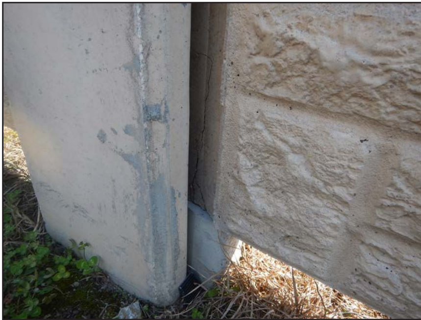
NO. 321 - COLUMN 19S - CRACKED AND FAILED TONGUE OF A PRECAST WALL PANEL IN A PRECAST COLUMN
