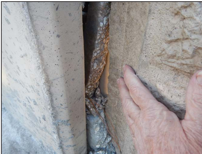
NO. 313 - COLUMN 13NM - CRACKED AND FAILED TONGUE OF A PRECAST WALL PANEL IN A PRECAST COLUMN
