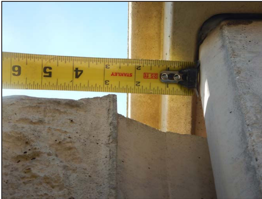
NO. 203 - COLUMN 9NM - INSUFFICIENT SEATING OF A PRECAST WALL PANEL IN A PRECAST COLUMN
