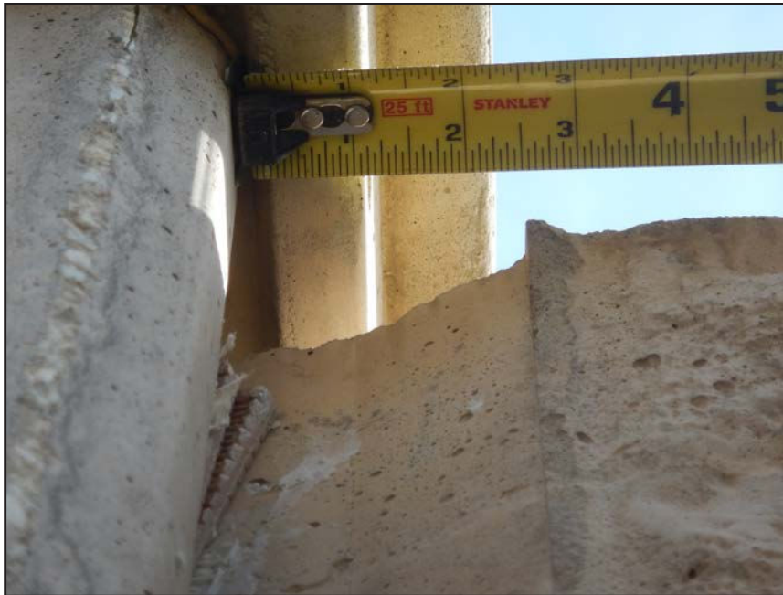
NO. 217 - COLUMN 13S - INSUFFICIENT SEATING OF A PRECAST WALL PANEL IN A PRECAST COLUMN
