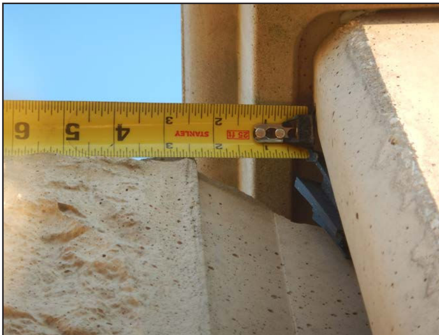
NO. 286 - COLUMN 50SS - INADEQUATE SHIMS STABILIZING A WALL PANEL TO COLUMN CONNECTION AT EXCESSIVE PLAY BETWEEN ADJACENT MEMBERS
