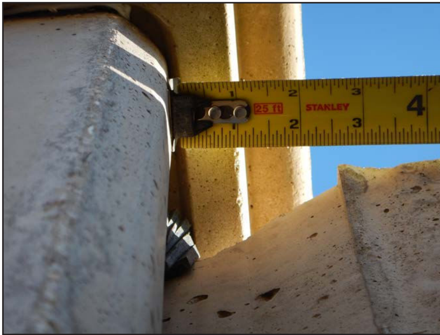
NO. 183 - COLUMN 3N - INSUFFICIENT SEATING OF A PRECAST WALL PANEL IN A PRECAST COLUMN
