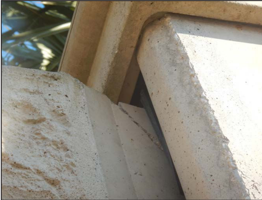
NO. 342 - COLUMN 6SS - CRACKED AND FAILED TONGUE OF A PRECAST WALL PANEL IN A PRECAST COLUMN
