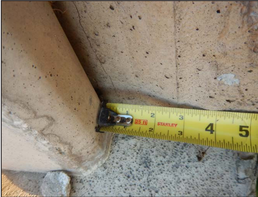
NO. 376 - COLUMN 47SS - CRACKED AND FAILED TONGUE OF A PRECAST WALL PANEL IN A PRECAST COLUMN
