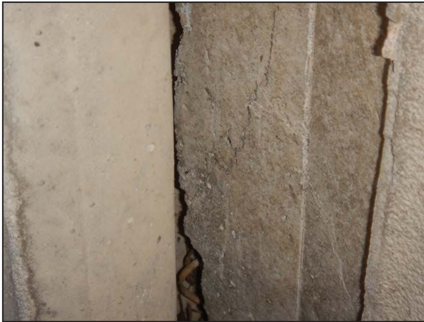
NO. 397 - COLUMN 76SS - CRACKED AND FAILED TONGUE OF A PRECAST WALL PANEL IN A PRECAST COLUMN
