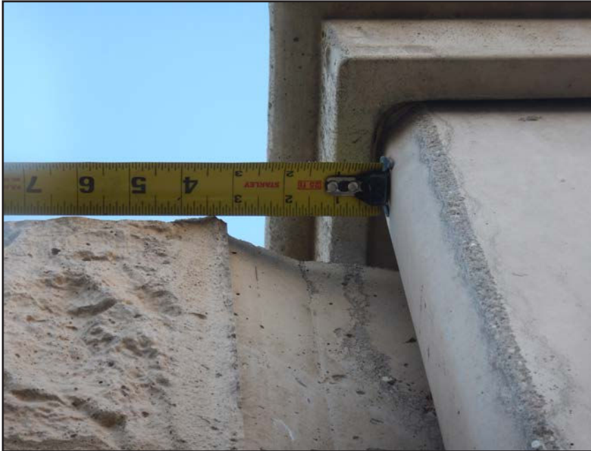
NO. 260 - COLUMN 71SS - INSUFFICIENT SEATING OF A PRECAST WALL PANEL IN A PRECAST COLUMN
