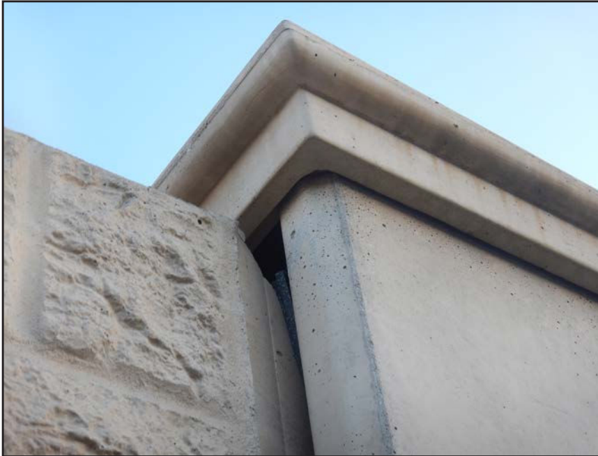
NO. 389 - COLUMN 65SS - CRACKED AND FAILED TONGUE OF A PRECAST WALL PANEL IN A PRECAST COLUMN
