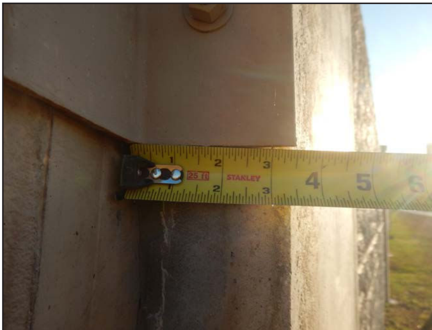
NO. 453 - COLUMN 41SS - INADEQUATE ADDED CLIP ANGLE CONNECTION AT A DEFICIENT WALL PANEL TO COLUMN CONNECTION
