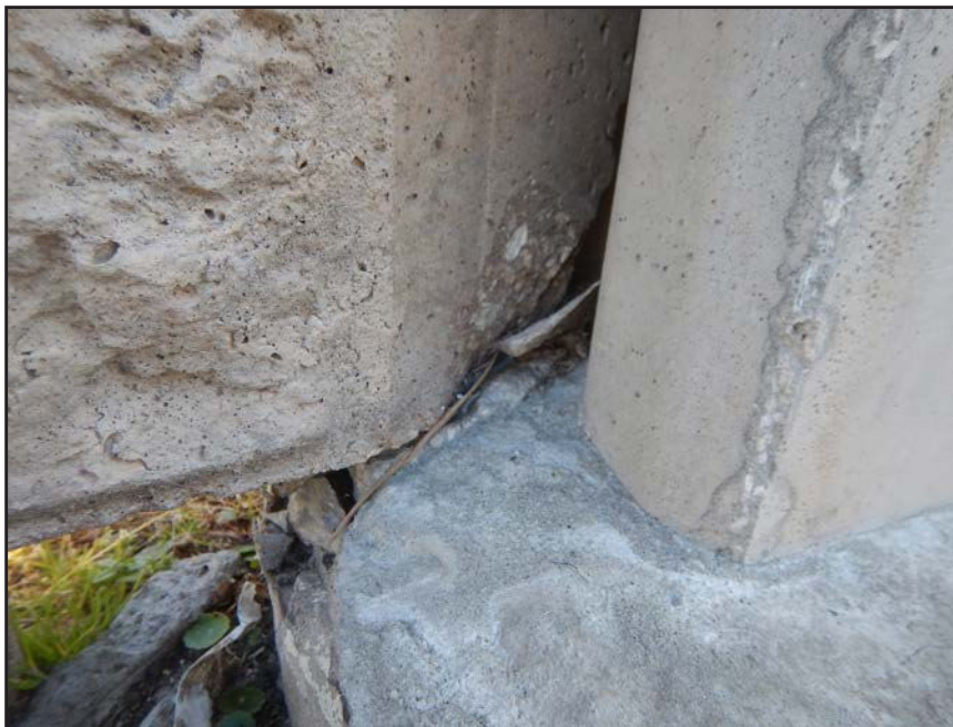
NO. 153 - COLUMN 79S - INADEQUATE BEARING OF A PRECAST WALL PANEL ON A FAILED GROUT PEDESTAL OR A FAILED PRECAST TONGUE
