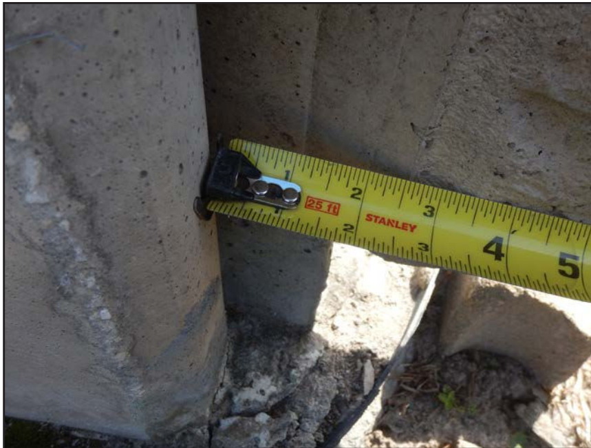
NO. 214 - COLUMN 4S - INSUFFICIENT SEATING OF A PRECAST WALL PANEL IN A PRECAST COLUMN
