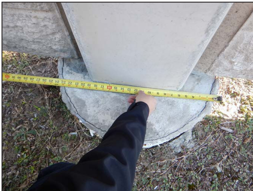
NO. 12 - COLUMN 3N - TYPICAL PRECAST COLUMN FOUNDATION
