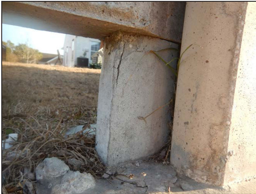
NO. 172 - COLUMN 43SS - INADEQUATE BEARING OF A PRECAST WALL PANEL ON A FAILED GROUT PEDESTAL OR A FAILED PRECAST TONGUE
