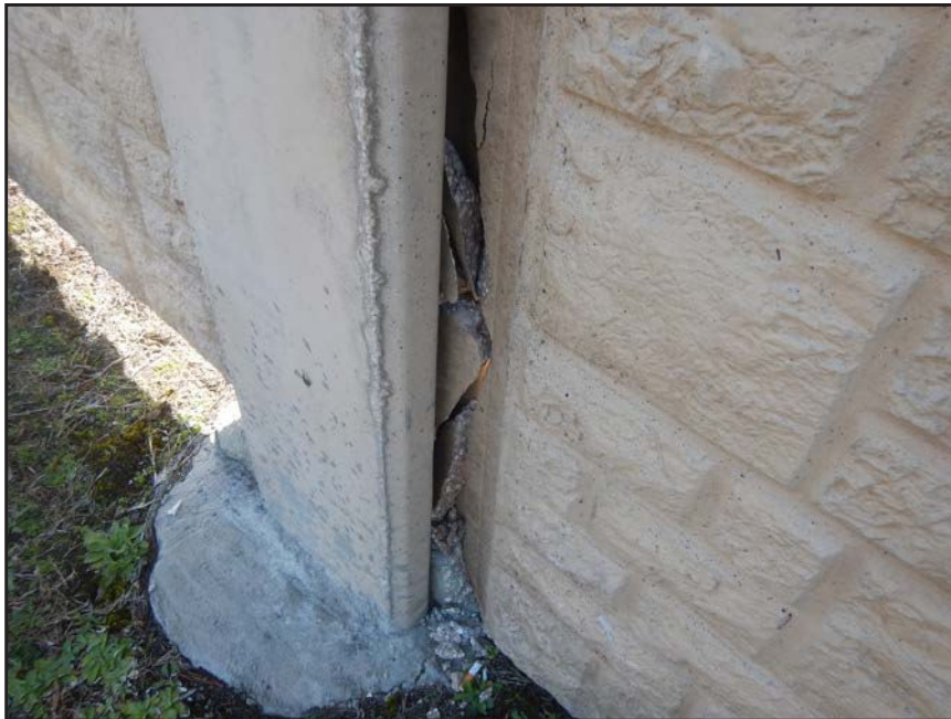
NO. 312 - COLUMN 13NM - CRACKED AND FAILED TONGUE OF A PRECAST WALL PANEL IN A PRECAST COLUMN
