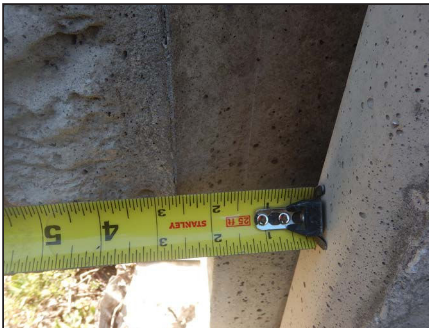
NO. 204 - COLUMN 9NM - INSUFFICIENT SEATING OF A PRECAST WALL PANEL IN A PRECAST COLUMN
