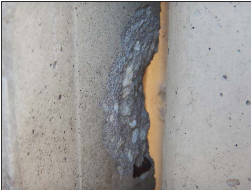
NO. 495 - COLUMN 56N - EXPOSED REINFORCING STEEL WITH INADEQUATE CONCRETE COVER
