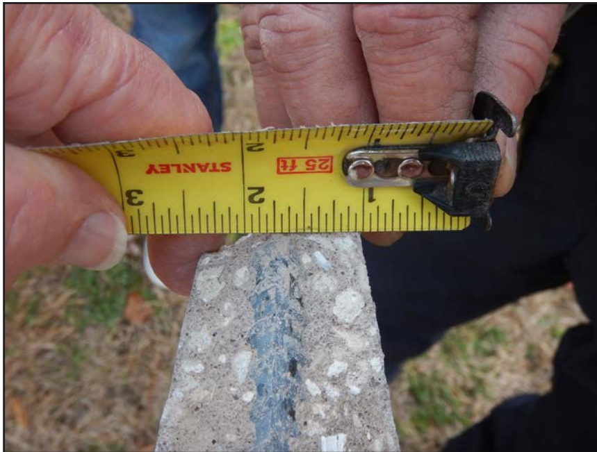
NO. 58 - SPALLED WALL PANEL ON THE SOUTH SIDE OF COLUMN 13NM - TONGUE REINFORCING DOWEL WITH INADEQUATE CONCRETE COVER
