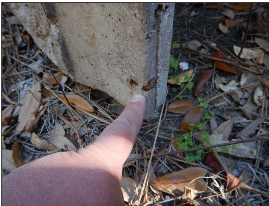
NO. 38 - STORED EXCESS WALL PANEL - TONGUE REINFORCING STEEL WITH INADEQUATE CONCRETE COVER
