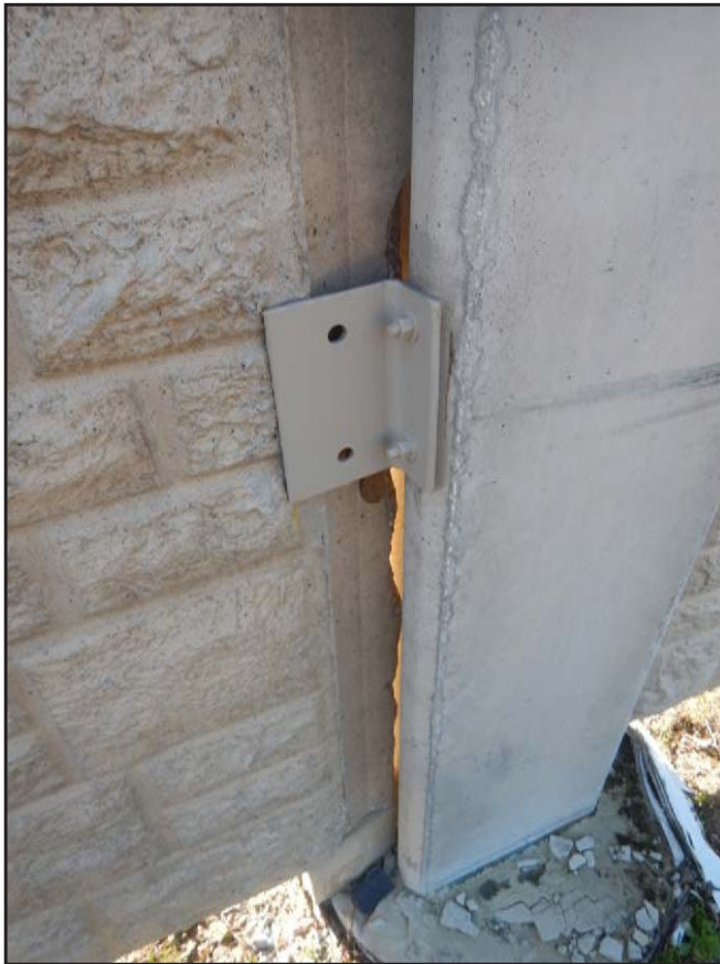
NO. 438 - COLUMN 50N - INADEQUATE ADDED CLIP ANGLE CONNECTION AT A DEFICIENT WALL PANEL TO COLUMN CONNECTION
