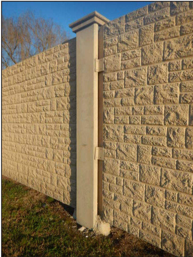
NO. 457 - COLUMN 45SS - INADEQUATE ADDED CLIP ANGLE CONNECTION AT A DEFICIENT WALL PANEL TO COLUMN CONNECTION
