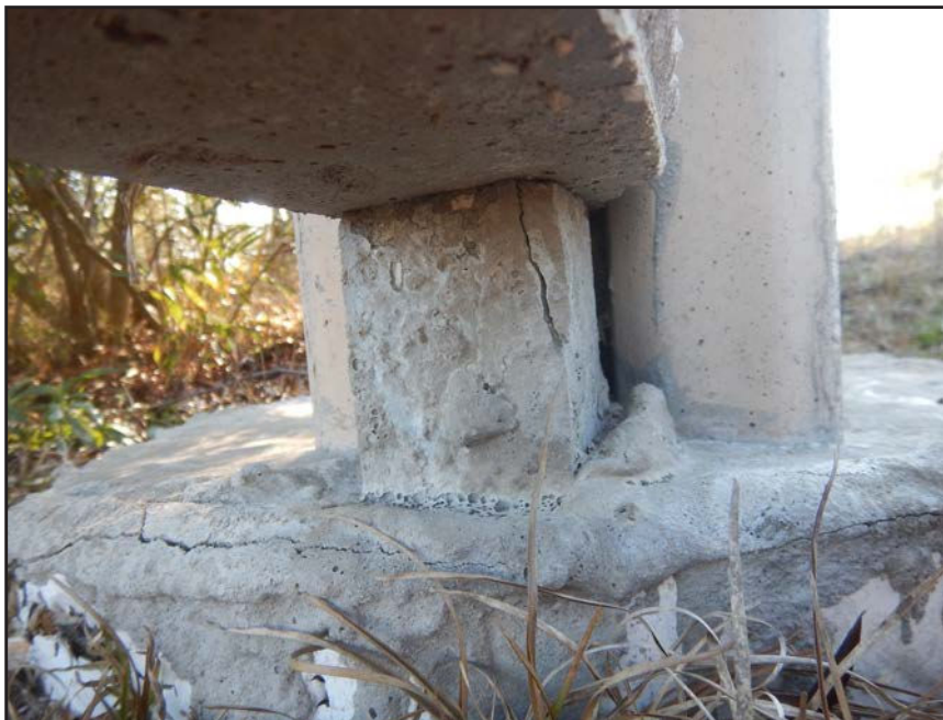
NO. 156 - COLUMN 82S - INADEQUATE BEARING OF A PRECAST WALL PANEL ON A FAILED GROUT PEDESTAL OR A FAILED PRECAST TONGUE
