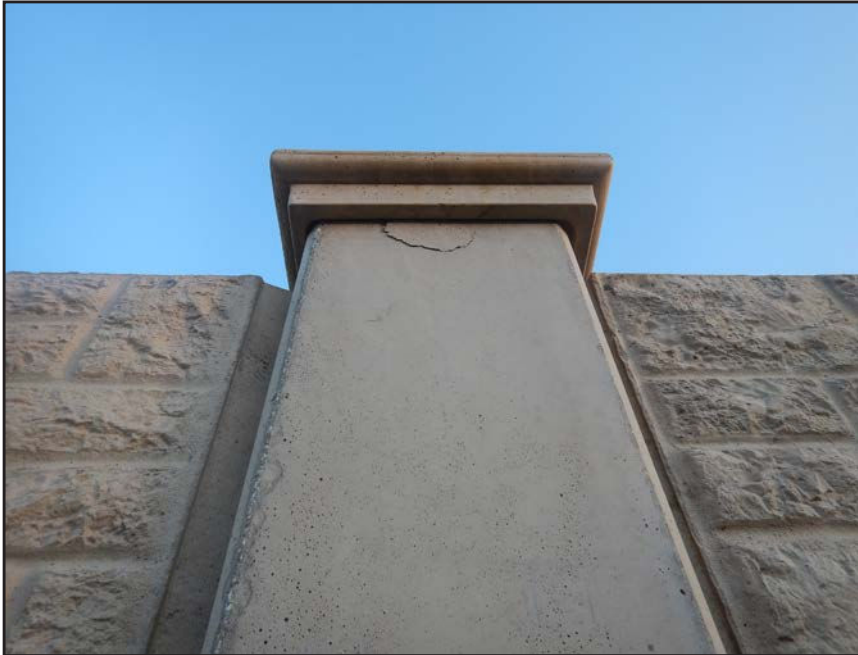
NO. 486 - COLUMN 64SS - CRACKED AND SPALLED PRECAST CONCRETE
