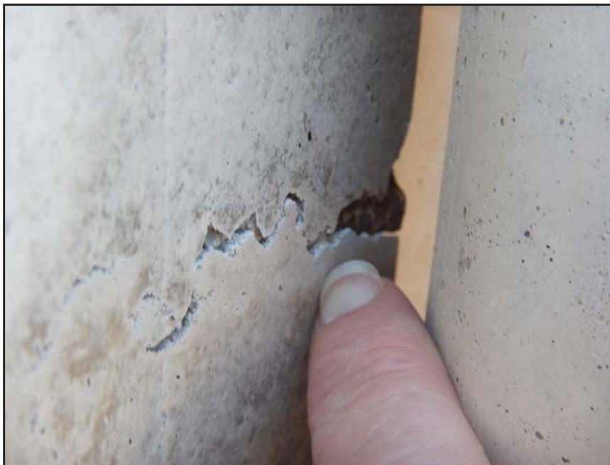
NO. 502 - COLUMN 55S - EXPOSED REINFORCING STEEL WITH INADEQUATE CONCRETE COVER
