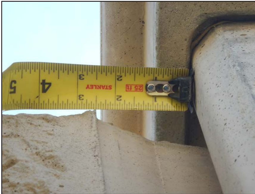
NO. 223 - COLUMN 35S - INSUFFICIENT SEATING OF A PRECAST WALL PANEL IN A PRECAST COLUMN
