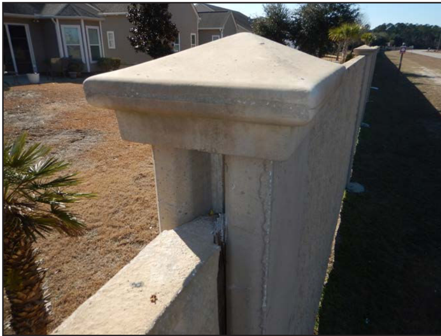
NO. 262 - COLUMN 22N - INADEQUATE SHIMS STABILIZING A WALL PANEL TO COLUMN CONNECTION AT EXCESSIVE PLAY BETWEEN ADJACENT MEMBERS
