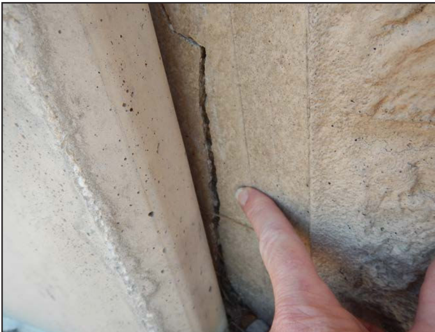
NO. 362 - COLUMN 28SS - CRACKED AND FAILED TONGUE OF A PRECAST WALL PANEL IN A PRECAST COLUMN
