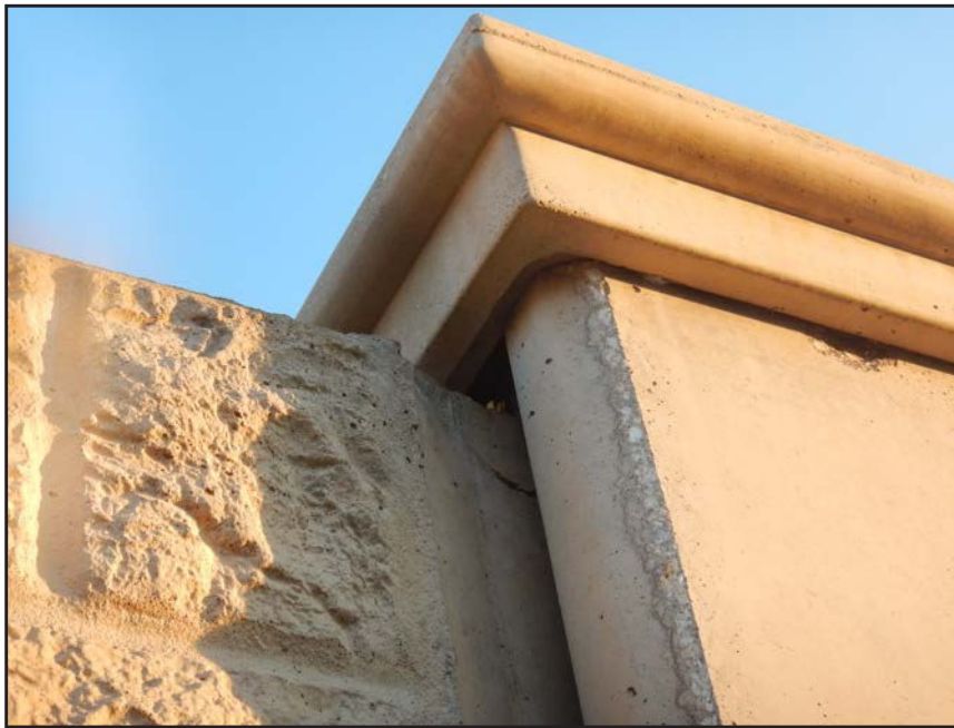
NO. 378 - COLUMN 59SS - CRACKED AND FAILED TONGUE OF A PRECAST WALL PANEL IN A PRECAST COLUMN
