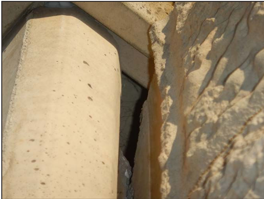
NO. 366 - COLUMN 39SS - CRACKED AND FAILED TONGUE OF A PRECAST WALL PANEL IN A PRECAST COLUMN
