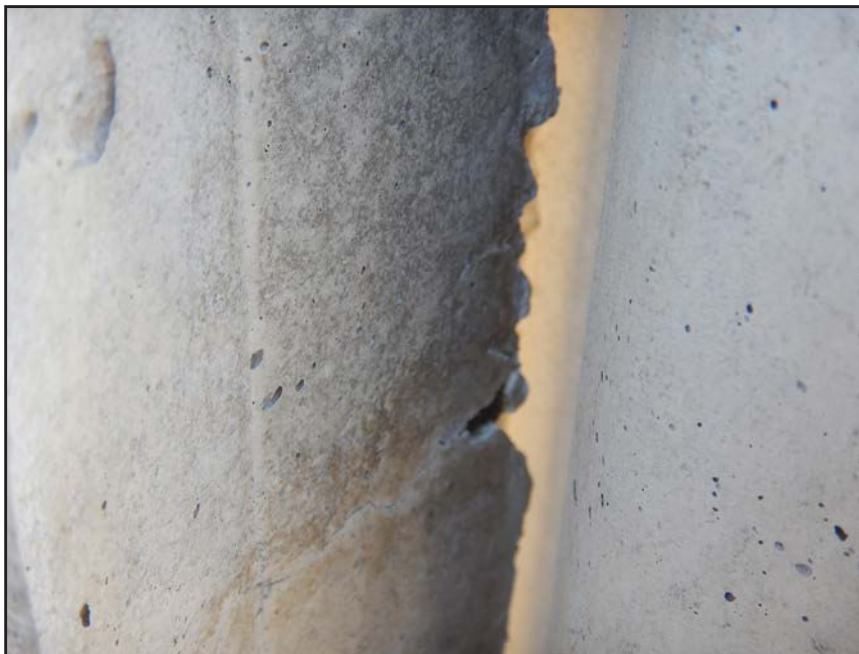
NO. 496 - COLUMN 56N - EXPOSED REINFORCING STEEL WITH INADEQUATE CONCRETE COVER
