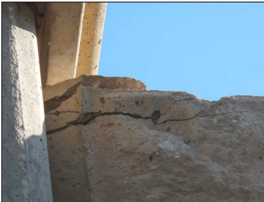
NO. 477 - COLUMN 78S - CRACKED AND SPALLED PRECAST CONCRETE
