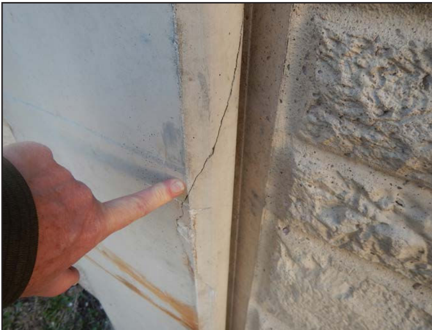
NO. 485 - COLUMN 63SS - CRACKED AND SPALLED PRECAST CONCRETE
