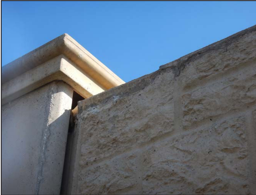
NO. 468 - COLUMN 52S - CRACKED AND SPALLED PRECAST CONCRETE
