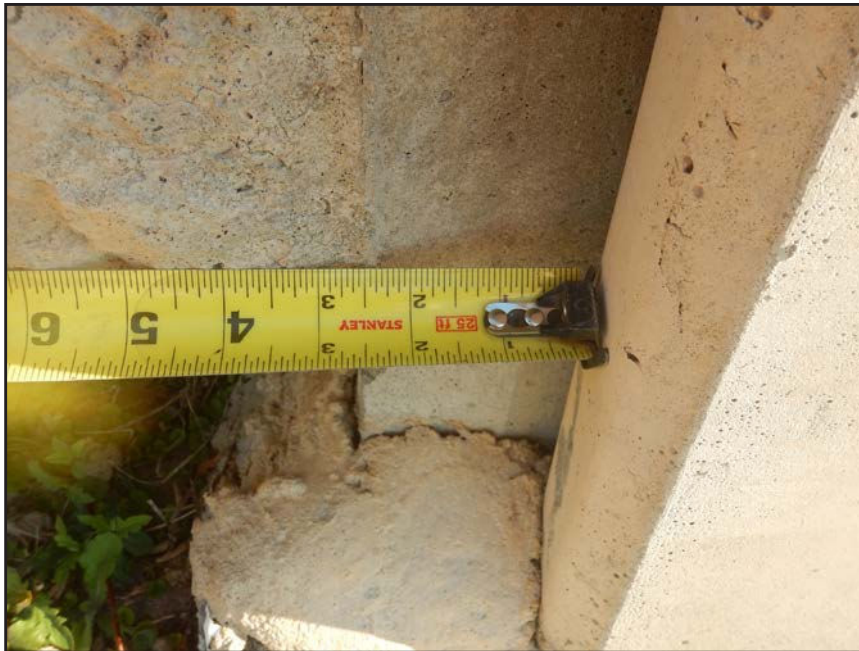
NO. 247 - COLUMN 13SS - INSUFFICIENT SEATING OF A PRECAST WALL PANEL IN A PRECAST COLUMN
