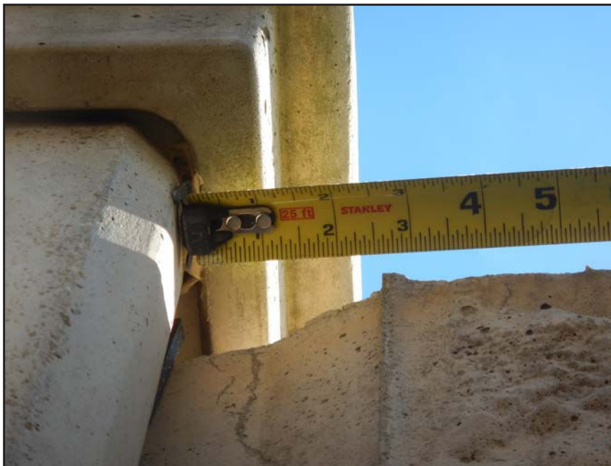
NO. 218 - COLUMN 24S - INSUFFICIENT SEATING OF A PRECAST WALL PANEL IN A PRECAST COLUMN
