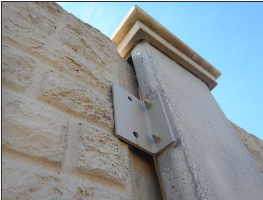
NO. 435 - COLUMN 49N - INADEQUATE ADDED CLIP ANGLE CONNECTION AT A DEFICIENT WALL PANEL TO COLUMN CONNECTION
