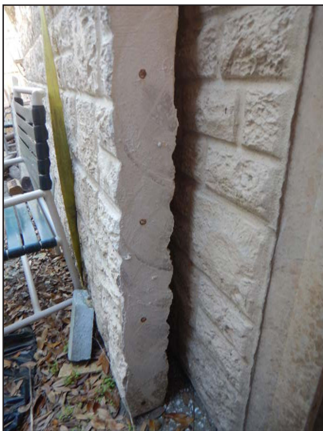
NO. 43 - SAW CUT STORED EXCESS WALL PANEL - TYPICAL HORIZONTAL REINFORCING BARS
