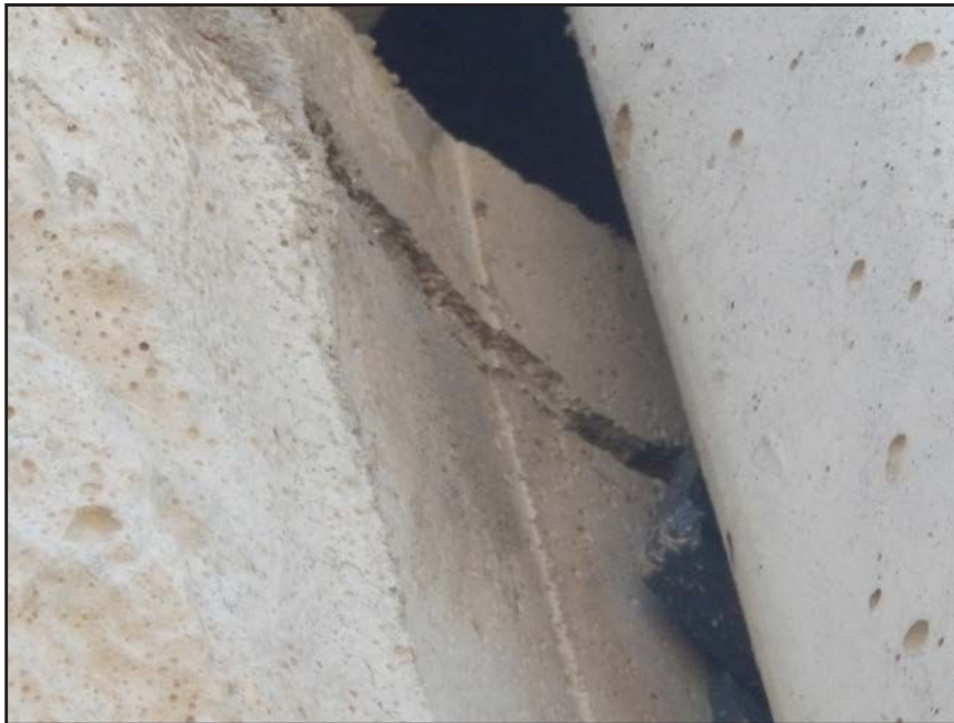
NO. 330 - COLUMN 56S - CRACKED AND FAILED TONGUE OF A PRECAST WALL PANEL IN A PRECAST COLUMN
