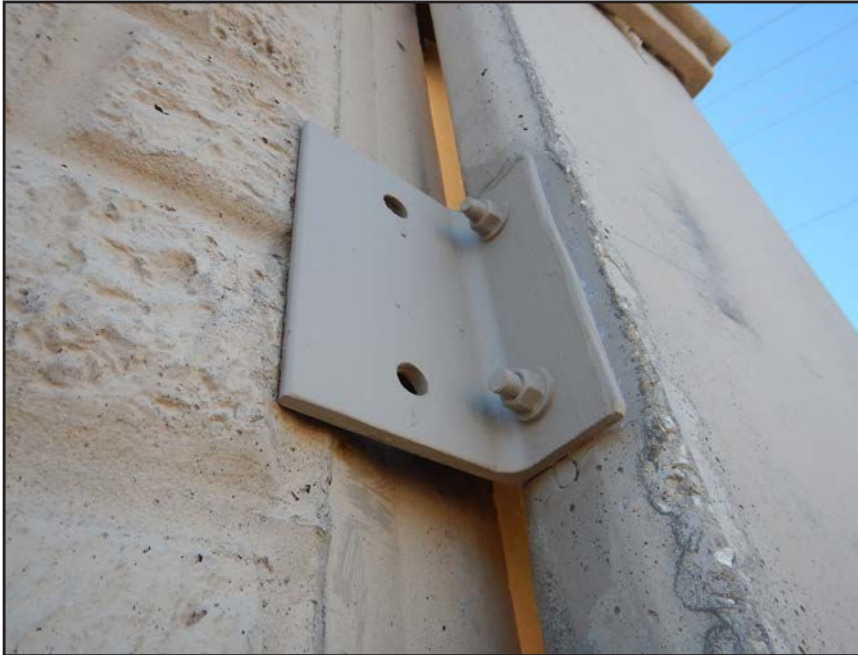
NO. 402 - COLUMN 1NE - INADEQUATE ADDED CLIP ANGLE CONNECTION AT A DEFICIENT WALL PANEL TO COLUMN CONNECTION
