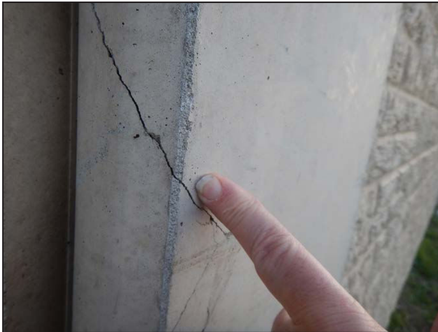
NO. 492 - COLUMN 70SS - CRACKED AND SPALLED PRECAST CONCRETE
