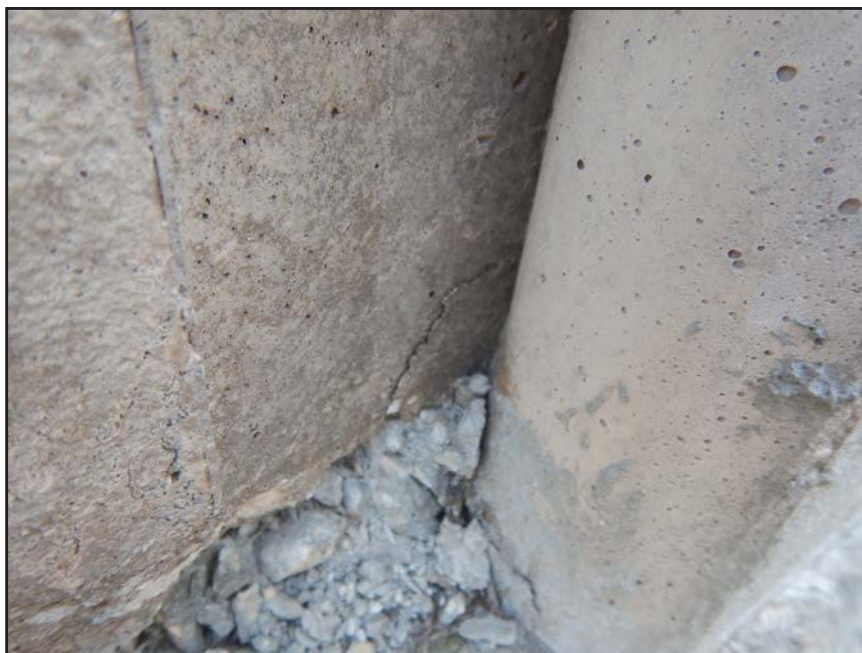
NO. 126 - COLUMN 12S - INADEQUATE BEARING OF A PRECAST WALL PANEL ON A FAILED GROUT PEDESTAL OR A FAILED PRECAST TONGUE
