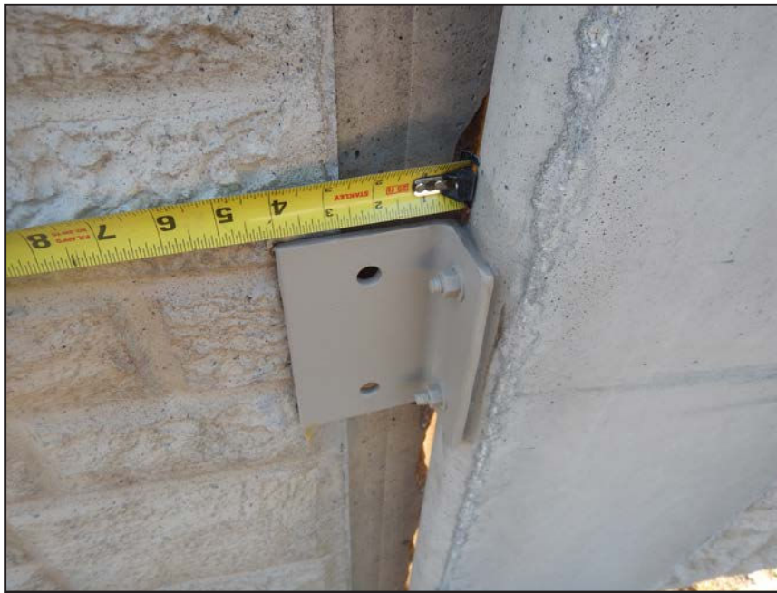
NO. 440 - COLUMN 50N - INADEQUATE ADDED CLIP ANGLE CONNECTION AT A DEFICIENT WALL PANEL TO COLUMN CONNECTION
