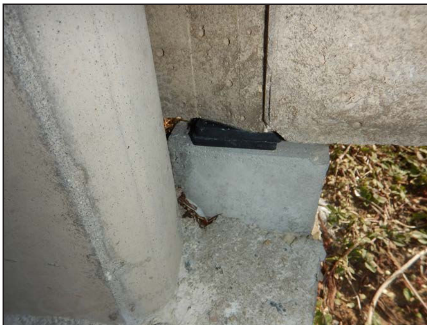
NO. 65 - COLUMN 2N - INADEQUATE BEARING OF A PRECAST WALL PANEL ON A 2" x 2" NEOPRENE BEARING PAD
