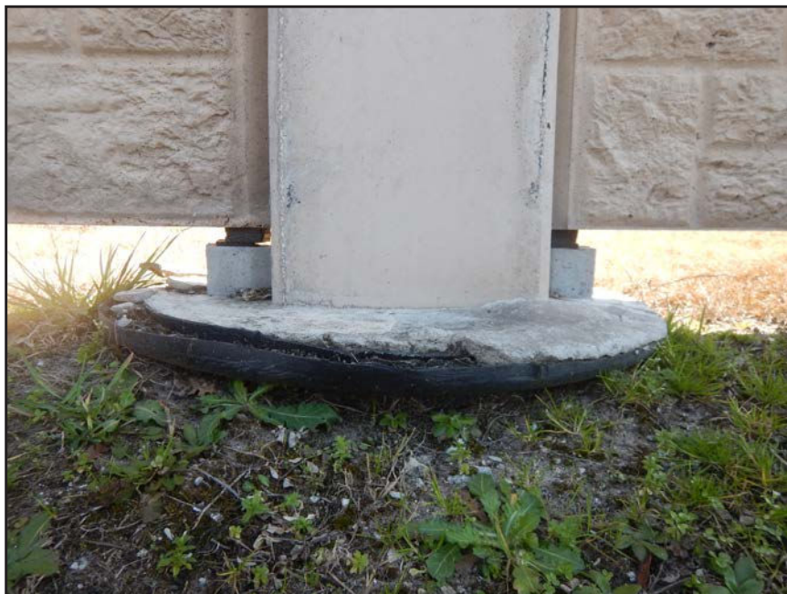
NO. 94 - COLUMN 46S - INADEQUATE BEARING OF A PRECAST WALL PANEL ON A 2" x 2" NEOPRENE BEARING PAD
