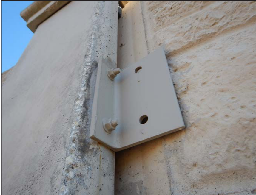
NO. 410 - COLUMN 6N - INADEQUATE ADDED CLIP ANGLE CONNECTION AT A DEFICIENT WALL PANEL TO COLUMN CONNECTION
