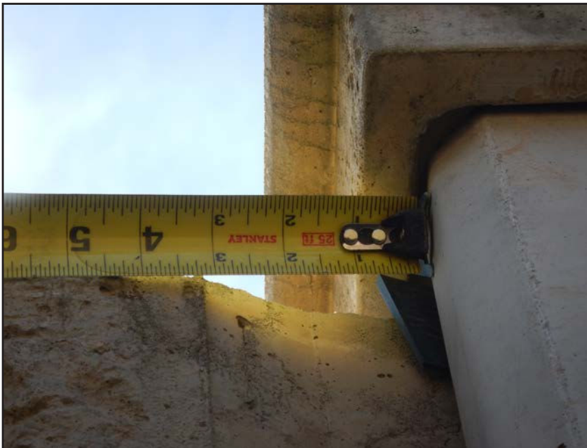
NO. 206 - COLUMN 14NM - INSUFFICIENT SEATING OF A PRECAST WALL PANEL IN A PRECAST COLUMN
