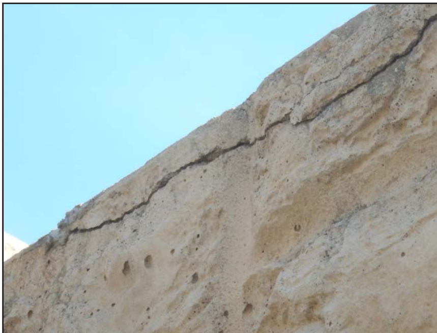
NO. 467 - COLUMN 17S - CRACKED AND SPALLED PRECAST CONCRETE
