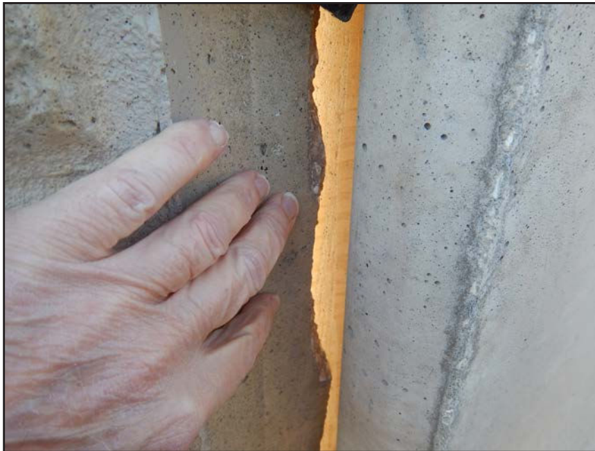
NO. 301 - COLUMN 50N - CRACKED AND FAILED TONGUE OF A PRECAST WALL PANEL IN A PRECAST COLUMN
