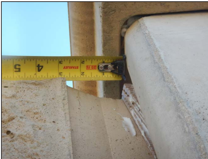
NO. 231 - COLUMN 53S - INSUFFICIENT SEATING OF A PRECAST WALL PANEL IN A PRECAST COLUMN
