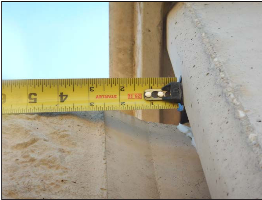
NO. 219 - COLUMN 28S - INSUFFICIENT SEATING OF A PRECAST WALL PANEL IN A PRECAST COLUMN
