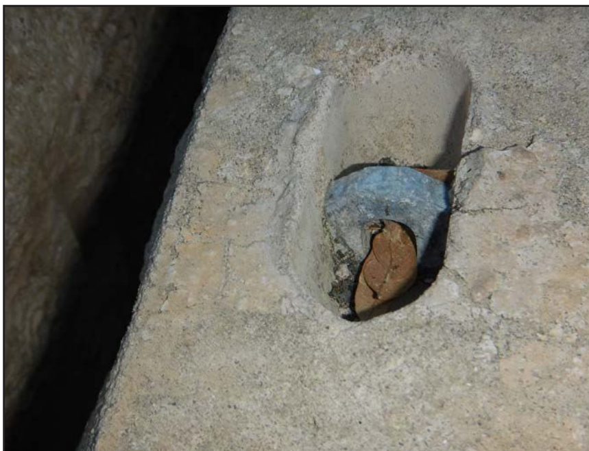
NO. 34 - STORED EXCESS WALL PANELS - TYPICAL LIFTING EYE
