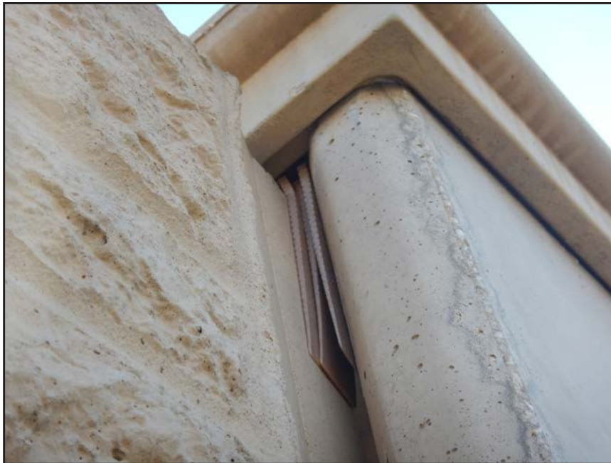
NO. 285 - COLUMN 66S - INADEQUATE SHIMS STABILIZING A WALL PANEL TO COLUMN CONNECTION AT EXCESSIVE PLAY BETWEEN ADJACENT MEMBERS
