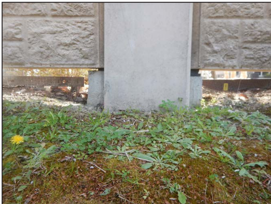
NO. 88 - COLUMN 8S - INADEQUATE BEARING OF A PRECAST WALL PANEL ON A 2" x 2" NEOPRENE BEARING PAD
