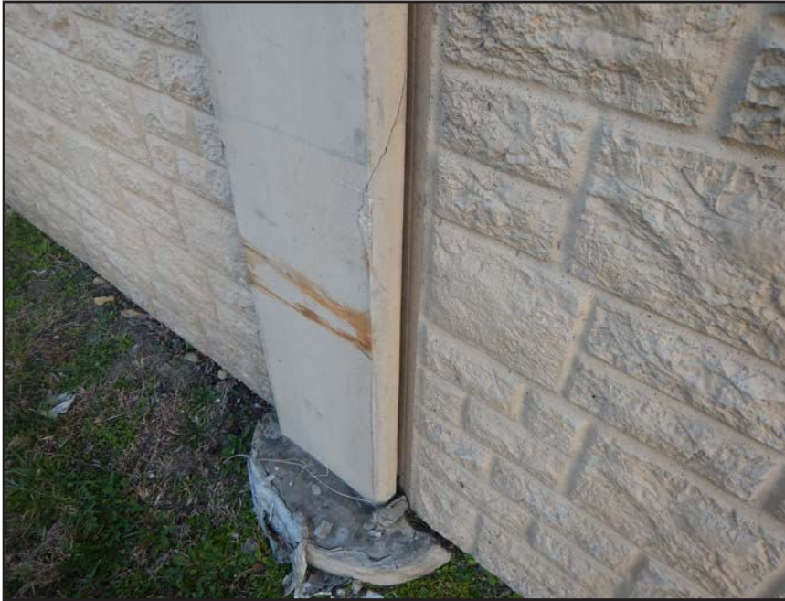
NO. 484 - COLUMN 63SS - CRACKED AND SPALLED PRECAST CONCRETE
