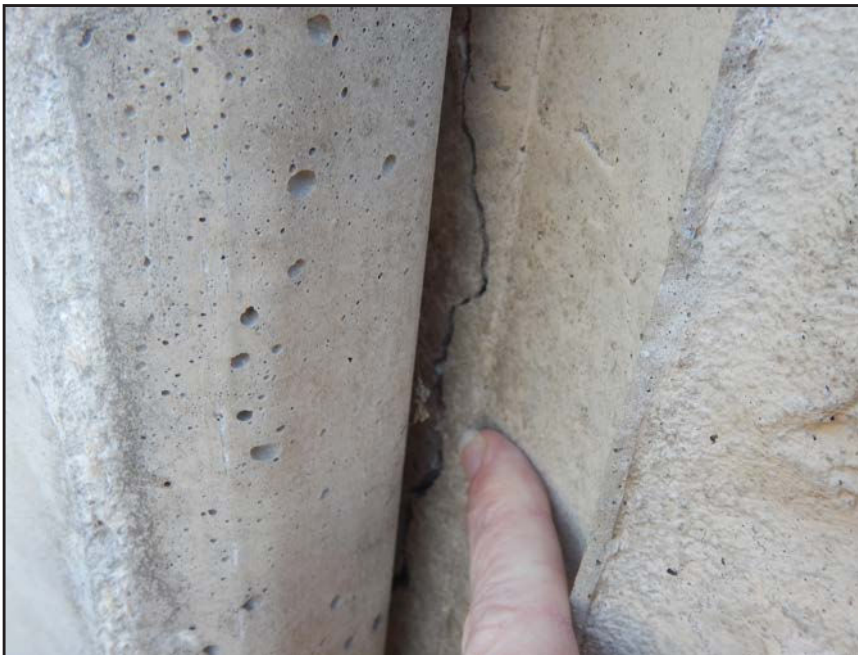
NO. 304 - COLUMN 51N - CRACKED AND FAILED TONGUE OF A PRECAST WALL PANEL IN A PRECAST COLUMN
