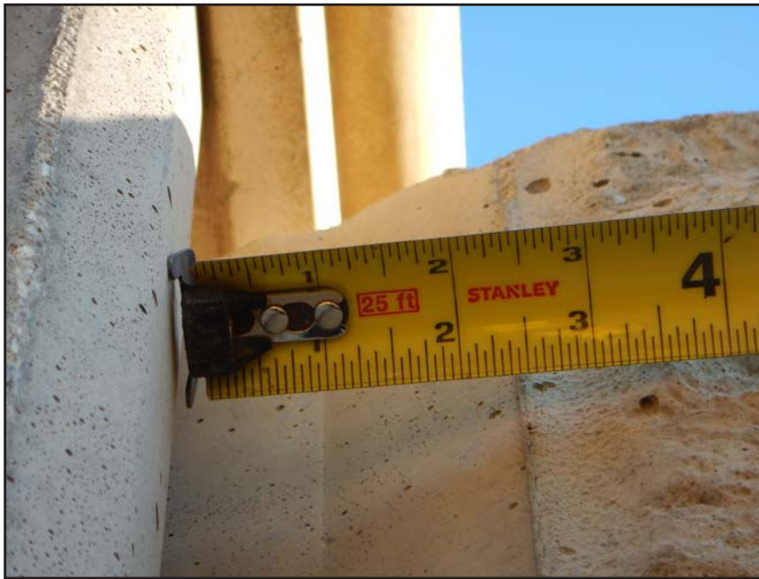
NO. 193 - COLUMN 36N - INSUFFICIENT SEATING OF A PRECAST WALL PANEL IN A PRECAST COLUMN
