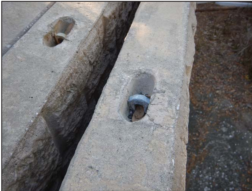
NO. 33 - STORED EXCESS WALL PANELS - TYPICAL LIFTING EYES
