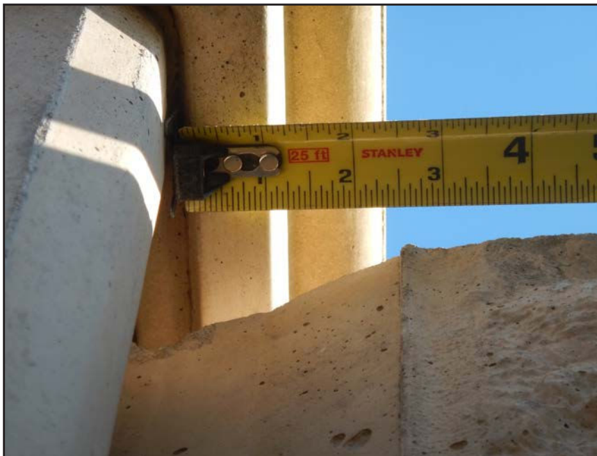
NO. 237 - COLUMN 72S - INSUFFICIENT SEATING OF A PRECAST WALL PANEL IN A PRECAST COLUMN
