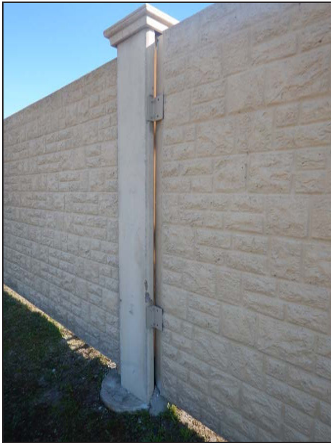
NO. 443 - COLUMN 55S - INADEQUATE ADDED CLIP ANGLE CONNECTION AT A DEFICIENT WALL PANEL TO COLUMN CONNECTION
