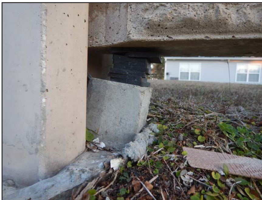
NO. 102 - COLUMN 67SS - INADEQUATE BEARING OF A PRECAST WALL PANEL ON A 2" x 2" NEOPRENE BEARING PAD
