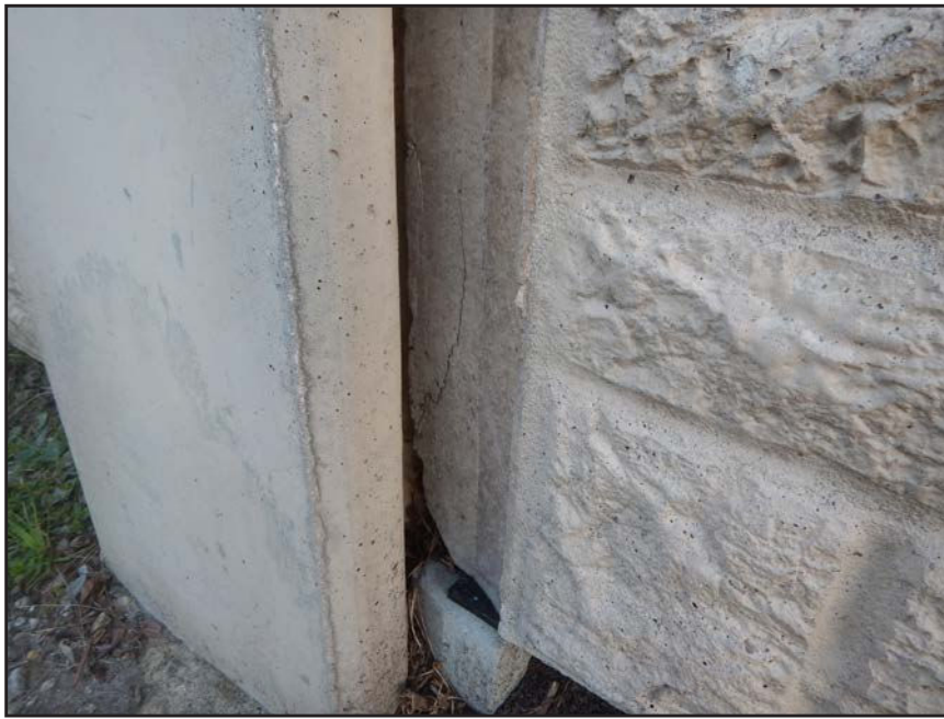
NO. 396 - COLUMN 76SS - CRACKED AND FAILED TONGUE OF A PRECAST WALL PANEL IN A PRECAST COLUMN
