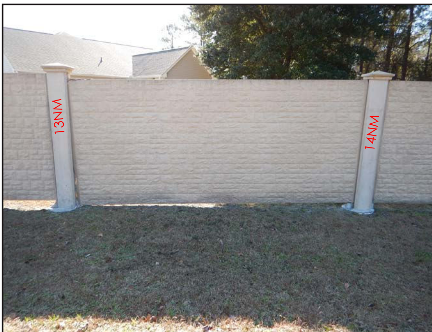
NO. 1 - DROPPED PRECAST WALL PANEL AT 3512 CLUB COURSE DRIVE, BETWEEN COLUMNS 13NM AND 14NM, AS VIEWED FROM WATER TOWER ROAD
