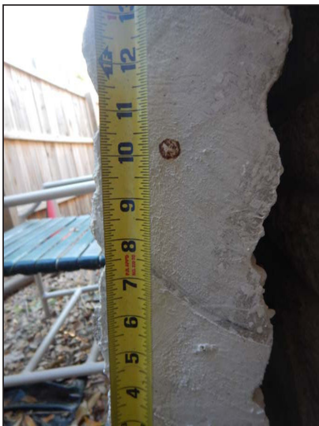
NO. 46 - SAW CUT STORED EXCESS WALL PANEL - TYPICAL HORIZONTAL REINFORCING BARS
