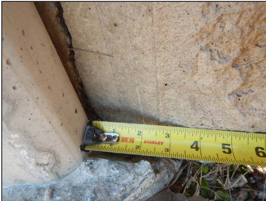
NO. 252 - COLUMN 28SS - INSUFFICIENT SEATING OF A PRECAST WALL PANEL IN A PRECAST COLUMN
