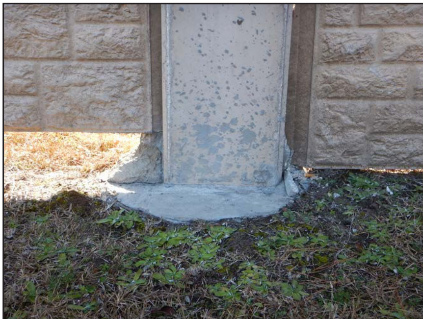
NO. 5 - COLUMN 13NM - DROPPED PRECAST SOUTH PANEL AND ELEVATED PRECAST NORTH PANEL
