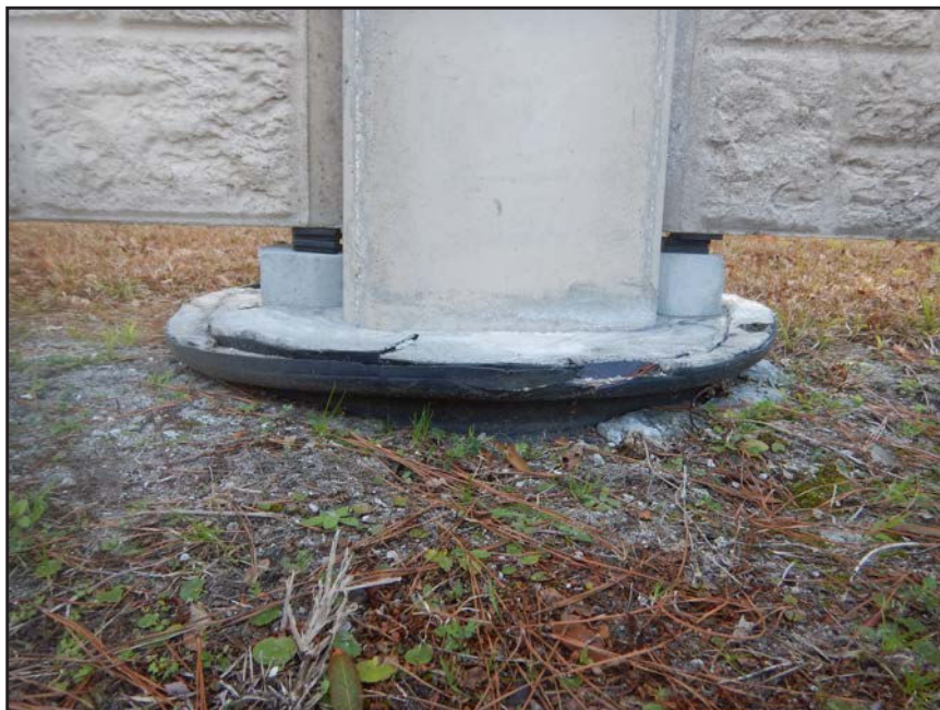
NO. 76 - COLUMN 2SM - INADEQUATE BEARING OF A PRECAST WALL PANEL ON A 2" x 2" NEOPRENE BEARING PAD
