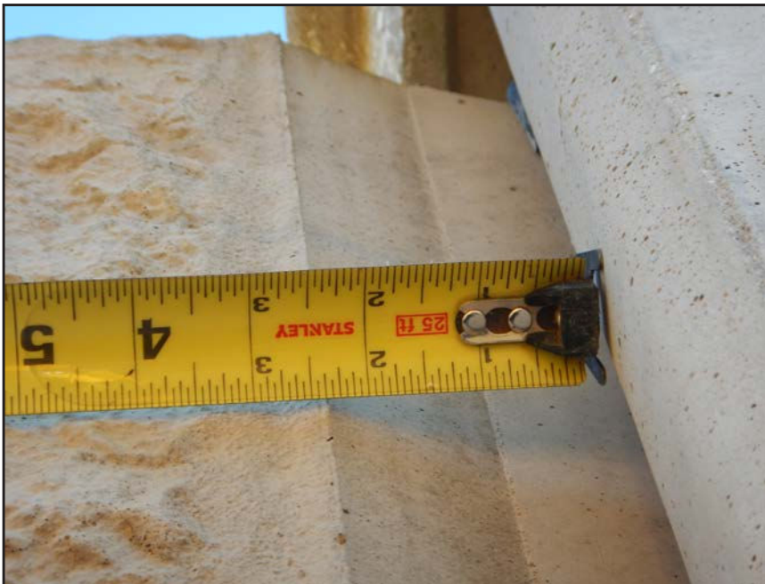
NO. 192 - COLUMN 35N - INSUFFICIENT SEATING OF A PRECAST WALL PANEL IN A PRECAST COLUMN
