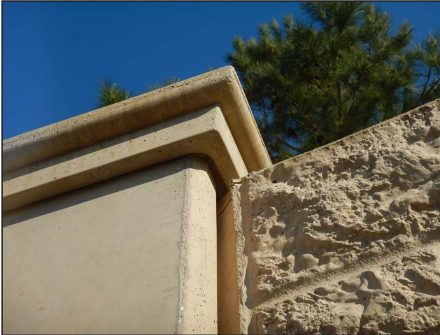
NO. 478 - COLUMN 3SS - CRACKED AND SPALLED PRECAST CONCRETE
