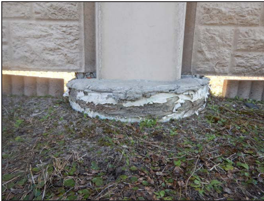
NO. 142 - COLUMN 73S - INADEQUATE BEARING OF A PRECAST WALL PANEL ON A FAILED GROUT PEDESTAL OR A FAILED PRECAST TONGUE
