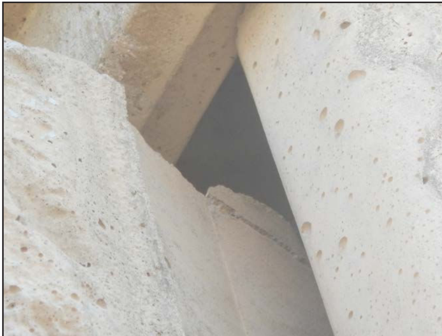
NO. 349 - COLUMN 16SS - CRACKED AND FAILED TONGUE OF A PRECAST WALL PANEL IN A PRECAST COLUMN
