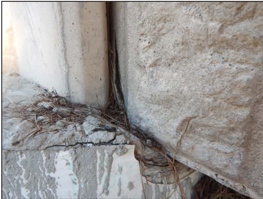
NO. 164 - COLUMN 24SS - INADEQUATE BEARING OF A PRECAST WALL PANEL ON A FAILED GROUT PEDESTAL OR A FAILED PRECAST TONGUE
