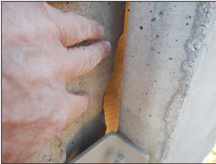
NO. 300 - COLUMN 50N - CRACKED AND FAILED TONGUE OF A PRECAST WALL PANEL IN A PRECAST COLUMN
