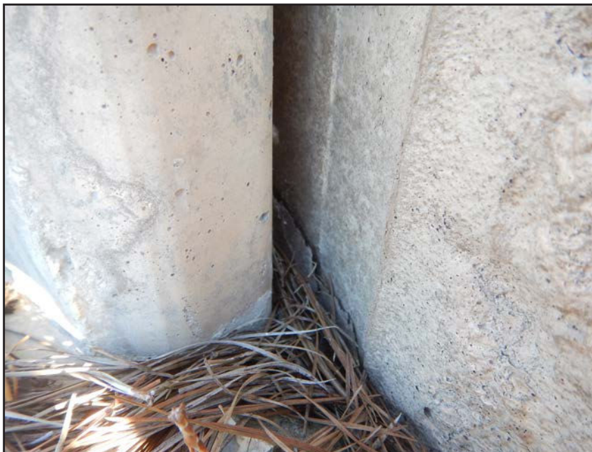
NO. 165 - COLUMN 26SS - INADEQUATE BEARING OF A PRECAST WALL PANEL ON A FAILED GROUT PEDESTAL OR A FAILED PRECAST TONGUE
