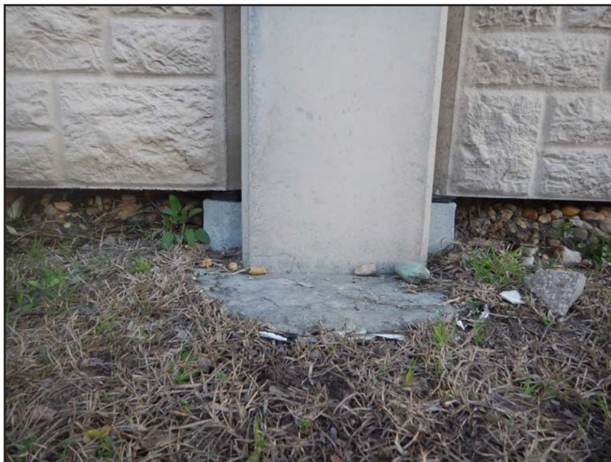
NO. 103 - COLUMN 78SS - INADEQUATE BEARING OF A PRECAST WALL PANEL ON A 2" x 2" NEOPRENE BEARING PAD
