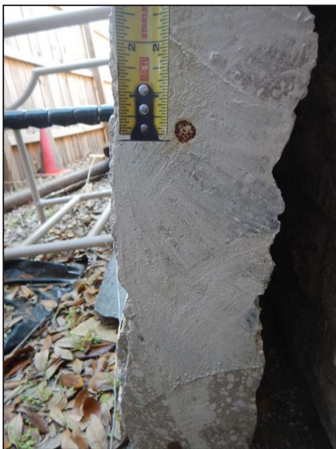
NO. 45 - SAW CUT STORED EXCESS WALL PANEL - TYPICAL HORIZONTAL REINFORCING BARS
