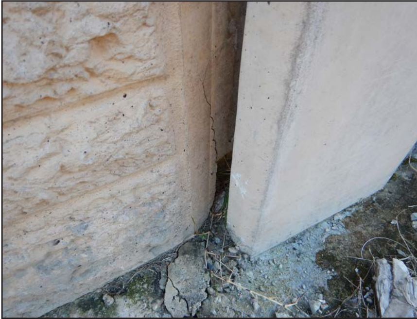
NO. 289 - COLUMN 28N - CRACKED AND FAILED TONGUE OF A PRECAST WALL PANEL IN A PRECAST COLUMN
