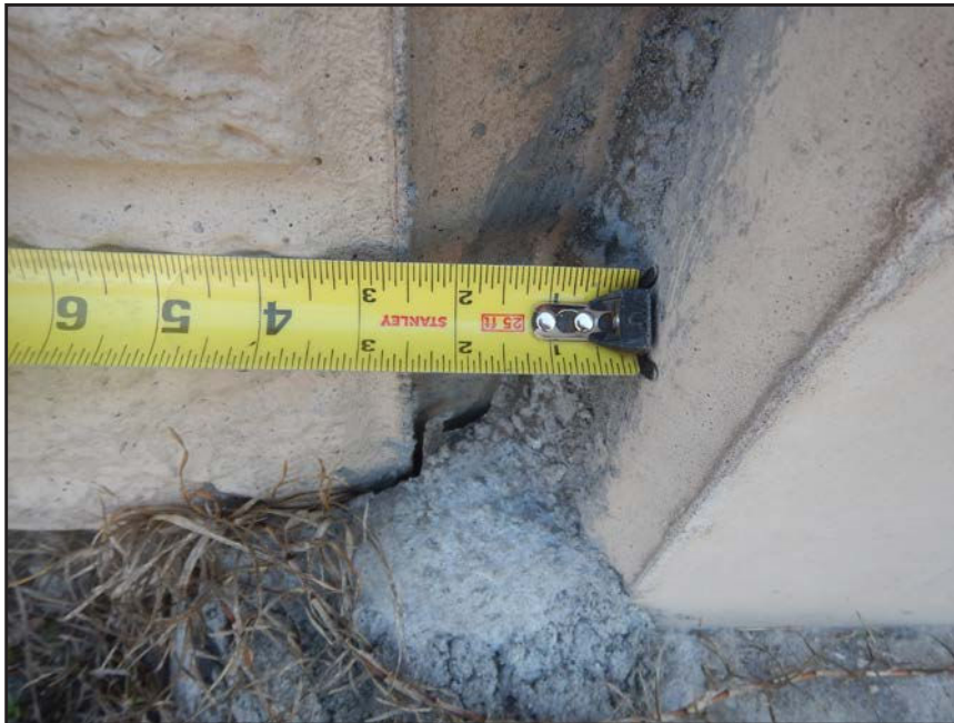
NO. 236 - COLUMN 70S - INSUFFICIENT SEATING OF A PRECAST WALL PANEL IN A PRECAST COLUMN
