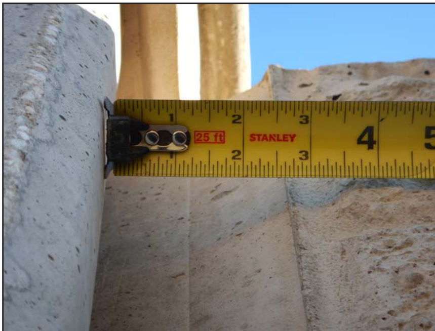
NO. 185 - COLUMN 12N - INSUFFICIENT SEATING OF A PRECAST WALL PANEL IN A PRECAST COLUMN
