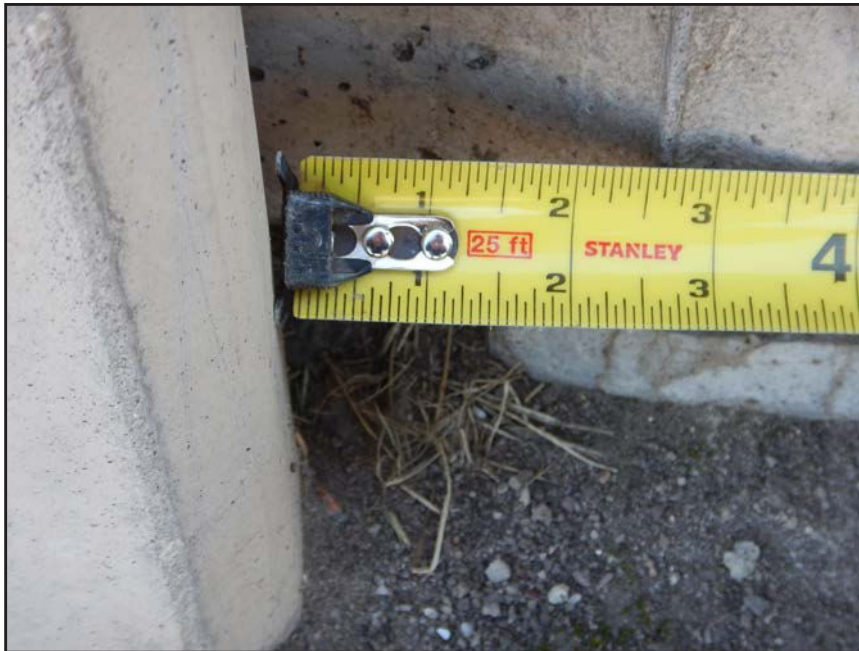
NO. 189 - COLUMN 20N - INSUFFICIENT SEATING OF A PRECAST WALL PANEL IN A PRECAST COLUMN
