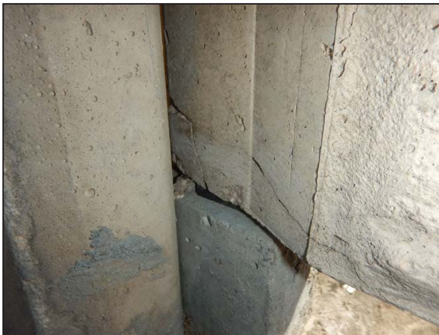
NO. 124 - COLUMN 4S - INADEQUATE BEARING OF A PRECAST WALL PANEL ON A FAILED GROUT PEDESTAL OR A FAILED PRECAST TONGUE
