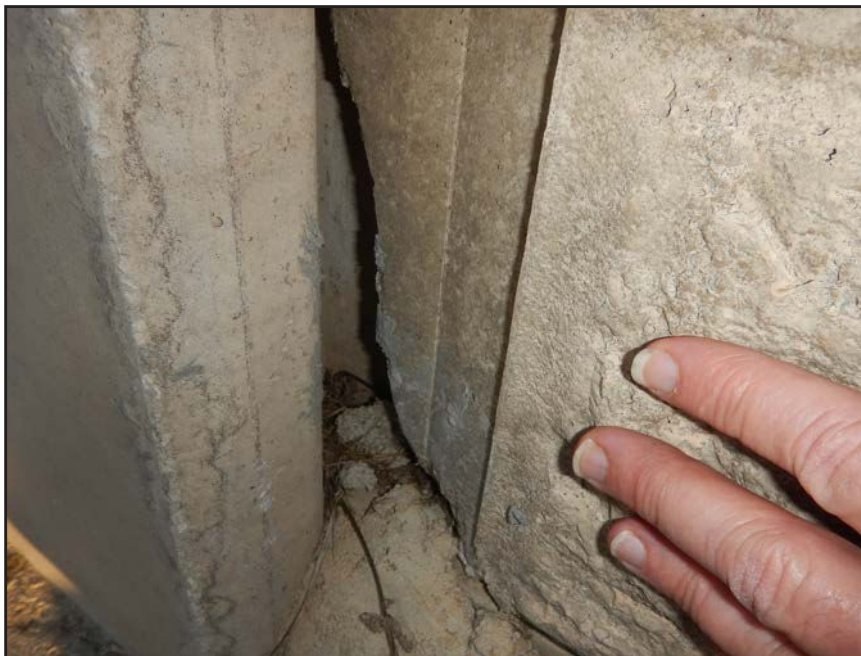
NO. 372 - COLUMN 46SS - CRACKED AND FAILED TONGUE OF A PRECAST WALL PANEL IN A PRECAST COLUMN
