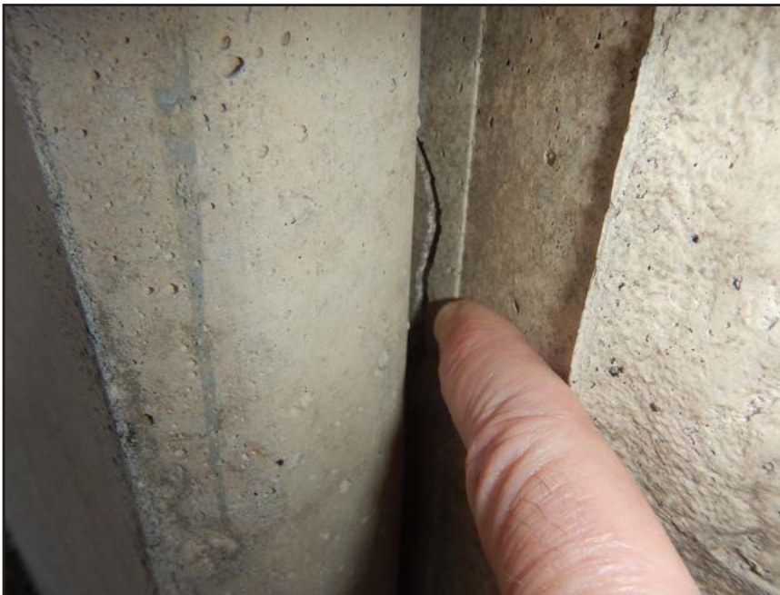
NO. 320 - COLUMN 15S - CRACKED AND FAILED TONGUE OF A PRECAST WALL PANEL IN A PRECAST COLUMN
