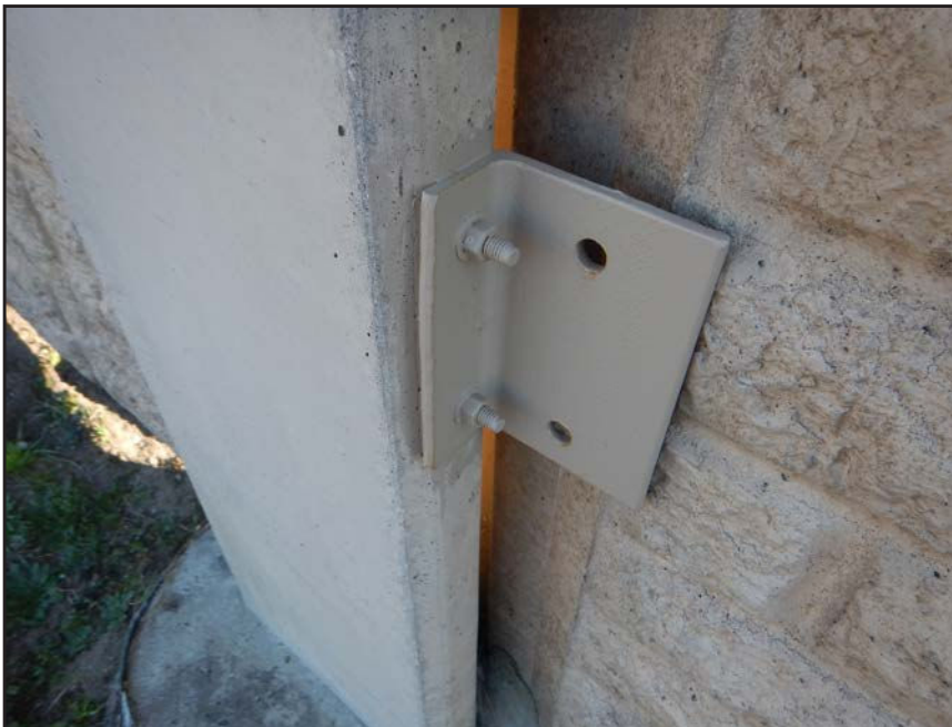
NO. 419 - COLUMN 10N - INADEQUATE ADDED CLIP ANGLE CONNECTION AT A DEFICIENT WALL PANEL TO COLUMN CONNECTION
