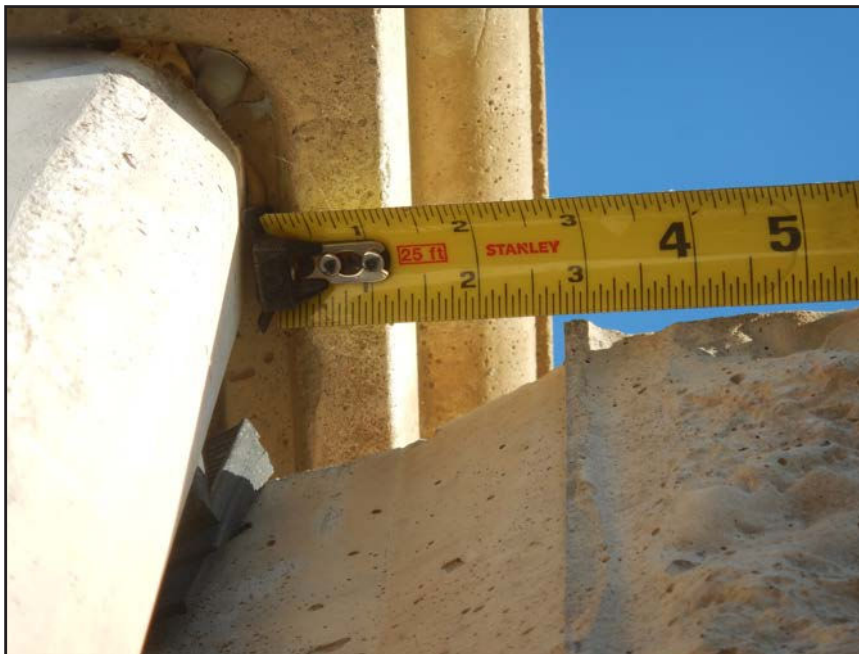
NO. 248 - COLUMN 18SS - INSUFFICIENT SEATING OF A PRECAST WALL PANEL IN A PRECAST COLUMN
