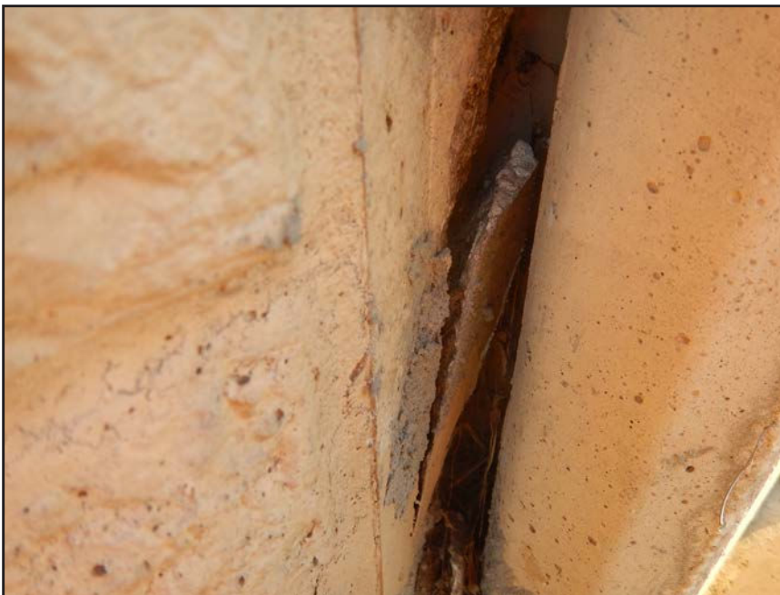
NO. 375 - COLUMN 47SS - CRACKED AND FAILED TONGUE OF A PRECAST WALL PANEL IN A PRECAST COLUMN
