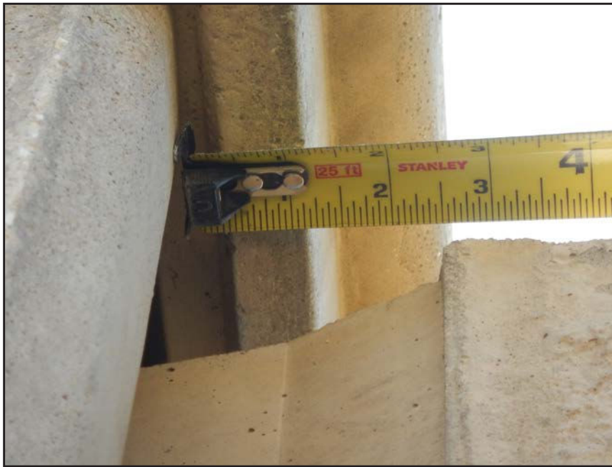
NO. 207 - COLUMN 6SM - INSUFFICIENT SEATING OF A PRECAST WALL PANEL IN A PRECAST COLUMN
