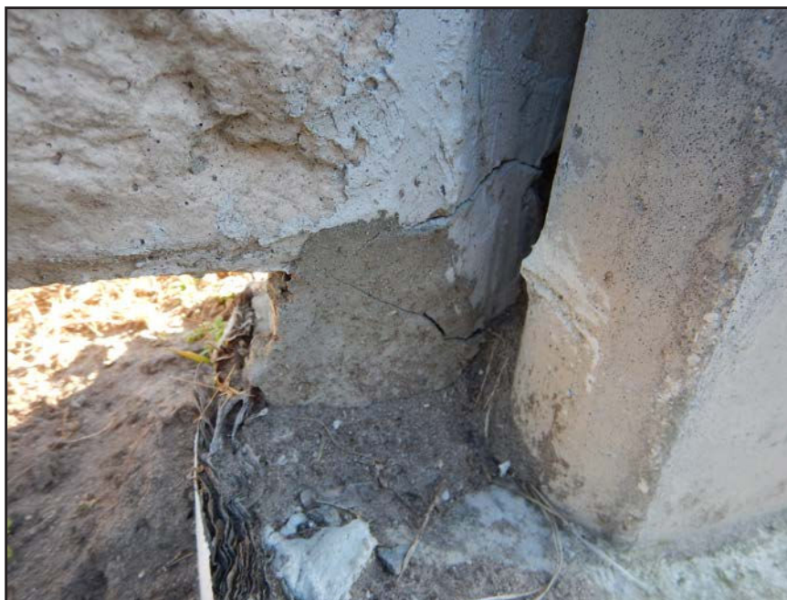
NO. 108 - COLUMN 25N - INADEQUATE BEARING OF A PRECAST WALL PANEL ON A FAILED GROUT PEDESTAL OR A FAILED PRECAST TONGUE
