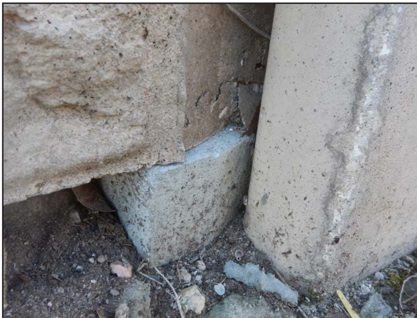
NO. 117 - COLUMN 5NM - INADEQUATE BEARING OF A PRECAST WALL PANEL ON A FAILED GROUT PEDESTAL OR A FAILED PRECAST TONGUE
