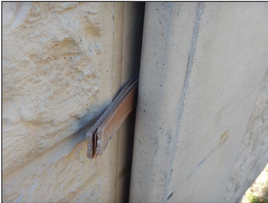
NO. 268 - COLUMN 17SM - INADEQUATE SHIMS STABILIZING A WALL PANEL TO COLUMN CONNECTION AT EXCESSIVE PLAY BETWEEN ADJACENT MEMBERS
