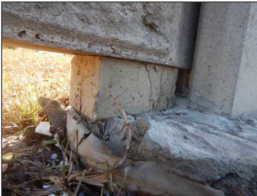
NO. 141 - COLUMN 69S - INADEQUATE BEARING OF A PRECAST WALL PANEL ON A FAILED GROUT PEDESTAL OR A FAILED PRECAST TONGUE
