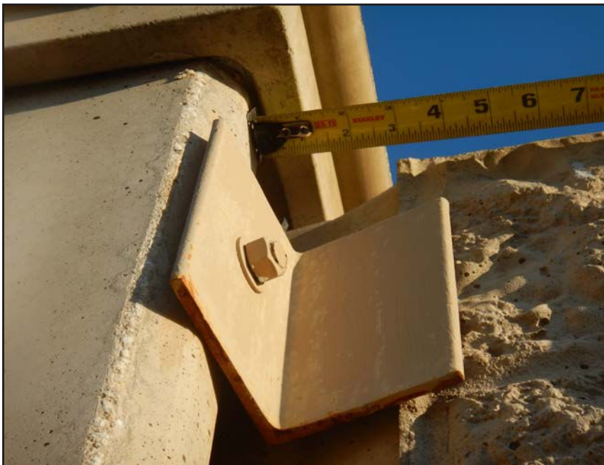
NO. 448 - COLUMN 40SS - INADEQUATE ADDED CLIP ANGLE CONNECTION AT A DEFICIENT WALL PANEL TO COLUMN CONNECTION
