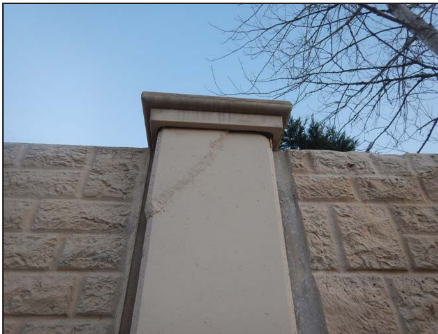
NO. 493 - COLUMN 79SS - CRACKED AND SPALLED PRECAST CONCRETE
