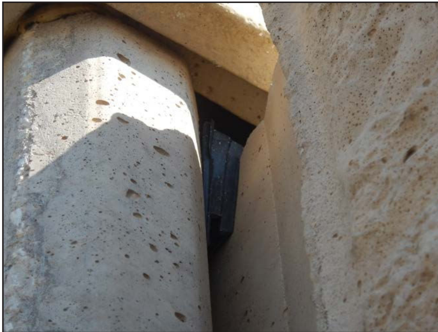
NO. 282 - COLUMN 45S - INADEQUATE SHIMS STABILIZING A WALL PANEL TO COLUMN CONNECTION AT EXCESSIVE PLAY BETWEEN ADJACENT MEMBERS
