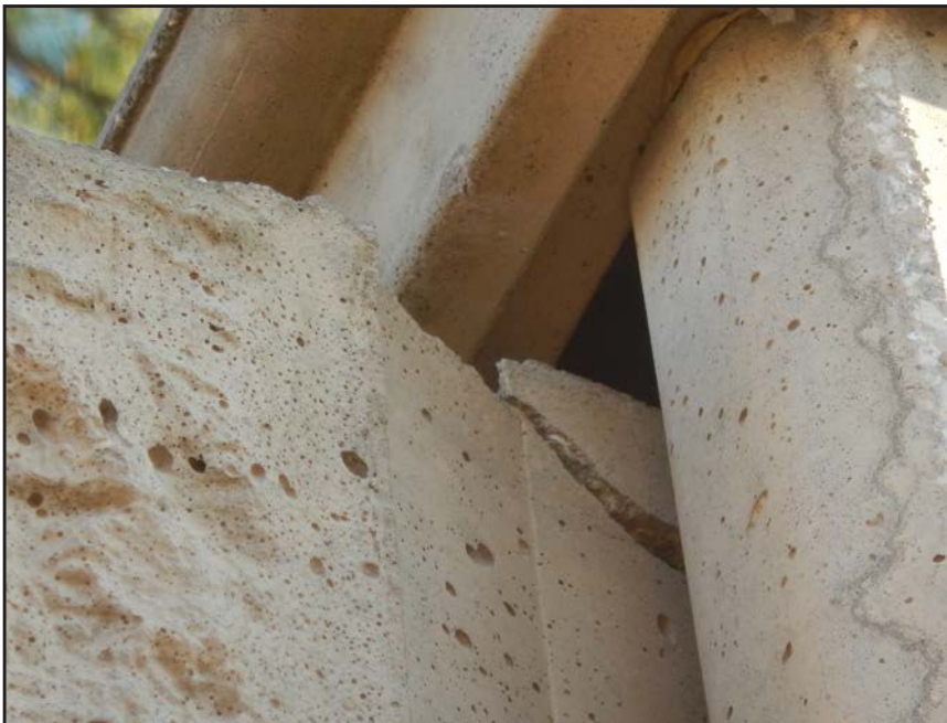
NO. 364 - COLUMN 37SS - CRACKED AND FAILED TONGUE OF A PRECAST WALL PANEL IN A PRECAST COLUMN
