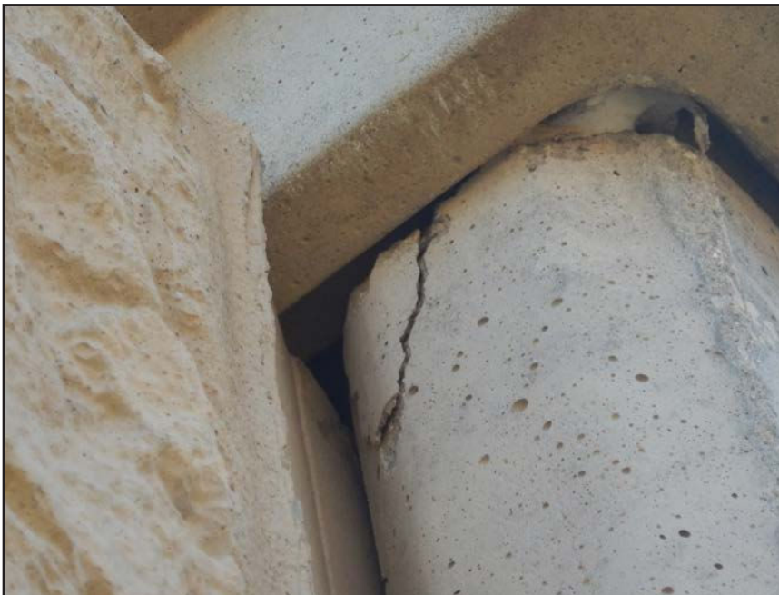
NO. 474 - COLUMN 77S - CRACKED AND SPALLED PRECAST CONCRETE
