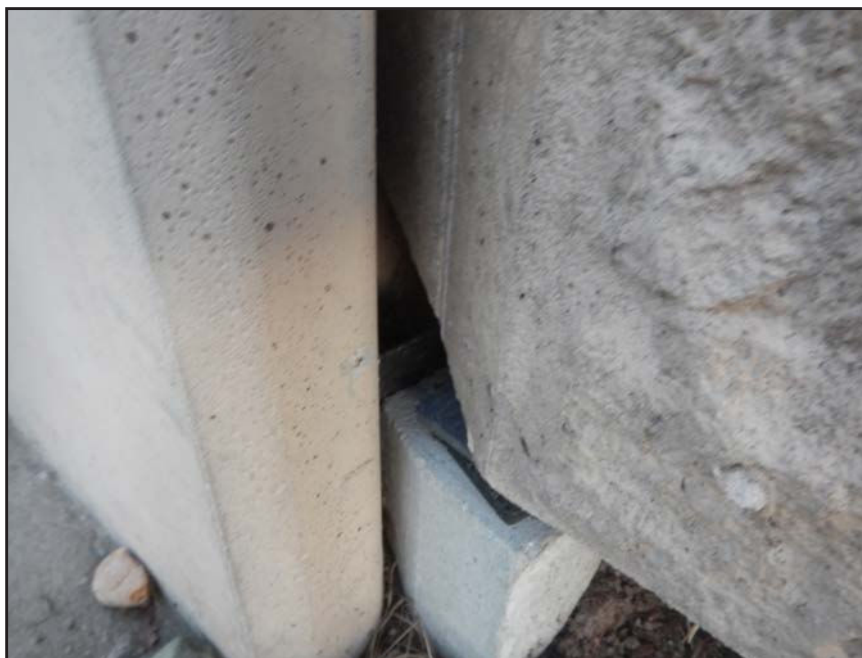
NO. 105 - COLUMN 78SS - INADEQUATE BEARING OF A PRECAST WALL PANEL ON A 2" x 2" NEOPRENE BEARING PAD
