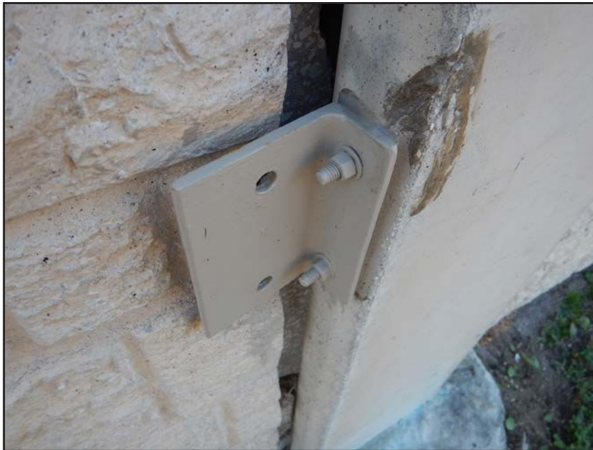
NO. 423 - COLUMN 14N - INADEQUATE ADDED CLIP ANGLE CONNECTION AT A DEFICIENT WALL PANEL TO COLUMN CONNECTION
