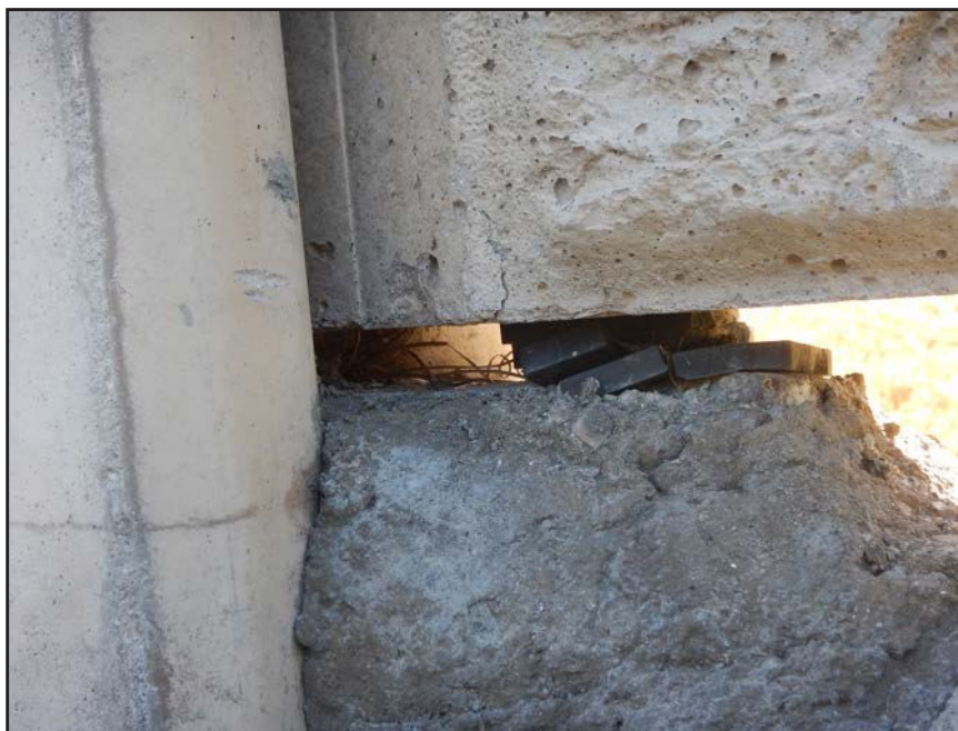
NO. 73 - COLUMN 10NM - INADEQUATE BEARING OF A PRECAST WALL PANEL ON A 2" x 2" NEOPRENE BEARING PAD
