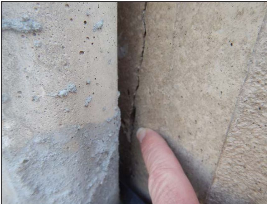
NO. 318 - COLUMN 13S - CRACKED AND FAILED TONGUE OF A PRECAST WALL PANEL IN A PRECAST COLUMN
