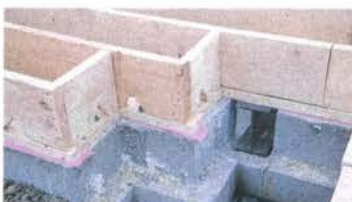
SILL PLATE INSTALLATION
