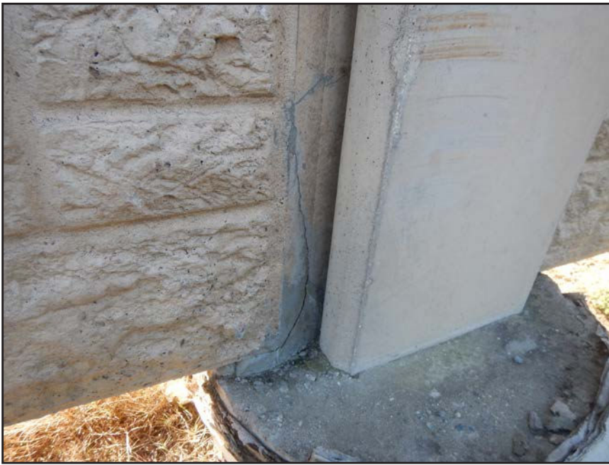
NO. 296 - COLUMN 49N - CRACKED AND FAILED TONGUE OF A PRECAST WALL PANEL IN A PRECAST COLUMN
