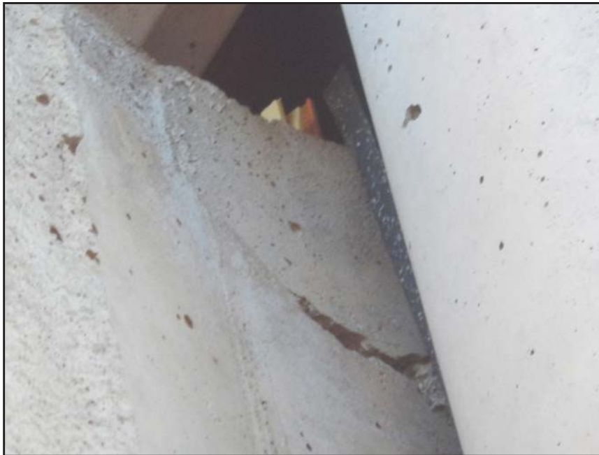
NO. 379 - COLUMN 59SS - CRACKED AND FAILED TONGUE OF A PRECAST WALL PANEL IN A PRECAST COLUMN
