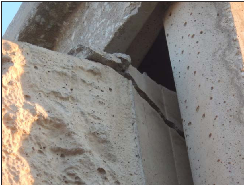
NO. 387 - COLUMN 62SS - CRACKED AND FAILED TONGUE OF A PRECAST WALL PANEL IN A PRECAST COLUMN
