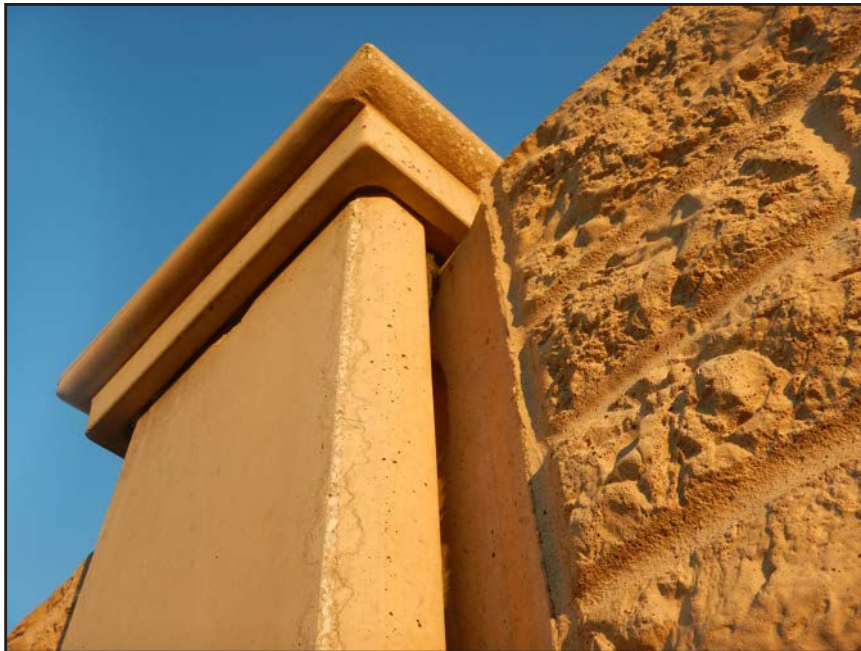
NO. 382 - COLUMN 59SS - CRACKED AND FAILED TONGUE OF A PRECAST WALL PANEL IN A PRECAST COLUMN
