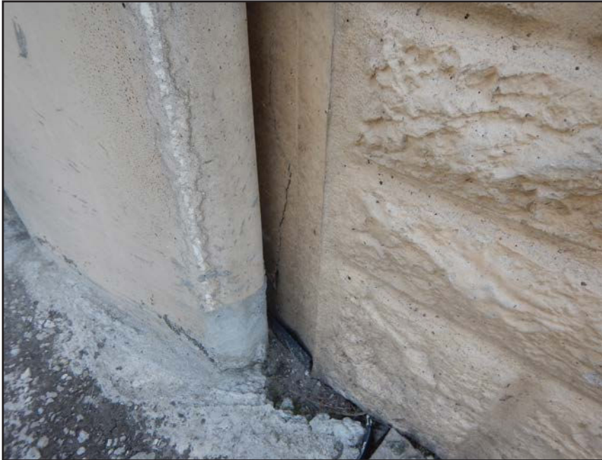
NO. 317 - COLUMN 13S - CRACKED AND FAILED TONGUE OF A PRECAST WALL PANEL IN A PRECAST COLUMN
