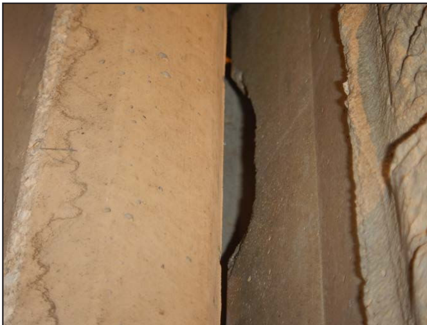
NO. 383 - COLUMN 59SS - CRACKED AND FAILED TONGUE OF A PRECAST WALL PANEL IN A PRECAST COLUMN
