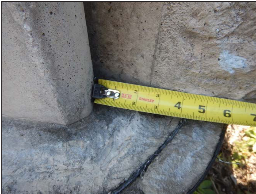
NO. 208 - COLUMN 6SM - INSUFFICIENT SEATING OF A PRECAST WALL PANEL IN A PRECAST COLUMN
