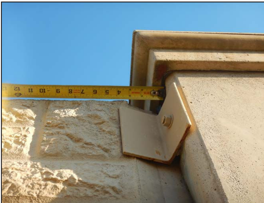
NO. 450 - COLUMN 41SS - INADEQUATE ADDED CLIP ANGLE CONNECTION AT A DEFICIENT WALL PANEL TO COLUMN CONNECTION
