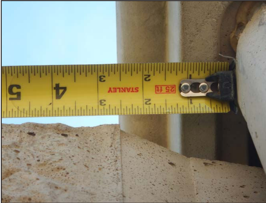
NO. 225 - COLUMN 41S - INSUFFICIENT SEATING OF A PRECAST WALL PANEL IN A PRECAST COLUMN
