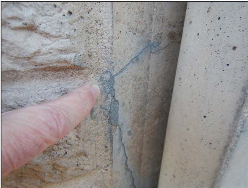
NO. 297 - COLUMN 49N - CRACKED AND FAILED TONGUE OF A PRECAST WALL PANEL IN A PRECAST COLUMN
