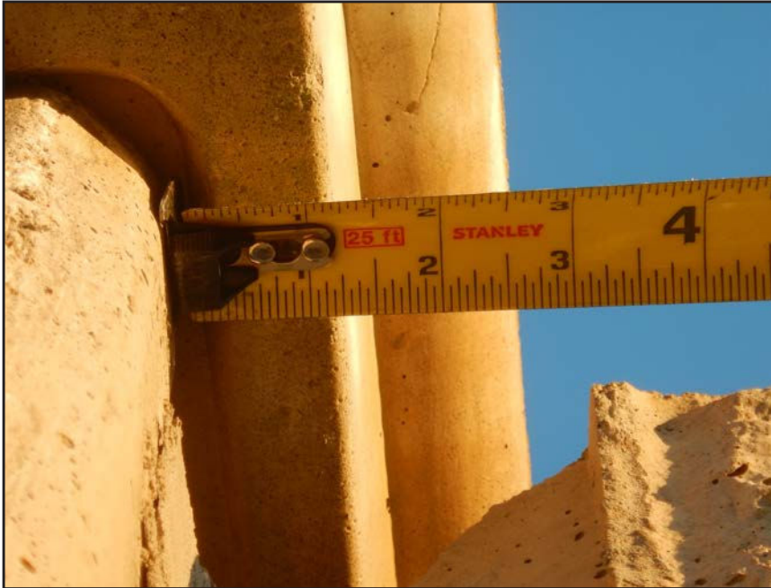
NO. 258 - COLUMN 55SS - INSUFFICIENT SEATING OF A PRECAST WALL PANEL IN A PRECAST COLUMN
