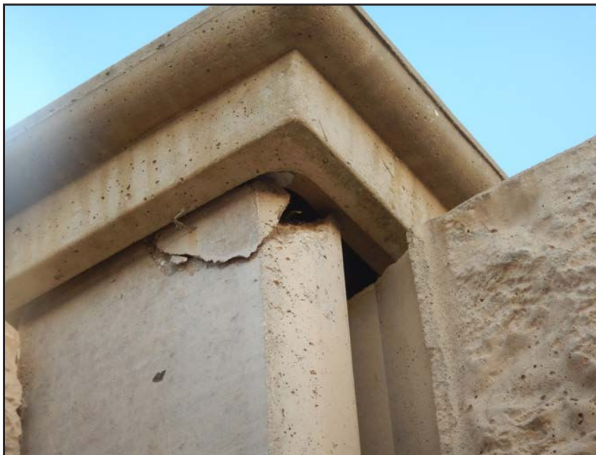
NO. 490 - COLUMN 68SS (BACK) - CRACKED AND SPALLED PRECAST CONCRETE
