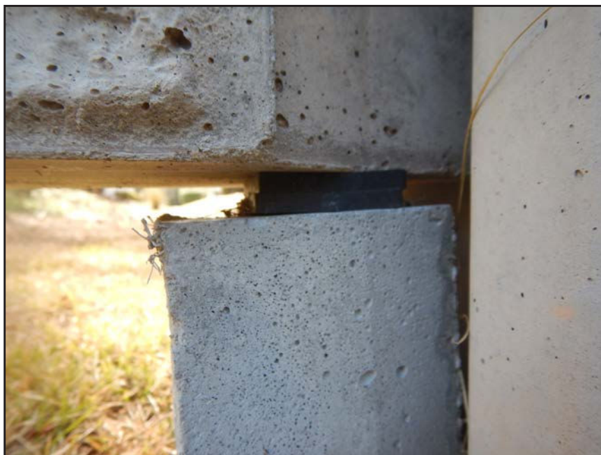
NO. 83 - COLUMN 15SM - INADEQUATE BEARING OF A PRECAST WALL PANEL ON A 2" x 2" NEOPRENE BEARING PAD
