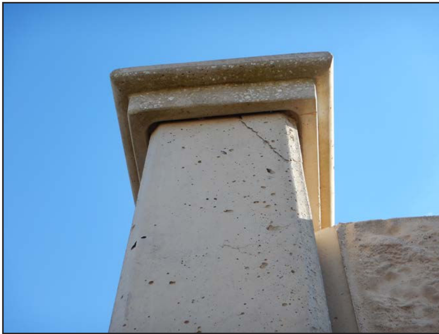
NO. 459 - COLUMN 1N - CRACKED AND SPALLED PRECAST CONCRETE
