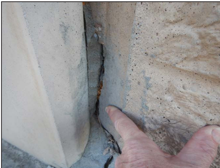
NO. 331 - COLUMN 61S - CRACKED AND FAILED TONGUE OF A PRECAST WALL PANEL IN A PRECAST COLUMN
