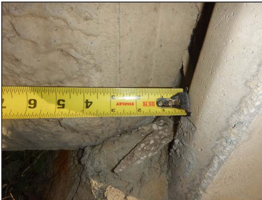
NO. 245 - COLUMN 6SS - INSUFFICIENT SEATING OF A PRECAST WALL PANEL IN A PRECAST COLUMN
