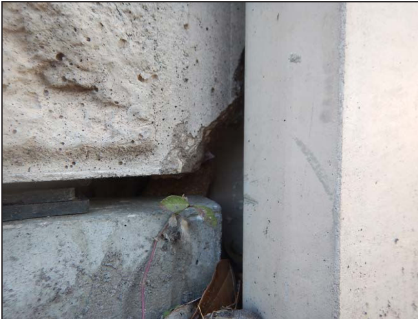
NO. 385 - COLUMN 60SS - CRACKED AND FAILED TONGUE OF A PRECAST WALL PANEL IN A PRECAST COLUMN
