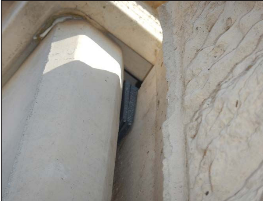
NO. 279 - COLUMN 41S - INADEQUATE SHIMS STABILIZING A WALL PANEL TO COLUMN CONNECTION AT EXCESSIVE PLAY BETWEEN ADJACENT MEMBERS
