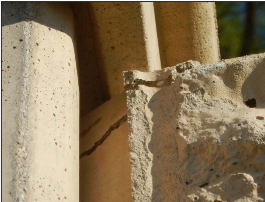
NO. 479 - COLUMN 3SS - CRACKED AND SPALLED PRECAST CONCRETE
