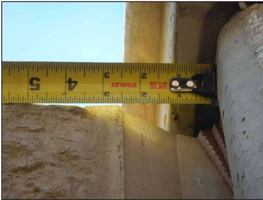
NO. 210 - COLUMN 11SM - INSUFFICIENT SEATING OF A PRECAST WALL PANEL IN A PRECAST COLUMN
