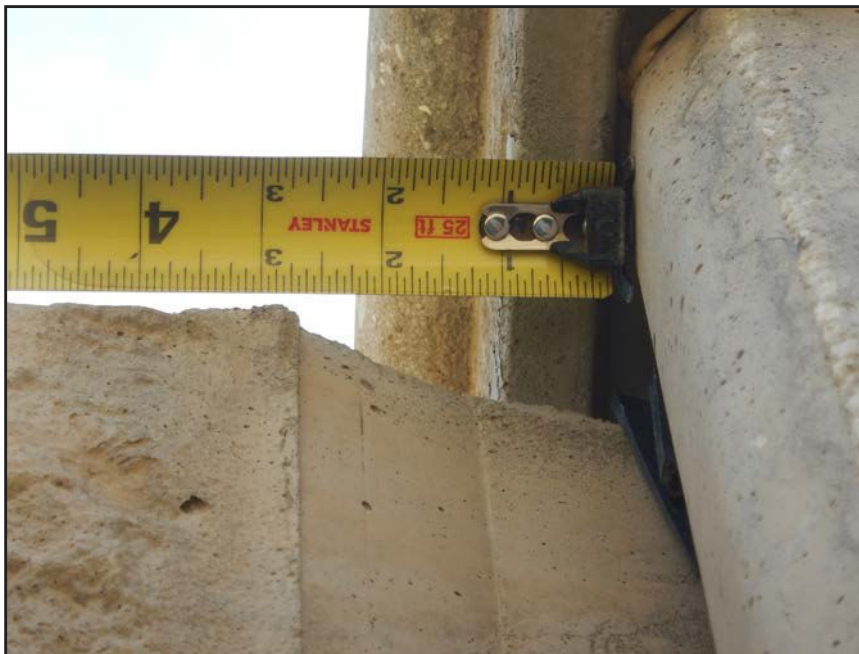
NO. 215 - COLUMN 10S - INSUFFICIENT SEATING OF A PRECAST WALL PANEL IN A PRECAST COLUMN
