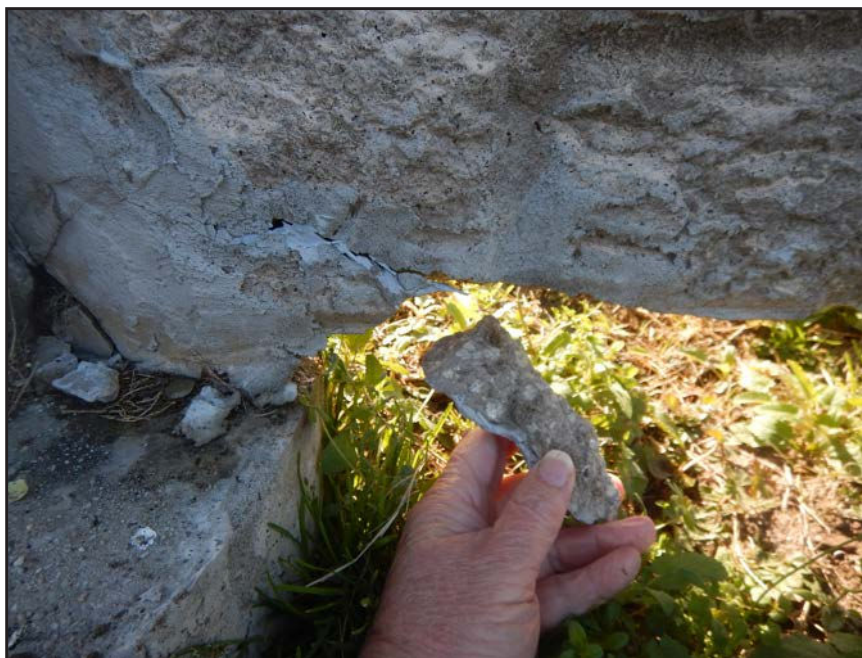
NO. 111 - COLUMN 43N - INADEQUATE BEARING OF A PRECAST WALL PANEL ON A FAILED GROUT PEDESTAL OR A FAILED PRECAST TONGUE
