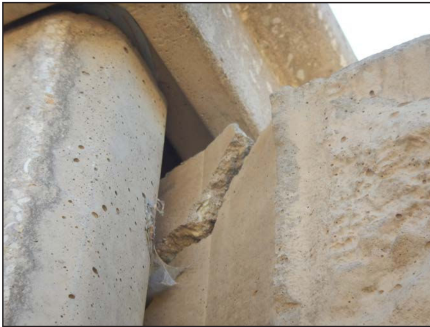
NO. 308 - COLUMN 5NM - CRACKED AND FAILED TONGUE OF A PRECAST WALL PANEL IN A PRECAST COLUMN
