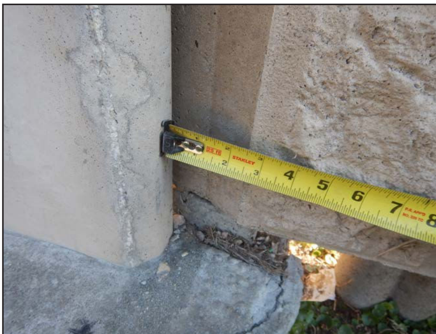
NO. 242 - COLUMN 79S - INSUFFICIENT SEATING OF A PRECAST WALL PANEL IN A PRECAST COLUMN
