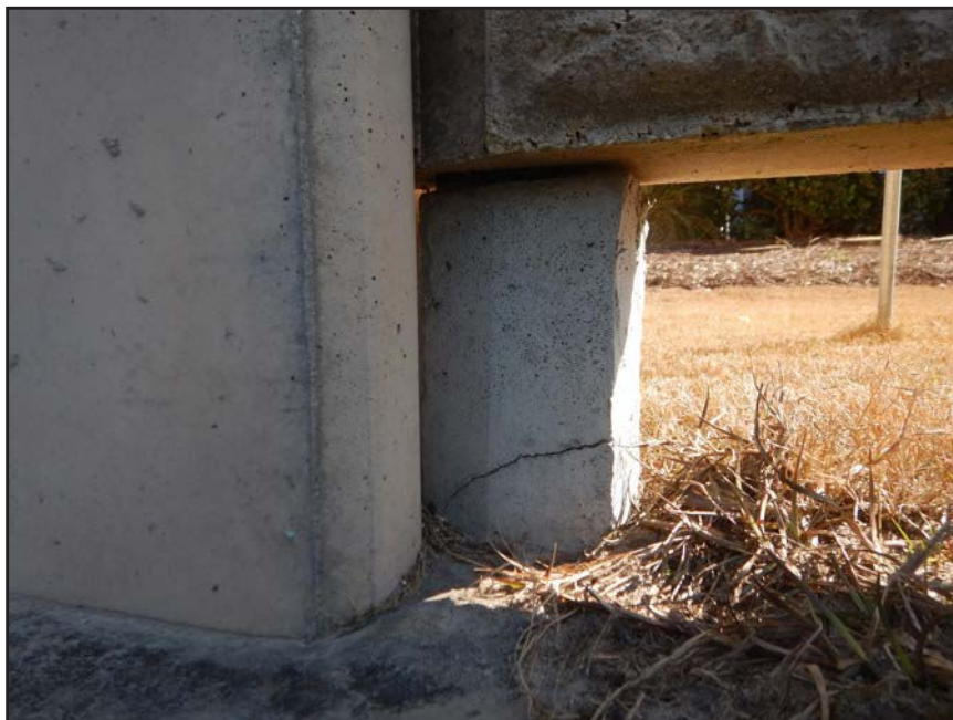
NO. 128 - COLUMN 28S - INADEQUATE BEARING OF A PRECAST WALL PANEL ON A FAILED GROUT PEDESTAL OR A FAILED PRECAST TONGUE
