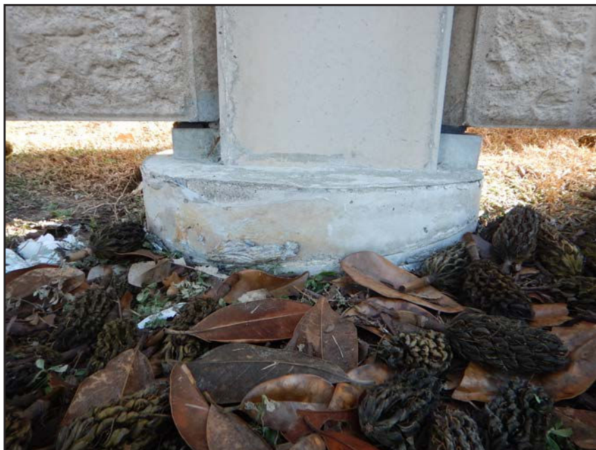
NO. 63 - COLUMN 2N - INADEQUATE BEARING OF A PRECAST WALL PANEL ON A 2" x 2" NEOPRENE BEARING PAD
