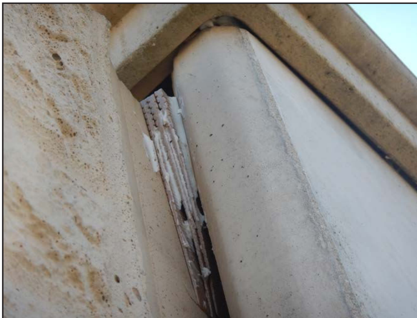
NO. 283 - COLUMN 53S - INADEQUATE SHIMS STABILIZING A WALL PANEL TO COLUMN CONNECTION AT EXCESSIVE PLAY BETWEEN ADJACENT MEMBERS
