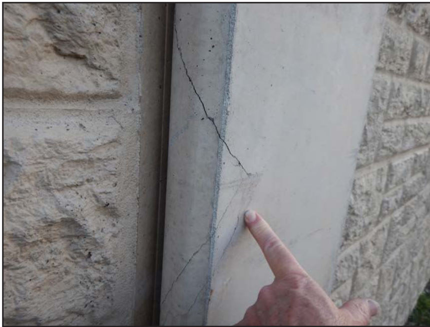
NO. 491 - COLUMN 70SS - CRACKED AND SPALLED PRECAST CONCRETE
