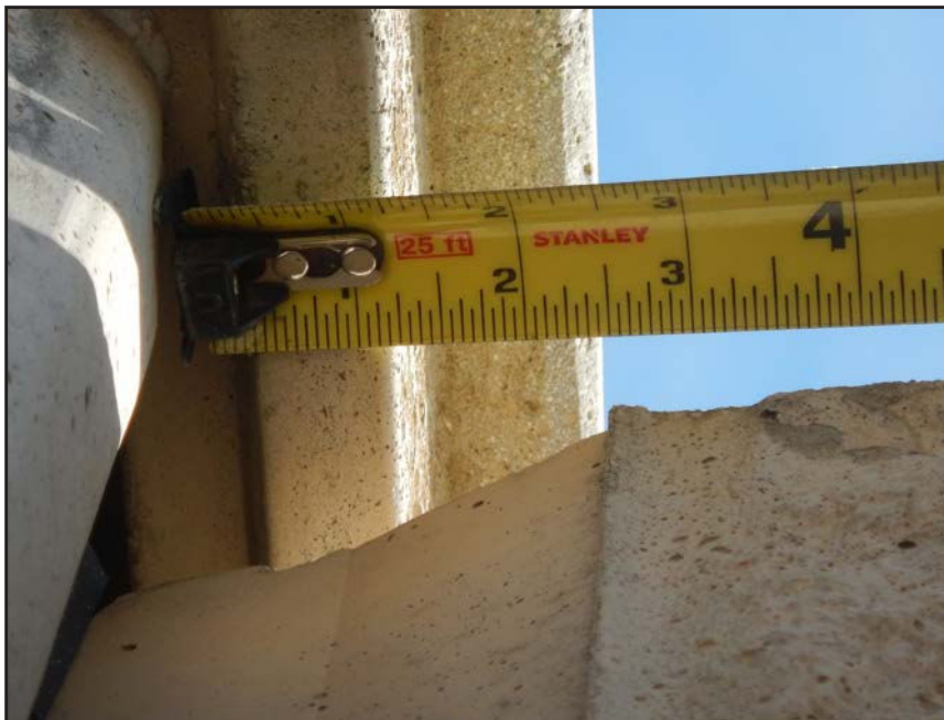
NO. 224 - COLUMN 37S - INSUFFICIENT SEATING OF A PRECAST WALL PANEL IN A PRECAST COLUMN
