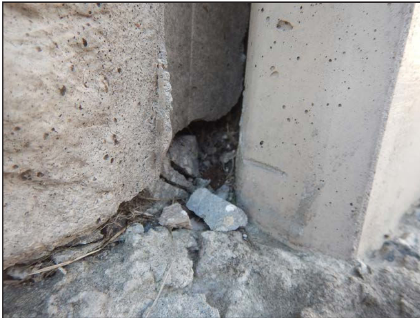
NO. 177 - COLUMN 64SS - INADEQUATE BEARING OF A PRECAST WALL PANEL ON A FAILED GROUT PEDESTAL OR A FAILED PRECAST TONGUE
