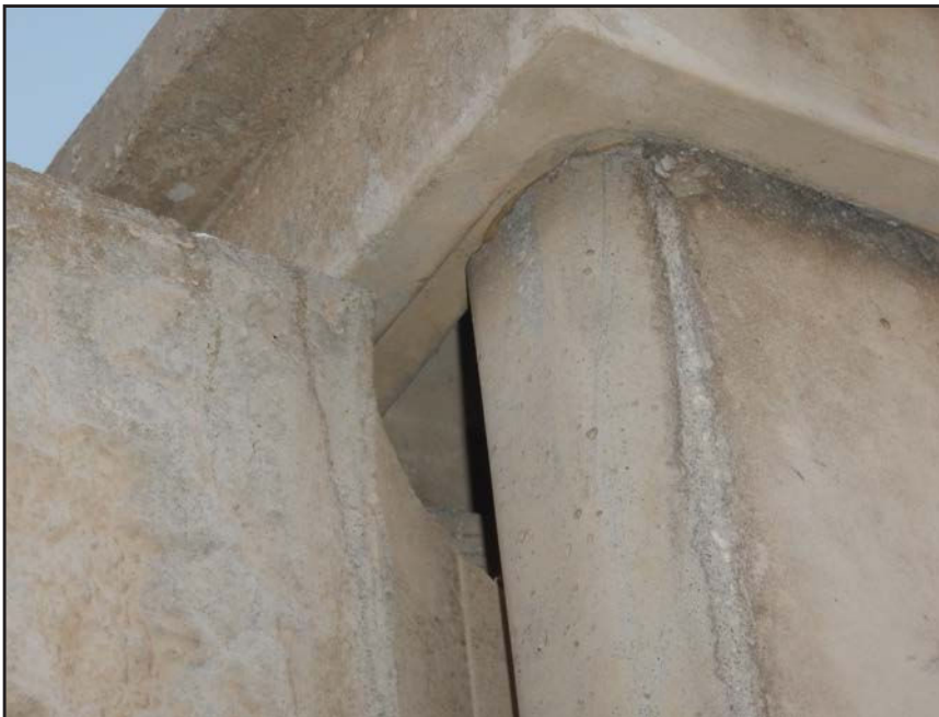
NO. 400 - COLUMN 78SS - CRACKED AND FAILED TONGUE OF A PRECAST WALL PANEL IN A PRECAST COLUMN
