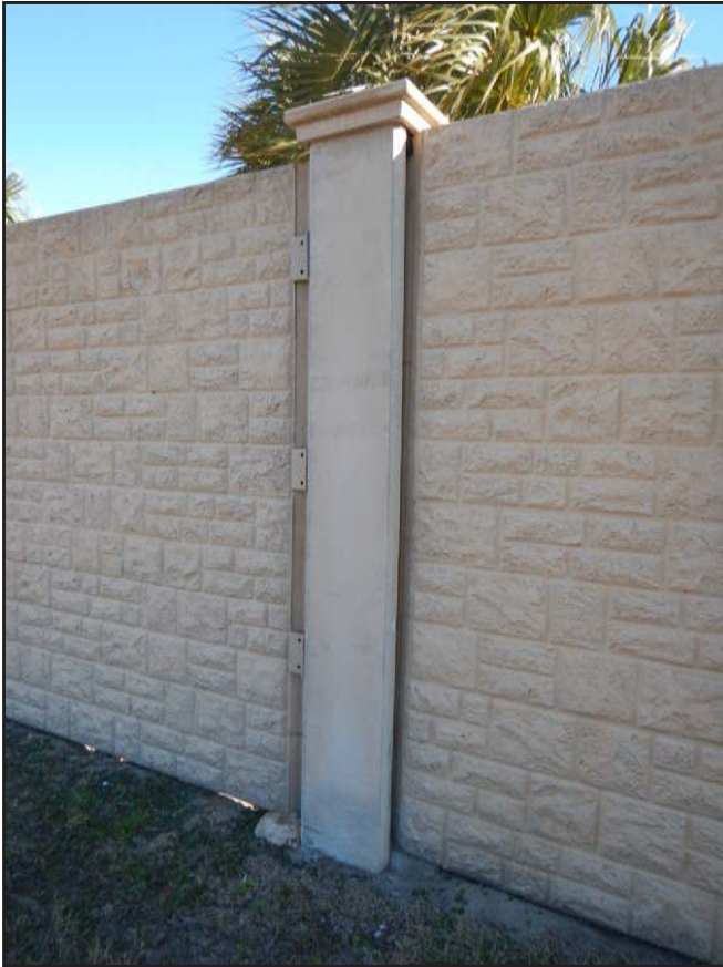
NO. 425 - COLUMN 19N - INADEQUATE ADDED CLIP ANGLE CONNECTION AT A DEFICIENT WALL PANEL TO COLUMN CONNECTION
