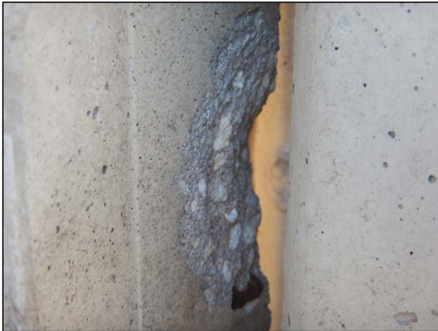
NO. 306 - COLUMN 56N - CRACKED AND FAILED TONGUE OF A PRECAST WALL PANEL IN A PRECAST COLUMN
