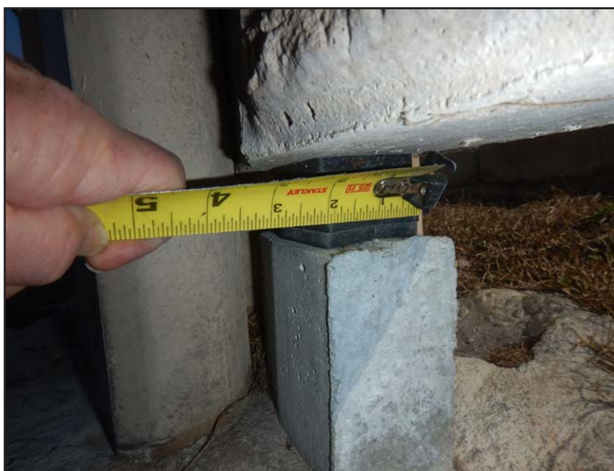
NO. 93 - COLUMN 33S - INADEQUATE BEARING OF A PRECAST WALL PANEL ON A 2" x 2" NEOPRENE BEARING PAD
