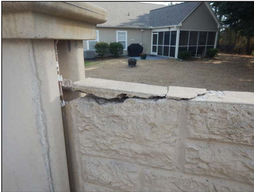
NO. 52 - SPALLED WALL PANEL ON THE SOUTH SIDE OF COLUMN 13NM
