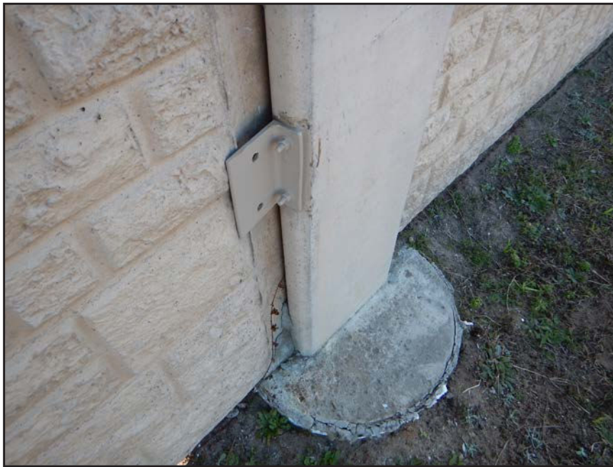
NO. 414 - COLUMN 9N - INADEQUATE ADDED CLIP ANGLE CONNECTION AT A DEFICIENT WALL PANEL TO COLUMN CONNECTION
