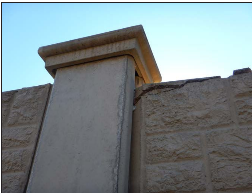
NO. 3 - COLUMN 13NM - DROPPED PRECAST PANEL WITH A CRACKED AND SPALLED TOP
