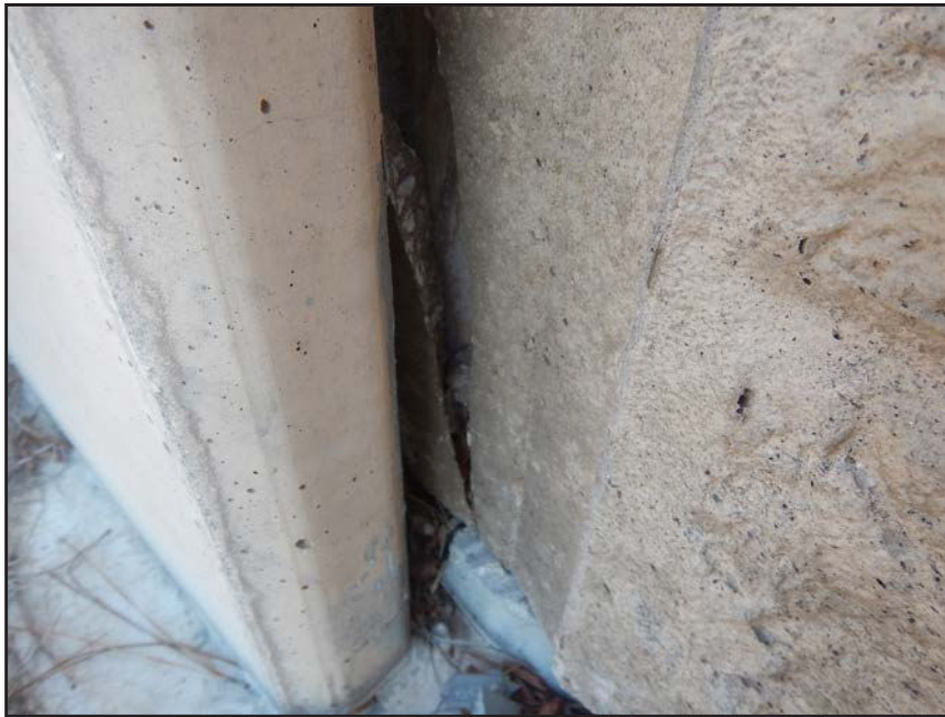
NO. 354 - COLUMN 22SS - CRACKED AND FAILED TONGUE OF A PRECAST WALL PANEL IN A PRECAST COLUMN
