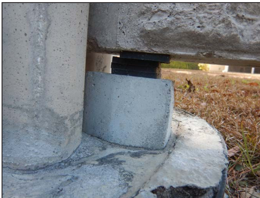
NO. 78 - COLUMN 2SM - INADEQUATE BEARING OF A PRECAST WALL PANEL ON A 2" x 2" NEOPRENE BEARING PAD
