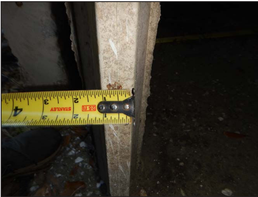
NO. 26 - STORED EXCESS WALL PANELS - TYPICAL TONGUE DIMENSIONS
