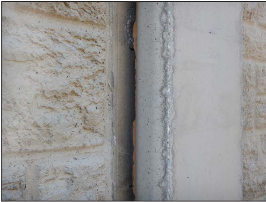
NO. 305 - COLUMN 56N - CRACKED AND FAILED TONGUE OF A PRECAST WALL PANEL IN A PRECAST COLUMN
