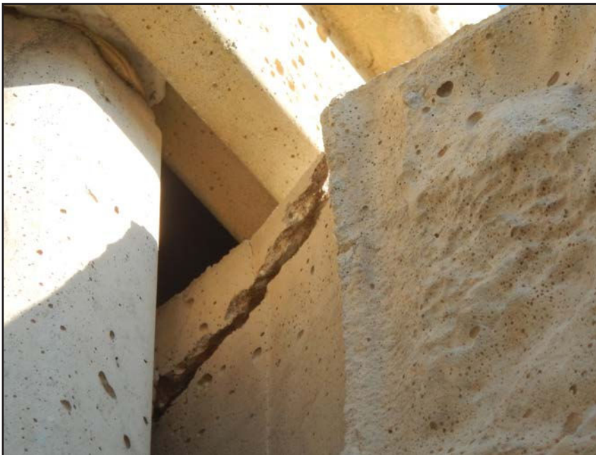
NO. 341 - COLUMN 77S - CRACKED AND FAILED TONGUE OF A PRECAST WALL PANEL IN A PRECAST COLUMN
