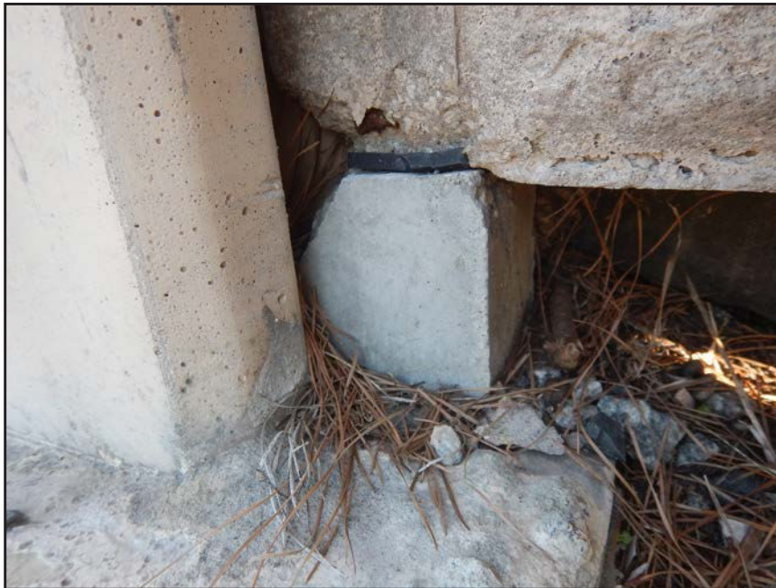
NO. 169 - COLUMN 32SS - INADEQUATE BEARING OF A PRECAST WALL PANEL ON A FAILED GROUT PEDESTAL OR A FAILED PRECAST TONGUE
