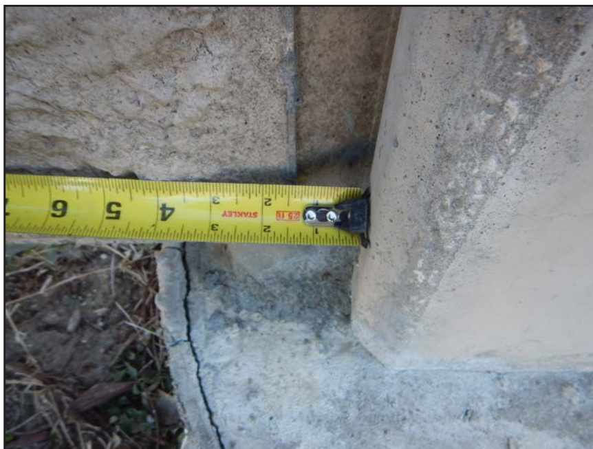
NO. 13 - COLUMN 3N - TYPICAL PRECAST COLUMN FOUNDATION
