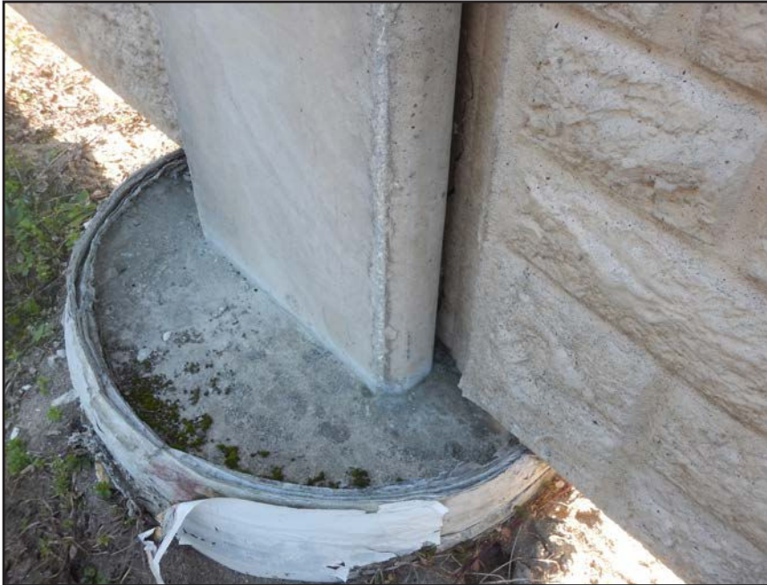
NO. 303 - COLUMN 51N - CRACKED AND FAILED TONGUE OF A PRECAST WALL PANEL IN A PRECAST COLUMN
