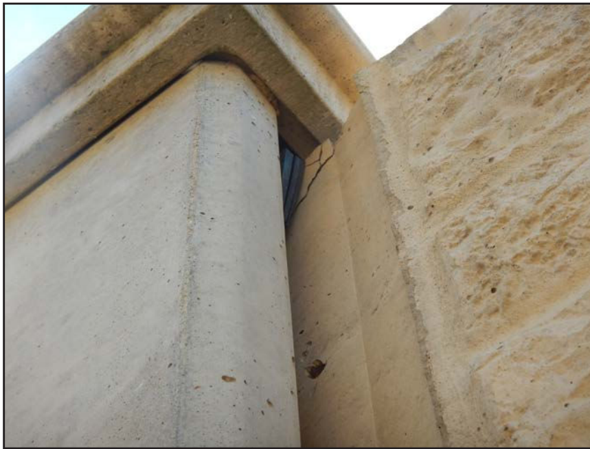
NO. 314 - COLUMN 16SM - CRACKED AND FAILED TONGUE OF A PRECAST WALL PANEL IN A PRECAST COLUMN
