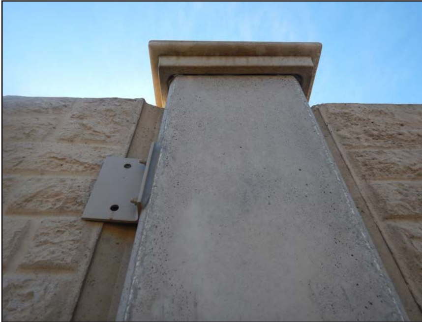
NO. 434 - COLUMN 49N - INADEQUATE ADDED CLIP ANGLE CONNECTION AT A DEFICIENT WALL PANEL TO COLUMN CONNECTION
