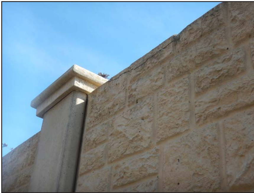
NO. 465 - COLUMN 17S - CRACKED AND SPALLED PRECAST CONCRETE
