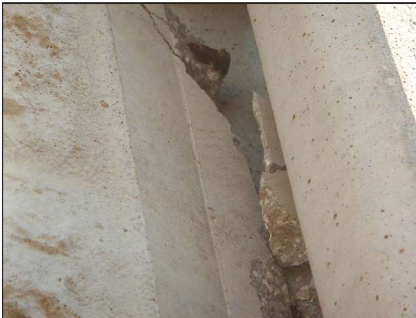
NO. 358- COLUMN 25SS - CRACKED AND FAILED TONGUE OF A PRECAST WALL PANEL IN A PRECAST COLUMN
