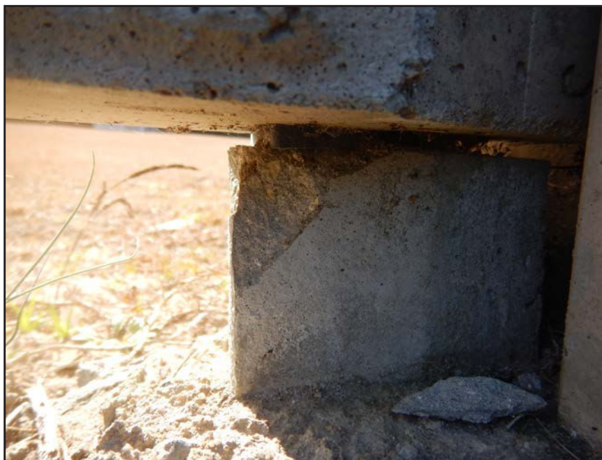
NO. 114 - COLUMN 53N - INADEQUATE BEARING OF A PRECAST WALL PANEL ON A FAILED GROUT PEDESTAL OR A FAILED PRECAST TONGUE
