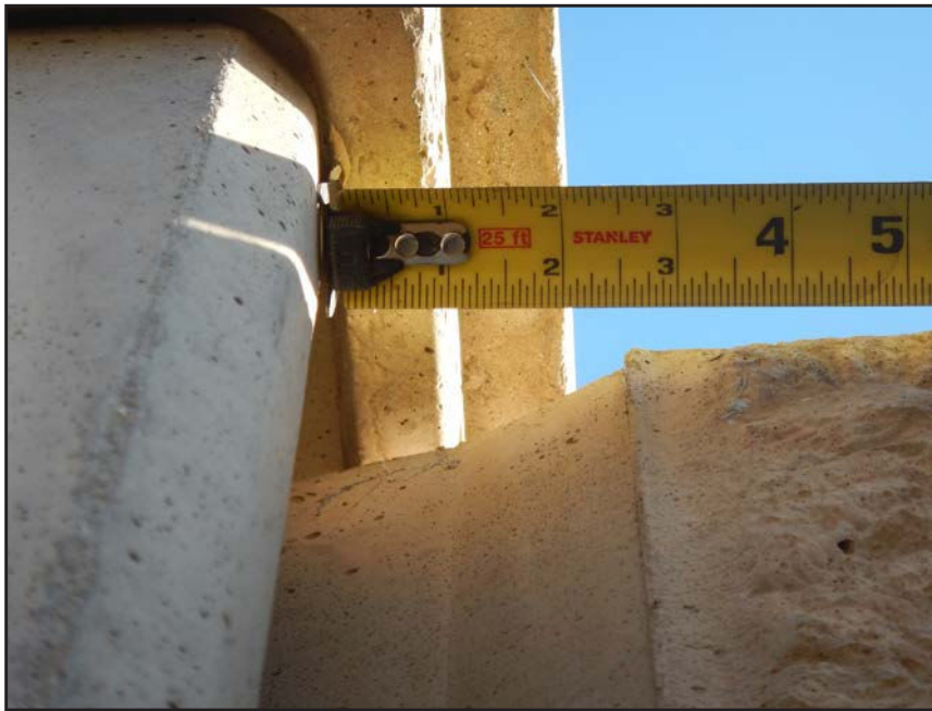
NO. 243 - COLUMN 80S - INSUFFICIENT SEATING OF A PRECAST WALL PANEL IN A PRECAST COLUMN
