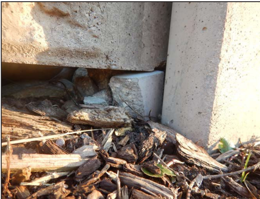
NO. 175 - COLUMN 56SS - INADEQUATE BEARING OF A PRECAST WALL PANEL ON A FAILED GROUT PEDESTAL OR A FAILED PRECAST TONGUE
