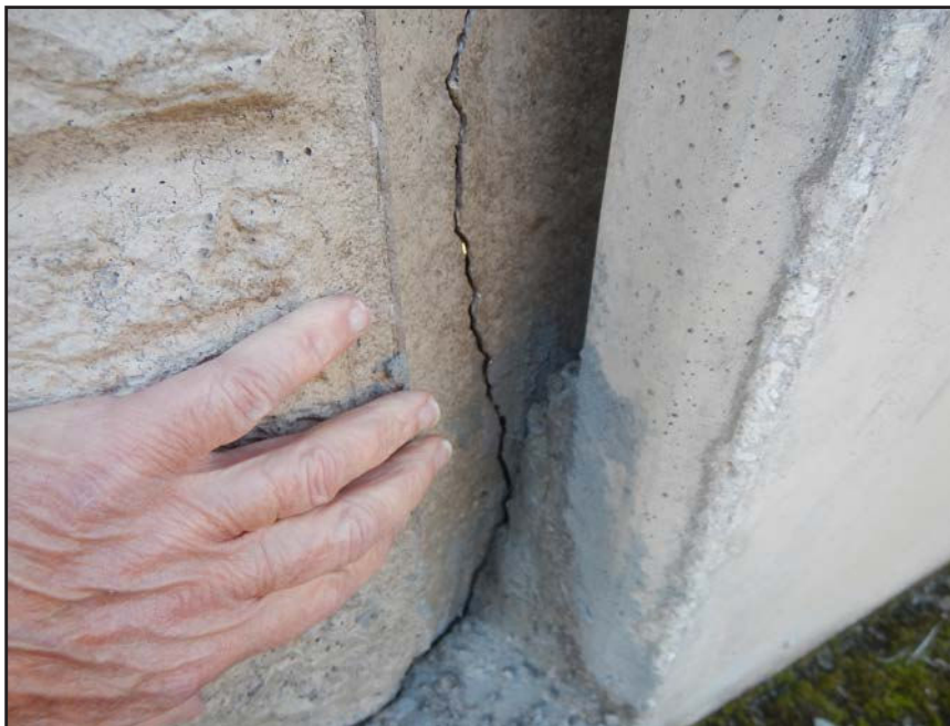
NO. 310 - COLUMN 7NM - CRACKED AND FAILED TONGUE OF A PRECAST WALL PANEL IN A PRECAST COLUMN
