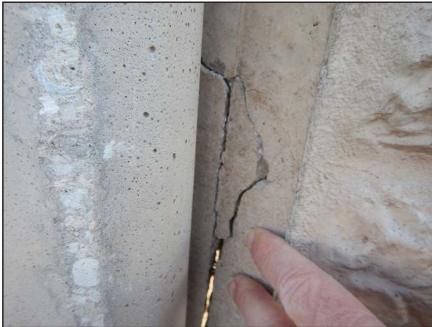
NO. 335 - COLUMN 67S - CRACKED AND FAILED TONGUE OF A PRECAST WALL PANEL IN A PRECAST COLUMN
