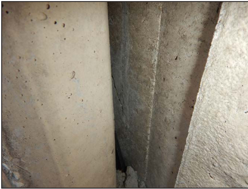
NO. 347 - COLUMN 8SS - CRACKED AND FAILED TONGUE OF A PRECAST WALL PANEL IN A PRECAST COLUMN
