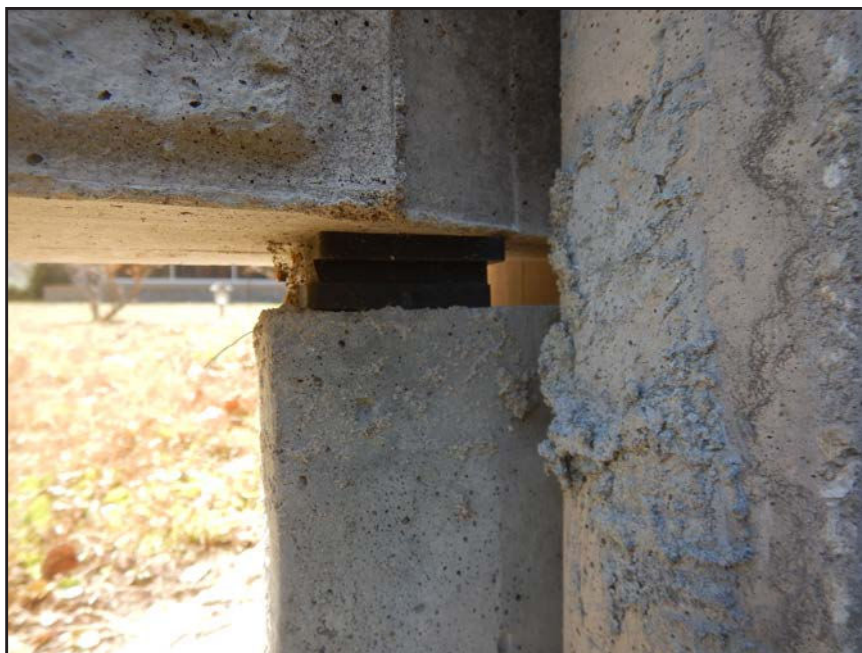
NO. 86 - COLUMN 22SM - INADEQUATE BEARING OF A PRECAST WALL PANEL ON A 2" x 2" NEOPRENE BEARING PAD
