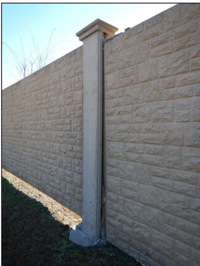
NO. 2 - COLUMN 13NM - DROPPED PRECAST PANEL WITH A CRACKED AND SPALLED TOP
