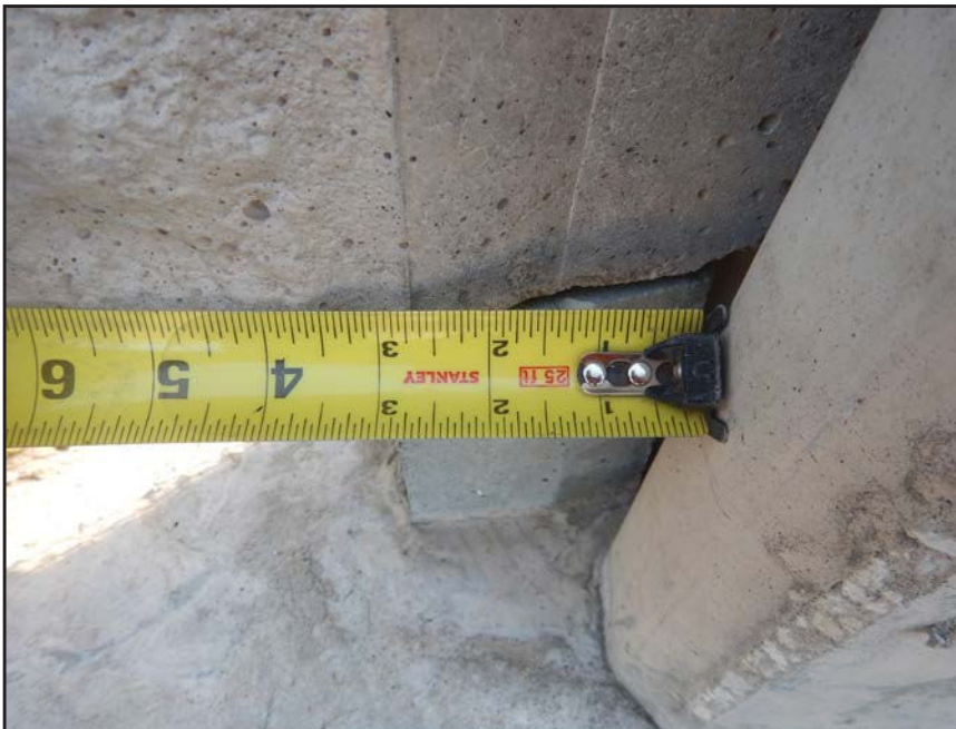
NO. 226 - COLUMN 41S - INSUFFICIENT SEATING OF A PRECAST WALL PANEL IN A PRECAST COLUMN
