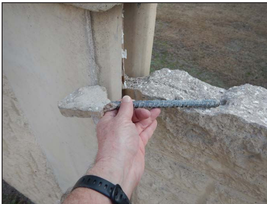
NO. 56 - SPALLED WALL PANEL ON THE SOUTH SIDE OF COLUMN 13NM - TONGUE REINFORCING DOWEL WITH INADEQUATE CONCRETE COVER
