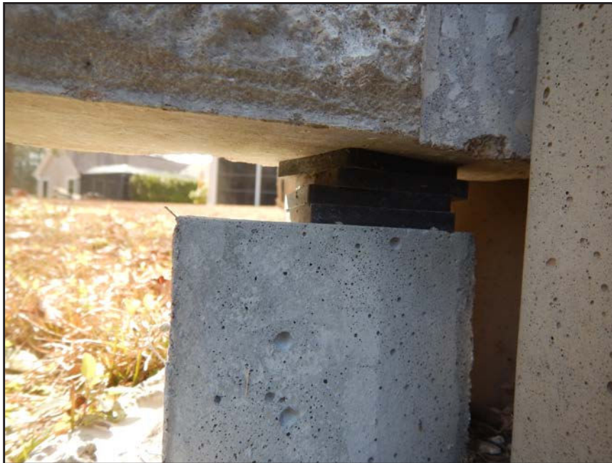
NO. 80 - COLUMN 3SM - INADEQUATE BEARING OF A PRECAST WALL PANEL ON A 2" x 2" NEOPRENE BEARING PAD
