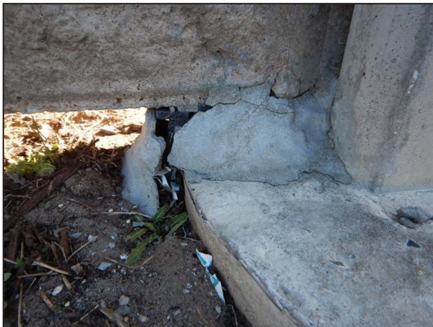
NO. 106 - COLUMN 8N - INADEQUATE BEARING OF A PRECAST WALL PANEL ON A FAILED GROUT PEDESTAL OR A FAILED PRECAST TONGUE
