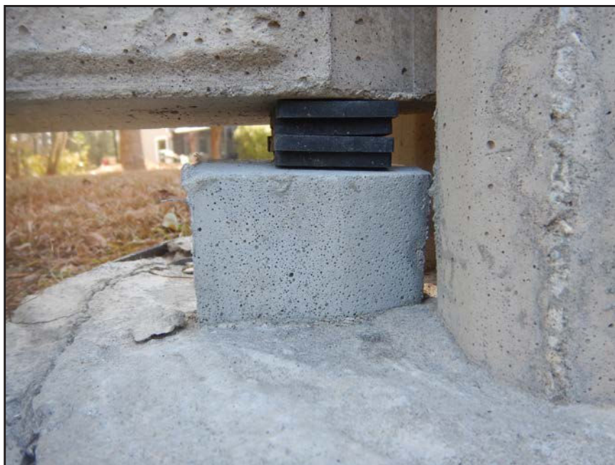
NO. 77 - COLUMN 2SM - INADEQUATE BEARING OF A PRECAST WALL PANEL ON A 2" x 2" NEOPRENE BEARING PAD
