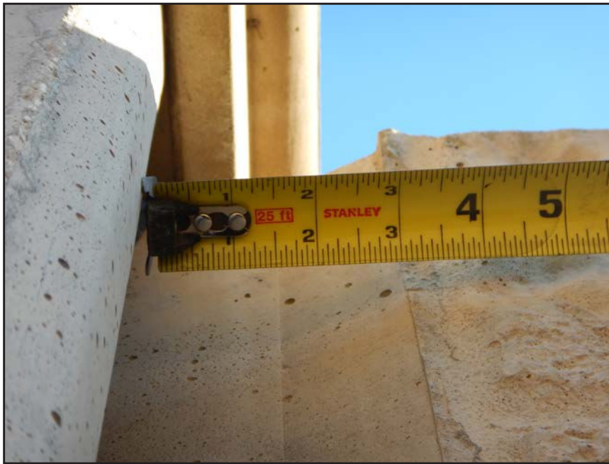
NO. 188 - COLUMN 20N - INSUFFICIENT SEATING OF A PRECAST WALL PANEL IN A PRECAST COLUMN
