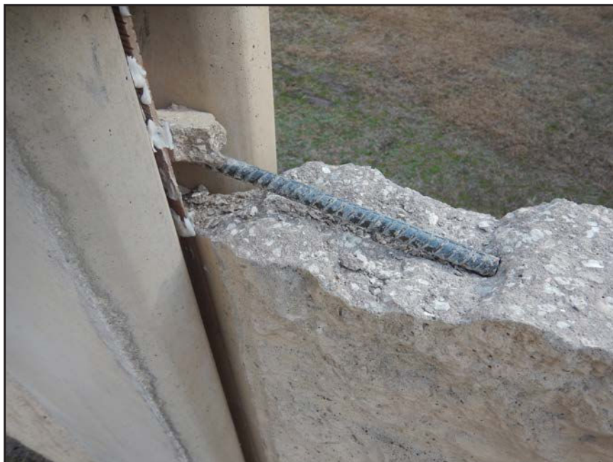
NO. 54 - SPALLED WALL PANEL ON THE SOUTH SIDE OF COLUMN 13NM - TONGUE REINFORCING DOWEL WITH INADEQUATE CONCRETE COVER
