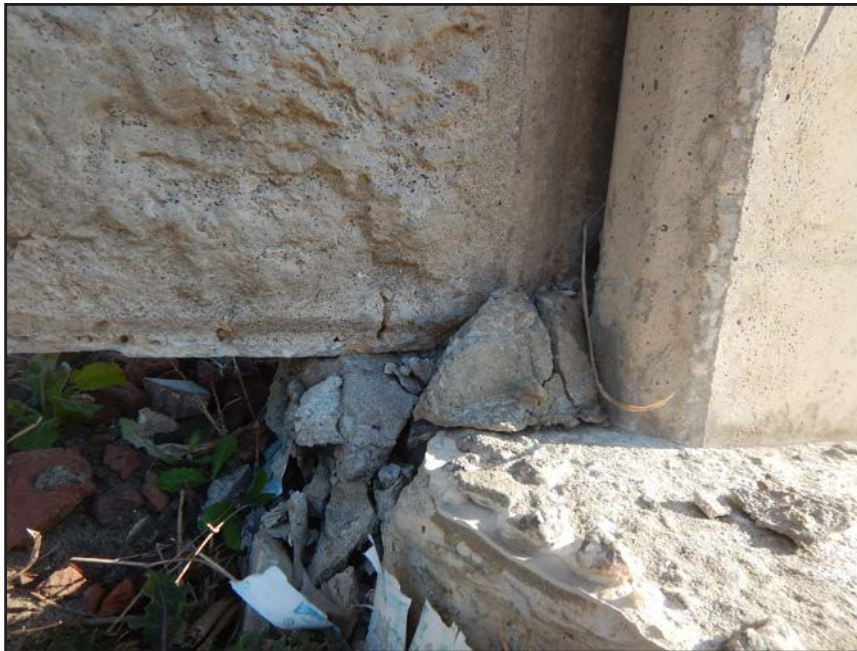
NO. 158 - COLUMN 9SS - INADEQUATE BEARING OF A PRECAST WALL PANEL ON A FAILED GROUT PEDESTAL OR A FAILED PRECAST TONGUE
