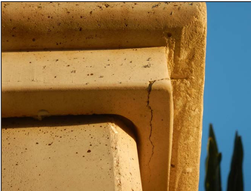
NO. 481 - COLUMN 54SS - CRACKED AND SPALLED PRECAST CONCRETE
