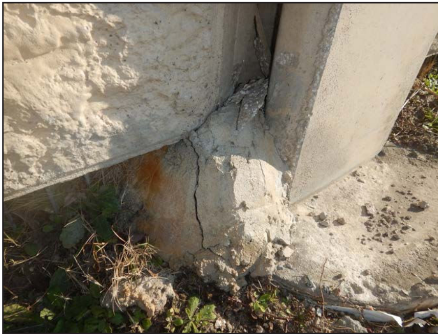
NO. 157 - COLUMN 6SS - INADEQUATE BEARING OF A PRECAST WALL PANEL ON A FAILED GROUT PEDESTAL OR A FAILED PRECAST TONGUE
