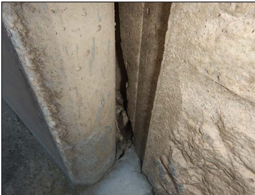
NO. 307 - COLUMN 56N - CRACKED AND FAILED TONGUE OF A PRECAST WALL PANEL IN A PRECAST COLUMN
