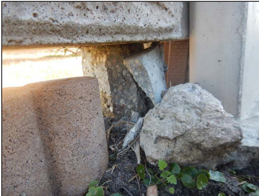
NO. 149 - COLUMN 76S - INADEQUATE BEARING OF A PRECAST WALL PANEL ON A FAILED GROUT PEDESTAL OR A FAILED PRECAST TONGUE
