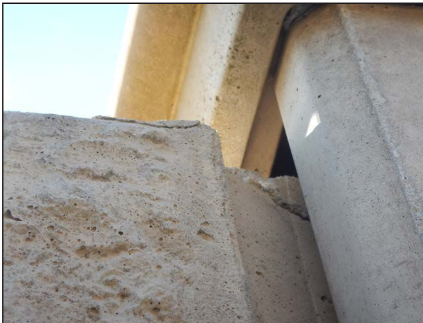
NO. 295 - COLUMN 47N - CRACKED AND FAILED TONGUE OF A PRECAST WALL PANEL IN A PRECAST COLUMN
