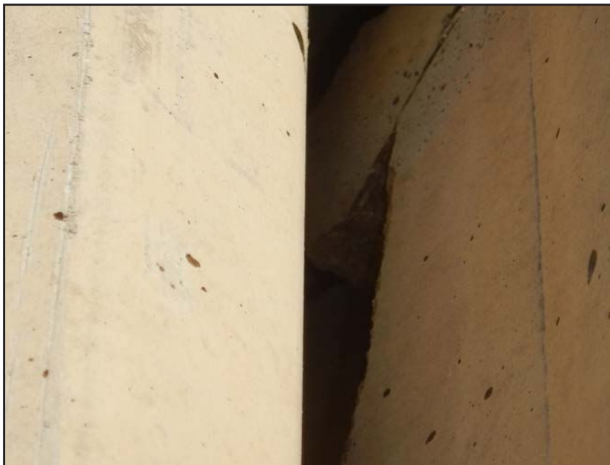
NO. 346 - COLUMN 8SS - CRACKED AND FAILED TONGUE OF A PRECAST WALL PANEL IN A PRECAST COLUMN
