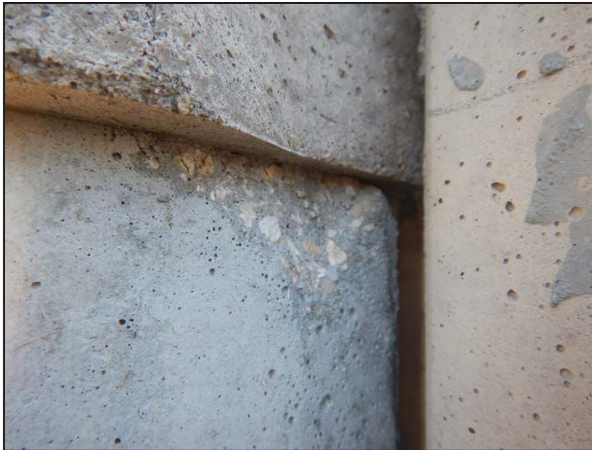
NO. 132 - COLUMN 42S - INADEQUATE BEARING OF A PRECAST WALL PANEL ON A FAILED GROUT PEDESTAL OR A FAILED PRECAST TONGUE
