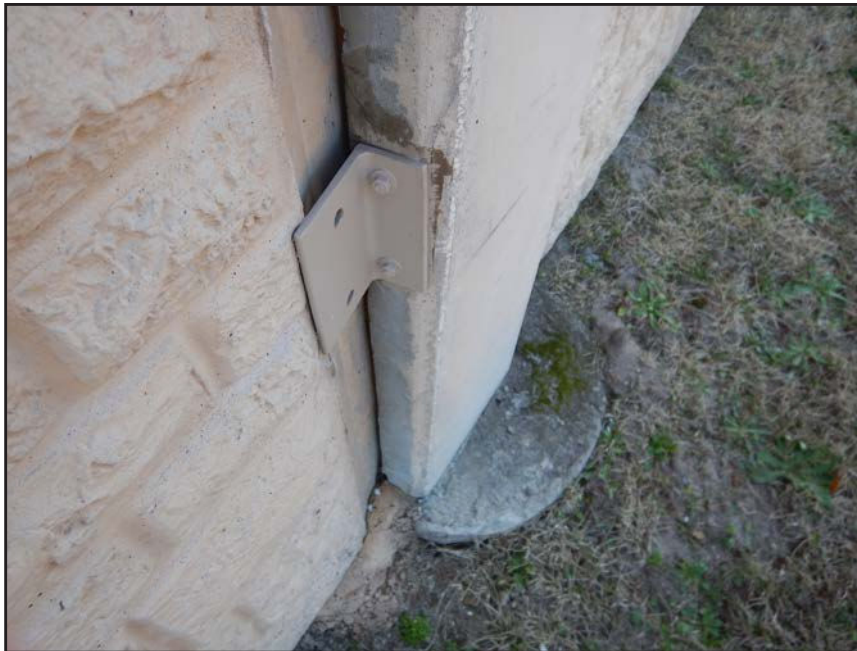
NO. 432 - COLUMN 20N - INADEQUATE ADDED CLIP ANGLE CONNECTION AT A DEFICIENT WALL PANEL TO COLUMN CONNECTION
