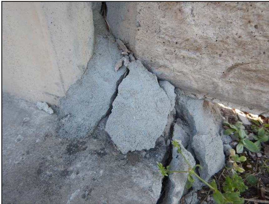
NO. 137 - COLUMN 61S - INADEQUATE BEARING OF A PRECAST WALL PANEL ON A FAILED GROUT PEDESTAL OR A FAILED PRECAST TONGUE
