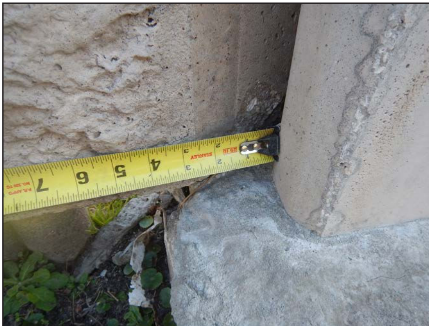
NO. 241 - COLUMN 79S - INSUFFICIENT SEATING OF A PRECAST WALL PANEL IN A PRECAST COLUMN
