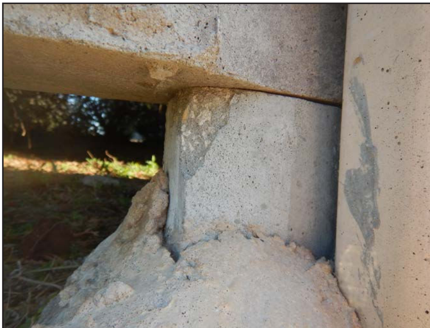
NO. 159 - COLUMN 13SS - INADEQUATE BEARING OF A PRECAST WALL PANEL ON A FAILED GROUT PEDESTAL OR A FAILED PRECAST TONGUE
