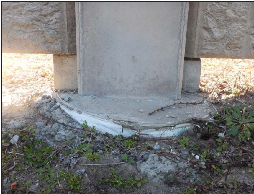
NO. 69 - COLUMN 52N - INADEQUATE BEARING OF A PRECAST WALL PANEL ON A 2" x 2" NEOPRENE BEARING PAD
