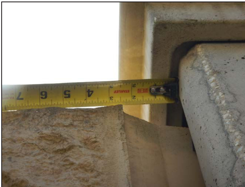
NO. 212 - COLUMN 21SM - INSUFFICIENT SEATING OF A PRECAST WALL PANEL IN A PRECAST COLUMN
