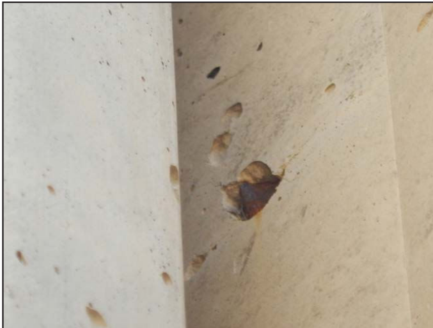
NO. 498 - COLUMN 16SM - EXPOSED REINFORCING STEEL WITH INADEQUATE CONCRETE COVER
