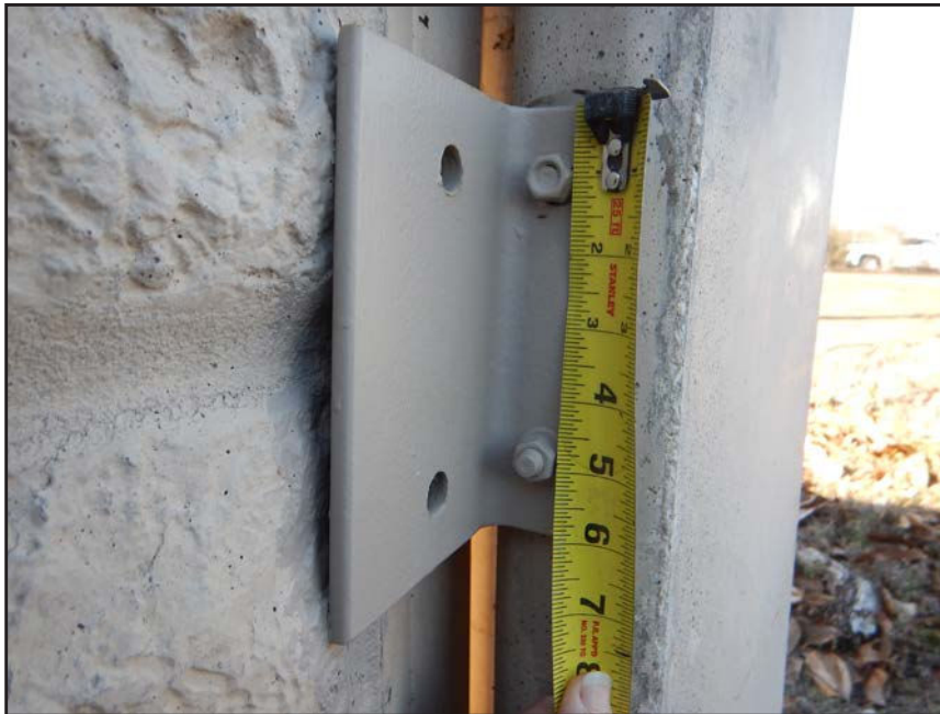
NO. 407 - COLUMN 1NE - INADEQUATE ADDED CLIP ANGLE CONNECTION AT A DEFICIENT WALL PANEL TO COLUMN CONNECTION
