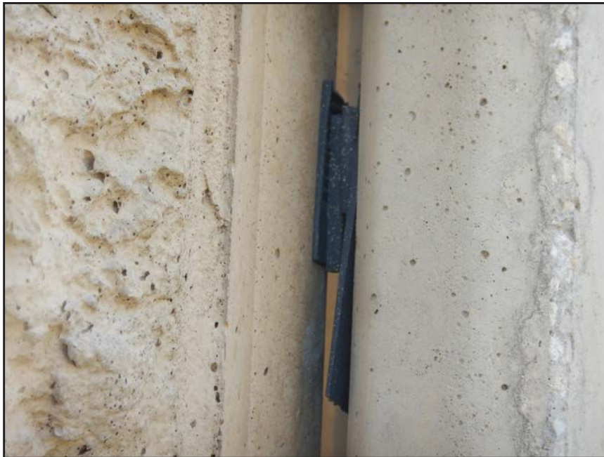
NO. 274 - COLUMN 10S - INADEQUATE SHIMS STABILIZING A WALL PANEL TO COLUMN CONNECTION AT EXCESSIVE PLAY BETWEEN ADJACENT MEMBERS
