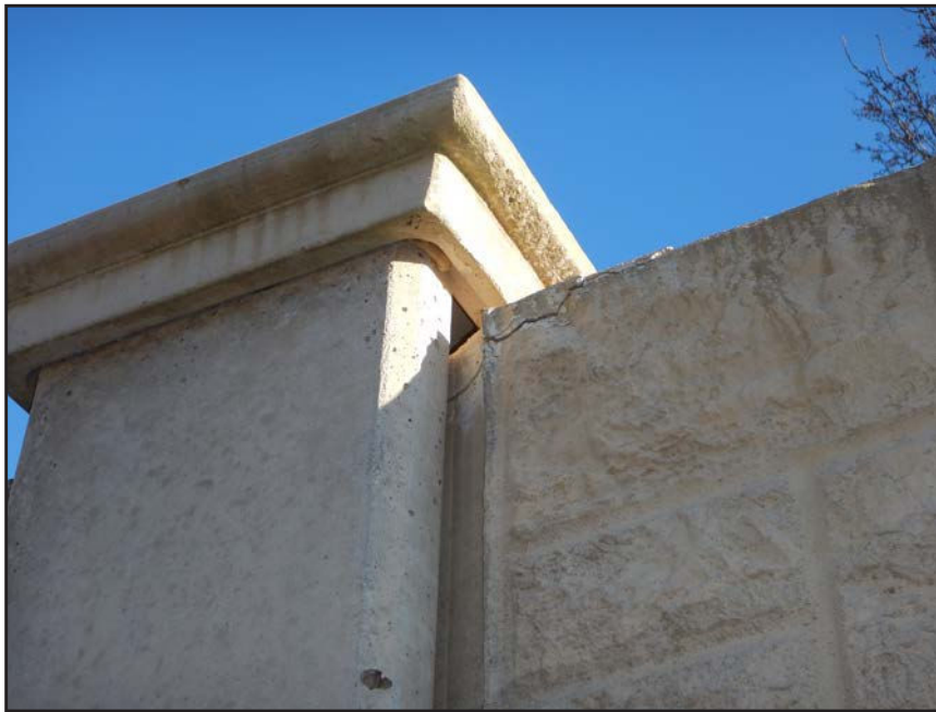
NO. 462 - COLUMN 42N - CRACKED AND SPALLED PRECAST CONCRETE
