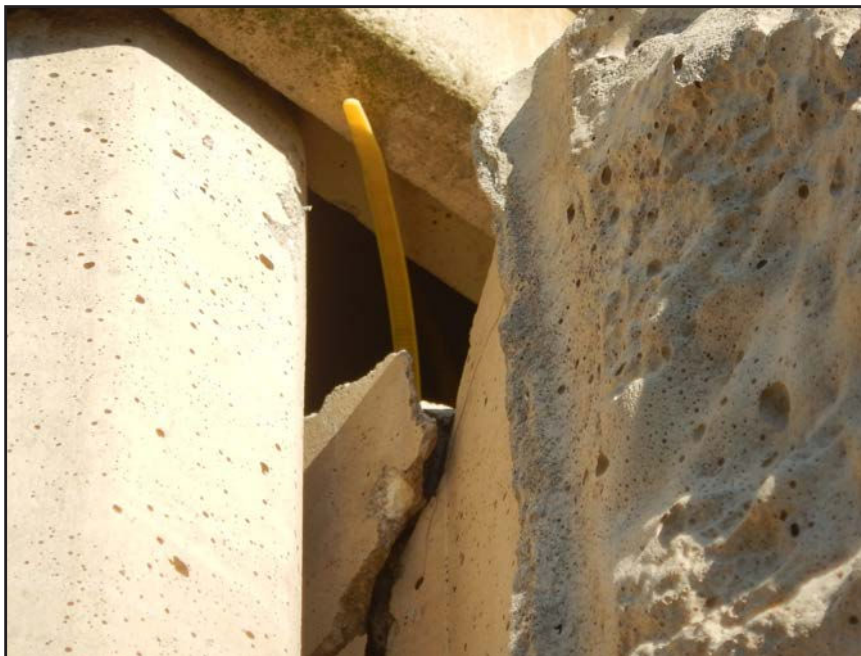
NO. 352 - COLUMN 20SS - CRACKED AND FAILED TONGUE OF A PRECAST WALL PANEL IN A PRECAST COLUMN
