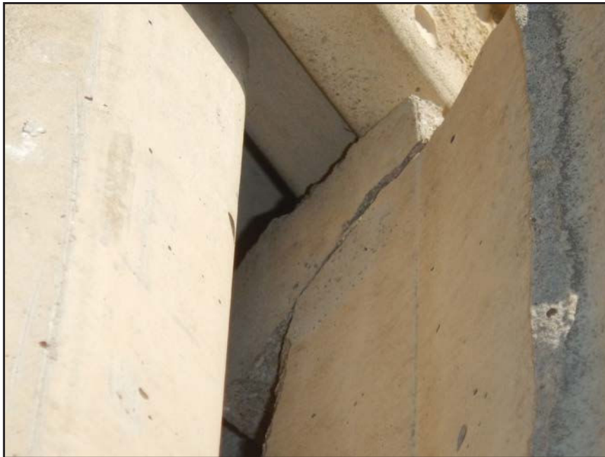
NO. 345 - COLUMN 8SS - CRACKED AND FAILED TONGUE OF A PRECAST WALL PANEL IN A PRECAST COLUMN
