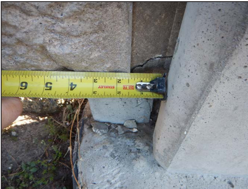
NO. 288 - COLUMN 10N - CRACKED AND FAILED TONGUE OF A PRECAST WALL PANEL IN A PRECAST COLUMN
