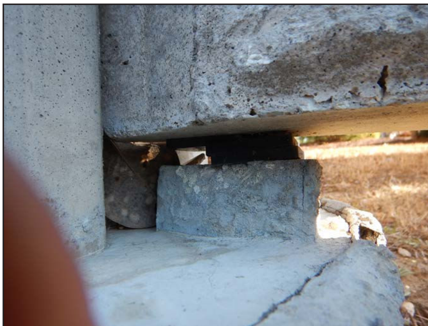
NO. 17 - COLUMN 3N - TYPICAL WALL PANEL BEARING CONDITION AT A GROUT PEDESTAL WITH 2" x 2" NEOPRENE BEARING PADS
