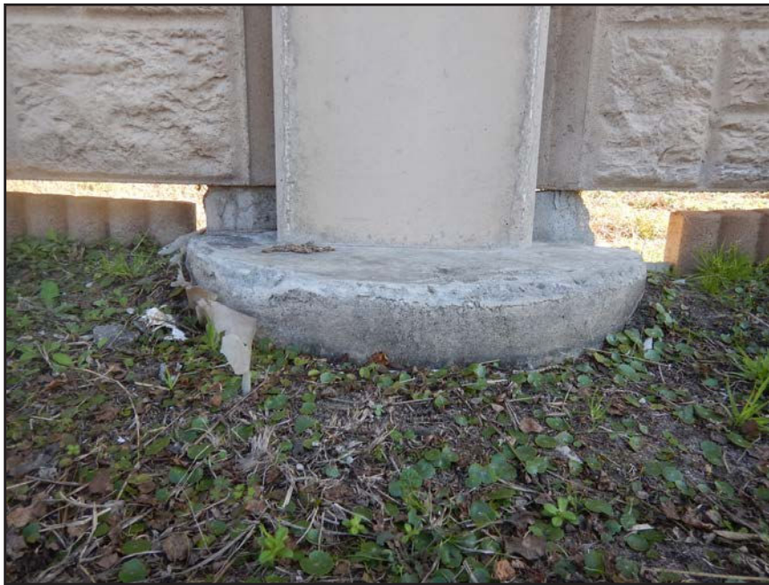
NO. 145 - COLUMN 75S - INADEQUATE BEARING OF A PRECAST WALL PANEL ON A FAILED GROUT PEDESTAL OR A FAILED PRECAST TONGUE
