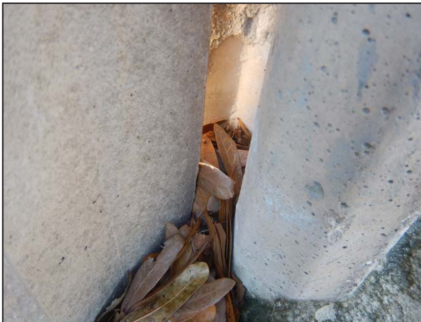
NO. 201 - COLUMN 2NM - INSUFFICIENT SEATING OF A PRECAST WALL PANEL IN A PRECAST COLUMN
