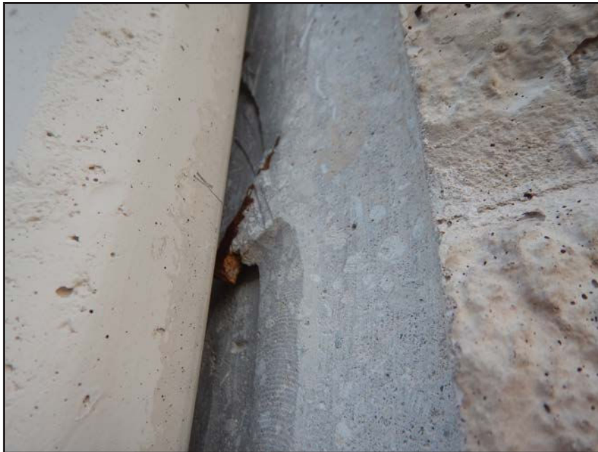
NO. 506 - COLUMN 79SS - EXPOSED REINFORCING STEEL WITH INADEQUATE CONCRETE COVER
