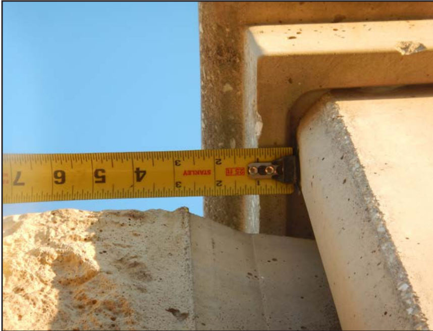
NO. 256 - COLUMN 51SS - INSUFFICIENT SEATING OF A PRECAST WALL PANEL IN A PRECAST COLUMN
