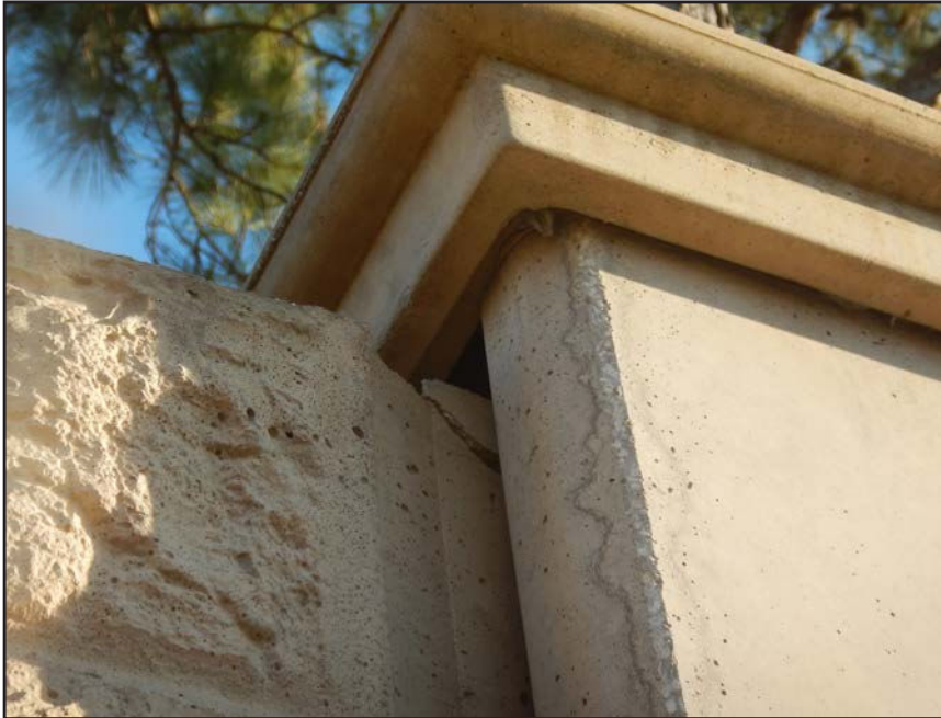
NO. 363 - COLUMN 37SS - CRACKED AND FAILED TONGUE OF A PRECAST WALL PANEL IN A PRECAST COLUMN
