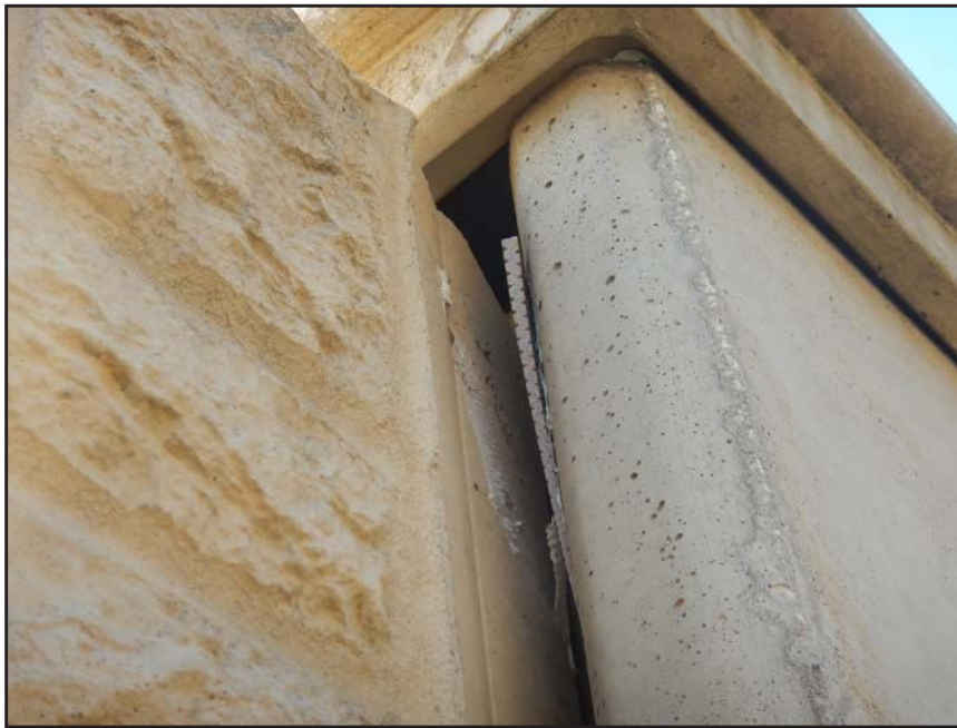
NO. 267 - COLUMN 17SM - INADEQUATE SHIMS STABILIZING A WALL PANEL TO COLUMN CONNECTION AT EXCESSIVE PLAY BETWEEN ADJACENT MEMBERS
