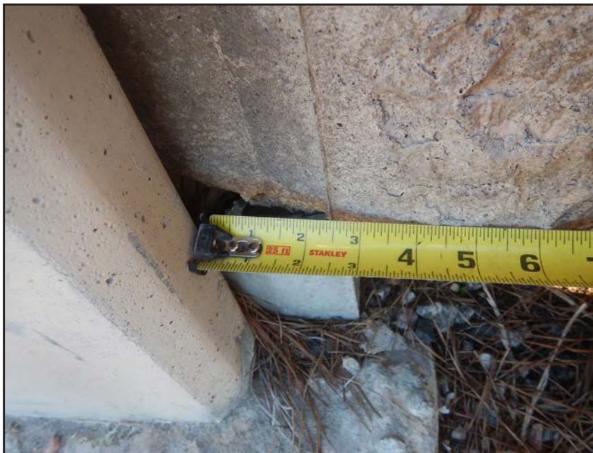
NO. 253 - COLUMN 32SS - INSUFFICIENT SEATING OF A PRECAST WALL PANEL IN A PRECAST COLUMN
