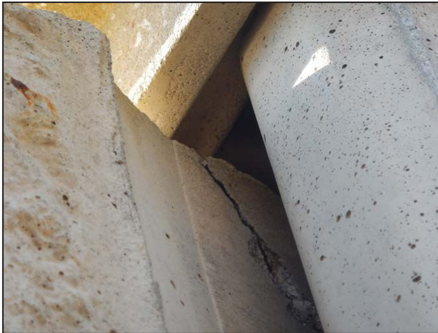
NO. 294 - COLUMN 44N - CRACKED AND FAILED TONGUE OF A PRECAST WALL PANEL IN A PRECAST COLUMN
