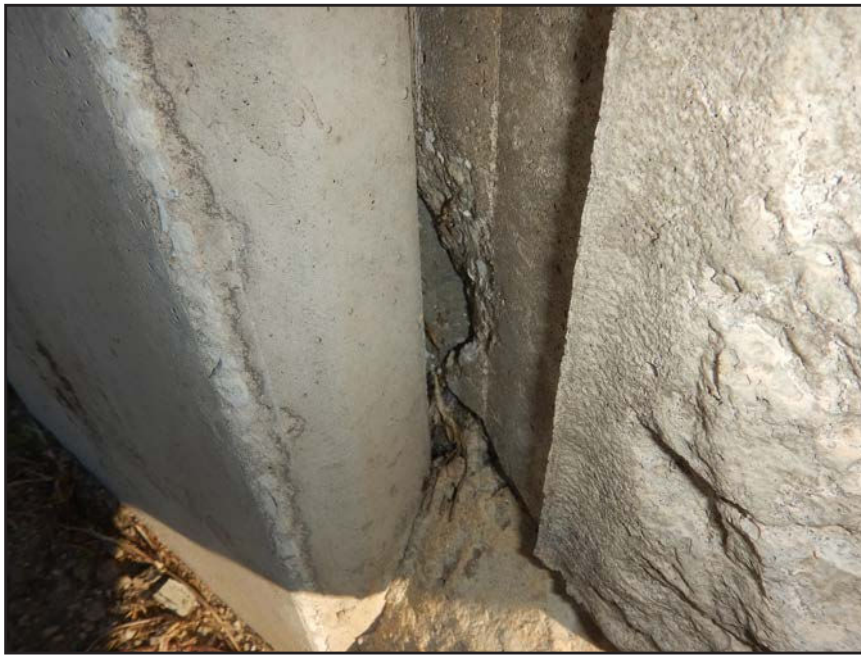
NO. 350 - COLUMN 18SS - CRACKED AND FAILED TONGUE OF A PRECAST WALL PANEL IN A PRECAST COLUMN
