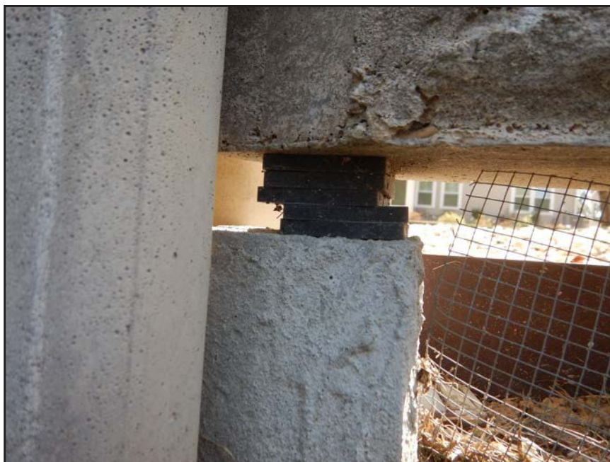
NO. 89 - COLUMN 8S - INADEQUATE BEARING OF A PRECAST WALL PANEL ON A 2" x 2" NEOPRENE BEARING PAD
