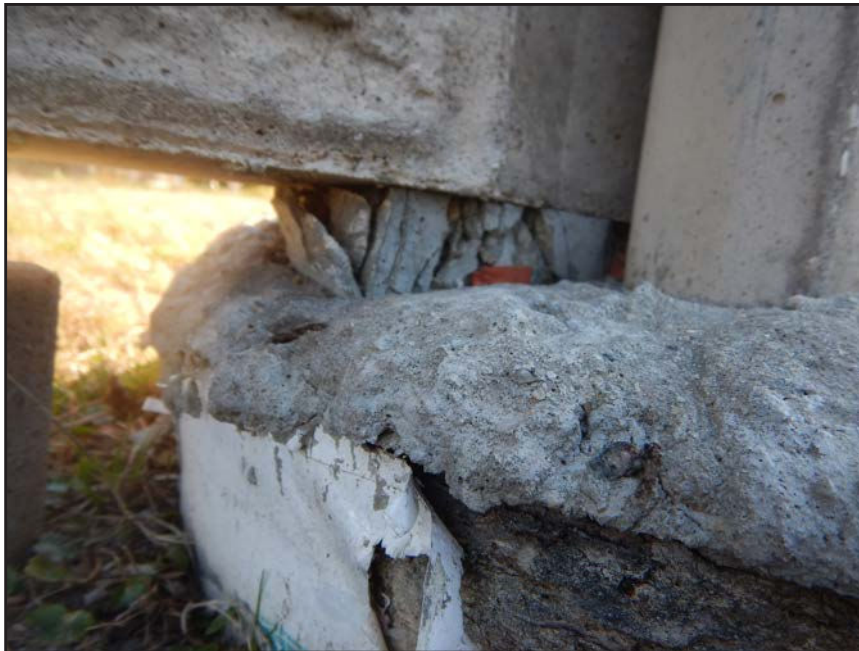
NO. 143 - COLUMN 73S - INADEQUATE BEARING OF A PRECAST WALL PANEL ON A FAILED GROUT PEDESTAL OR A FAILED PRECAST TONGUE
