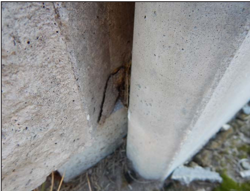
NO. 292 - COLUMN 33N - CRACKED AND FAILED TONGUE OF A PRECAST WALL PANEL IN A PRECAST COLUMN
