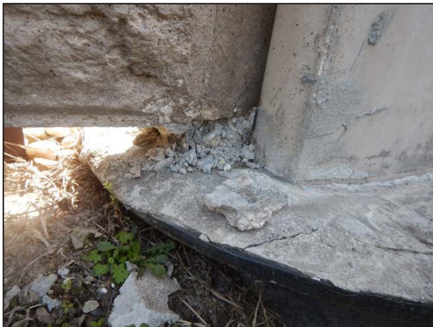
NO. 125 - COLUMN 12S - INADEQUATE BEARING OF A PRECAST WALL PANEL ON A FAILED GROUT PEDESTAL OR A FAILED PRECAST TONGUE
