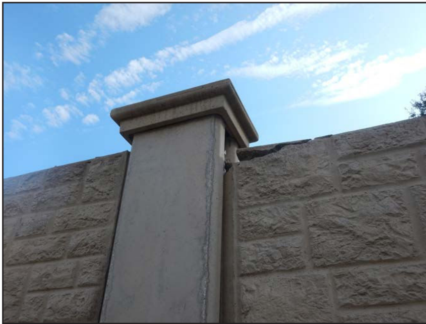
NO. 51 - SPALLED WALL PANEL ON THE SOUTH SIDE OF COLUMN 13NM
