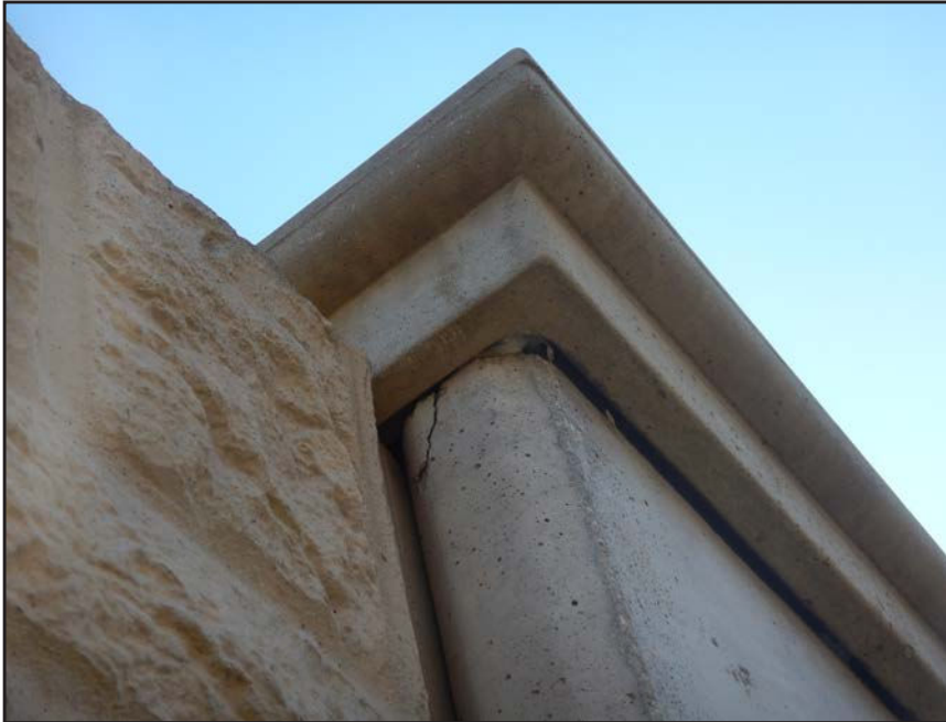
NO. 473 - COLUMN 77S - CRACKED AND SPALLED PRECAST CONCRETE
