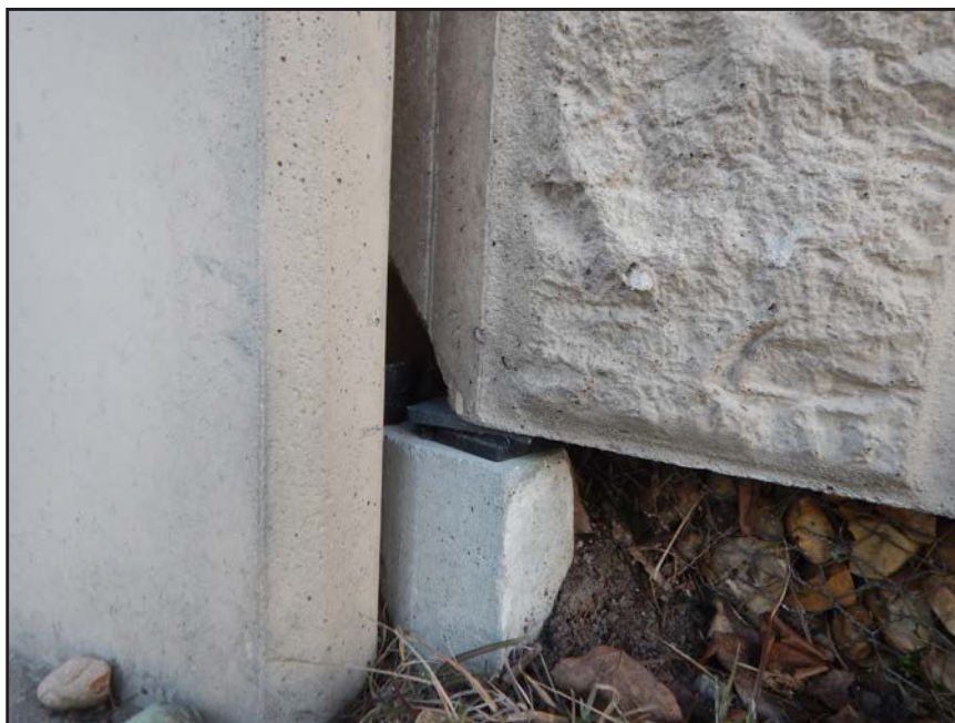
NO. 104 - COLUMN 78SS - INADEQUATE BEARING OF A PRECAST WALL PANEL ON A 2" x 2" NEOPRENE BEARING PAD
