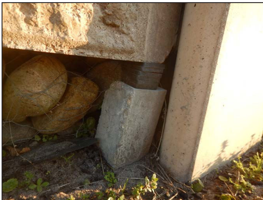
NO. 96 - COLUMN 51SS - INADEQUATE BEARING OF A PRECAST WALL PANEL ON A 2" x 2" NEOPRENE BEARING PAD
