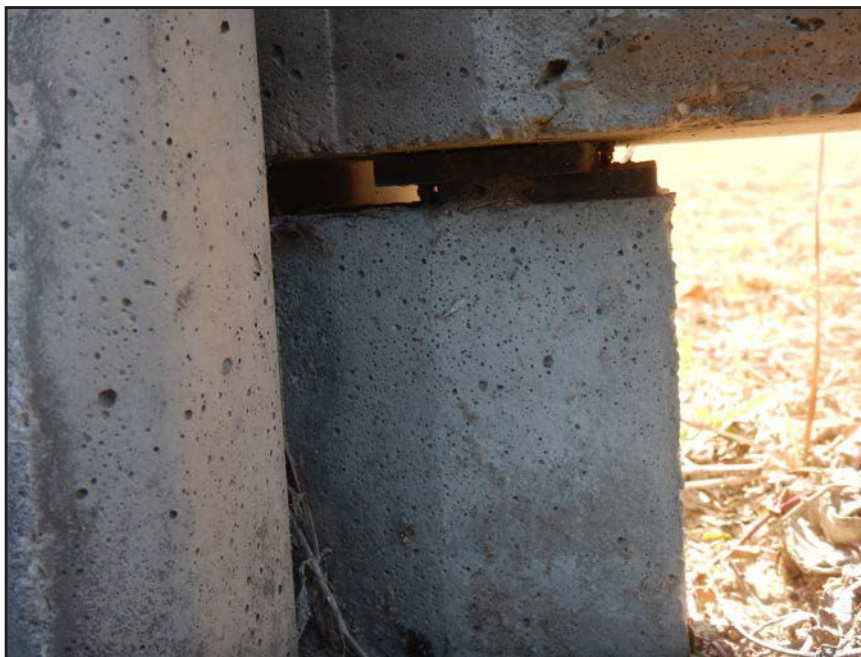
NO. 70 - COLUMN 52N - INADEQUATE BEARING OF A PRECAST WALL PANEL ON A 2" x 2" NEOPRENE BEARING PAD
