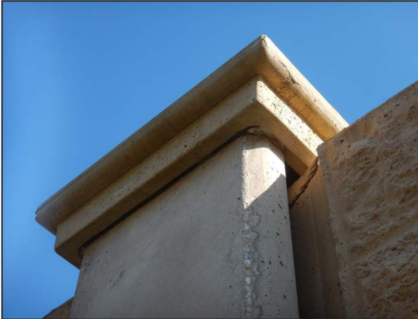
NO. 340 - COLUMN 77S - CRACKED AND FAILED TONGUE OF A PRECAST WALL PANEL IN A PRECAST COLUMN
