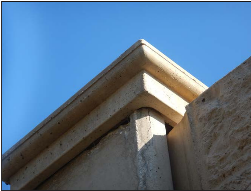
NO. 470 - COLUMN 75S - CRACKED AND SPALLED PRECAST CONCRETE
