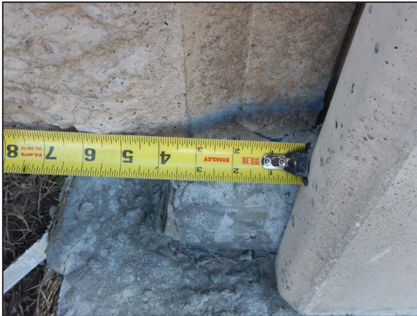
NO. 184 - COLUMN 12N - INSUFFICIENT SEATING OF A PRECAST WALL PANEL IN A PRECAST COLUMN
