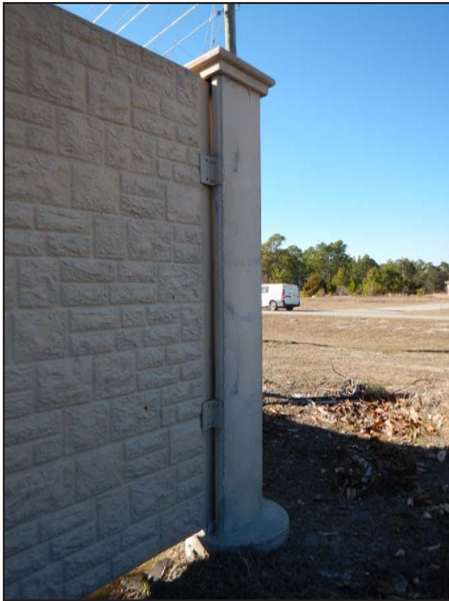
NO. 401 - COLUMN 1NE - INADEQUATE ADDED CLIP ANGLE CONNECTION AT A DEFICIENT WALL PANEL TO COLUMN CONNECTION
