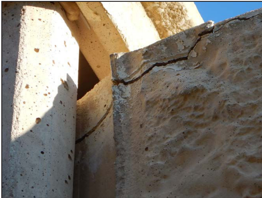
NO. 463 - COLUMN 42N - CRACKED AND SPALLED PRECAST CONCRETE
