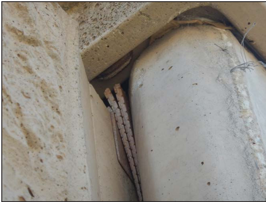
NO. 281 - COLUMN 45S - INADEQUATE SHIMS STABILIZING A WALL PANEL TO COLUMN CONNECTION AT EXCESSIVE PLAY BETWEEN ADJACENT MEMBERS
