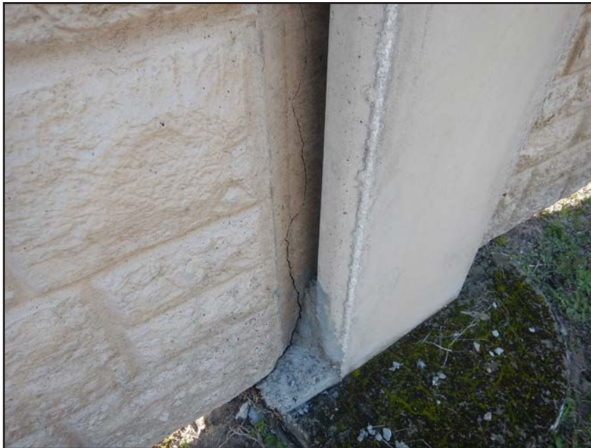
NO. 309 - COLUMN 7NM - CRACKED AND FAILED TONGUE OF A PRECAST WALL PANEL IN A PRECAST COLUMN
