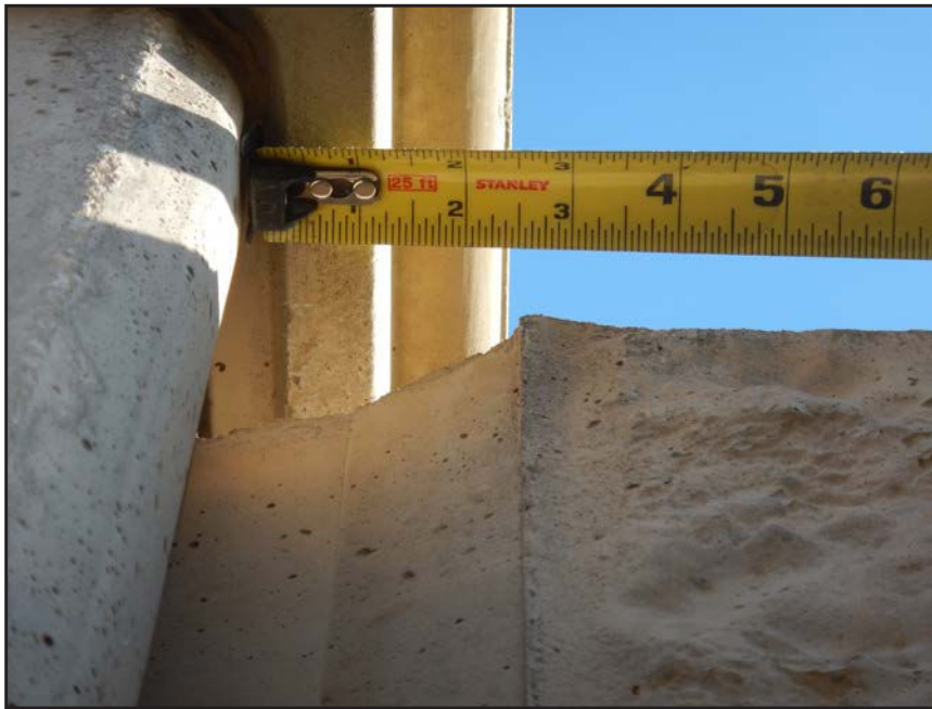
NO. 235 - COLUMN 69S - INSUFFICIENT SEATING OF A PRECAST WALL PANEL IN A PRECAST COLUMN
