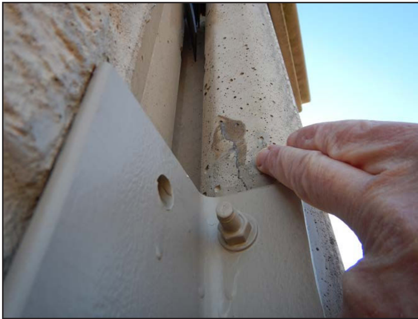
NO. 431 - COLUMN 20N - INADEQUATE ADDED CLIP ANGLE CONNECTION AT A DEFICIENT WALL PANEL TO COLUMN CONNECTION
