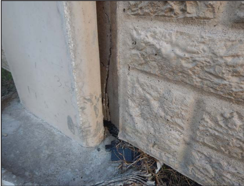
NO. 391 - COLUMN 69SS - CRACKED AND FAILED TONGUE OF A PRECAST WALL PANEL IN A PRECAST COLUMN
