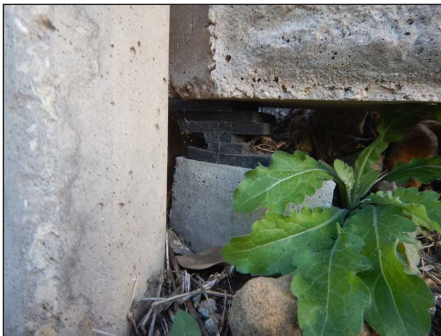
NO. 99 - COLUMN 66S - INADEQUATE BEARING OF A PRECAST WALL PANEL ON A 2" x 2" NEOPRENE BEARING PAD
