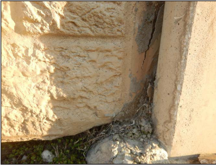
NO. 373 - COLUMN 47SS - CRACKED AND FAILED TONGUE OF A PRECAST WALL PANEL IN A PRECAST COLUMN
