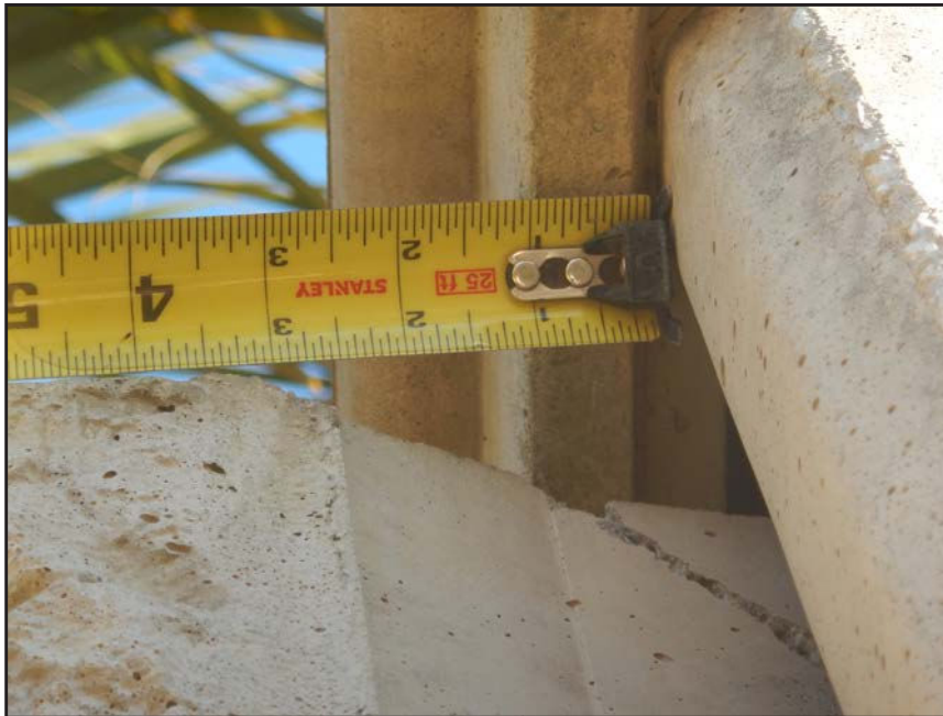
NO. 244 - COLUMN 6SS - INSUFFICIENT SEATING OF A PRECAST WALL PANEL IN A PRECAST COLUMN
