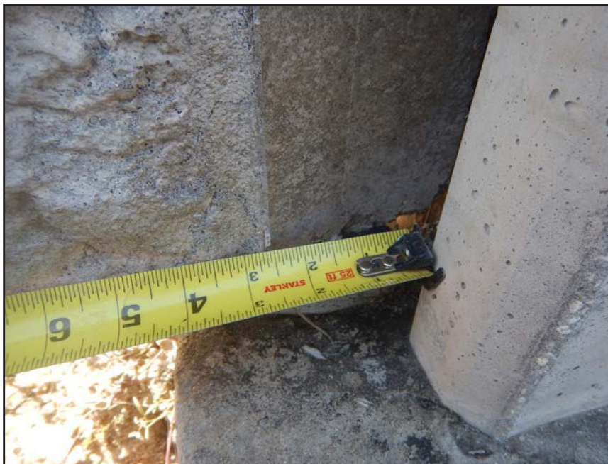
NO. 195 - COLUMN 54N - INSUFFICIENT SEATING OF A PRECAST WALL PANEL IN A PRECAST COLUMN
