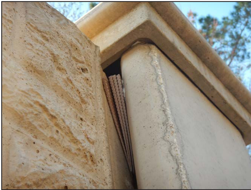
NO. 270 - COLUMN 25SM - INADEQUATE SHIMS STABILIZING A WALL PANEL TO COLUMN CONNECTION AT EXCESSIVE PLAY BETWEEN ADJACENT MEMBERS
