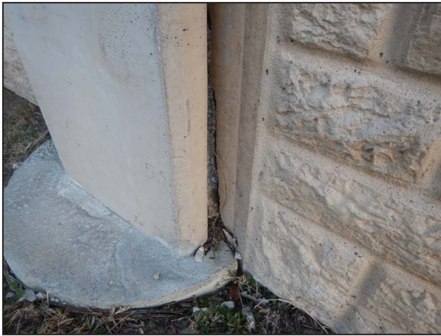
NO. 393 - COLUMN 70SS - CRACKED AND FAILED TONGUE OF A PRECAST WALL PANEL IN A PRECAST COLUMN
