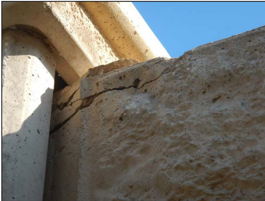
NO. 476 - COLUMN 78S - CRACKED AND SPALLED PRECAST CONCRETE
