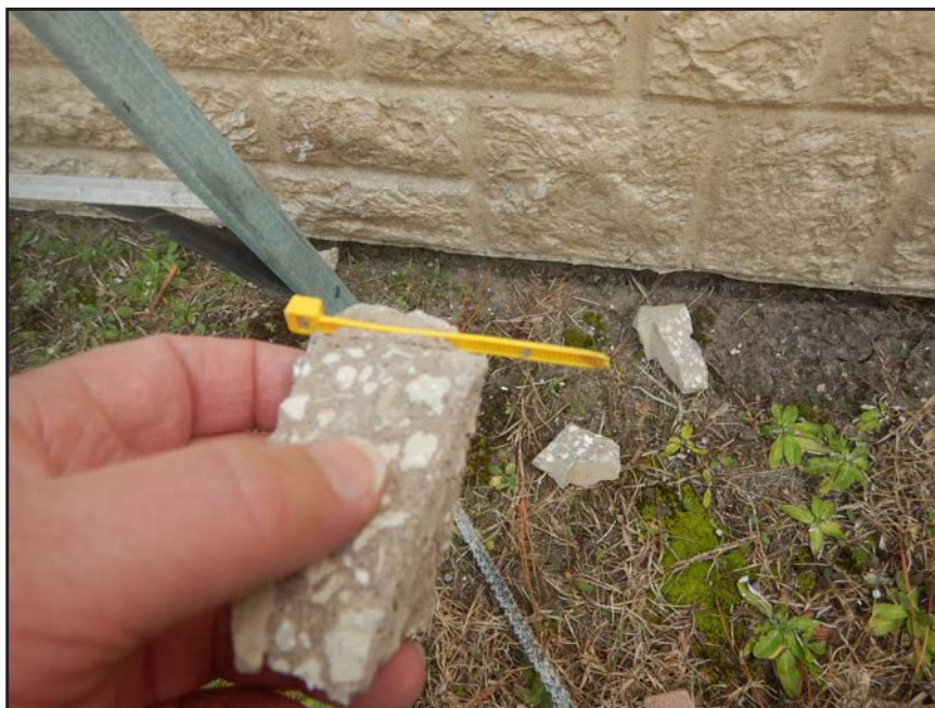
NO. 61 - SPALLED WALL PANEL ON THE SOUTH SIDE OF COLUMN 13NM - EMBEDDED ZIP TIES
