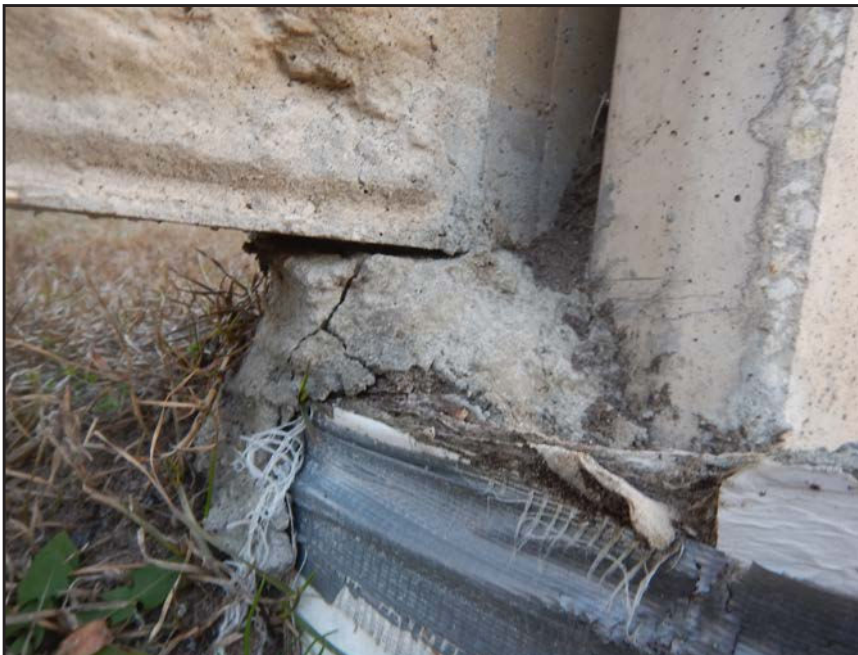
NO. 180 - COLUMN 69SS - INADEQUATE BEARING OF A PRECAST WALL PANEL ON A FAILED GROUT PEDESTAL OR A FAILED PRECAST TONGUE
