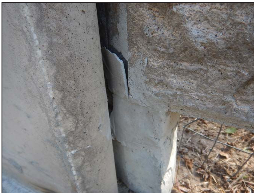
NO. 127 - COLUMN 20S - INADEQUATE BEARING OF A PRECAST WALL PANEL ON A FAILED GROUT PEDESTAL OR A FAILED PRECAST TONGUE
