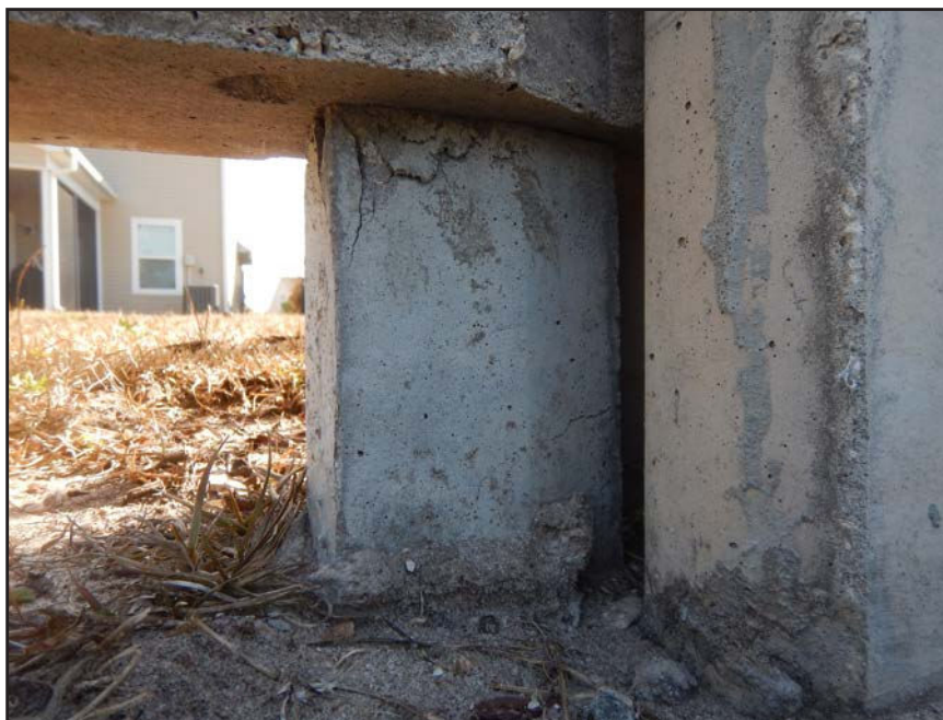
NO. 130 - COLUMN 40S - INADEQUATE BEARING OF A PRECAST WALL PANEL ON A FAILED GROUT PEDESTAL OR A FAILED PRECAST TONGUE
