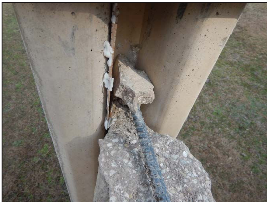
NO. 55 - SPALLED WALL PANEL ON THE SOUTH SIDE OF COLUMN 13NM - TONGUE REINFORCING DOWEL WITH INADEQUATE CONCRETE COVER
