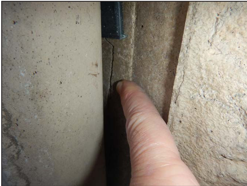
NO. 338 - COLUMN 70S - CRACKED AND FAILED TONGUE OF A PRECAST WALL PANEL IN A PRECAST COLUMN
