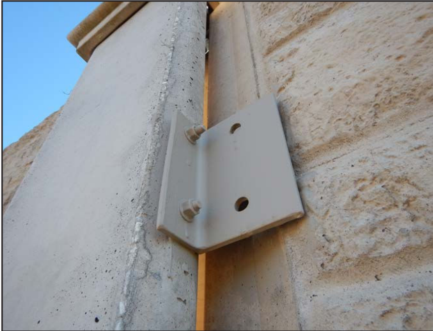
NO. 418 - COLUMN 10N - INADEQUATE ADDED CLIP ANGLE CONNECTION AT A DEFICIENT WALL PANEL TO COLUMN CONNECTION
