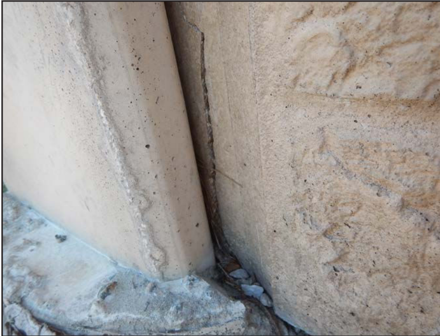
NO. 361 - COLUMN 28SS - CRACKED AND FAILED TONGUE OF A PRECAST WALL PANEL IN A PRECAST COLUMN
