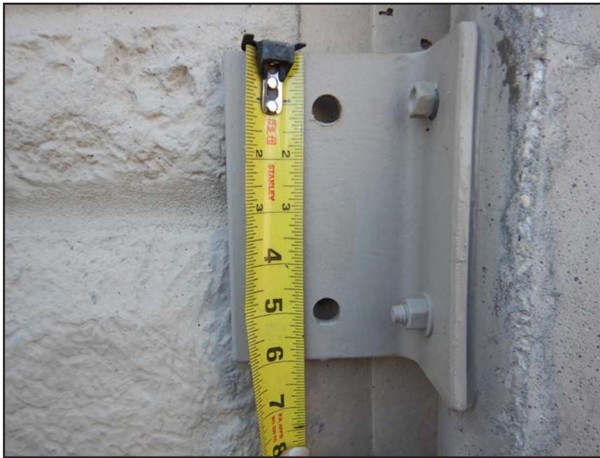
NO. 406 - COLUMN 1NE - INADEQUATE ADDED CLIP ANGLE CONNECTION AT A DEFICIENT WALL PANEL TO COLUMN CONNECTION
