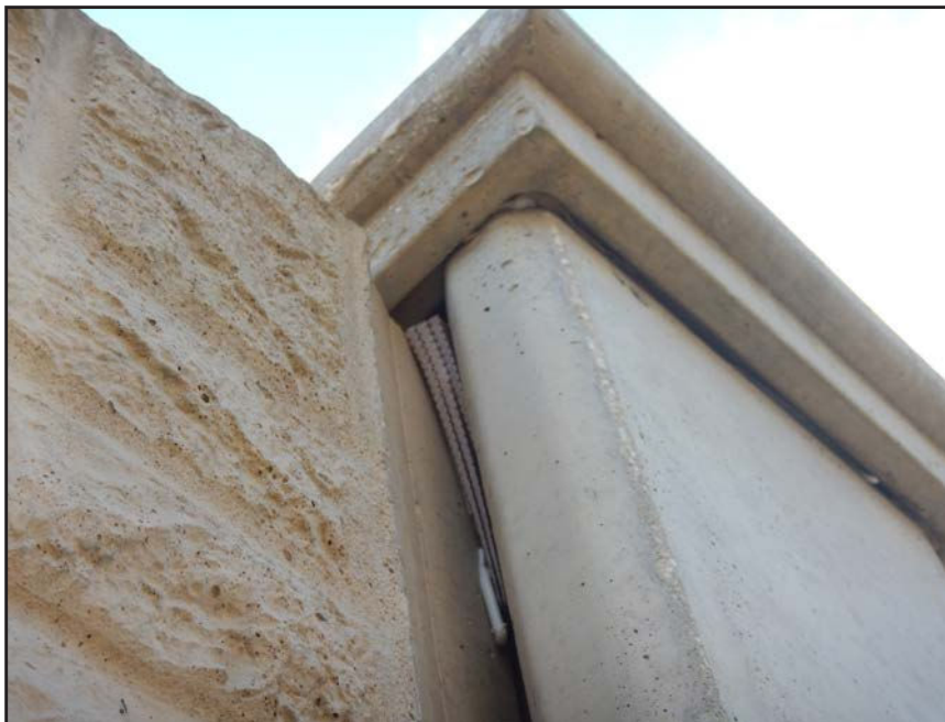
NO. 275 - COLUMN 23S - INADEQUATE SHIMS STABILIZING A WALL PANEL TO COLUMN CONNECTION AT EXCESSIVE PLAY BETWEEN ADJACENT MEMBERS
