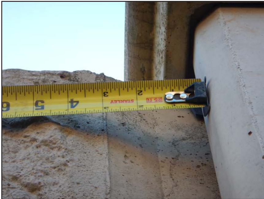
NO. 10 - COLUMN 14NM - DROPPED PRECAST PANEL WITH A 2 7/8" GAP AT THE TOP AND A 1" GAP AT THE BOTTOM
