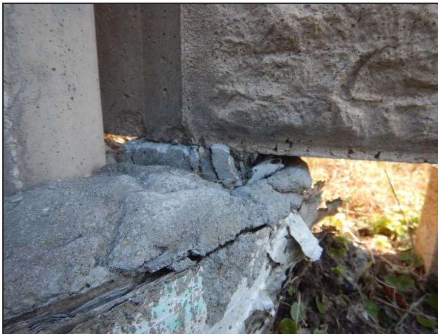
NO. 144 - COLUMN 73S - INADEQUATE BEARING OF A PRECAST WALL PANEL ON A FAILED GROUT PEDESTAL OR A FAILED PRECAST TONGUE
