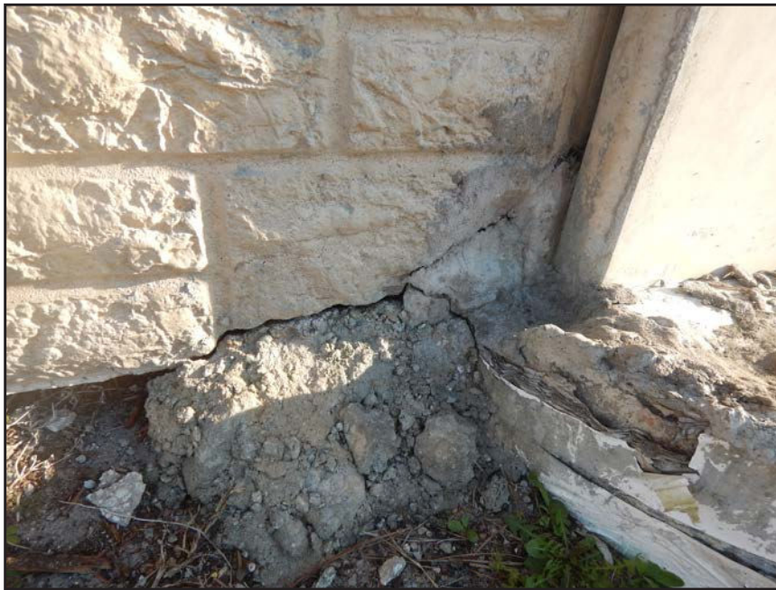
NO. 163 - COLUMN 21SS - INADEQUATE BEARING OF A PRECAST WALL PANEL ON A FAILED GROUT PEDESTAL OR A FAILED PRECAST TONGUE
