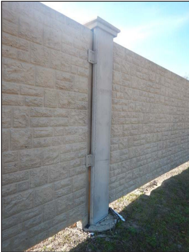
NO. 436 - COLUMN 50N - INADEQUATE ADDED CLIP ANGLE CONNECTION AT A DEFICIENT WALL PANEL TO COLUMN CONNECTION
