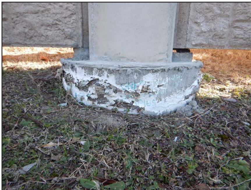
NO. 15 - COLUMN 3N - TYPICAL WALL PANEL BEARING CONDITIONS AT A GROUT PEDESTAL, AND AT A GROUT PEDESTAL WITH 2" x 2" NEOPRENE BEARING PADS
