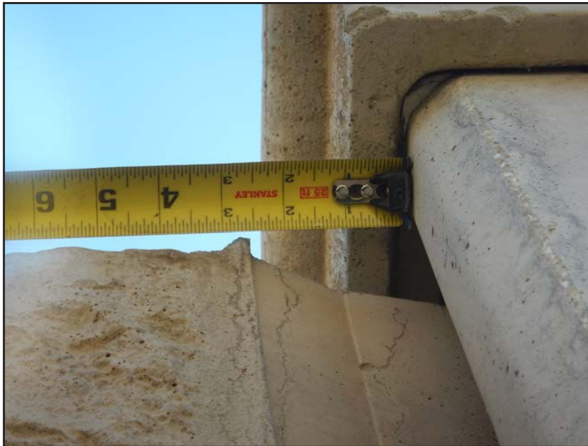
NO. 220 - COLUMN 29S - INSUFFICIENT SEATING OF A PRECAST WALL PANEL IN A PRECAST COLUMN
