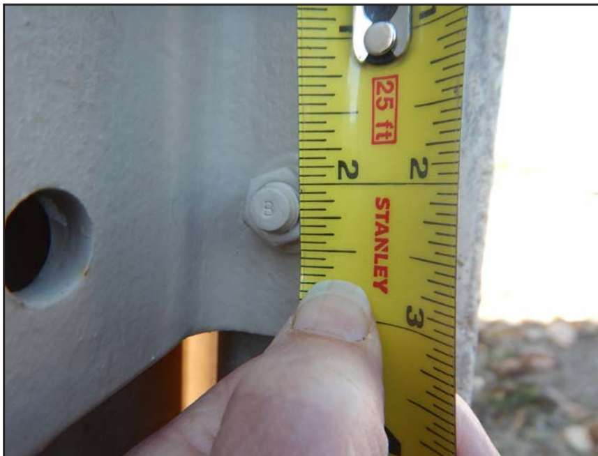
NO. 408 - COLUMN 1NE - INADEQUATE ADDED CLIP ANGLE CONNECTION AT A DEFICIENT WALL PANEL TO COLUMN CONNECTION
