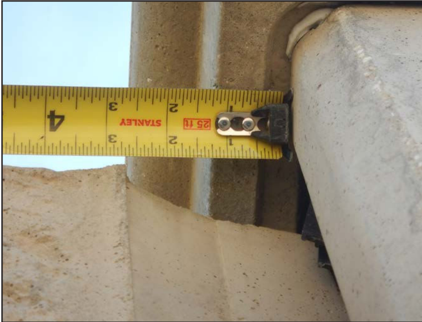
NO. 227 - COLUMN 42S - INSUFFICIENT SEATING OF A PRECAST WALL PANEL IN A PRECAST COLUMN
