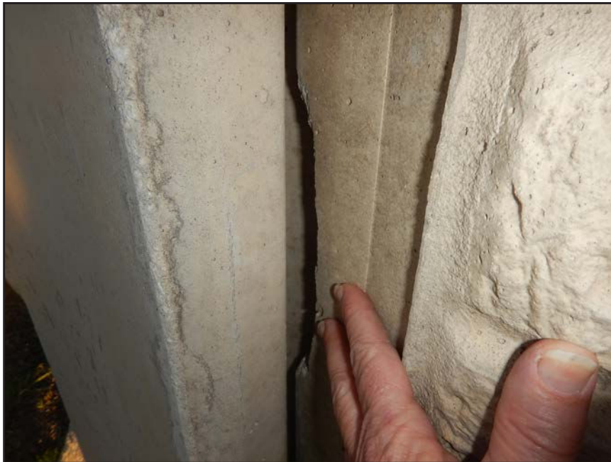
NO. 371 - COLUMN 46SS - CRACKED AND FAILED TONGUE OF A PRECAST WALL PANEL IN A PRECAST COLUMN
