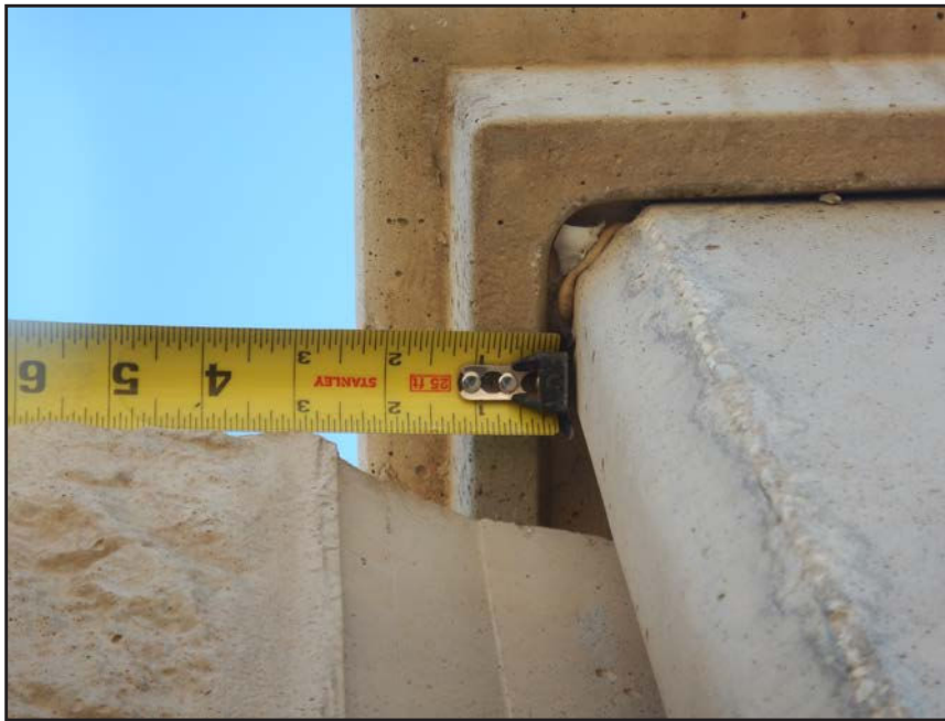
NO. 229 - COLUMN 47S - INSUFFICIENT SEATING OF A PRECAST WALL PANEL IN A PRECAST COLUMN
