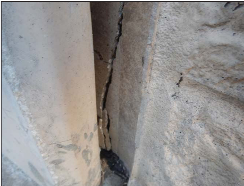
NO. 392 - COLUMN 69SS - CRACKED AND FAILED TONGUE OF A PRECAST WALL PANEL IN A PRECAST COLUMN
