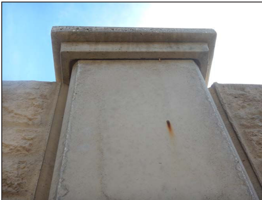
NO. 499 - COLUMN 6S - EXPOSED REINFORCING STEEL WITH INADEQUATE CONCRETE COVER
