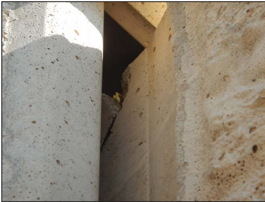
NO. 324 - COLUMN 25S - CRACKED AND FAILED TONGUE OF A PRECAST WALL PANEL IN A PRECAST COLUMN
