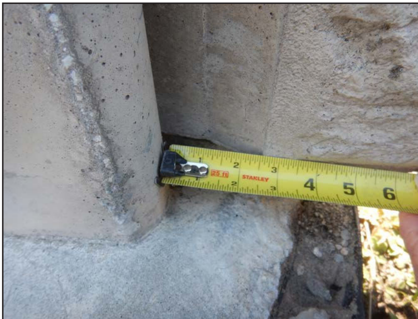
NO. 209 - COLUMN 8SM - INSUFFICIENT SEATING OF A PRECAST WALL PANEL IN A PRECAST COLUMN
