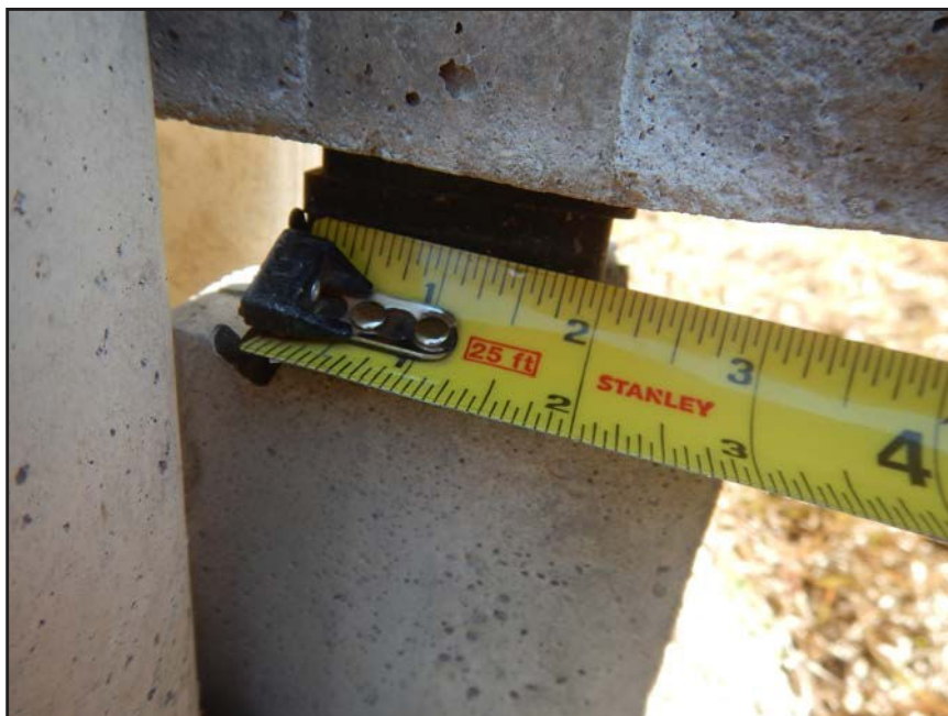
NO. 92 - COLUMN 33S - INADEQUATE BEARING OF A PRECAST WALL PANEL ON A 2" x 2" NEOPRENE BEARING PAD
