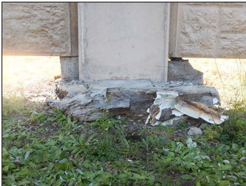
NO. 71 - COLUMN 10NM - INADEQUATE BEARING OF A PRECAST WALL PANEL ON A 2" x 2" NEOPRENE BEARING PAD
