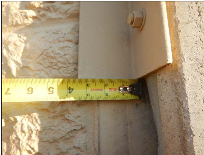
NO. 452 - COLUMN 41SS - INADEQUATE ADDED CLIP ANGLE CONNECTION AT A DEFICIENT WALL PANEL TO COLUMN CONNECTION
