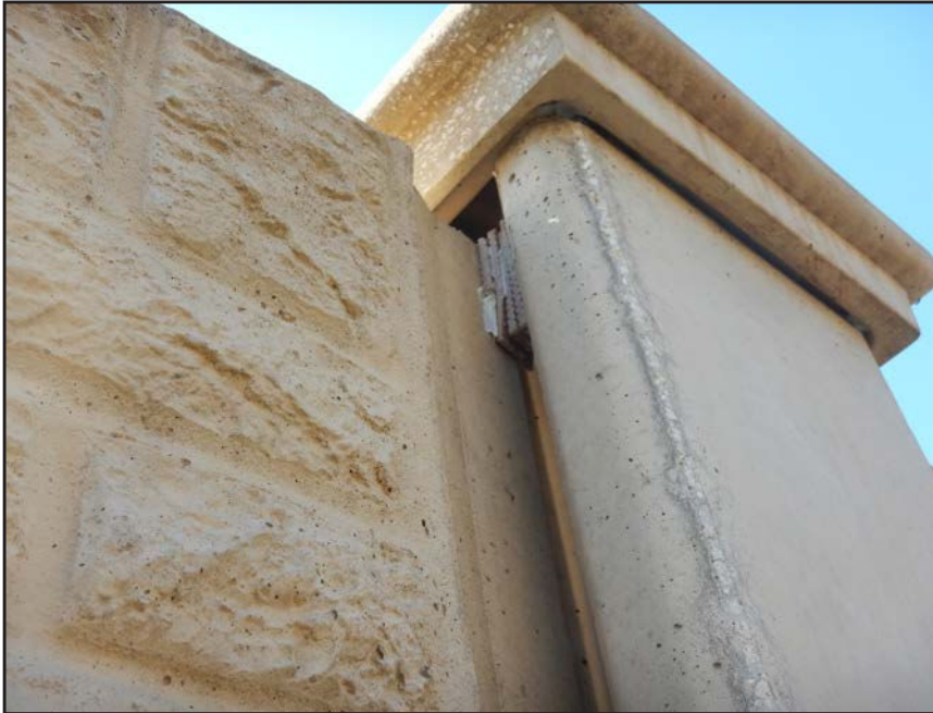
NO. 265 - COLUMN 7NM - INADEQUATE SHIMS STABILIZING A WALL PANEL TO COLUMN CONNECTION AT EXCESSIVE PLAY BETWEEN ADJACENT MEMBERS
