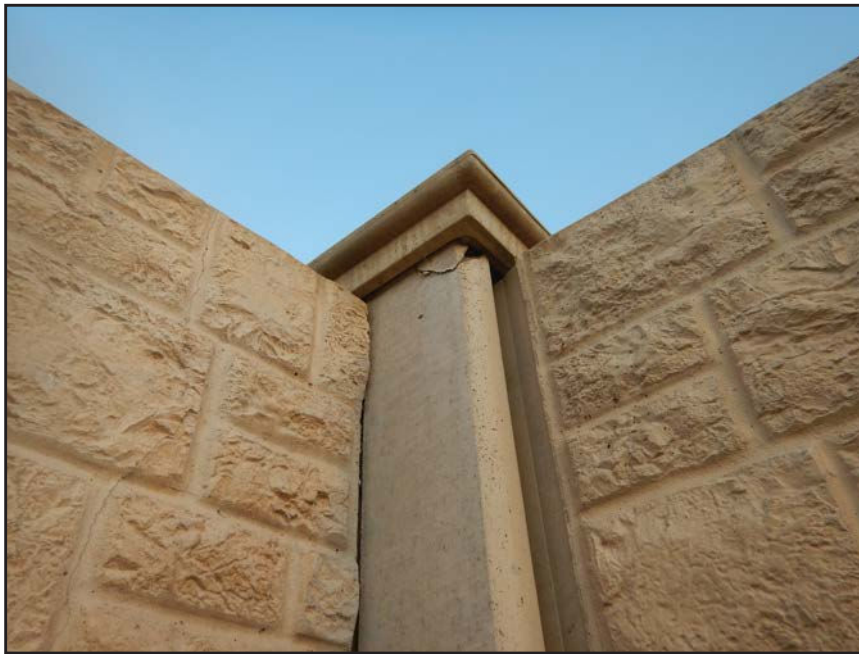
NO. 488 - COLUMN 68SS (BACK) - CRACKED AND SPALLED PRECAST CONCRETE
