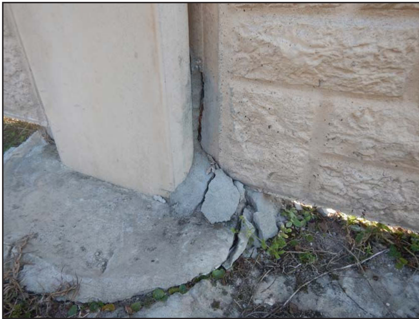
NO. 136 - COLUMN 61S - INADEQUATE BEARING OF A PRECAST WALL PANEL ON A FAILED GROUT PEDESTAL OR A FAILED PRECAST TONGUE
