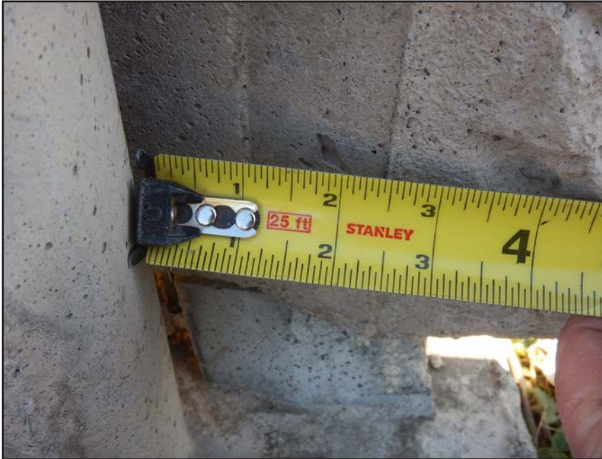
NO. 238 - COLUMN 75S - INSUFFICIENT SEATING OF A PRECAST WALL PANEL IN A PRECAST COLUMN
