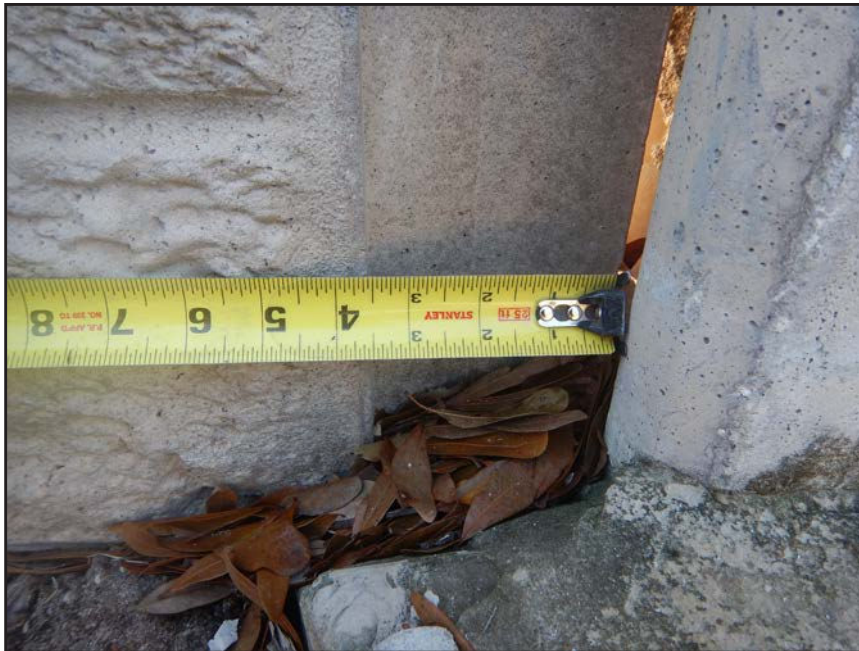
NO. 200 - COLUMN 2NM - INSUFFICIENT SEATING OF A PRECAST WALL PANEL IN A PRECAST COLUMN
