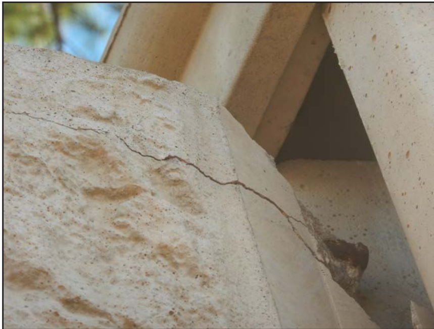
NO. 357 - COLUMN 25SS - CRACKED AND FAILED TONGUE OF A PRECAST WALL PANEL IN A PRECAST COLUMN
