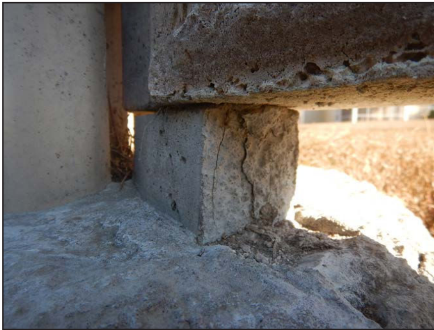
NO. 154 - COLUMN 80S - INADEQUATE BEARING OF A PRECAST WALL PANEL ON A FAILED GROUT PEDESTAL OR A FAILED PRECAST TONGUE
