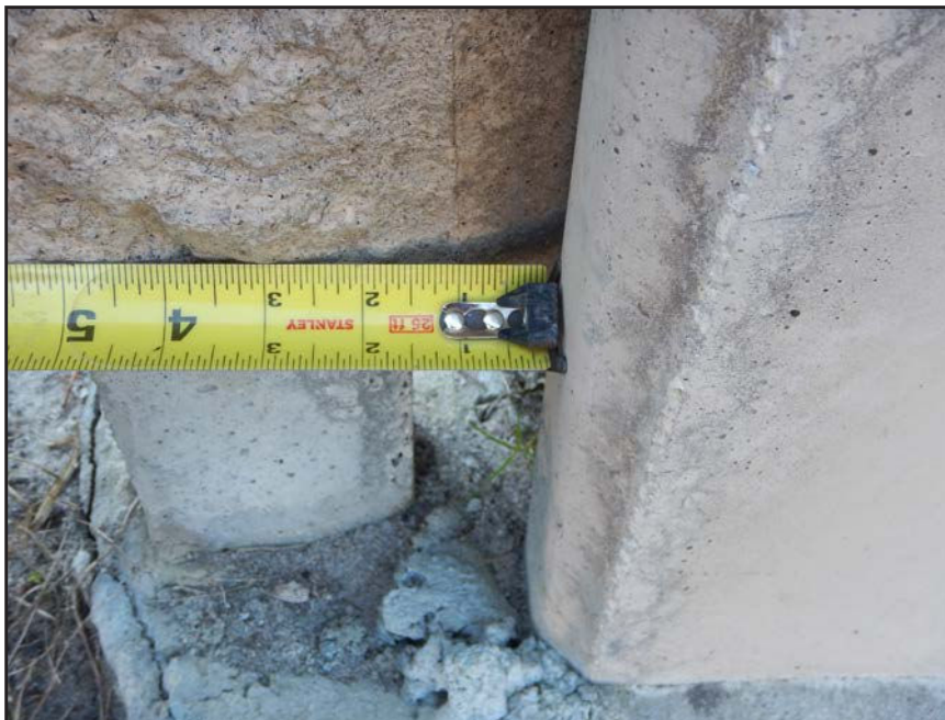
NO. 11 - COLUMN 14NM - DROPPED PRECAST PANEL WITH A 2 7/8" GAP AT THE TOP AND A 1" GAP AT THE BOTTOM
