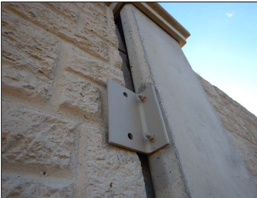
NO. 421 - COLUMN 14N - INADEQUATE ADDED CLIP ANGLE CONNECTION AT A DEFICIENT WALL PANEL TO COLUMN CONNECTION
