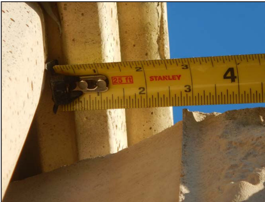
NO. 250 - COLUMN 27SS - INSUFFICIENT SEATING OF A PRECAST WALL PANEL IN A PRECAST COLUMN
