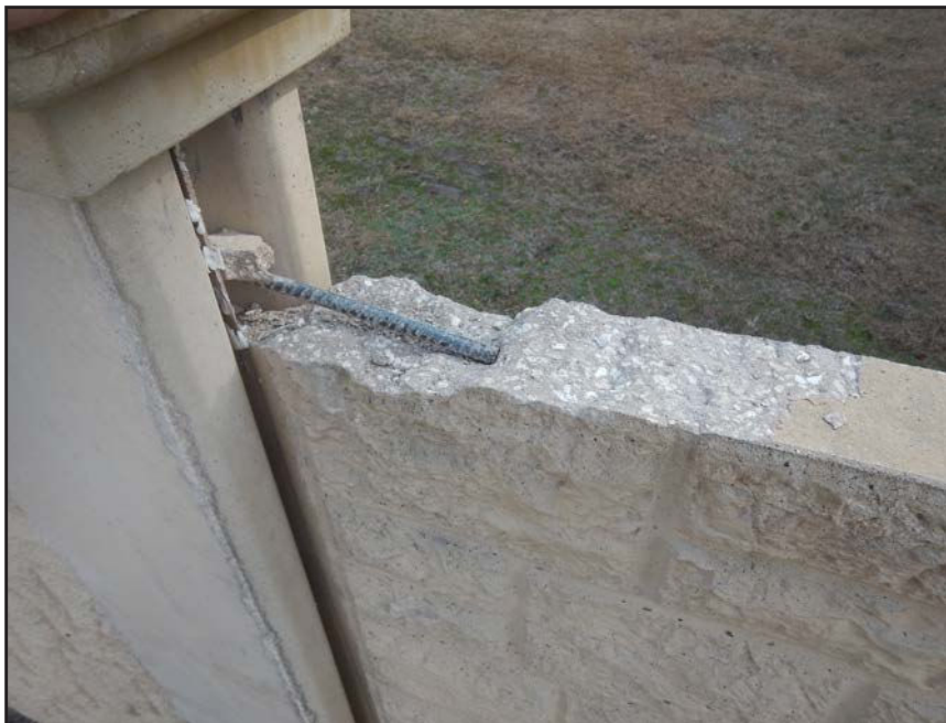
NO. 53 - SPALLED WALL PANEL ON THE SOUTH SIDE OF COLUMN 13NM - TONGUE REINFORCING DOWEL WITH INADEQUATE CONCRETE COVER
