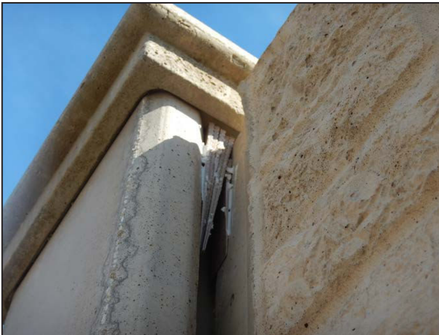
NO. 280 - COLUMN 42S - INADEQUATE SHIMS STABILIZING A WALL PANEL TO COLUMN CONNECTION AT EXCESSIVE PLAY BETWEEN ADJACENT MEMBERS
