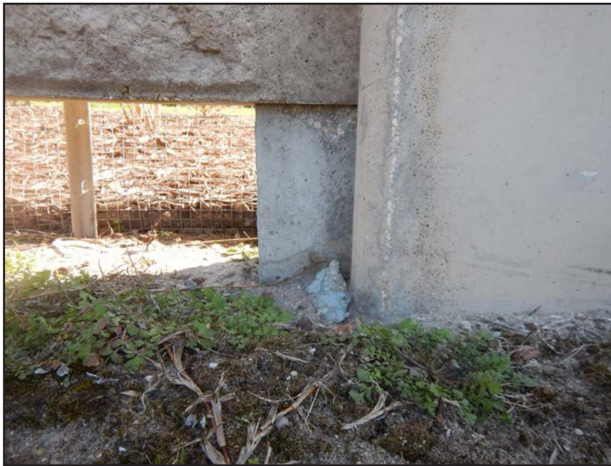
NO. 131 - COLUMN 42S - INADEQUATE BEARING OF A PRECAST WALL PANEL ON A FAILED GROUT PEDESTAL OR A FAILED PRECAST TONGUE
