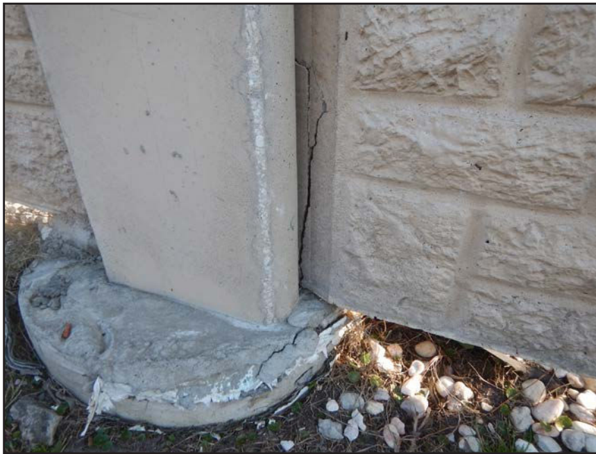
NO. 334 - COLUMN 67S - CRACKED AND FAILED TONGUE OF A PRECAST WALL PANEL IN A PRECAST COLUMN
