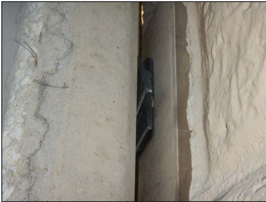
NO. 284 - COLUMN 59S - INADEQUATE SHIMS STABILIZING A WALL PANEL TO COLUMN CONNECTION AT EXCESSIVE PLAY BETWEEN ADJACENT MEMBERS
