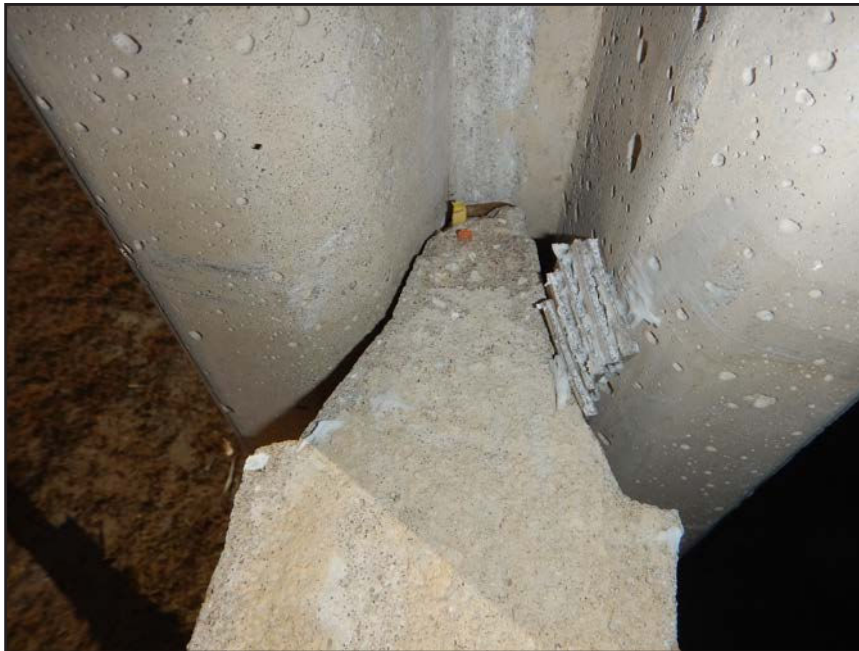
NO. 263 - COLUMN 22N - INADEQUATE SHIMS STABILIZING A WALL PANEL TO COLUMN CONNECTION AT EXCESSIVE PLAY BETWEEN ADJACENT MEMBERS
