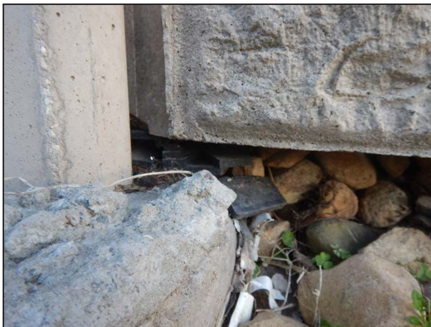
NO. 98 - COLUMN 64SS - INADEQUATE BEARING OF A PRECAST WALL PANEL ON A 2" x 2" NEOPRENE BEARING PAD
