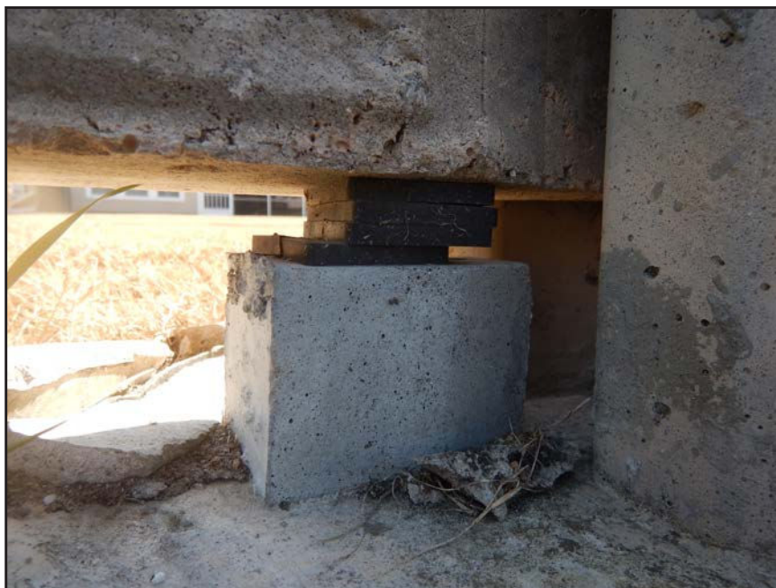
NO. 95 - COLUMN 46S - INADEQUATE BEARING OF A PRECAST WALL PANEL ON A 2" x 2" NEOPRENE BEARING PAD
