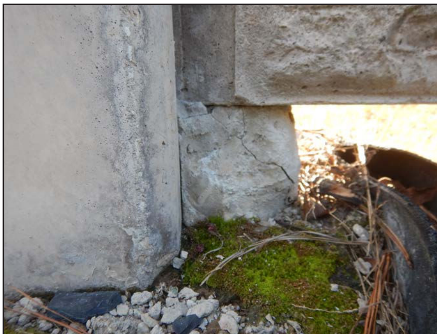
NO. 120 - COLUMN 25SM - INADEQUATE BEARING OF A PRECAST WALL PANEL ON A FAILED GROUT PEDESTAL OR A FAILED PRECAST TONGUE
