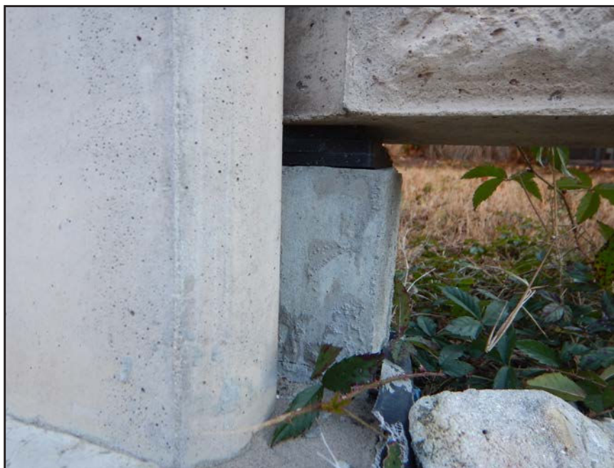
NO. 68 - COLUMN 11N - INADEQUATE BEARING OF A PRECAST WALL PANEL ON A 2" x 2" NEOPRENE BEARING PAD
