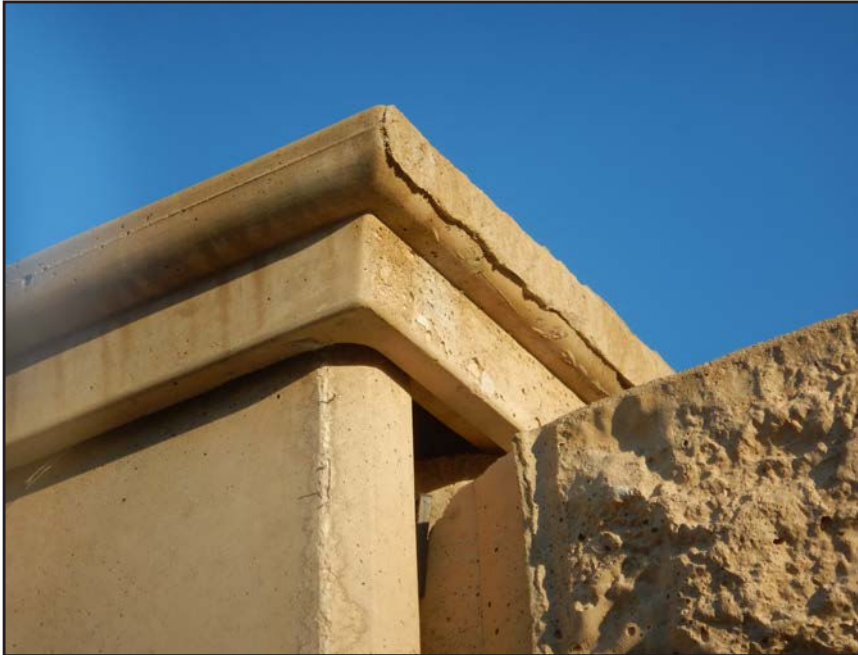
NO. 368 - COLUMN 46SS - CRACKED AND FAILED TONGUE OF A PRECAST WALL PANEL IN A PRECAST COLUMN
