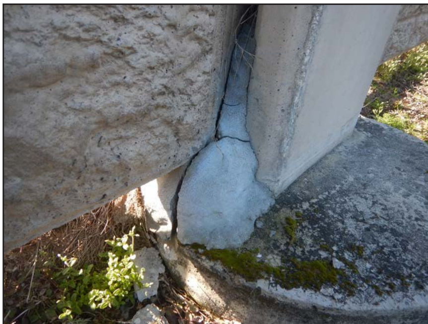
NO. 113 - COLUMN 45N - INADEQUATE BEARING OF A PRECAST WALL PANEL ON A FAILED GROUT PEDESTAL OR A FAILED PRECAST TONGUE
