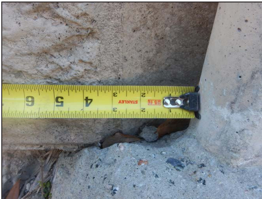
NO. 197 - COLUMN 57N - INSUFFICIENT SEATING OF A PRECAST WALL PANEL IN A PRECAST COLUMN
