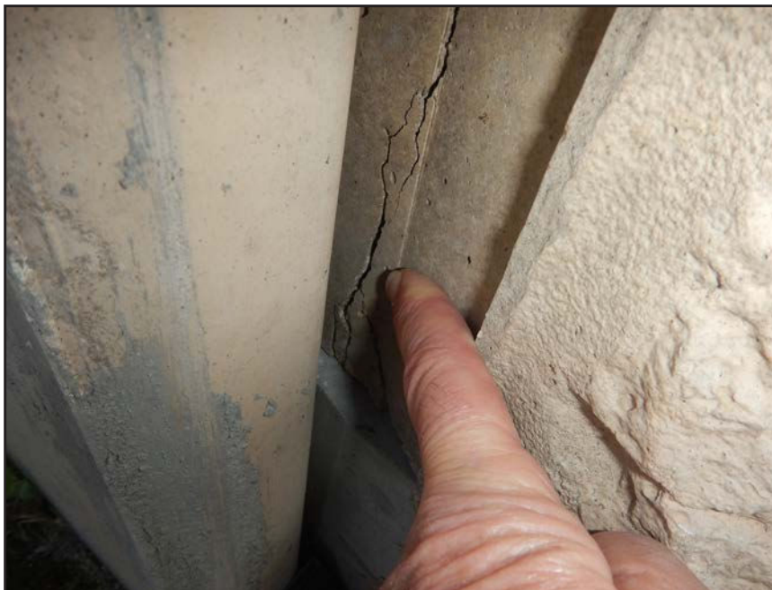
NO. 323 - COLUMN 19S - CRACKED AND FAILED TONGUE OF A PRECAST WALL PANEL IN A PRECAST COLUMN
