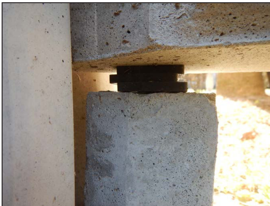
NO. 87 - COLUMN 22SM - INADEQUATE BEARING OF A PRECAST WALL PANEL ON A 2" x 2" NEOPRENE BEARING PAD
