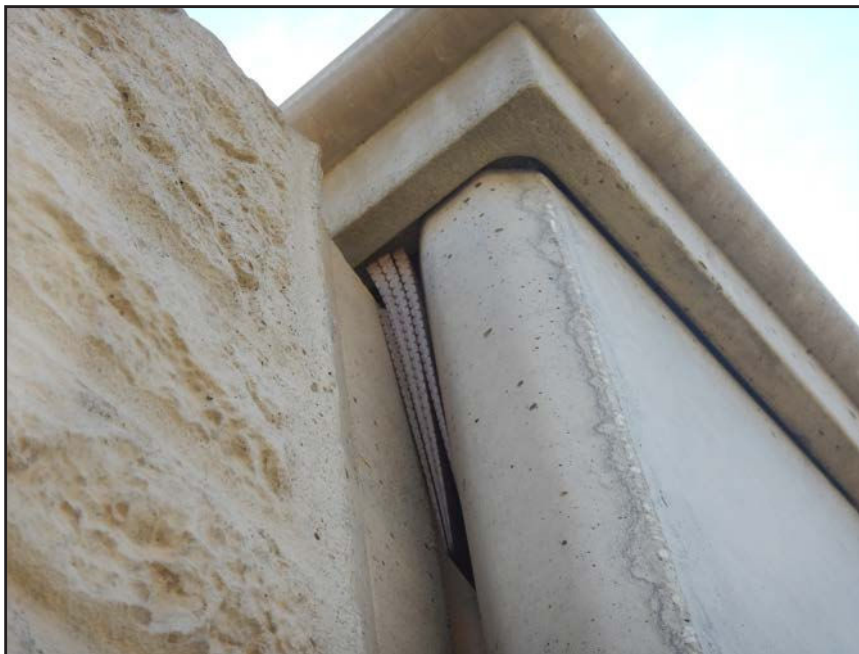
NO. 278 - COLUMN 34S - INADEQUATE SHIMS STABILIZING A WALL PANEL TO COLUMN CONNECTION AT EXCESSIVE PLAY BETWEEN ADJACENT MEMBERS
