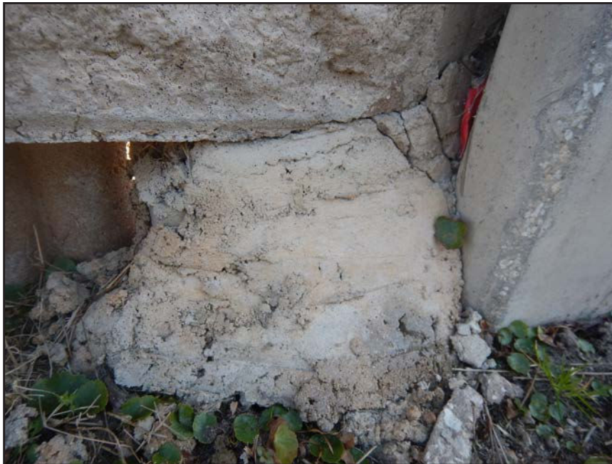
NO. 152 - COLUMN 78S - INADEQUATE BEARING OF A PRECAST WALL PANEL ON A FAILED GROUT PEDESTAL OR A FAILED PRECAST TONGUE
