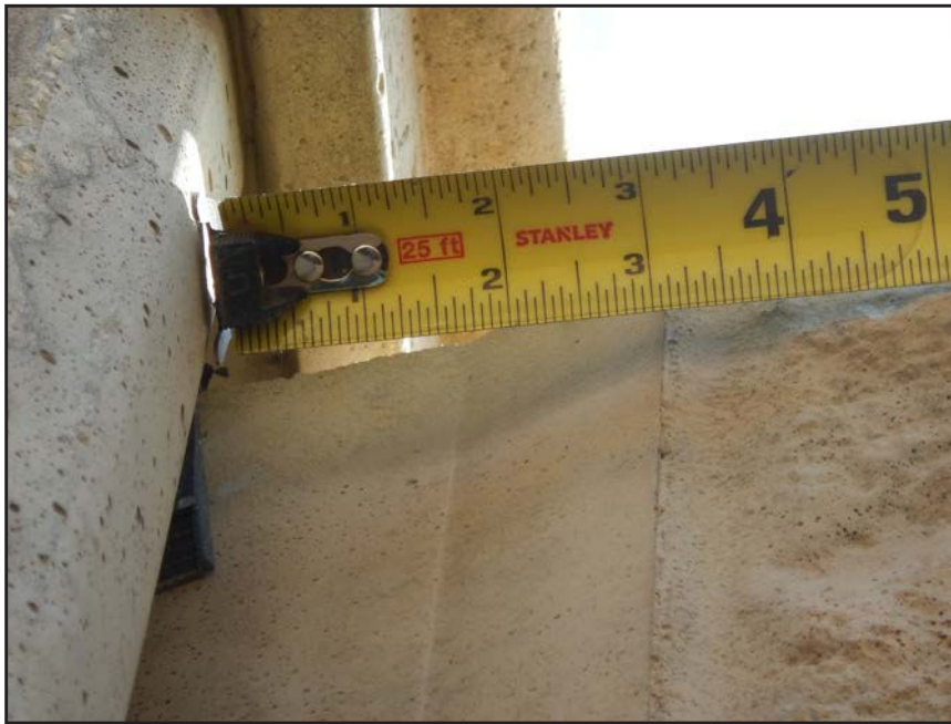
NO. 213 - COLUMN 4S - INSUFFICIENT SEATING OF A PRECAST WALL PANEL IN A PRECAST COLUMN
