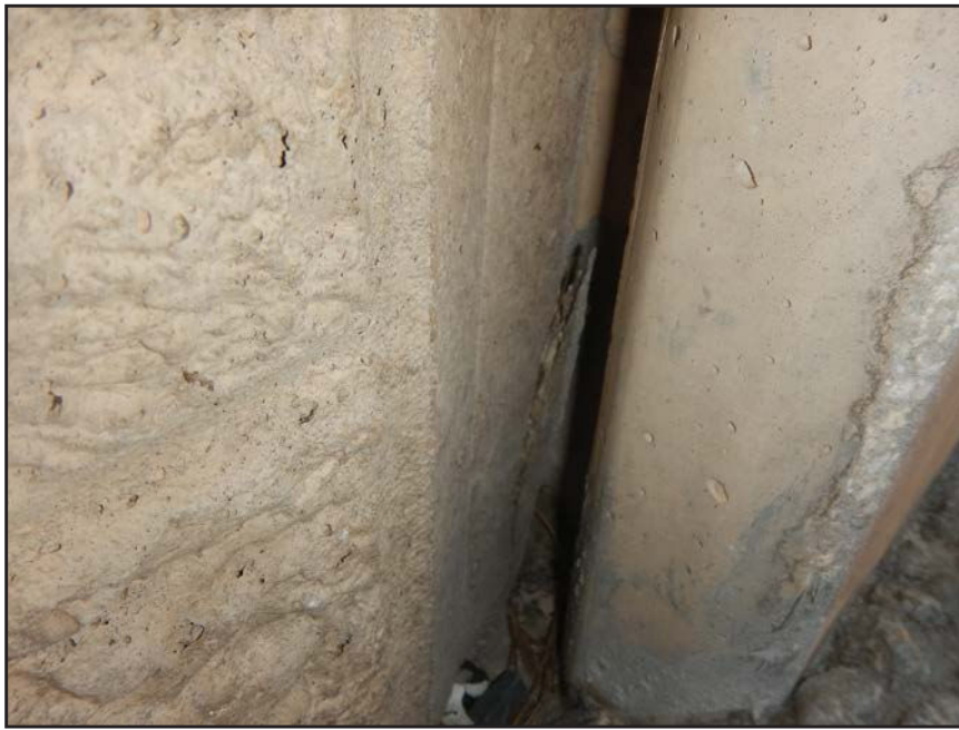
NO. 381 - COLUMN 59SS - CRACKED AND FAILED TONGUE OF A PRECAST WALL PANEL IN A PRECAST COLUMN
