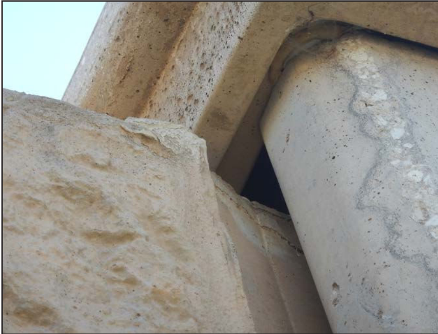
NO. 327 - COLUMN 54S - CRACKED AND FAILED TONGUE OF A PRECAST WALL PANEL IN A PRECAST COLUMN
