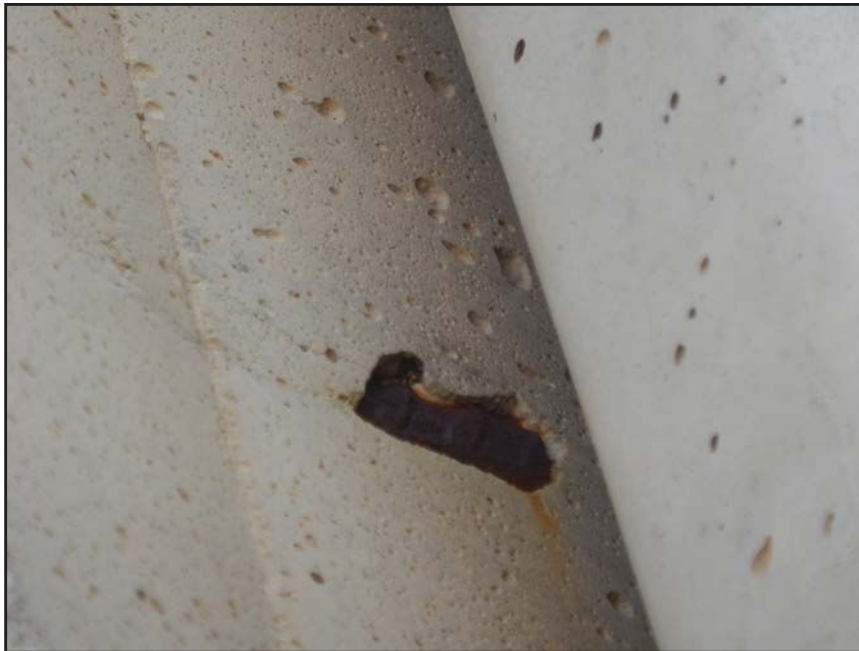
NO. 501 - COLUMN 48S - EXPOSED REINFORCING STEEL WITH INADEQUATE CONCRETE COVER
