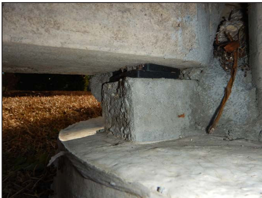
NO. 64 - COLUMN 2N - INADEQUATE BEARING OF A PRECAST WALL PANEL ON A 2" x 2" NEOPRENE BEARING PAD
