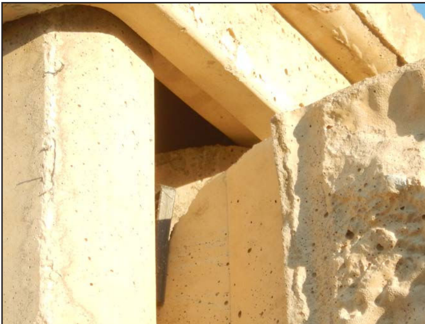
NO. 369 - COLUMN 46SS - CRACKED AND FAILED TONGUE OF A PRECAST WALL PANEL IN A PRECAST COLUMN
