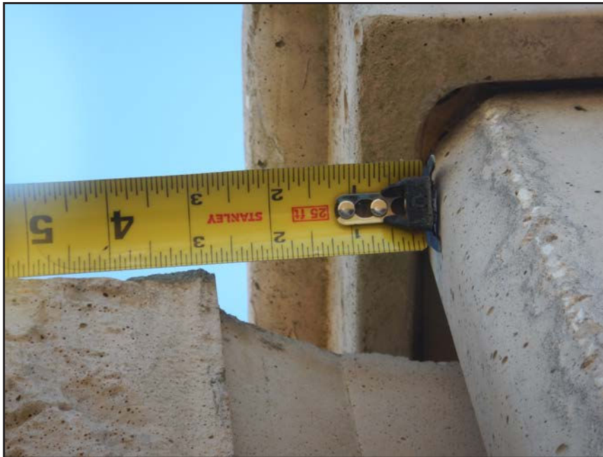
NO. 233 - COLUMN 63S - INSUFFICIENT SEATING OF A PRECAST WALL PANEL IN A PRECAST COLUMN
