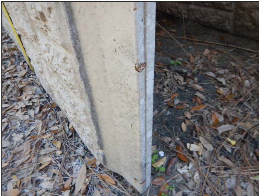
NO. 37 - STORED EXCESS WALL PANEL - TONGUE REINFORCING STEEL WITH INADEQUATE CONCRETE COVER
