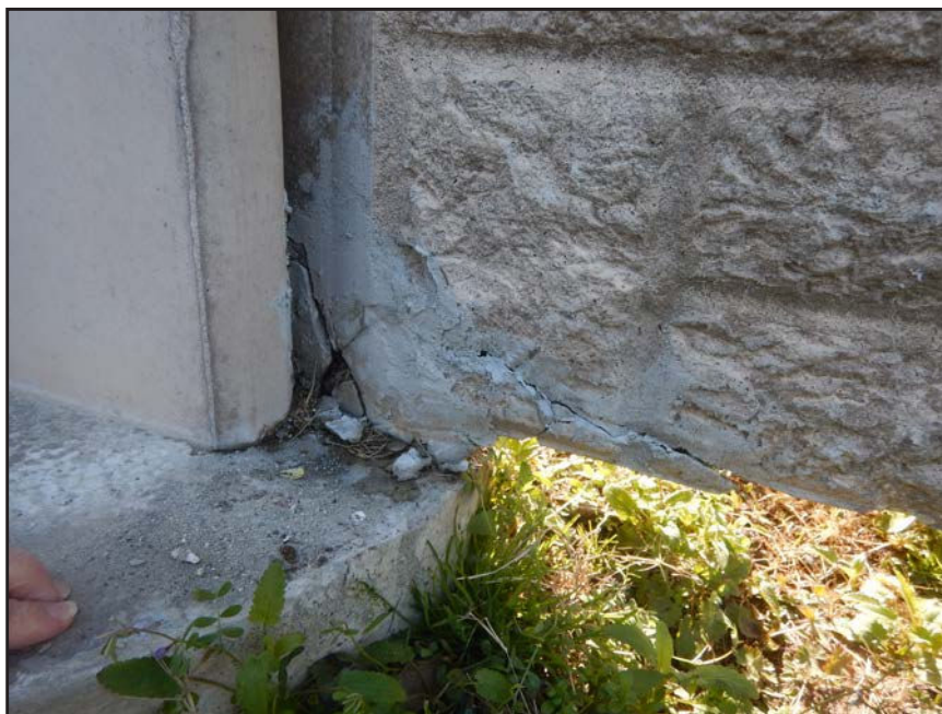
NO. 110 - COLUMN 43N - INADEQUATE BEARING OF A PRECAST WALL PANEL ON A FAILED GROUT PEDESTAL OR A FAILED PRECAST TONGUE
