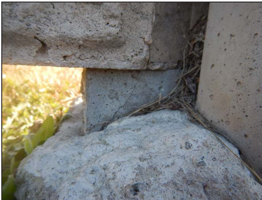
NO. 138 - COLUMN 62S - INADEQUATE BEARING OF A PRECAST WALL PANEL ON A FAILED GROUT PEDESTAL OR A FAILED PRECAST TONGUE
