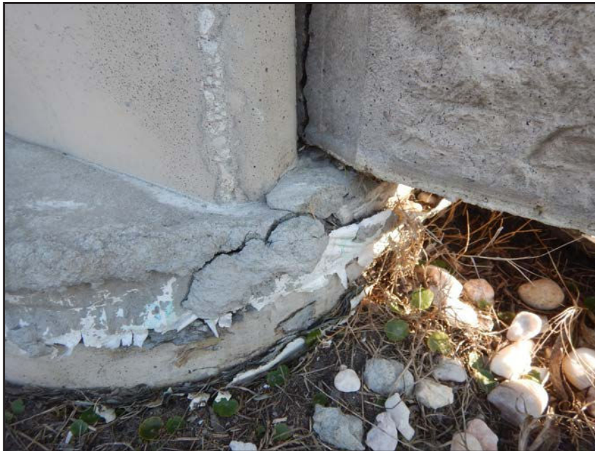
NO. 140 - COLUMN 67S - INADEQUATE BEARING OF A PRECAST WALL PANEL ON A FAILED GROUT PEDESTAL OR A FAILED PRECAST TONGUE
