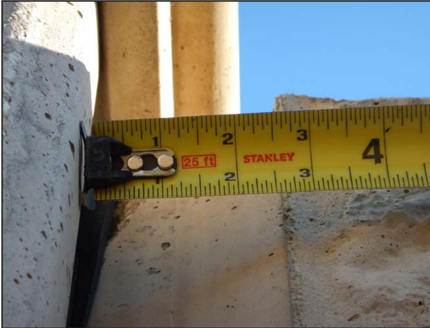
NO. 186 - COLUMN 14N - INSUFFICIENT SEATING OF A PRECAST WALL PANEL IN A PRECAST COLUMN
