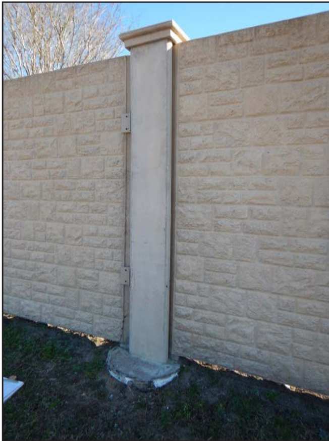
NO. 412 - COLUMN 9N - INADEQUATE ADDED CLIP ANGLE CONNECTION AT A DEFICIENT WALL PANEL TO COLUMN CONNECTION
