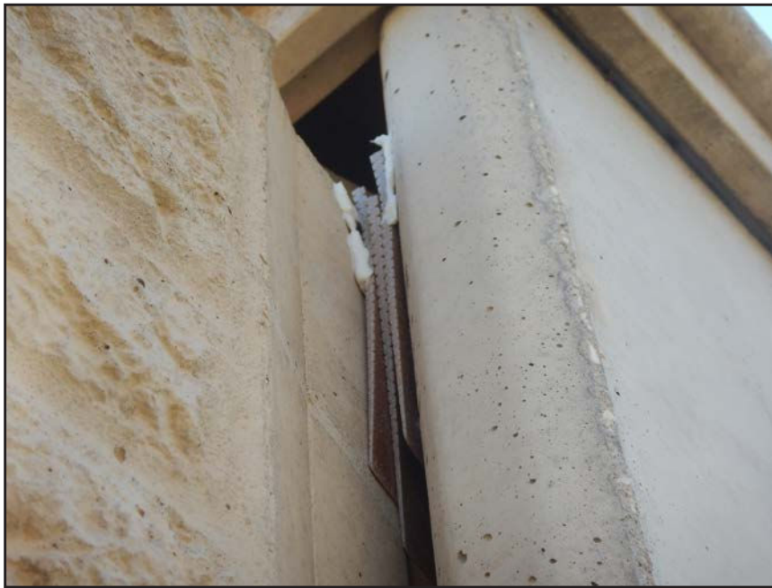
NO. 276 - COLUMN 28S - INADEQUATE SHIMS STABILIZING A WALL PANEL TO COLUMN CONNECTION AT EXCESSIVE PLAY BETWEEN ADJACENT MEMBERS
