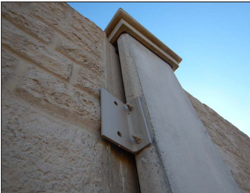
NO. 413 - COLUMN 9N - INADEQUATE ADDED CLIP ANGLE CONNECTION AT A DEFICIENT WALL PANEL TO COLUMN CONNECTION
