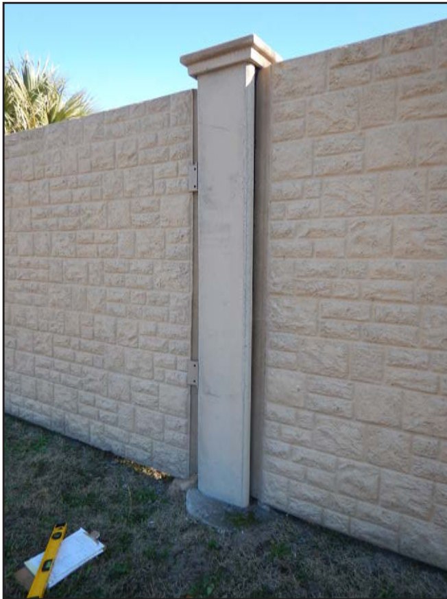
NO. 429 - COLUMN 20N - INADEQUATE ADDED CLIP ANGLE CONNECTION AT A DEFICIENT WALL PANEL TO COLUMN CONNECTION
